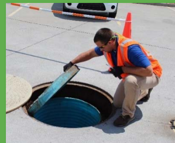
Inspecting a containment sump
