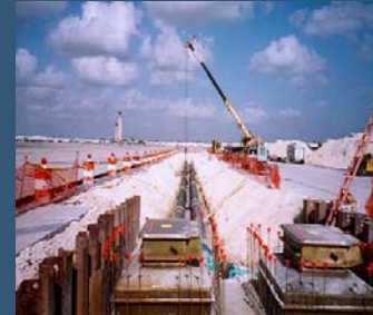
Installation of AHS piping and vaults
