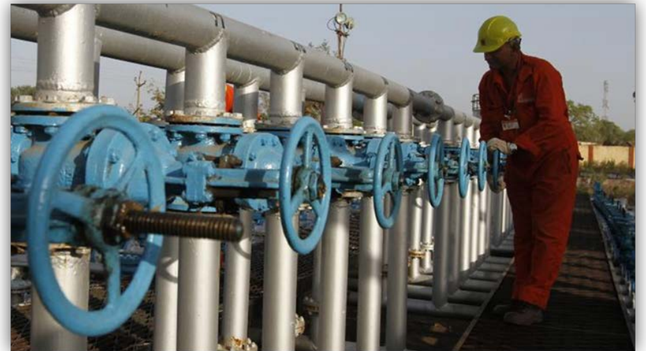
A technician opens a pressure gas valve inside the Oil and Natural Gas Corp (ONGC) group gathering station on the outskirts of the western Indian city of Ahmedabad
