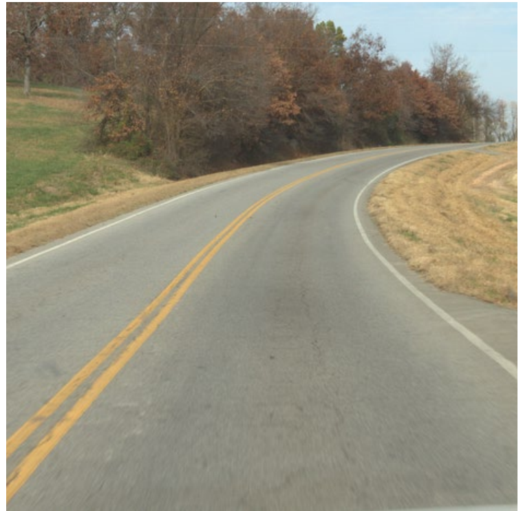
Curves and hills come with limited line of sight for drivers and prove more dangerous without shoulders, especially on two-lane highways.
