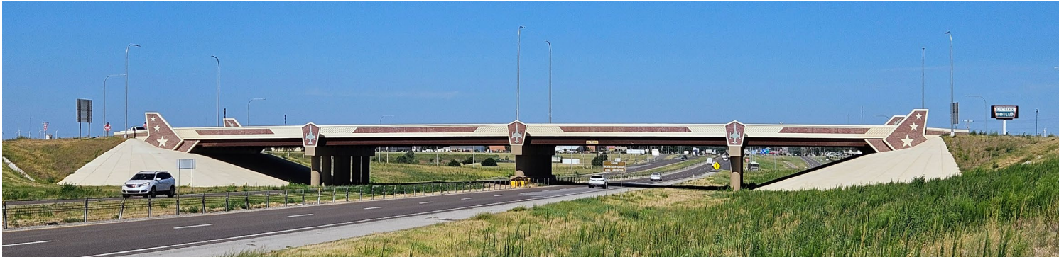
The I-40/Airport Rd. bridge in Weatherford replaced a previously functionally obsolete and at-risk of becoming structurally deficient bridge. The new five-lane configuration will improve traffic flow.
