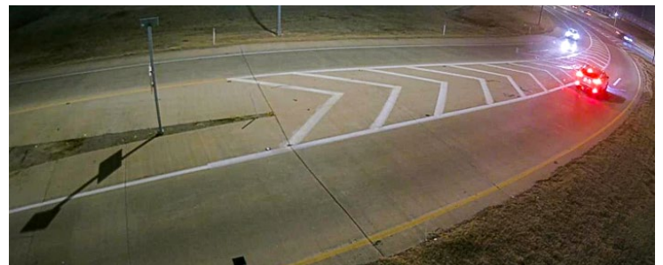
ODOT's wrong way detection technology flashes red lights (not seen from this angle) to alert drivers of their error.
