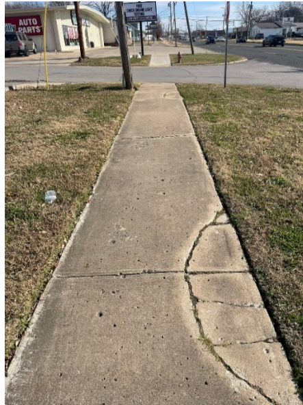
Figure 4: Deteriorated Sidewalk near Moss Avenue
