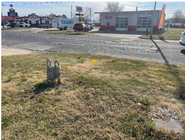
Figure 24: Gas Meter in R/W
