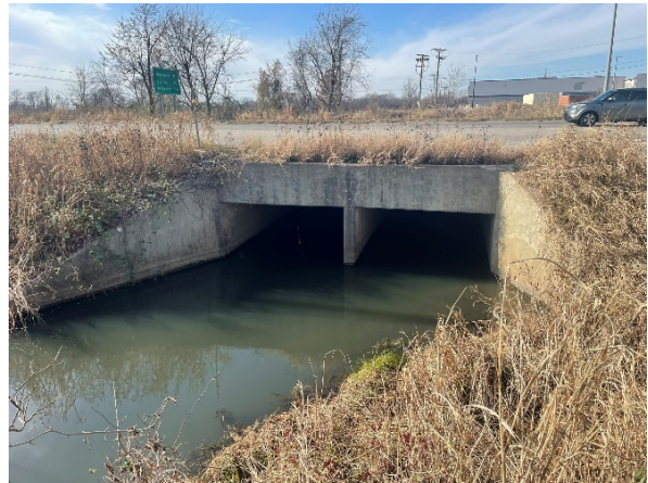
Figure 15: RCB at US-69 Creek Crossing.
