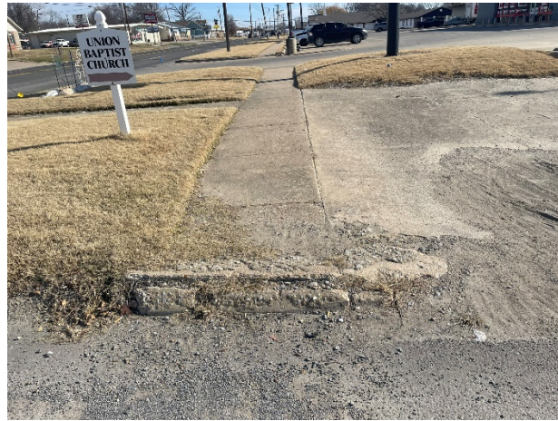
Figure 8: No ADA Ramp at Street Crossing
