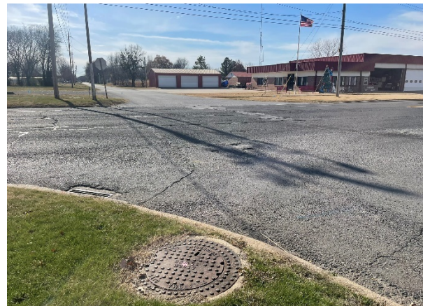
Figure 25: Storm Water Manhole in R/W
