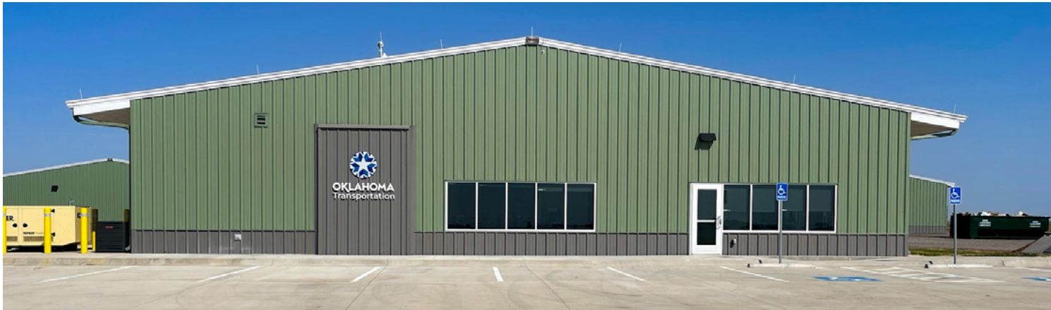
The entrance to District 4's new maintenance building.
