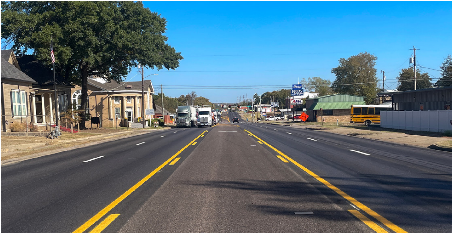
Upgrades on US-69 in the City of Atoka include resurfacing and striping.
