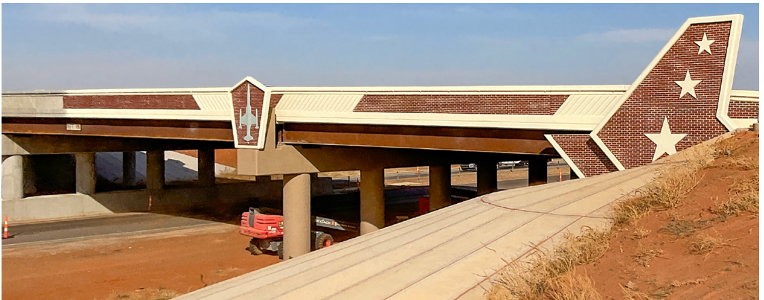
Two angles of the new Airport Road bridge over I-40 show the bridge's jet, star, and wing-shape details incorporated into the design.
