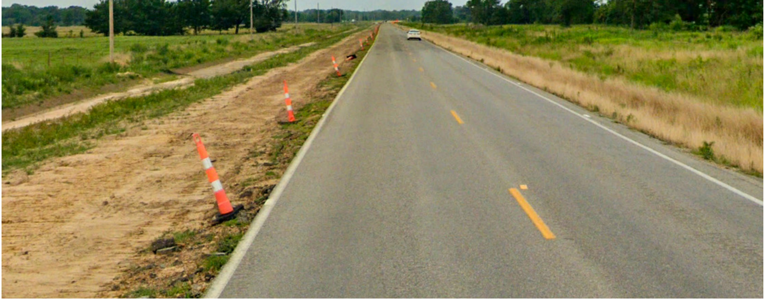
Before: SH-3 without shoulders under construction between Atoka and Antlers.
