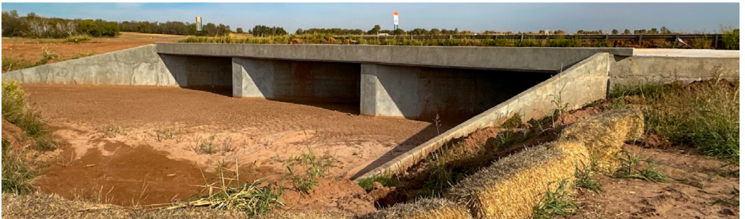
A completed box bridge on SH-19 in Grady County.
