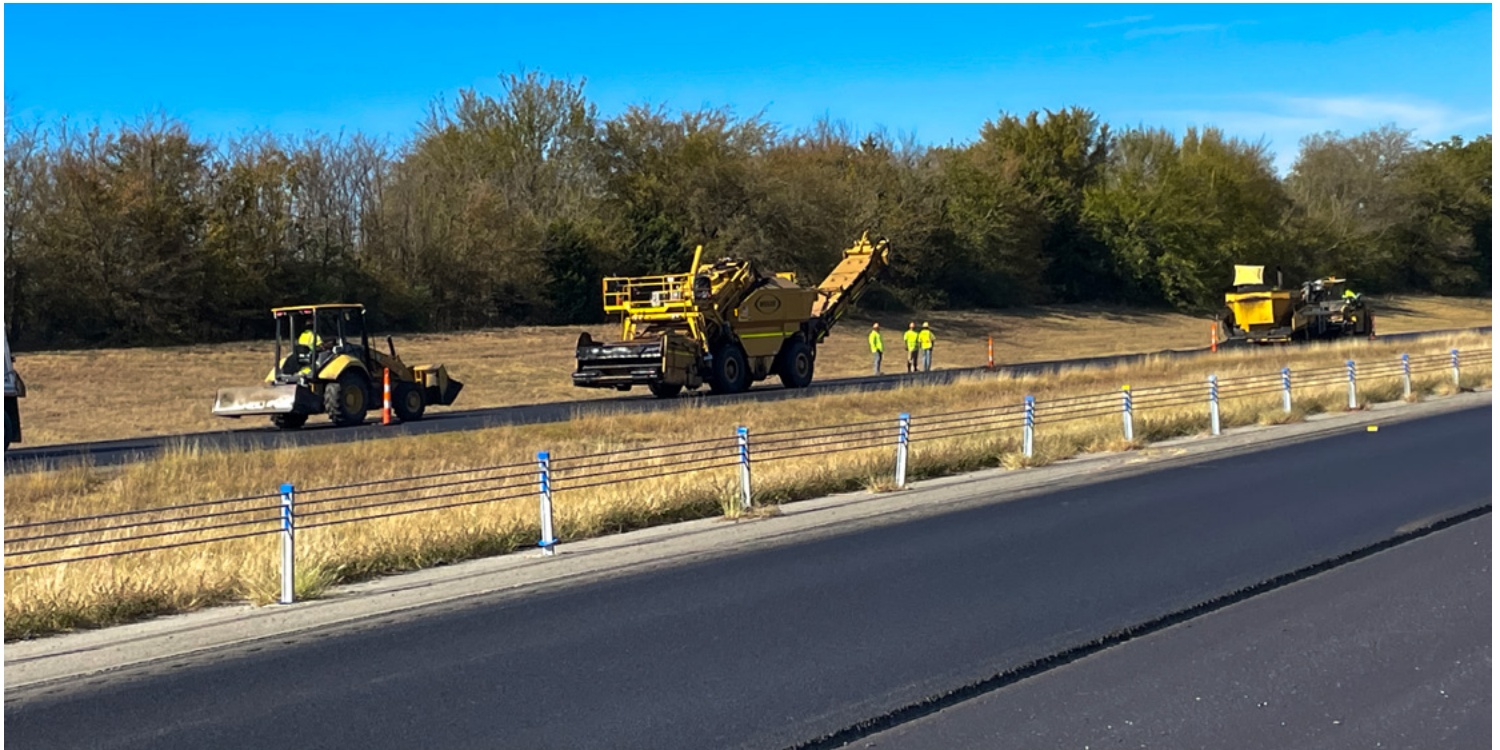
District 1 crews resurface US-69.
