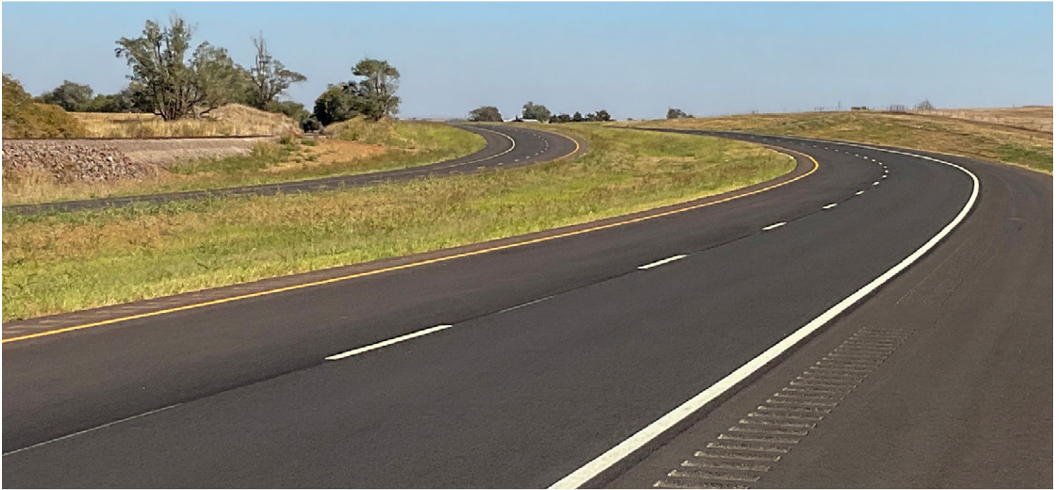
A sharp curve on rural SH-183 with limited sight distance is now safer with lanes divided by a grass median and new shoulders.
