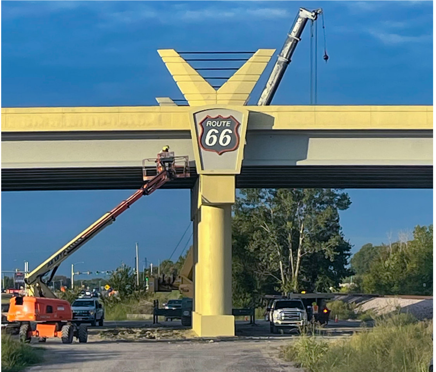
Crews work on the bridge connecting SH-20 and Route 66 in Claremore.
