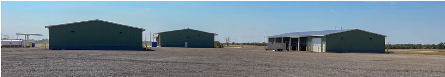
Three buildings stand on the 20-acre property, from left to right, fuel station, equipment shed with shop, maintenance building, and the equipment shed with wash bay.
