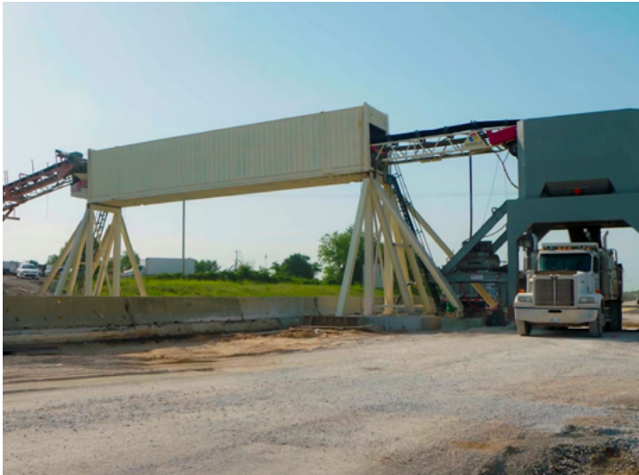
The conveyor bridge spans I-35 with a dump truck receiving material on the other side.
