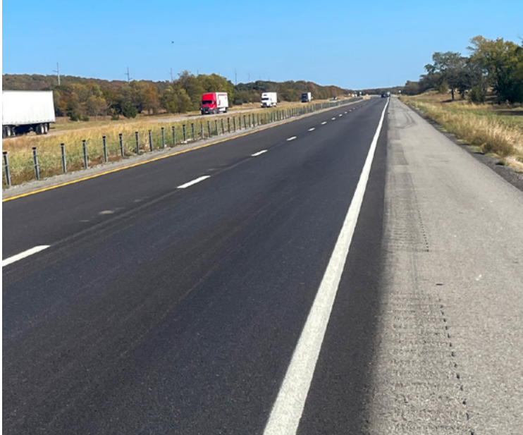
New pavement near Limestone Gap in rural Atoka County.
