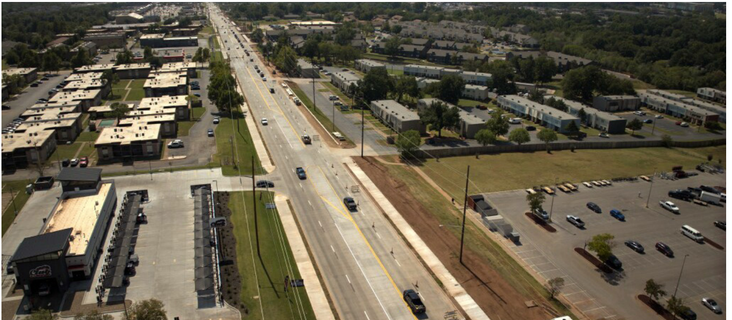
Facing South/McElroy: An aerial view of upgrades made to US-177/Perkins Road.
