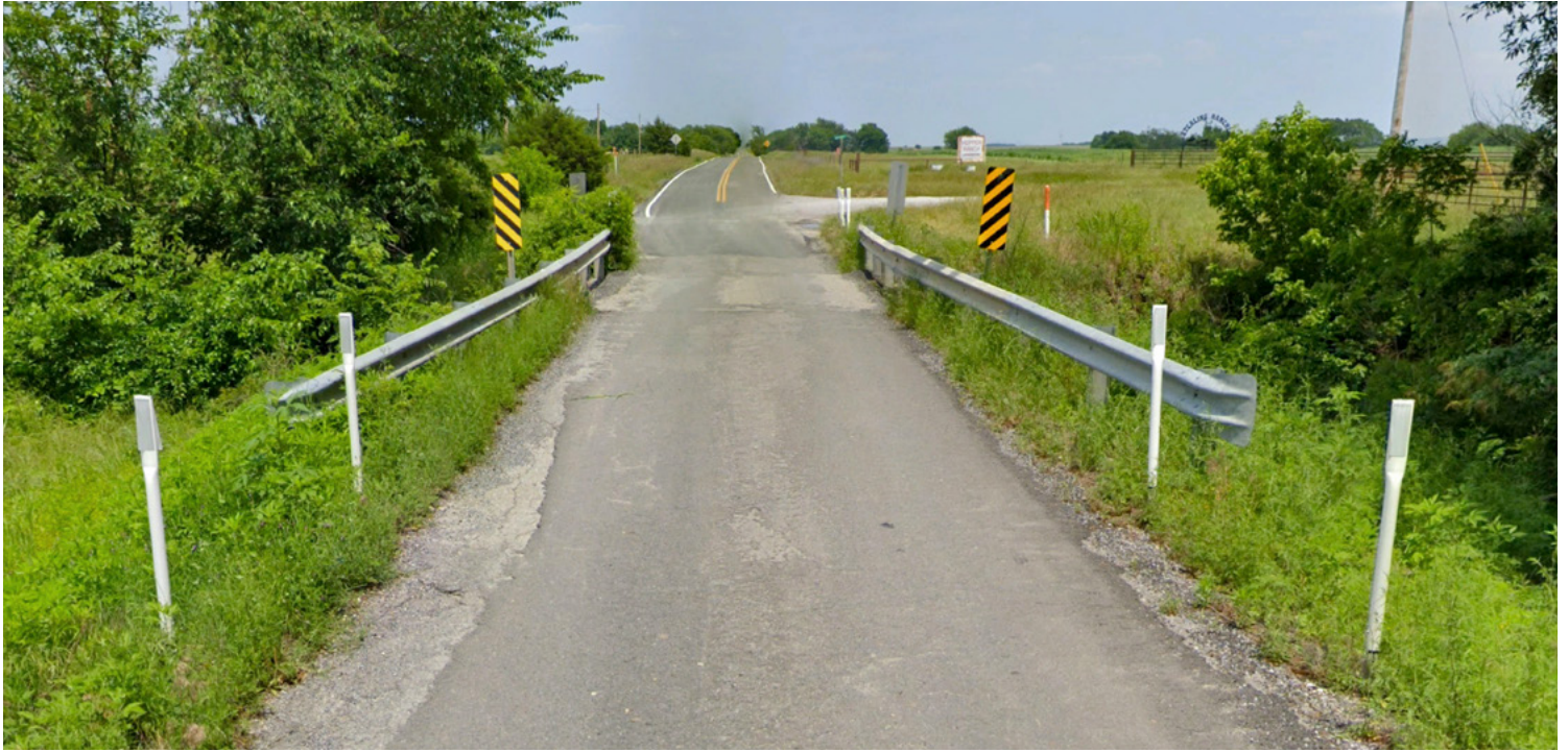
Before: single-lane bridge on SH-63 outside of Pittsburg
