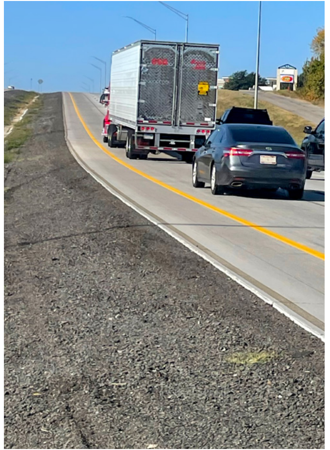
US-69 upgrades in the City of McAlester.
