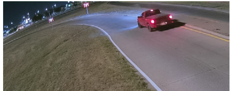
ODOT's new wrong way technology flashes red lights to alert drivers of their error.
