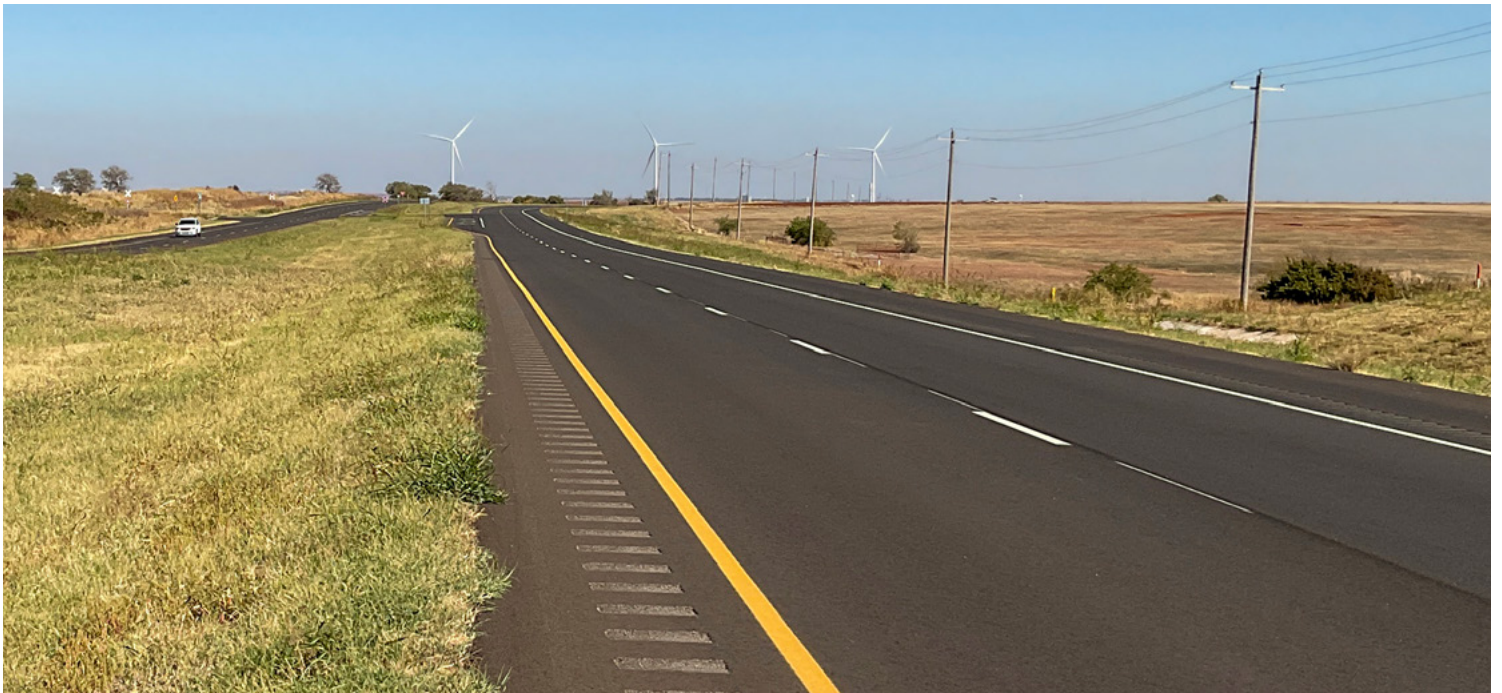
New pavement, shoulders and left turn lanes enhance US-183 between Rocky and Cordell.
