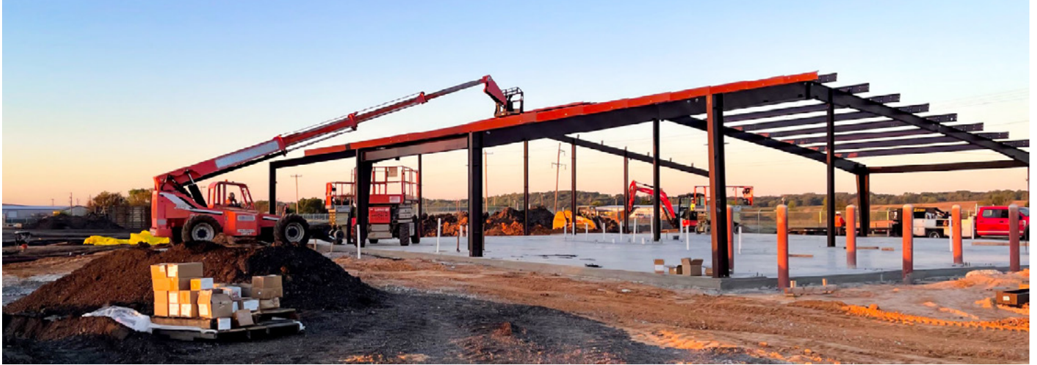
Construction continues on District 7's new facility to combine three crews.
