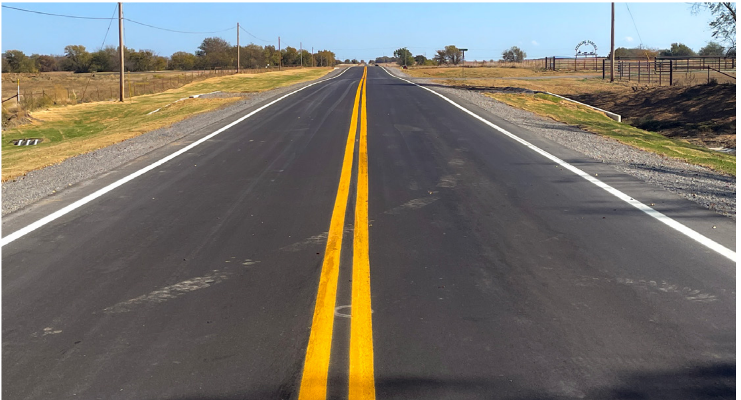
After: new wider structure and pavement on SH-63 outside of Pittsburg.
