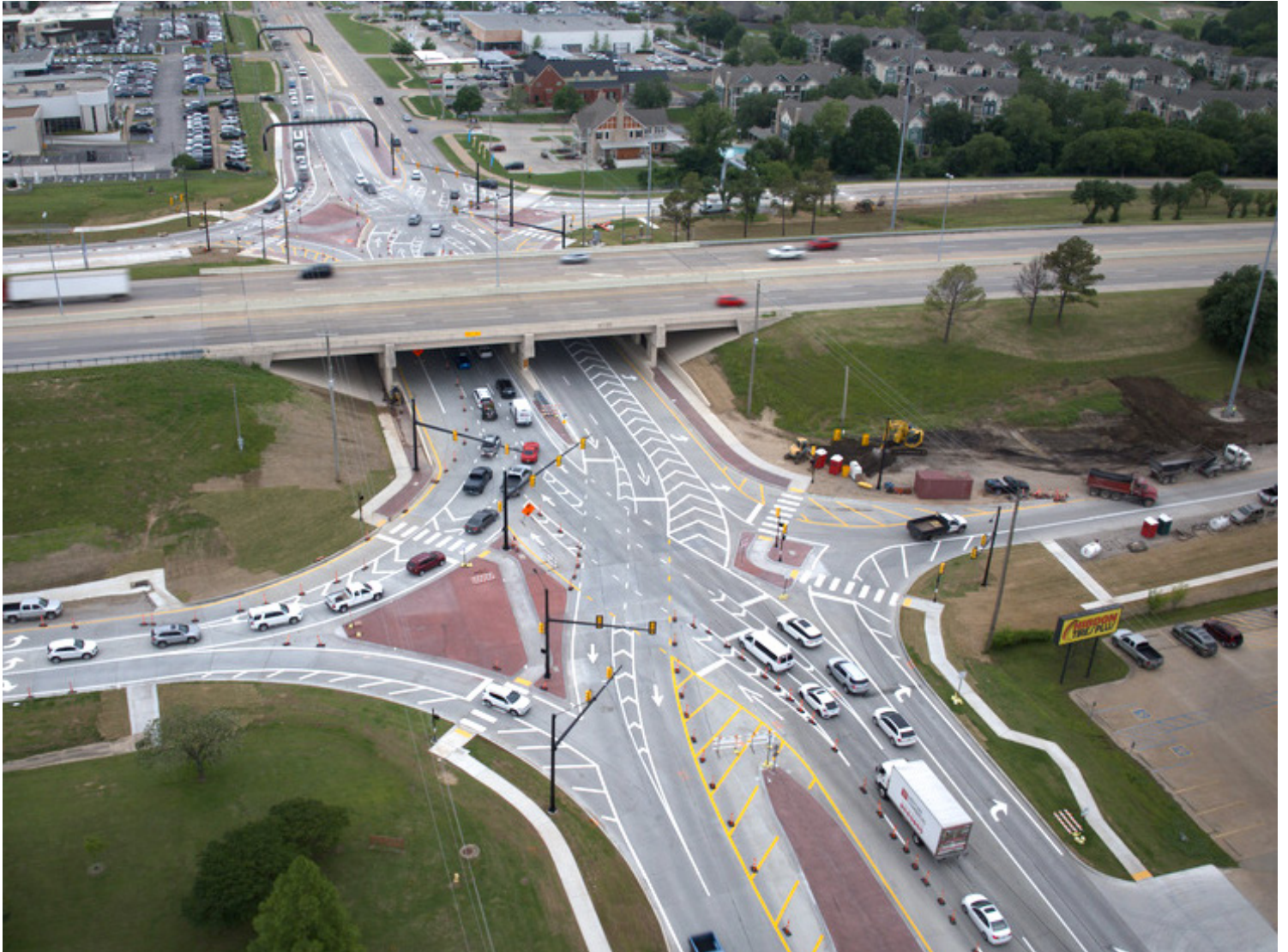
An aerial view of Tulsa traffic navigating the Memorial Road/US-169 diverging diamond interchange.
