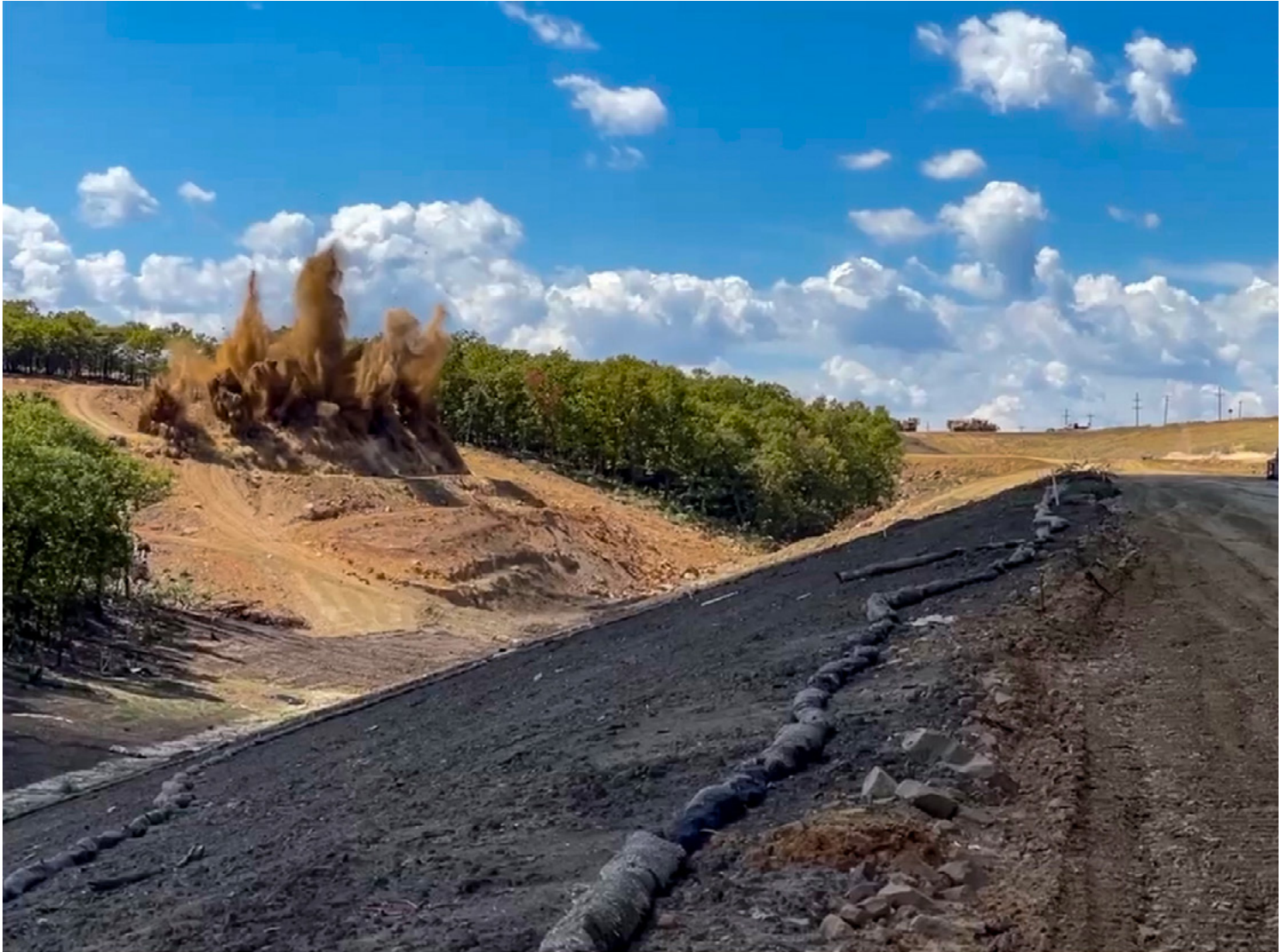
Explosives blast soil high into above the trees, during District 8's 630,000 cubic yards of rock excavation required to realign and widen a section of US-60 in Osage County.
