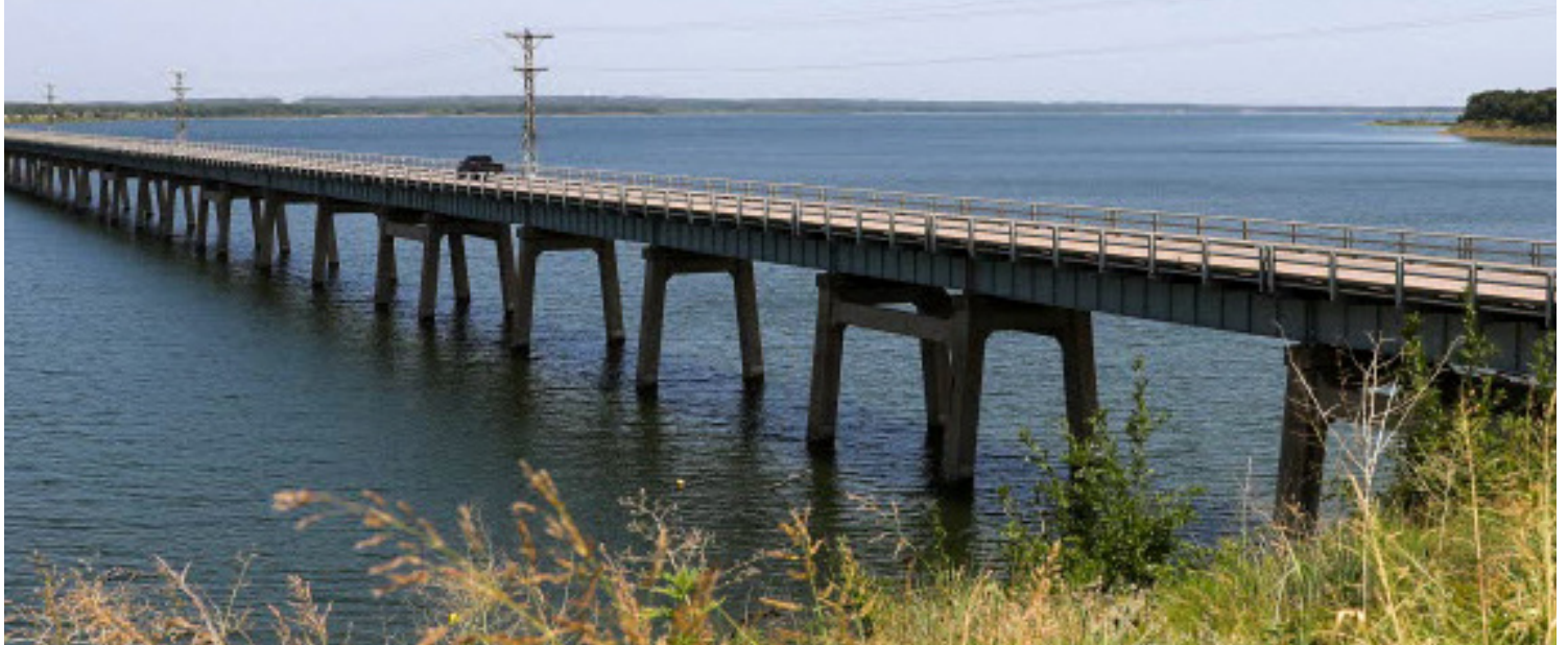
Pictured is the current Roosevelt Bridge crossing Lake Texoma.
