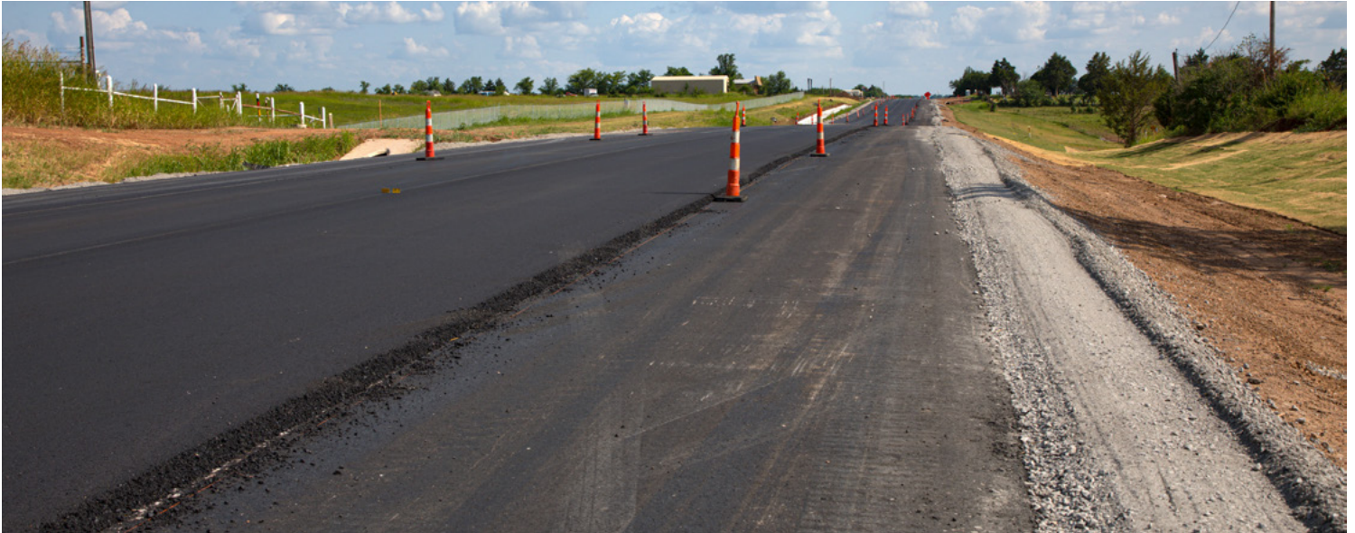
Shoulder construction in rural Oklahoma.
