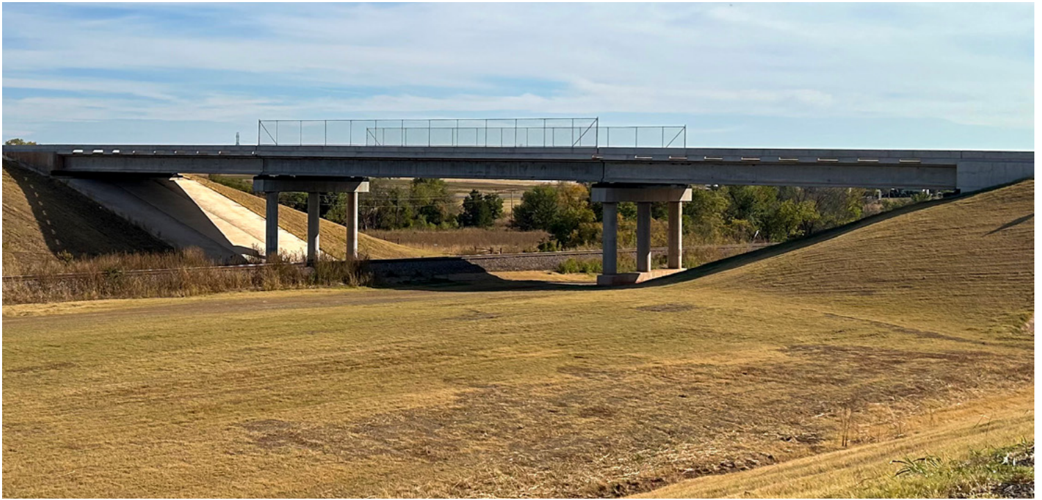
The new SH-51 bridge over the railroad in Logan County.
