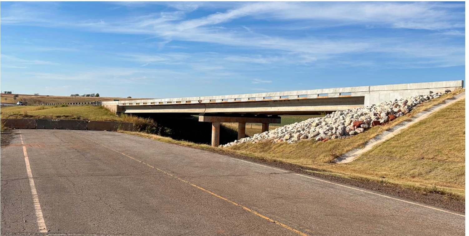
The new bridge over East Beaver Creek on SH-51 was reconfigured to straighten the previous route. Pictured is the dead end on one side of the 1-mile section with the new bridge spanning the creek in the background.
