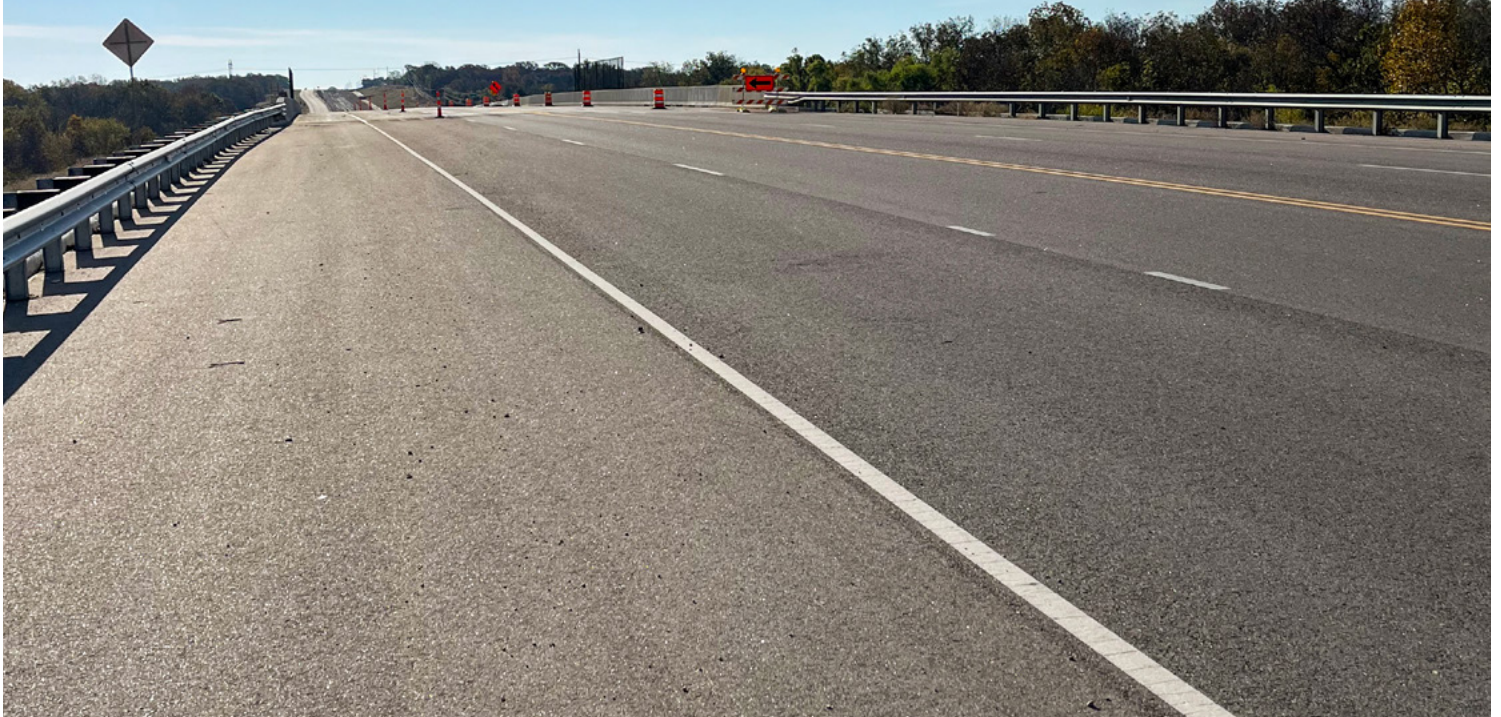
Four lanes with shoulders span a bridge on US-270 with construction continuing in the distance.
