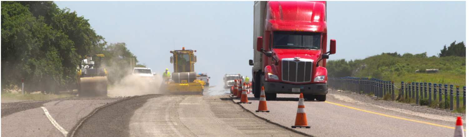
ODOT maintenance crews work to improve lane miles alongside highway traffic.
