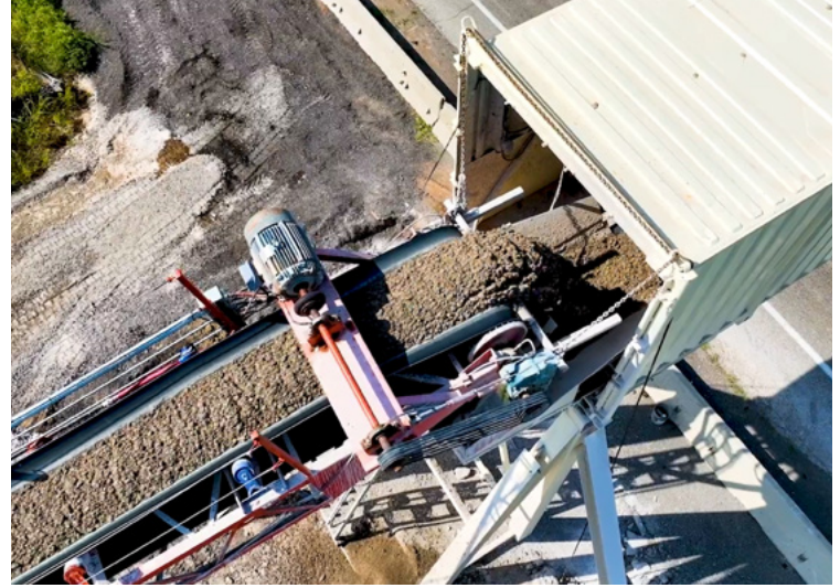
Wet-concrete-treated base material is transferred via conveyor belt.
