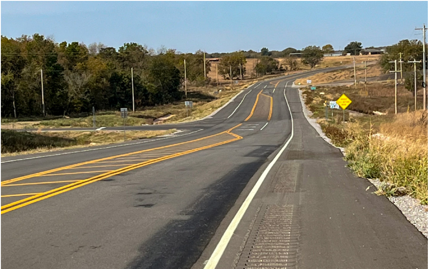
Facing West: A wide angle of the SH-39/SH-102 junction with new shoulders and two left turn lanes for eastbound drivers.
