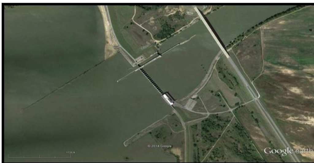
Figure 20 Aerial View of Robert S. Kerr Lock and Dam
