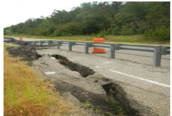
Figure 1 Active Slide in Eastern Oklahoma
