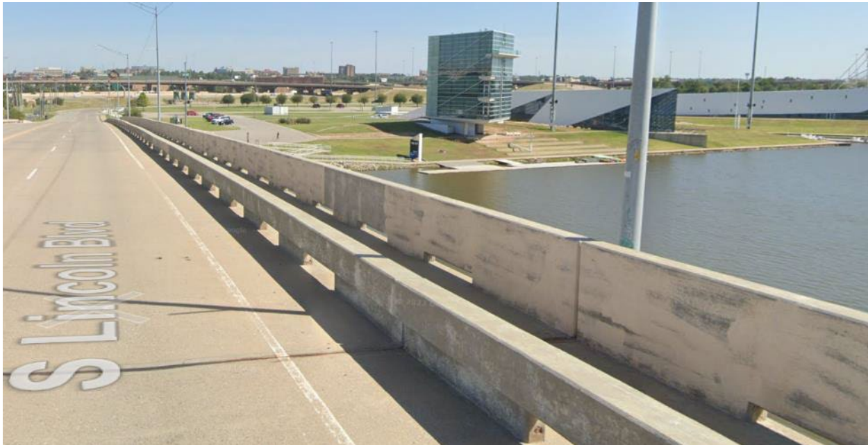
Figure 5: S. Lincoln Boulevard Sidewalk (facing North)
