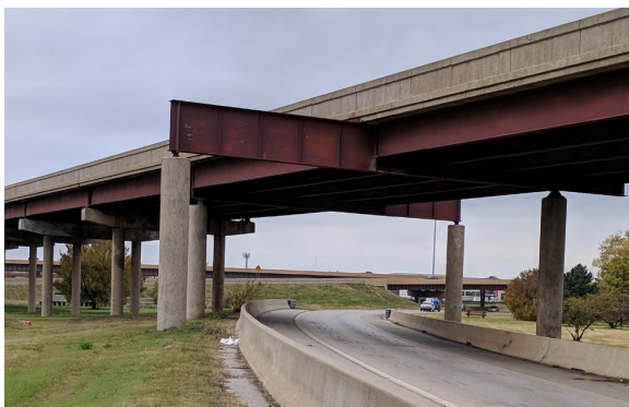
Figure 11: Fracture Critical Members (FCM)
