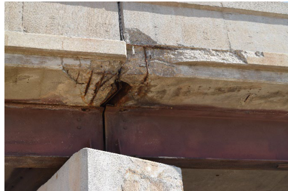
Figure 9: Concrete Spalling
