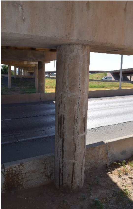
Figure 10: Column Deterioration
