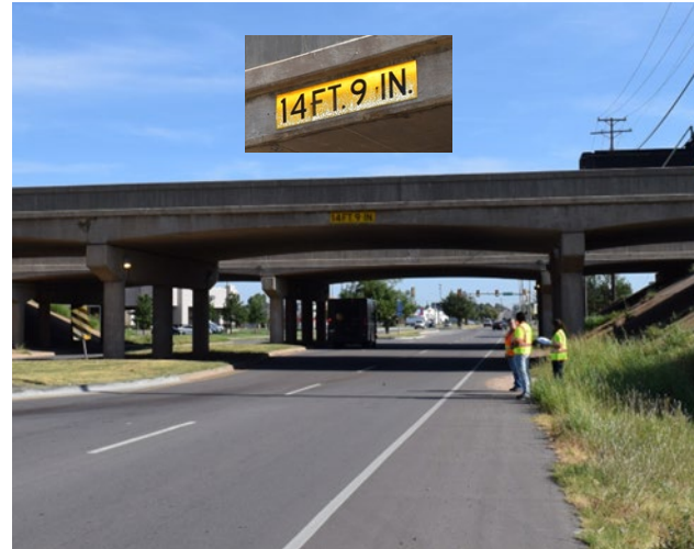
Figure 7: I-40 Bridge over Portland (looking North)
