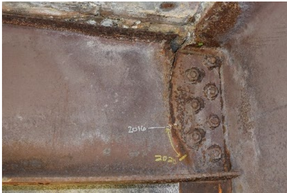
Figure 8: Crack Progression
