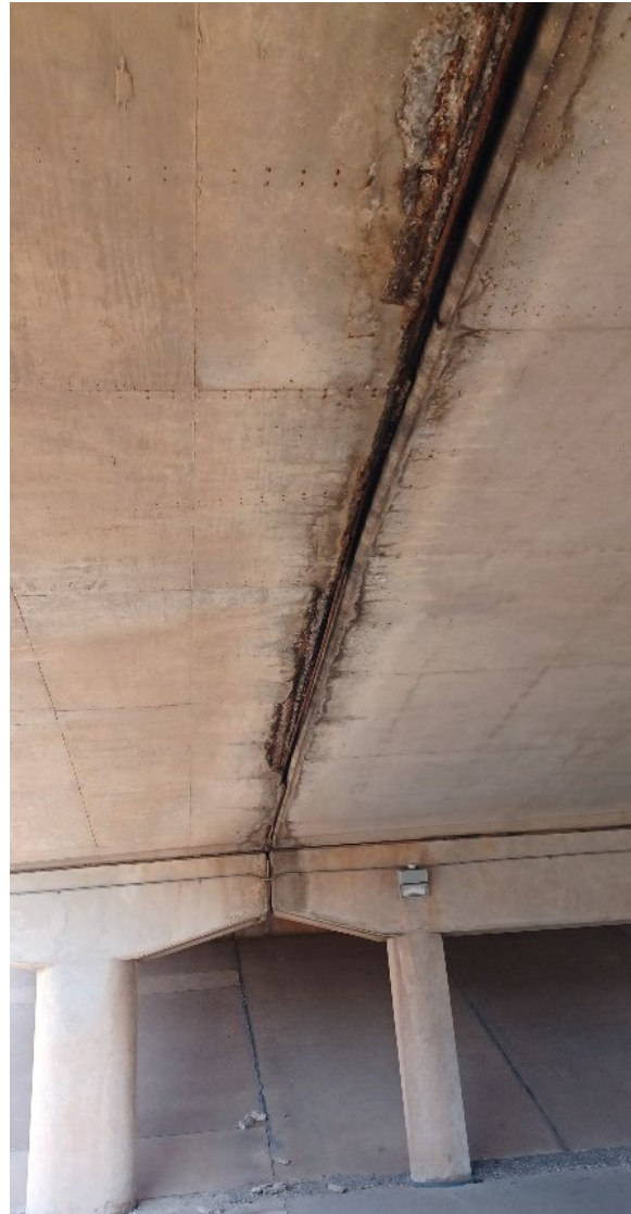
Figure 12: Concrete Spalling
