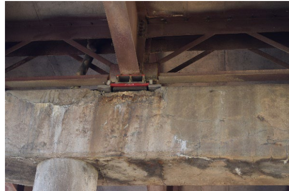
Figure 14: Concrete Spalling
