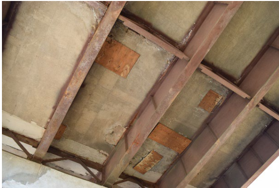
Figure 13: Plywood Formwork
