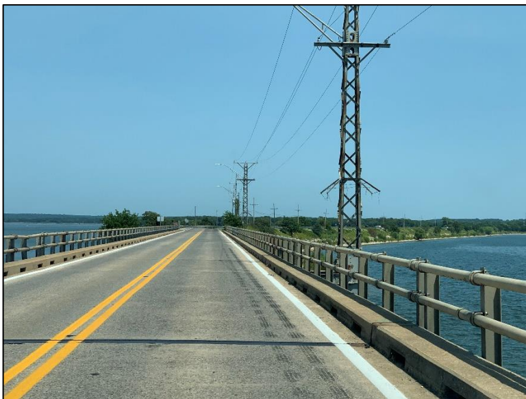
Figure 2: Overhead Power Lines on the Roosevelt Bridge
