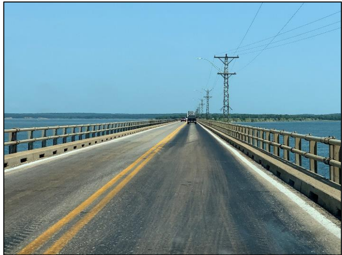
Figure 16: Narrow Deck on Roosevelt Bridge
