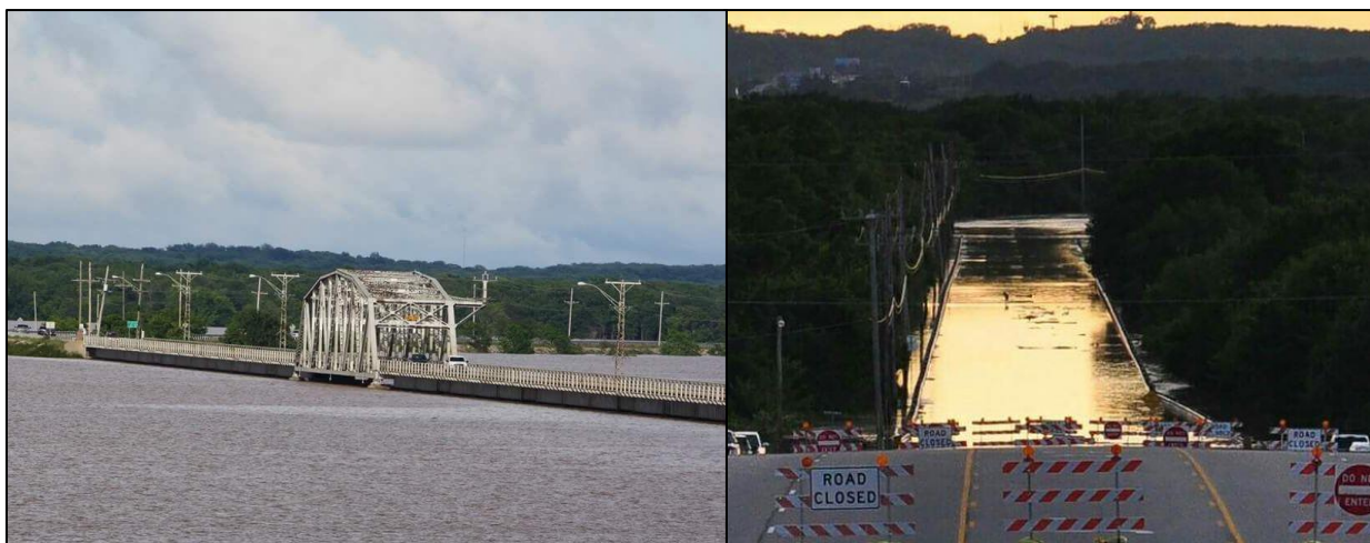
Figure 6: Roosevelt Bridge Flooding, 2015
