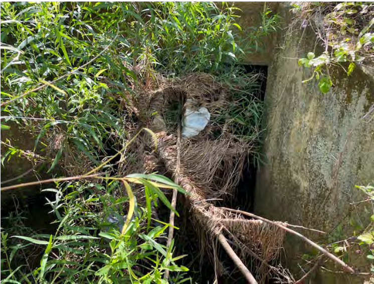
Photograph 18-A: Structure #10 carrying R4SBC-02 across US-69 NB and SB lanes.
