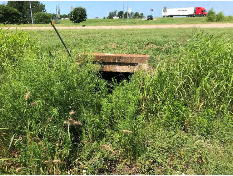
Photograph 16-B: Structure # 9, no swallows observed.
