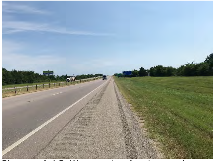
Photograph 1-B: Western edge of study area, along US-69 lanes, facing north into study area.
