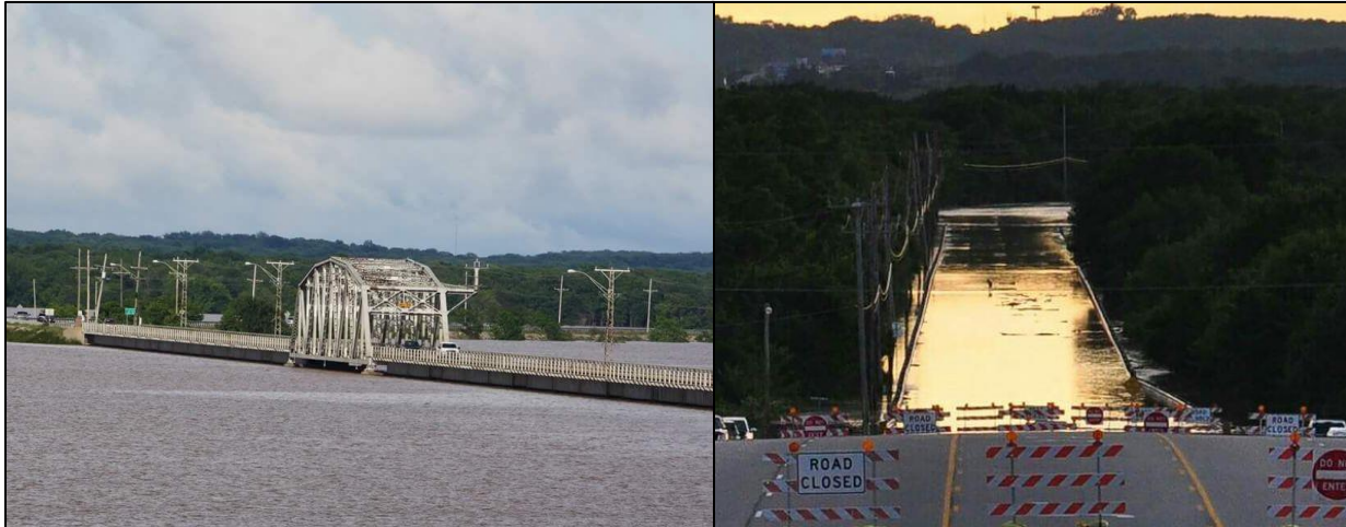
FIGURE 4: ROOSEVELT BRIDGE FLOODING, 2015
