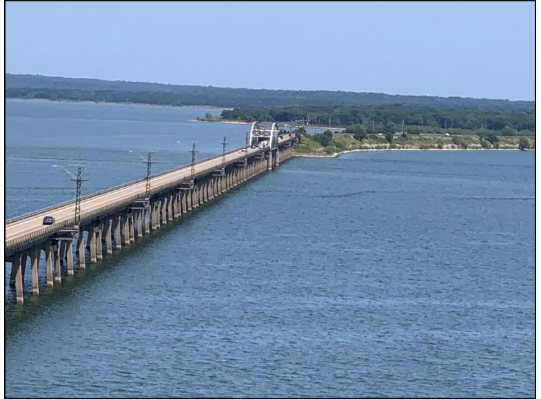
FIGURE 1: ROOSEVELT MEMORIAL BRIDGE
