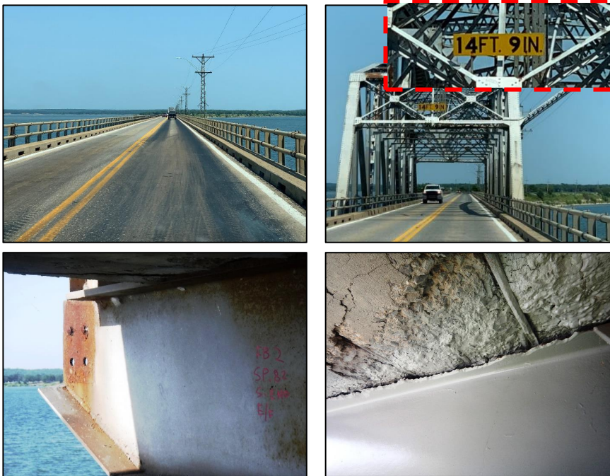
FIGURE 6: ROOSEVELT BRIDGE INSPECTION PHOTOS (2021)
