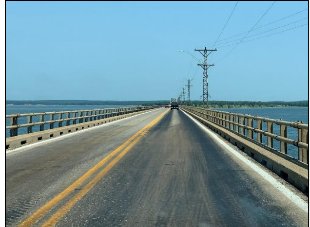
FIGURE 2: ROOSEVELT BRIDGE NARROW DECK WIDTH
