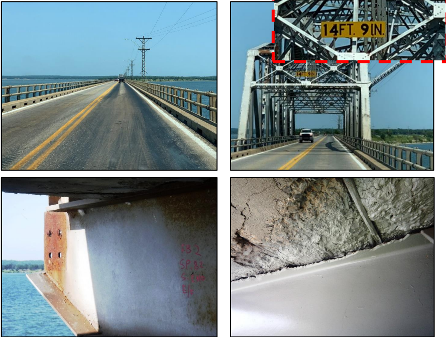
FIGURE 6: ROOSEVELT BRIDGE INSPECTION PHOTOS (2021)
