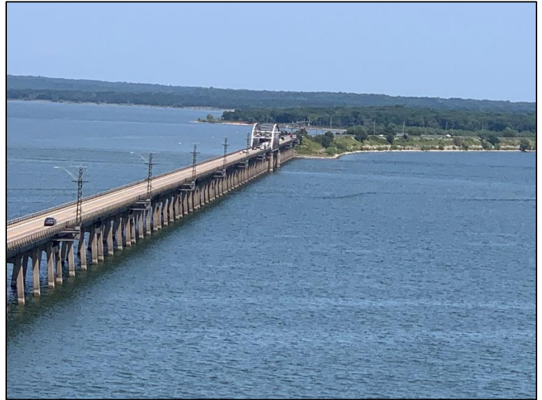
FIGURE 1: ROOSEVELT MEMORIAL BRIDGE
