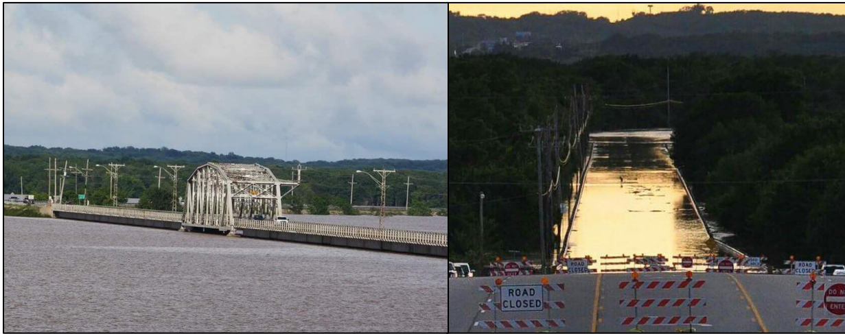
FIGURE 4: ROOSEVELT BRIDGE FLOODING, 2015
