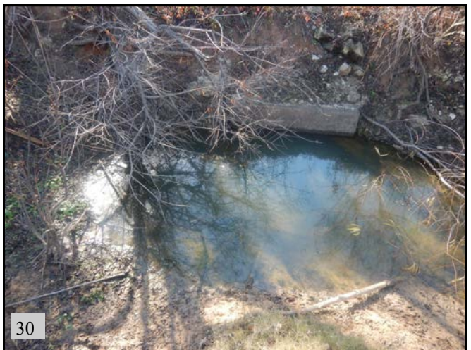
▲ (PS 7): View of flooded structure that OW 4a, 4b, and OW 5 flow into. View is to the south.
