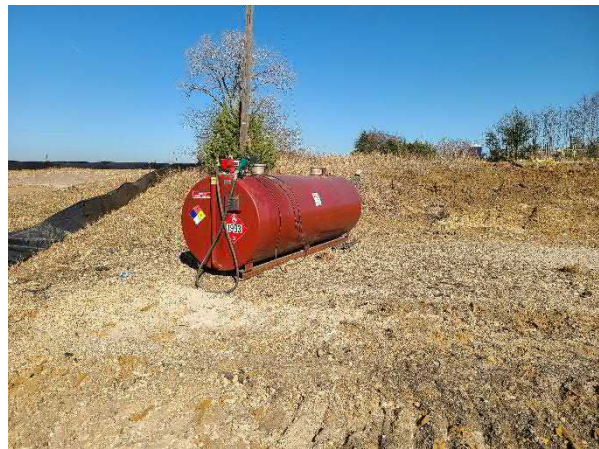
Photo 12 View of diesel AST.
