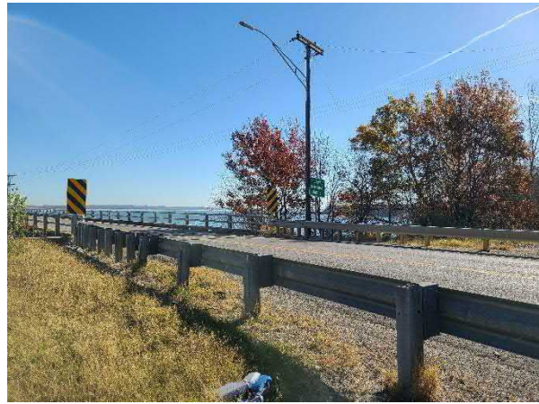
Photo 2 View of the bridge approach and signage.
