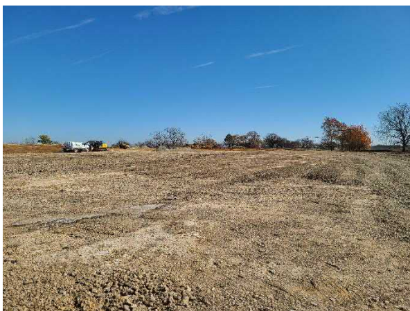
Photo 11 View of area of construction.
