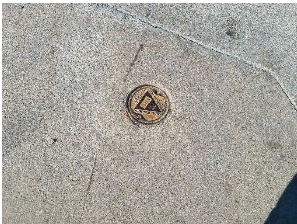
Photo 9 View of a monitoring well.
