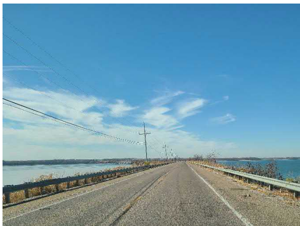
Photo 5 Typical view of the site.
