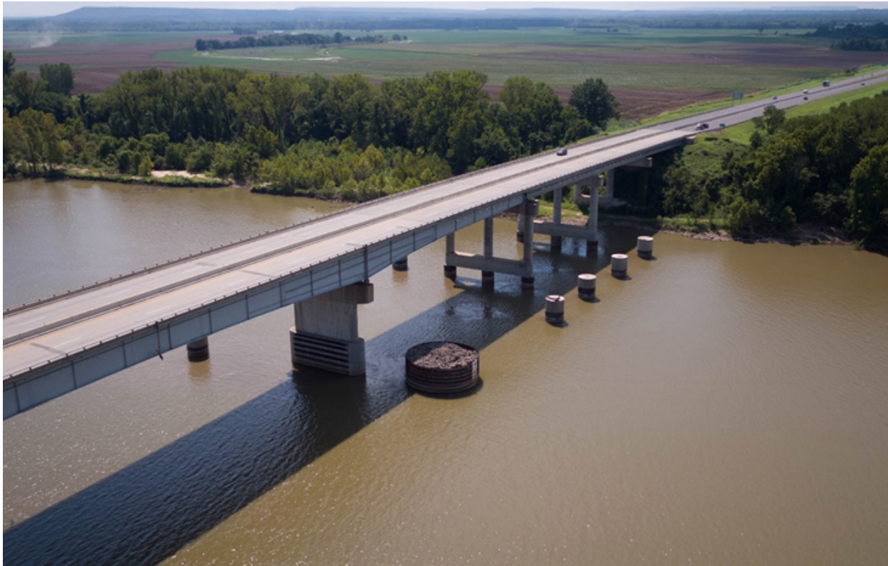
Figure 1: I-40 Bridge over the Arkansas River at Webbers Falls
