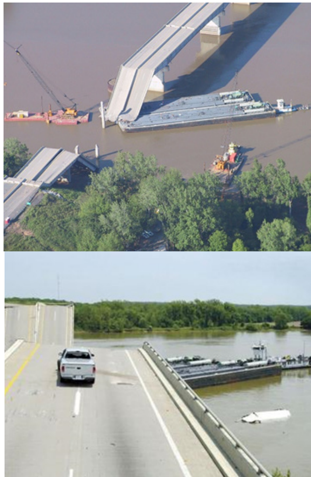
Figure 4: I-40 Bridge Collapse on May 26, 2002
