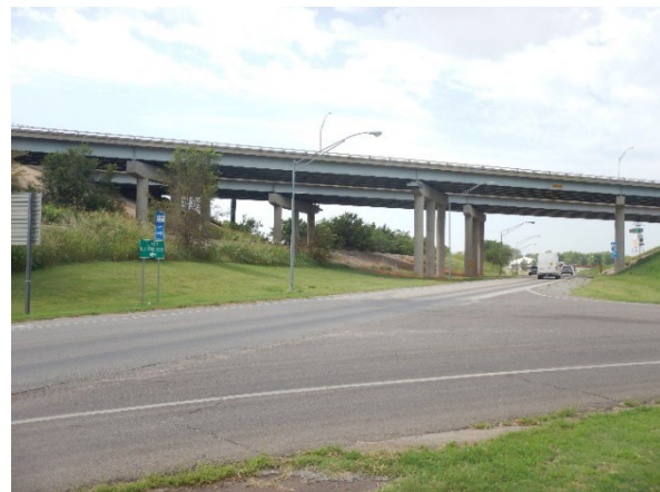
Figure 2: Neptune Drive Bridges
