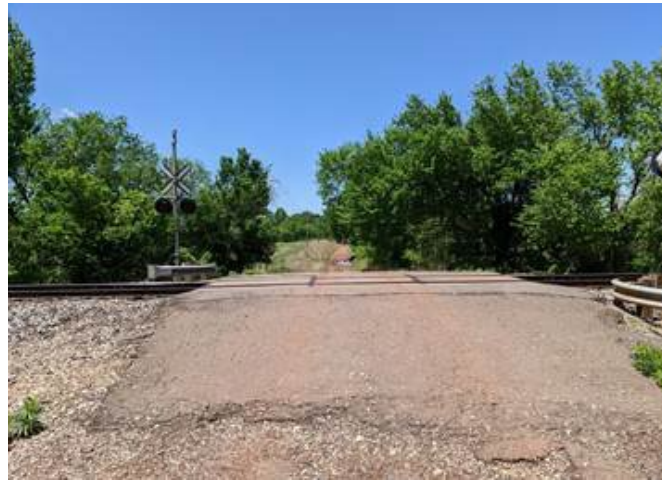
Figure 6. Guthrie Prairie Grove Road at-grade Crossing
