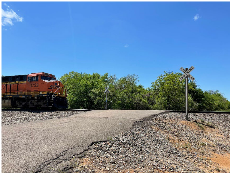
Figure 1. Road 0740 at-rail Crossing in Logan County
