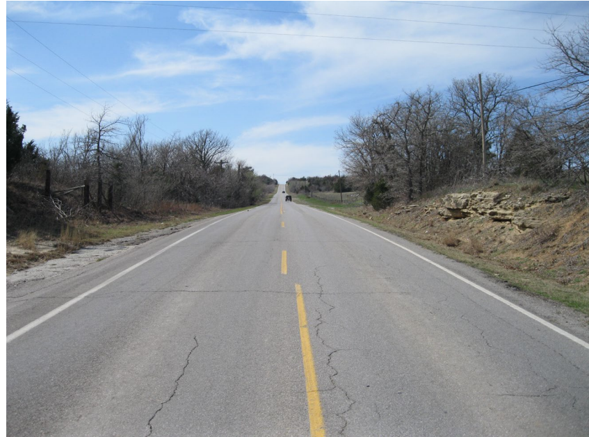
Rural Oklahoma roadway with no shoulder US 277, Cement County
