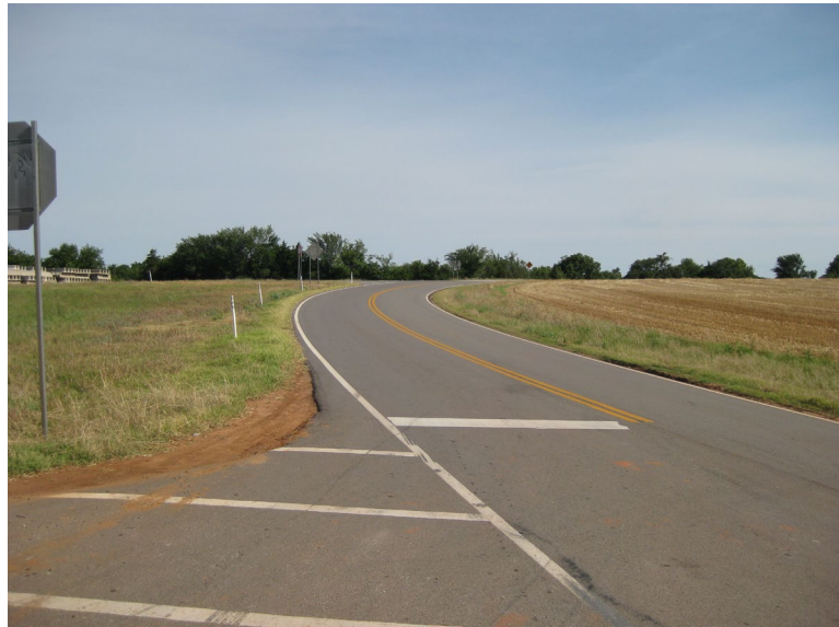
Roadway curvature on rural roadways. US 77 and SH 51, Logan County
