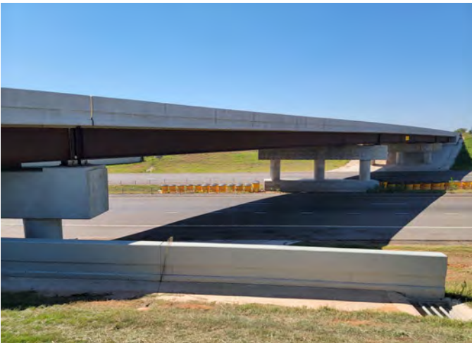
15. Bridge at C19
