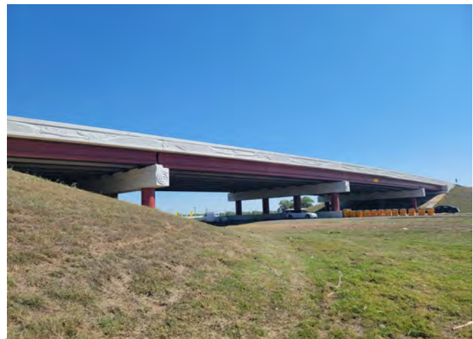
16. Bridge at C8
