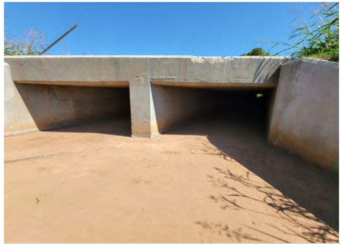
16. Bridge at C14
