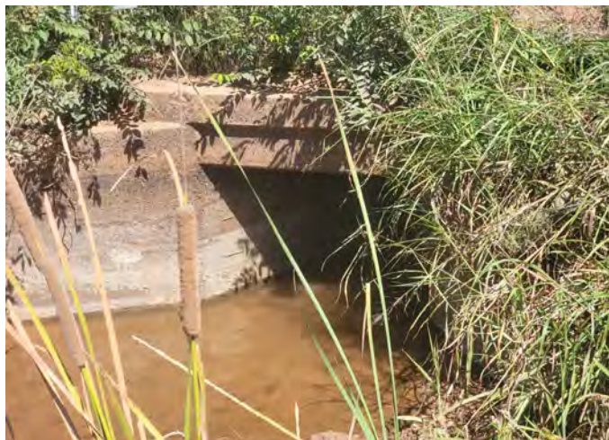
17. Bridge at C21
