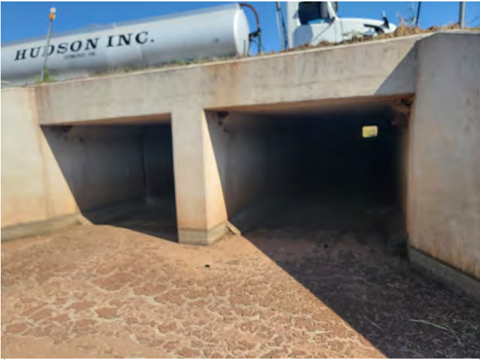
13. Bridge at C5
