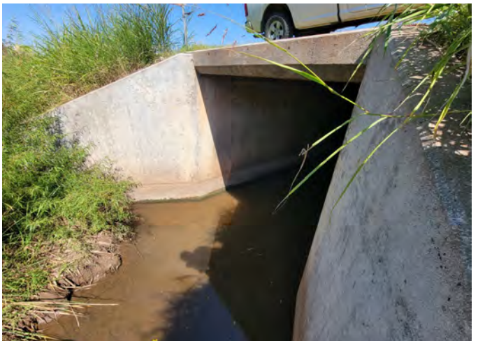
18. Bridge at C16
