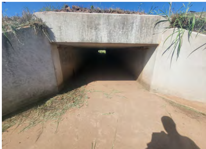
17. Bridge at C9
