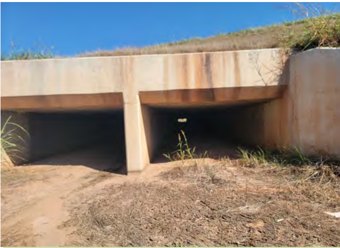
15. Bridge at C7
