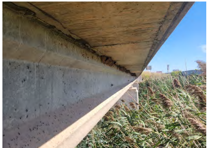
9. Bridge at C4
