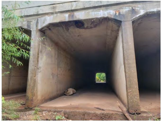
14. Bridge at C18
