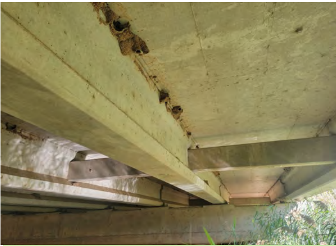
9. Bridge at C1
