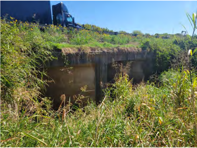
13. Bridge at C11
