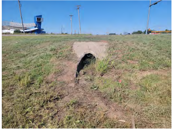
14. Culvert at C6
