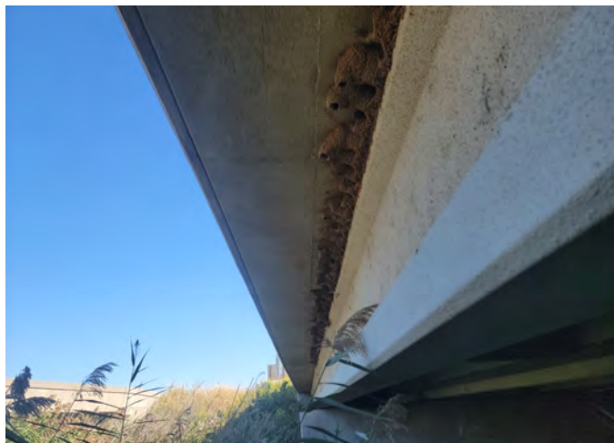
9. Bridge at C3
