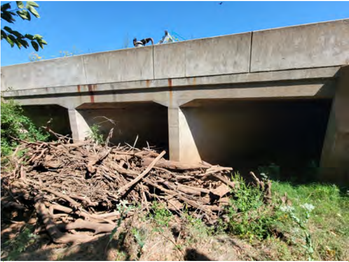
13. Bridge at C17
