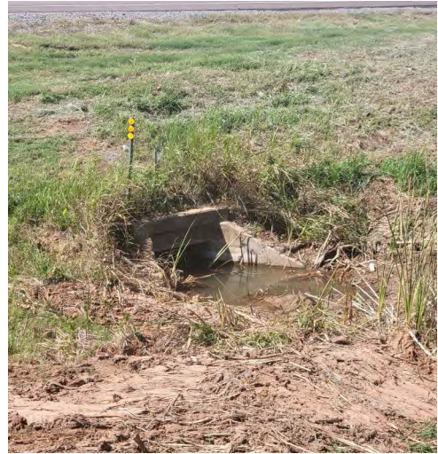
16. Culvert at C20
