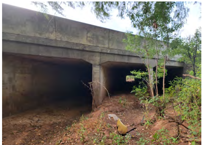
18. Bridge at C22
