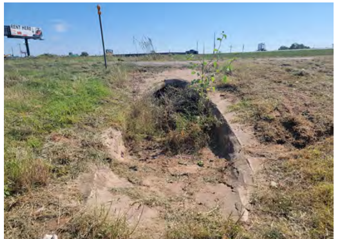
18. Culvert at C10
