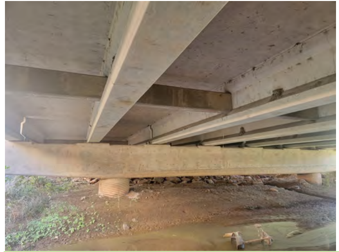
10. Bridge at C2
