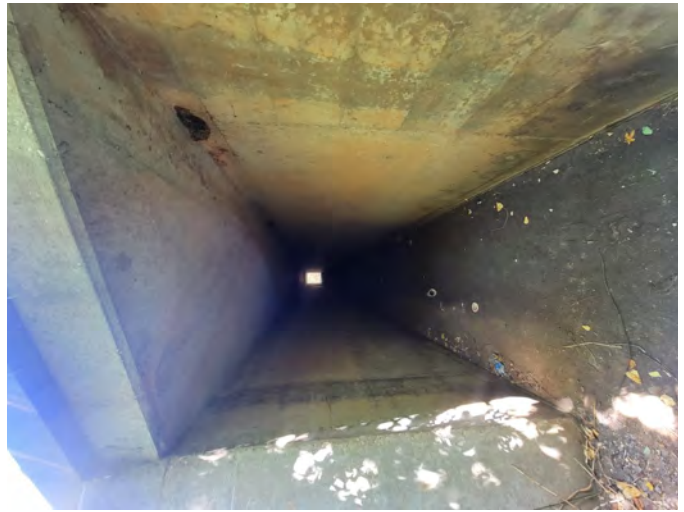
14. Bridge at C12
