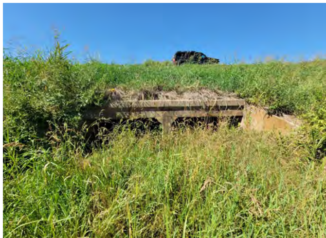
17. Bridge at C15
