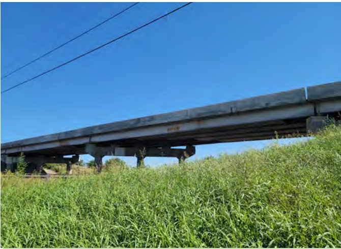
15. Bridge at C13
