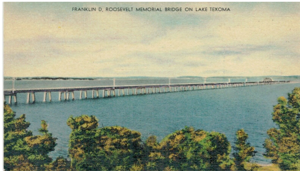
Image 2. A c. 1950 postcard of the Roosevelt Bridge. The Warren through-truss with a polygonal top chord can be seen at far right; view facing northeast.
