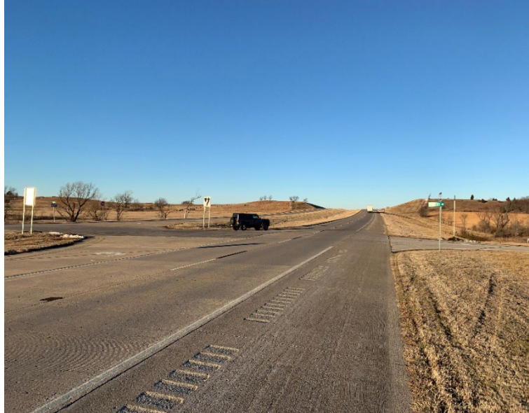
Example of an at-grade intersection on US-412 in the corridor. Source: ODOT
