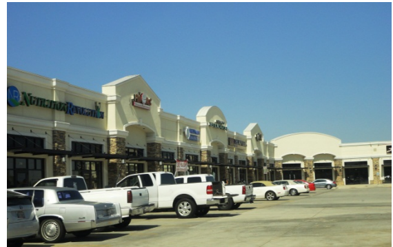
New Shopping Center along Western Avenue
