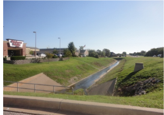
Major drainage way separating retail buildings from Hefner Road
