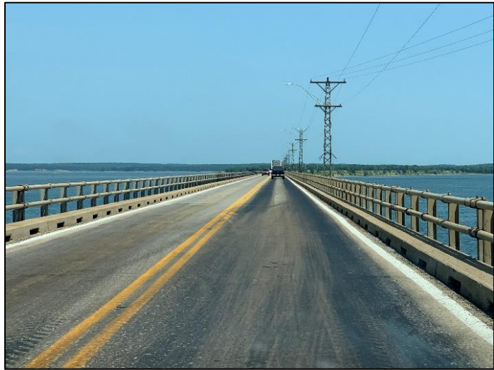
Figure 10: Narrow Deck on Roosevelt Bridge
