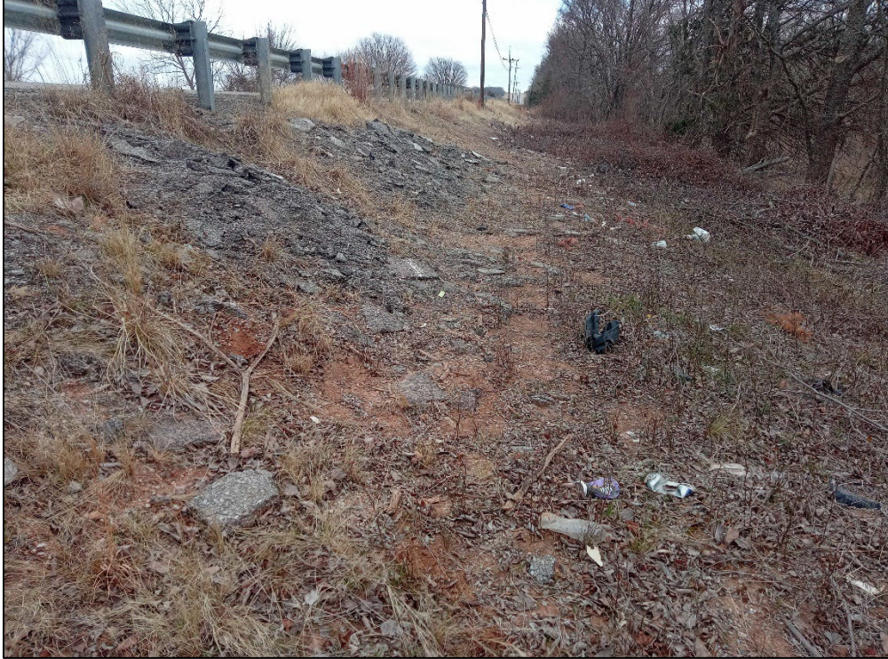
Photo 11: Asphalt and trash on sloped right-of-way – Viewing northeast.
