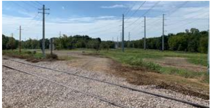
Figure 5. Disjointed Roadway Segment along Patrol Road
