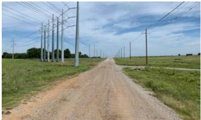
Figure 1. Existing Patrol Road Conditions
