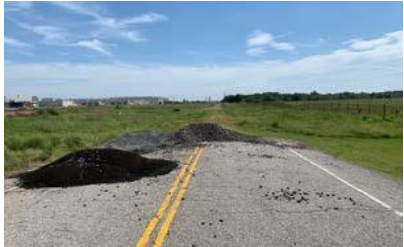
Figure 2. Existing Williams Road Conditions
