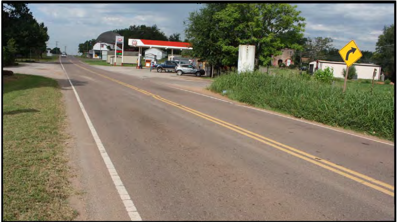
State Highway 66 Roadbed in Arcadia and vicinity Oklahoma County, Arcadia, Oklahoma Intersection of State Highway 66 and Odor St. Anna Eddings--ODOT Cultural Resources Program
