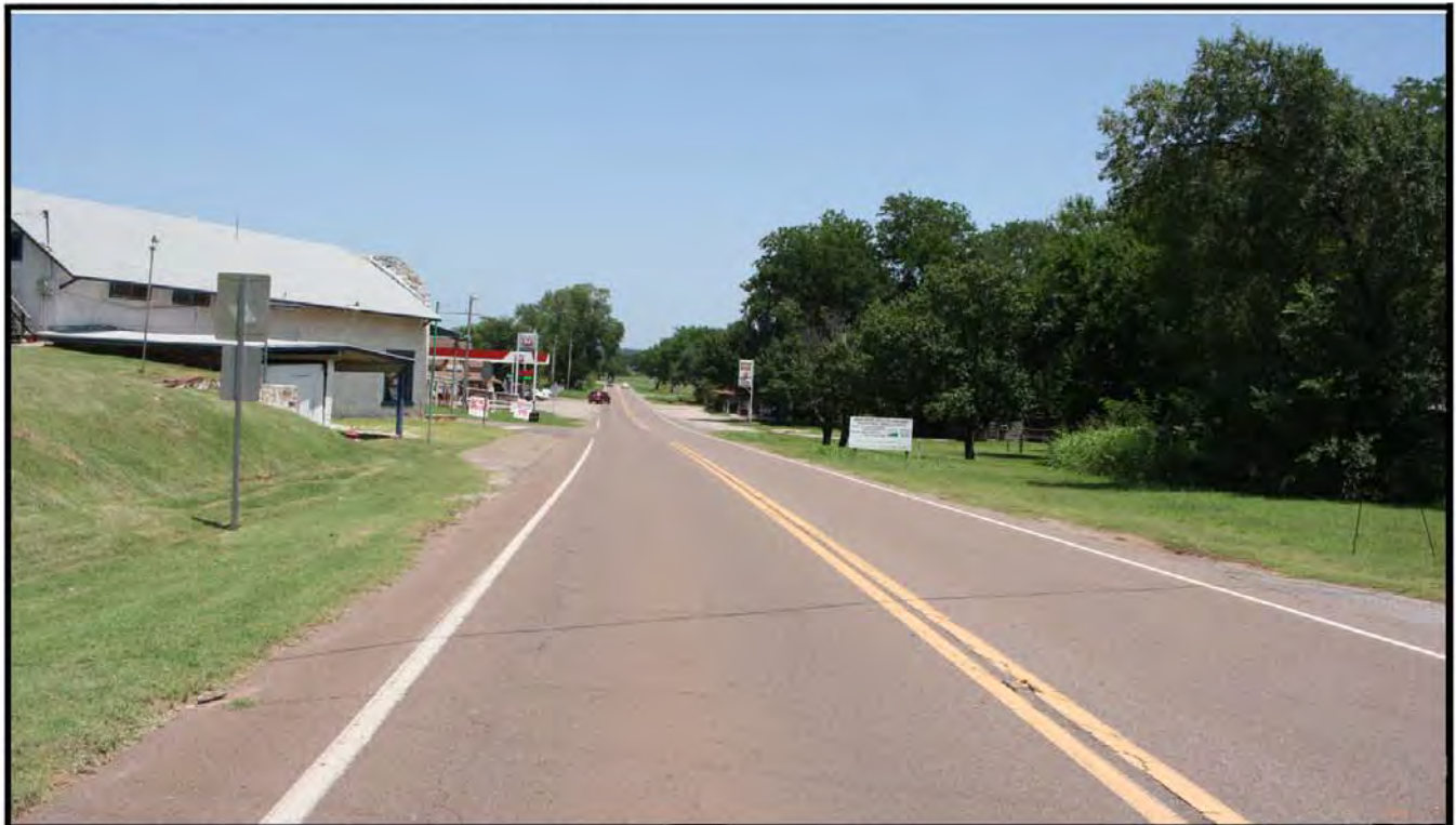
State Highway 66 Roadbed in Arcadia and vicinity Oklahoma County, Arcadia, Oklahoma State Highway 66 between Division & Main Streets Anna Eddings--ODOT Cultural Resources Program
