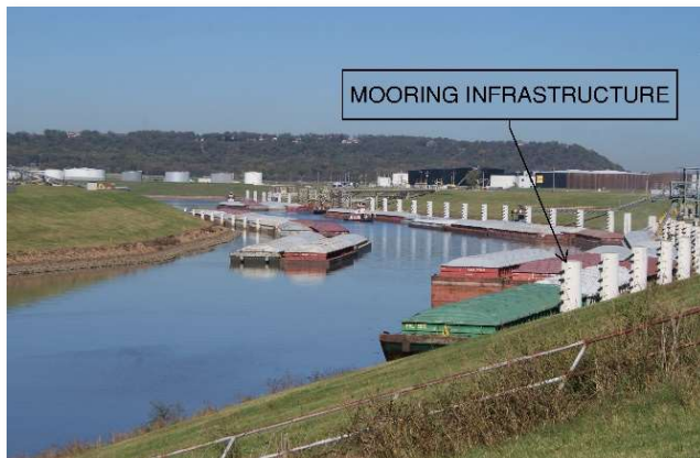
June 2021: Mooring Infrastructure – Tulsa Port of Catoosa
