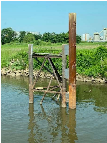
Existing Dolphin at the Port of Muskogee
