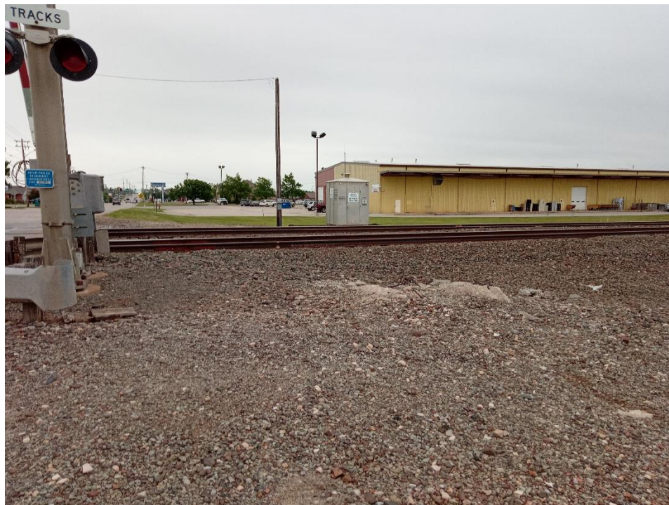
Photo 2. BNSF Railroad; facing east.
