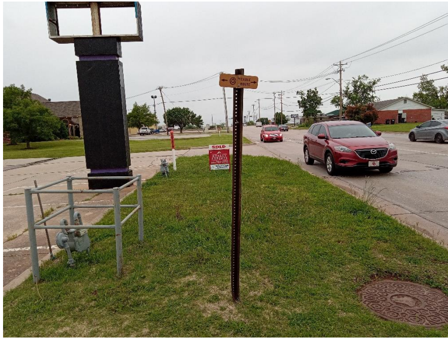
Photo 1. East end of project area; facing west. Note the disturbances: sewer, cable route, gas line, power lines, parking lots, driveway.
