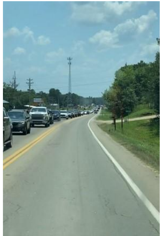
Traffic Backups are frequent on US-259 through Hochatown
