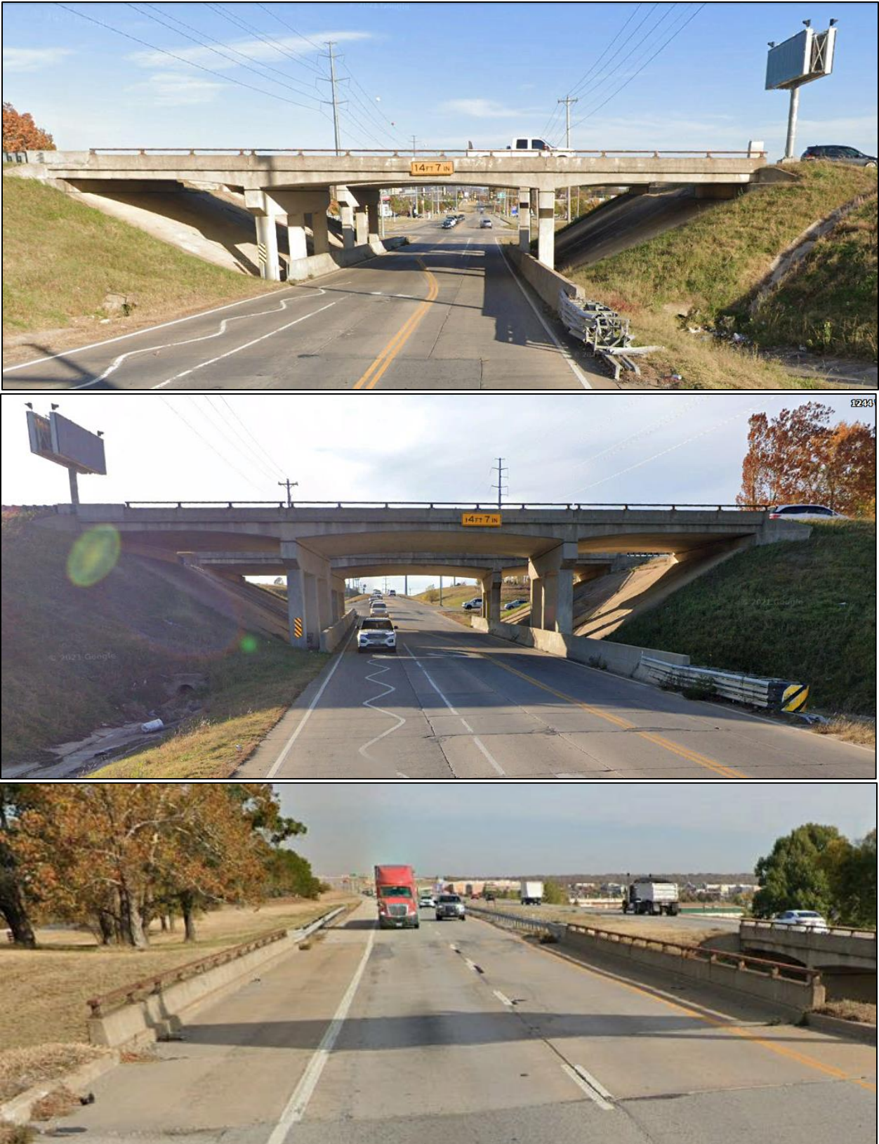
Figure 10: Existing US-75 Bridges over W. 81st Street
