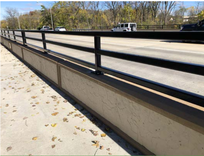
Figure 5.3: Farnsworth Ave over Indian Creek, Aurora, IL
