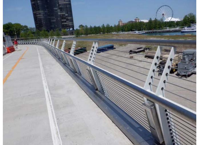
Figure 5.5: Lakefront Trail Bridge, Chicago, IL
