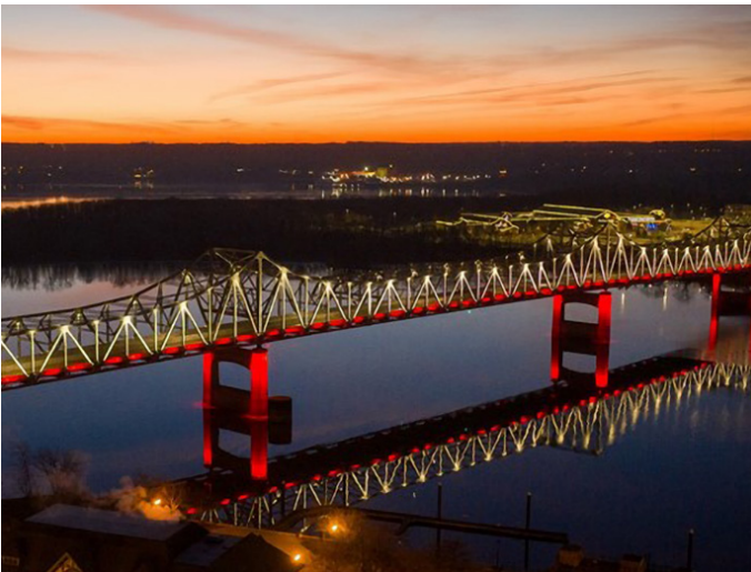
Figure 6.3: Murray Baker Bridge, Peoria, IL
