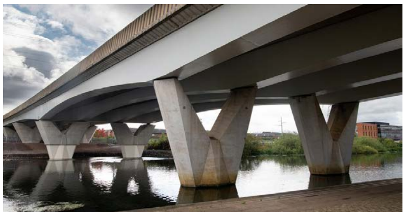
Figure 2.3: Nene Bridge, Peterborough, United Kingdom
