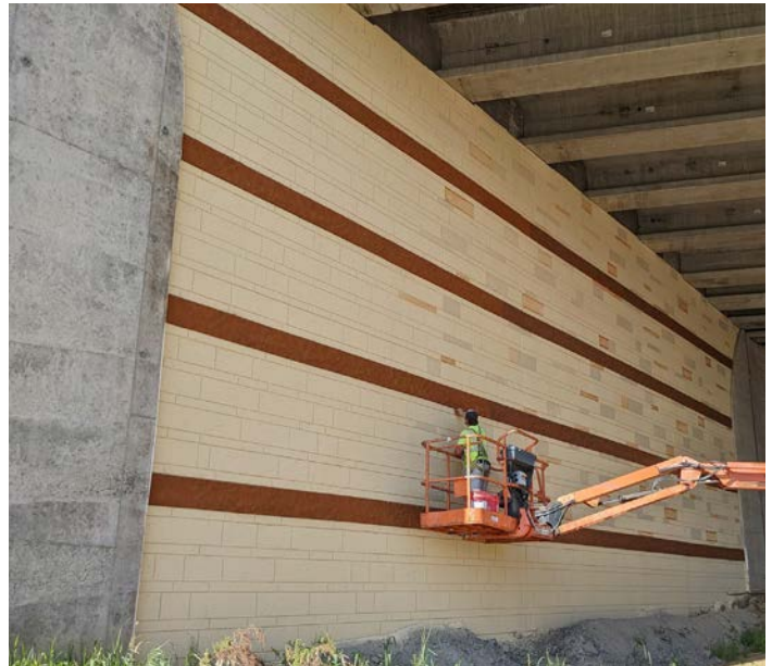
Figure 8.6: I-80/I-380 Interchange, Johnson County, IA
