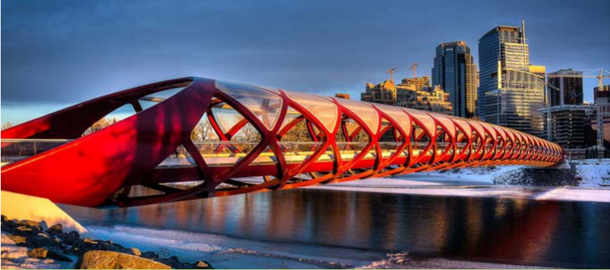
Figure 3.7: Peace Bridge, Alberta, Canada
