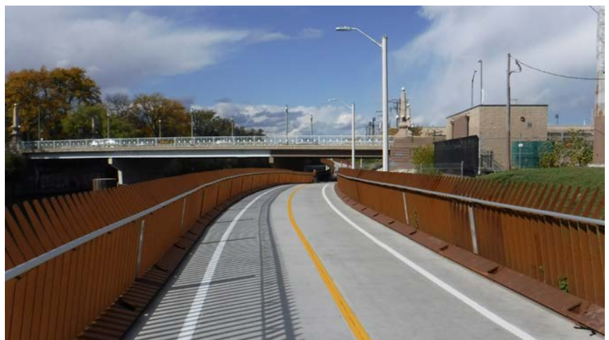
Figure 9.3: Addison Pedestrian Bridge, Chicago, IL
