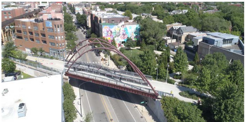
Figure 3.3: Milwaukee 606 Trail Bridge, Chicago, IL
