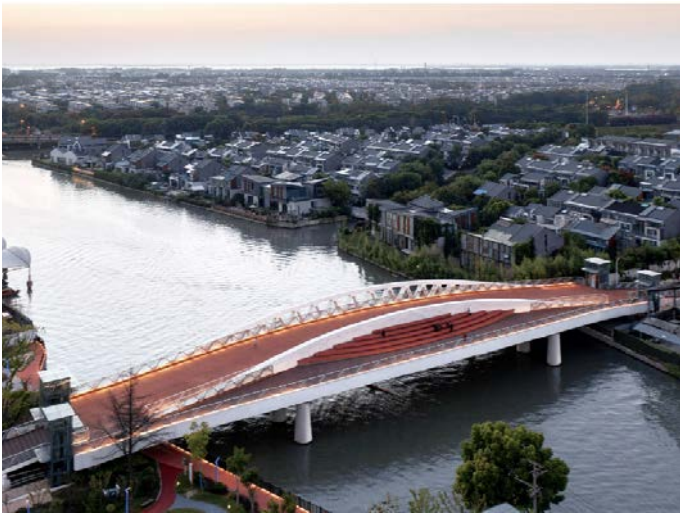
Figure 4.6: Dawn Bridge, Shanghai, China
