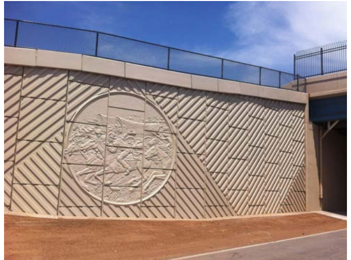
Figure 8.2: Main Street and I-35 Bridge, Norman, OK
