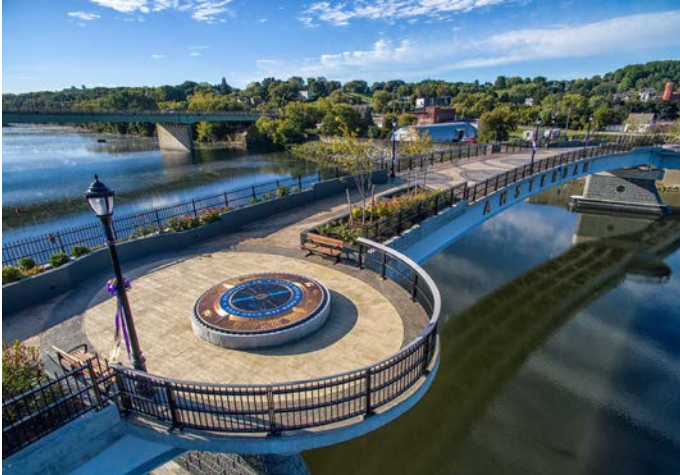
Figure 4.5: Mohawk Valley Gateway Overlook Bridge, Amsterdam, Netherlands
