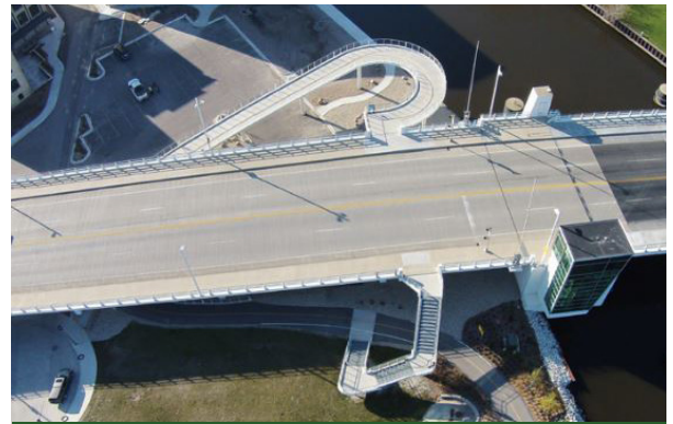
Figure 11.2: Menomonee Valley Bike Path Bridge, Milwaukee, WI
