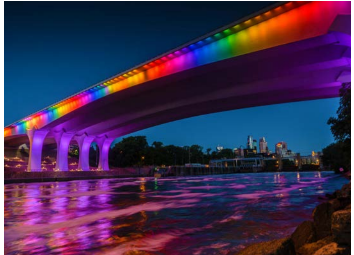
Figure 6.5: I35 W. Bridge, Minneapolis, MN
