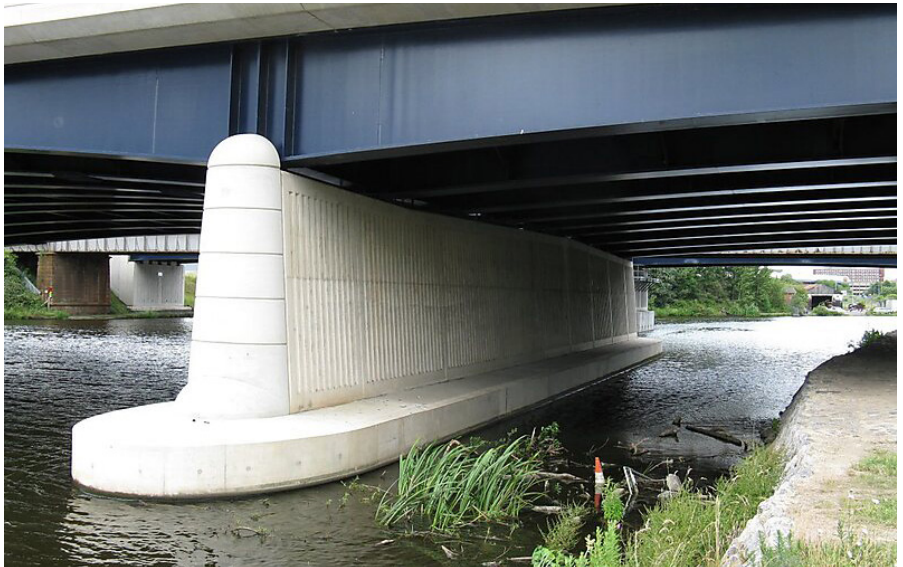
Figure 1.1: Surtees Bridge, Stockton-On-Tees, United Kingdom
