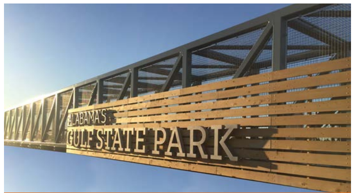
Figure 7.6: Gulf State Park Bridge, Gulf State Park, AL
