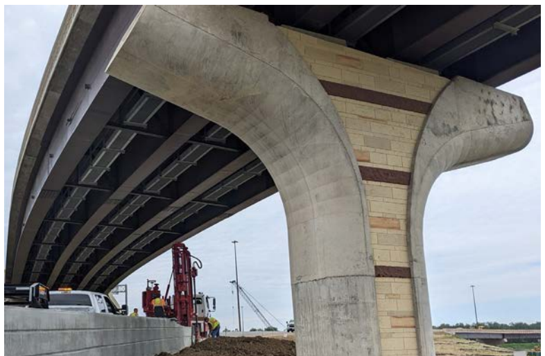
Figure 1.5: I-80/I-380 Interchange, Johnson County, IA
