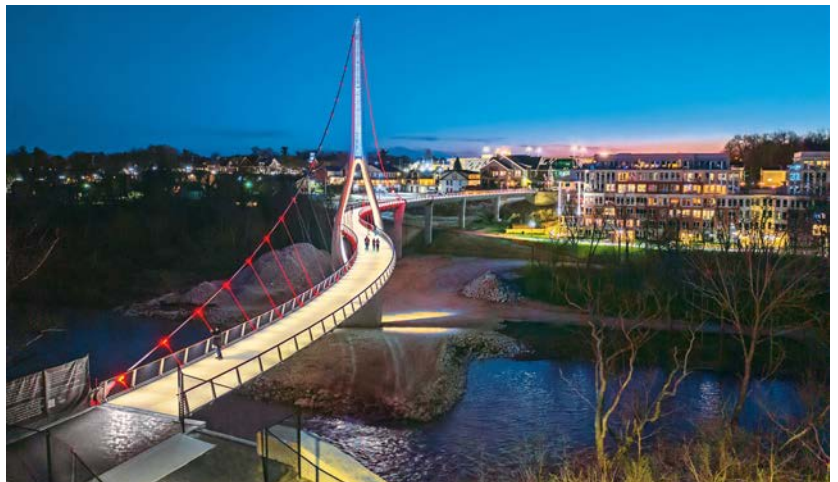
Figure 3.6: Dublin Link Bridge, Dublin, OH
