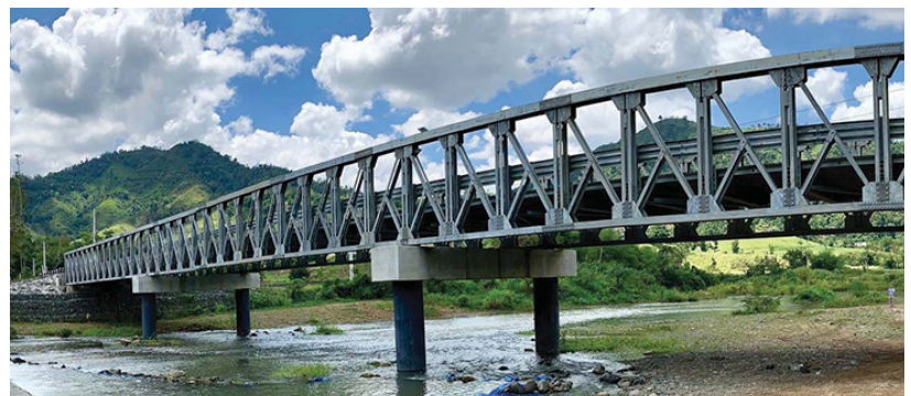
Figure 9.6: Steel Truss Bridge - Galvanized
