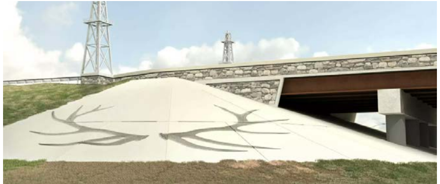
Figure 10.1: Elk Street Diverging Diamond Interchange, Elk City, OK
