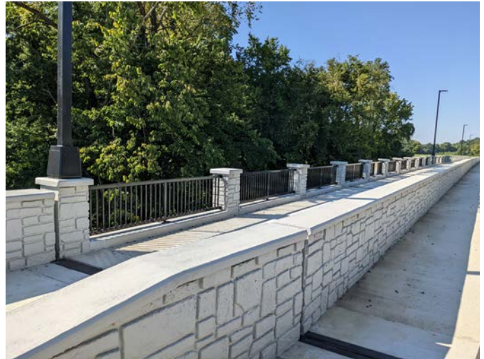
Figure 5.2: SE Park Bridge, Franklin, TN
