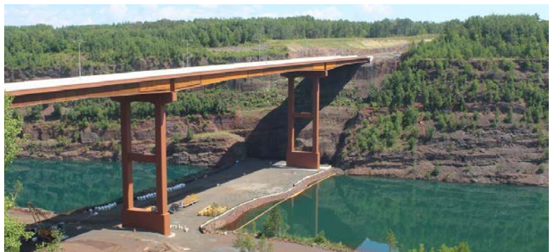
Figure 2.2: Rouchleau Mine Bridge, Eveleth, MN
