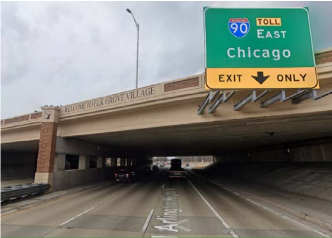
Figure 5.1: I-90 Over Arlington Heights Bridge, Village of Elk Grove, IL
