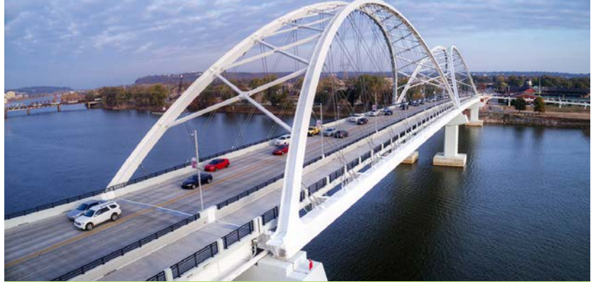
Figure 3.4: Broadway Bridge over Arkansas River, Little Rock, AR
