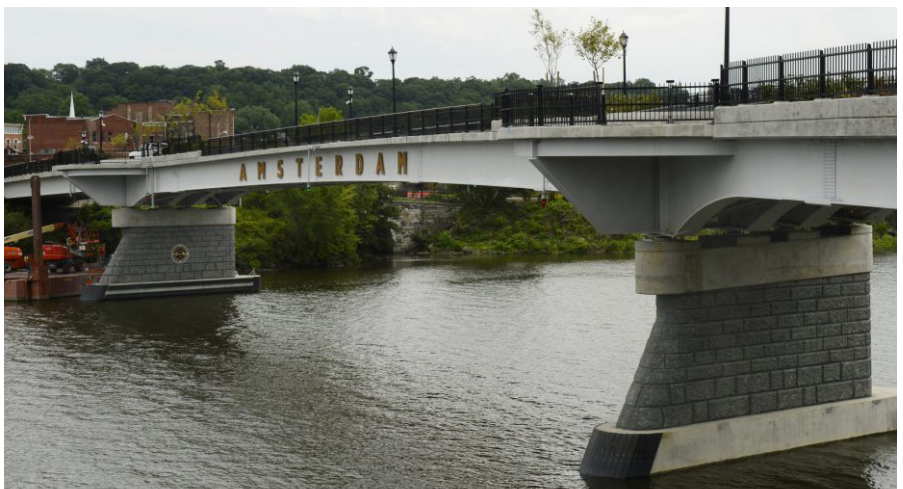
Figure 1.2: Mohawk Valley Gateway Overlook Bridge, Amsterdam, Netherlands
