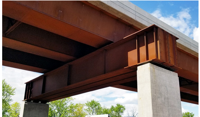
Figure 9.4: I-91 Interchange 29 Exit Ramp Flyover Bridge, Hartford, CT
