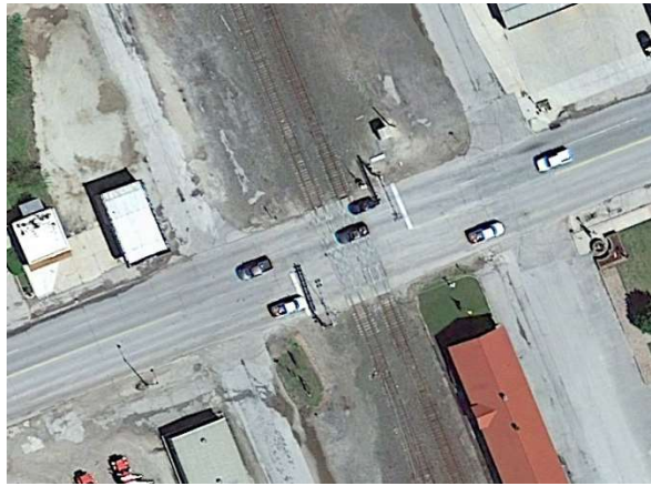
Figure 6: Main Street Crossing (Aerial)
