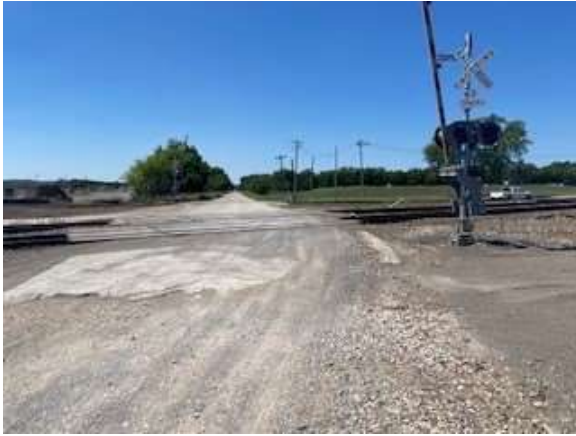
Figure 9: Hanover Road Crossing (020739P)
