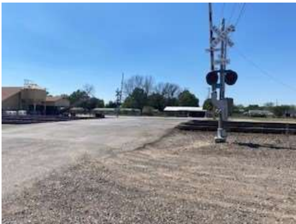
Figure 7: Atlanta Avenue Crossing (020740J)
