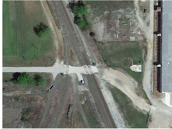
Figure 10: Hanover Road Crossing (Aerial)
