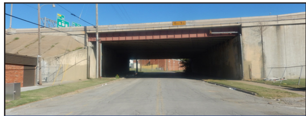
Figure 11: I-244 Underpass at Cheyenne
