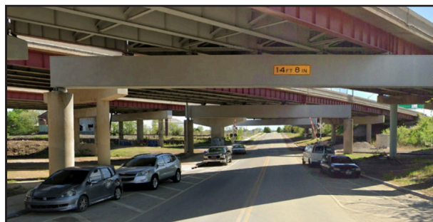
Figure 3: Archer Street under I-244
