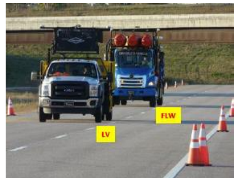
Source: Autonomous Truck Mounted Attenuator (ATMA) Pilot
