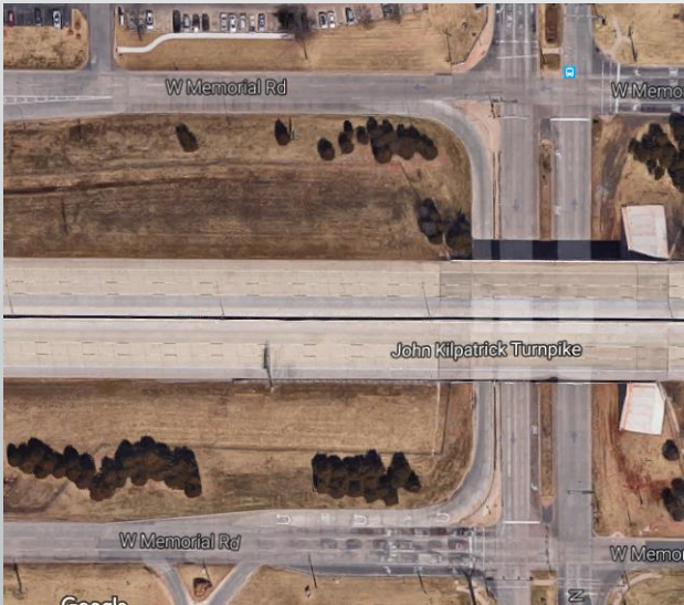
“Protected Turnaround” Under Kilpatrick Turnpike at Penn Ave.
