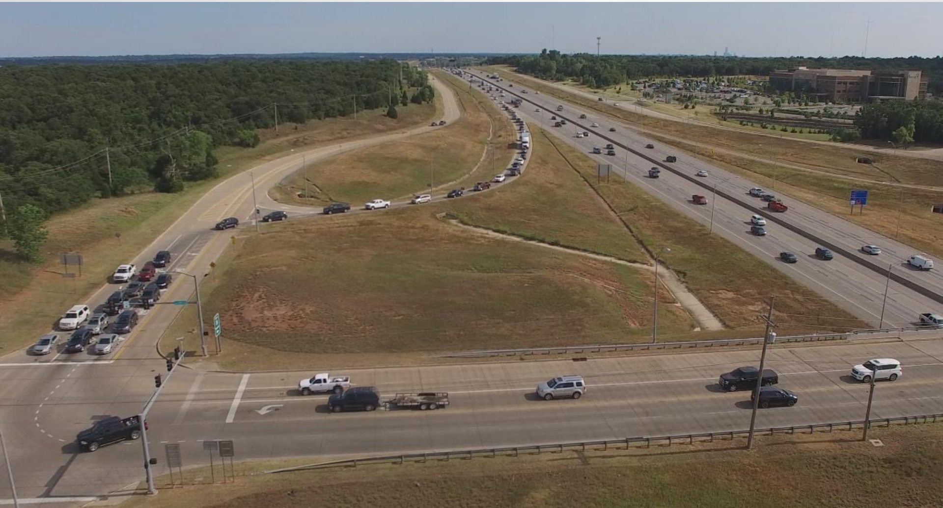
Drone View of Existing Ramp Backup onto I-35 at E. 15 th Street
