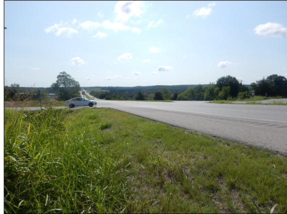
SH-51 and 265 th W. Avenue Intersection (looking west)
