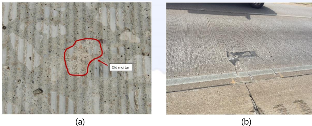
Figure 1 (a) Identification of RCA with old mortar from the field survey in I-40 EB Segment 3, and (b) Picture of a Typical Punchout from I-35 SB
