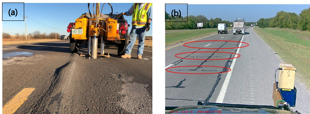
Figure 1 (a) Rutting on SH-7; (b) reflective cracking on I-35
