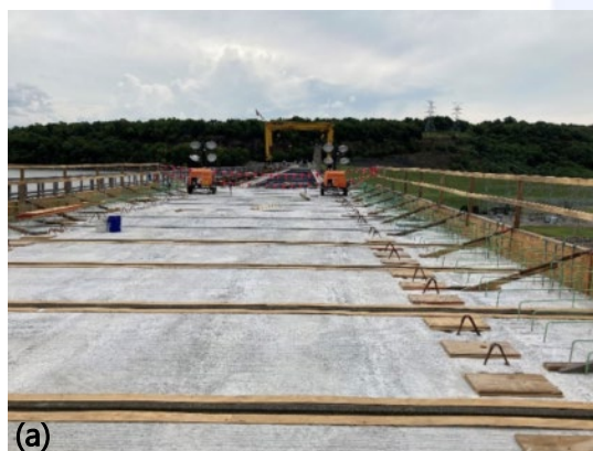
Figure 4 Bridge deck (a) immediately before; (b) during; and (c) after completion of joint placement
