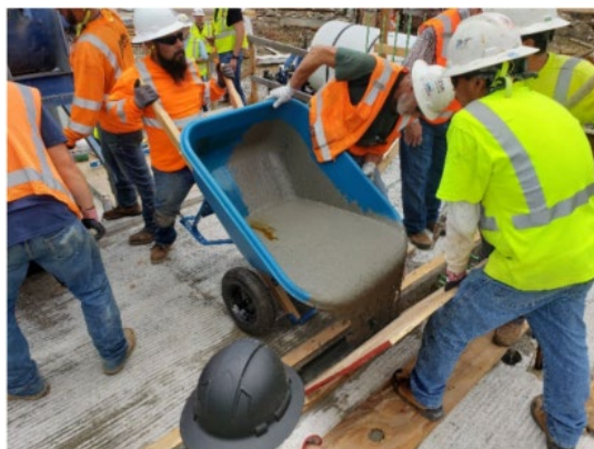
Figure 2 Placement of UHPC into transverse deck joints of the mock-up
