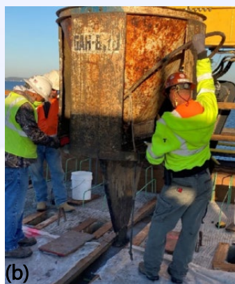
Figure 4 Bridge deck (a) immediately before; (b) during; and (c) after completion of joint placement
