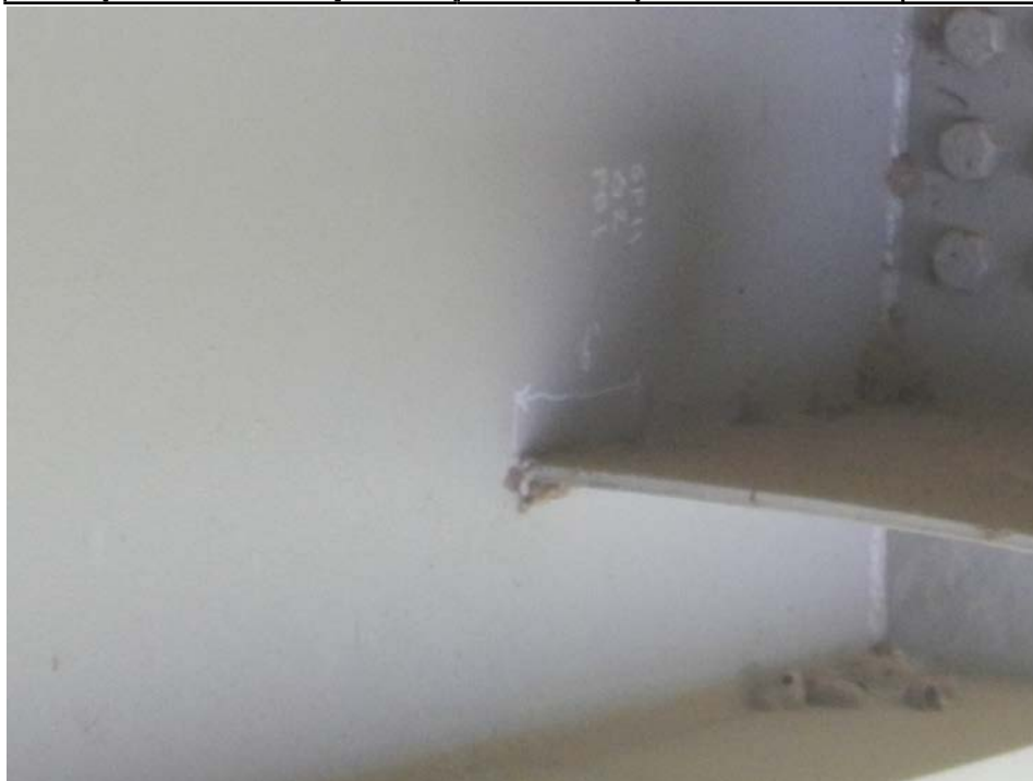
Photograph 22 - Looking east at span 11, girder 2 at floor beam 1. Note: no change to 6-inch-long crack at the lower lateral bracing gusset plate.
