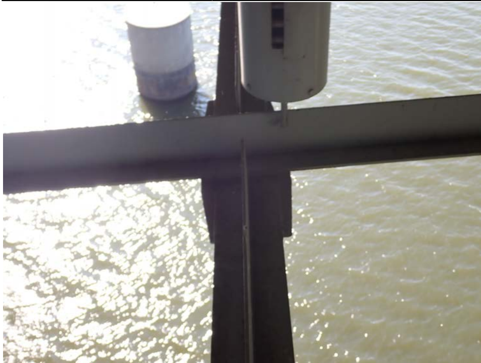
Photograph 36 - Looking southeast at span 4, girder bay 1-2 and floor beam bay 5-6. Note: fractured connection bolt at bottom of anti-vibration dampener (typical).
