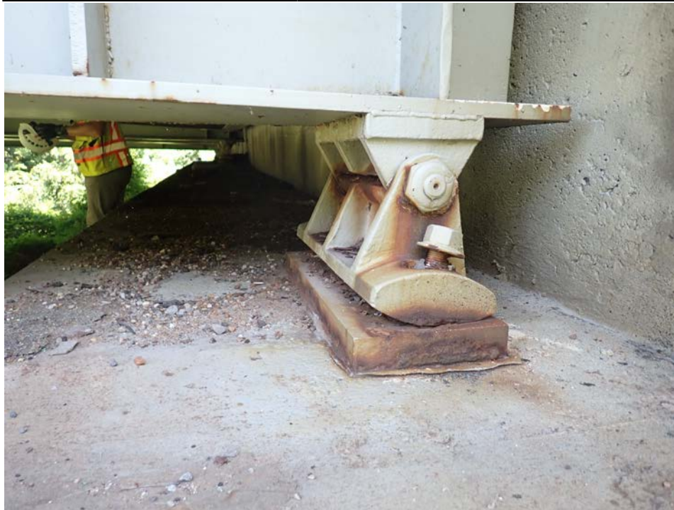
Photograph 43 - Looking north at beam 1 bearing at the east abutment. Note: bolts are disconnected at beam 1 bearing north, beam 2 both sides, beam 4 bearing south side.
