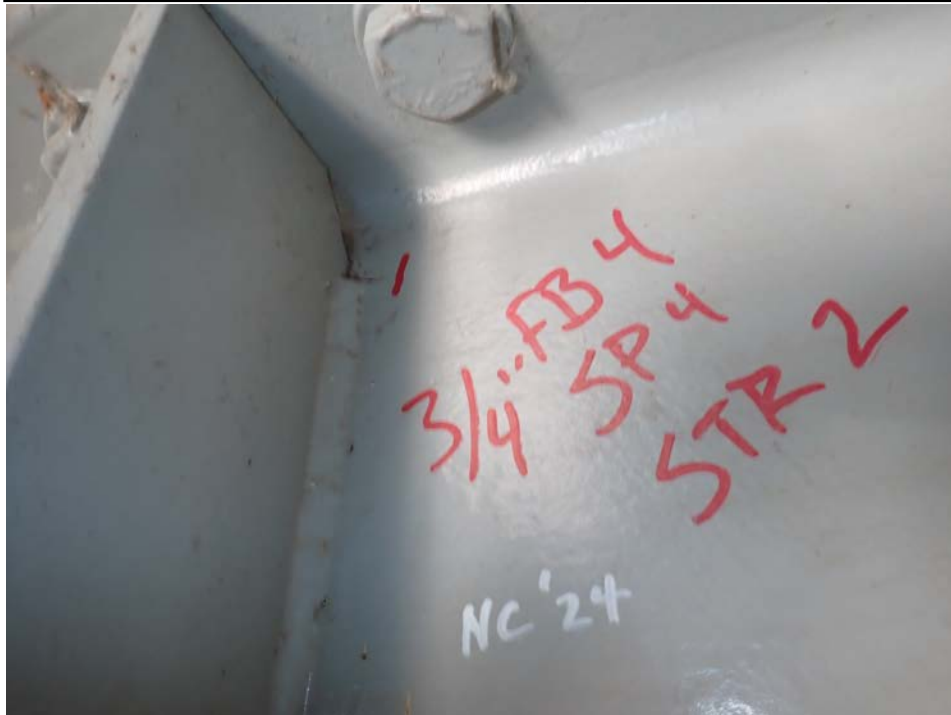
Photograph 18 - Looking southwest at span 4, floor beam 4, stringer 2. Note: no change to 3/4-inch-long horizontal crack.
