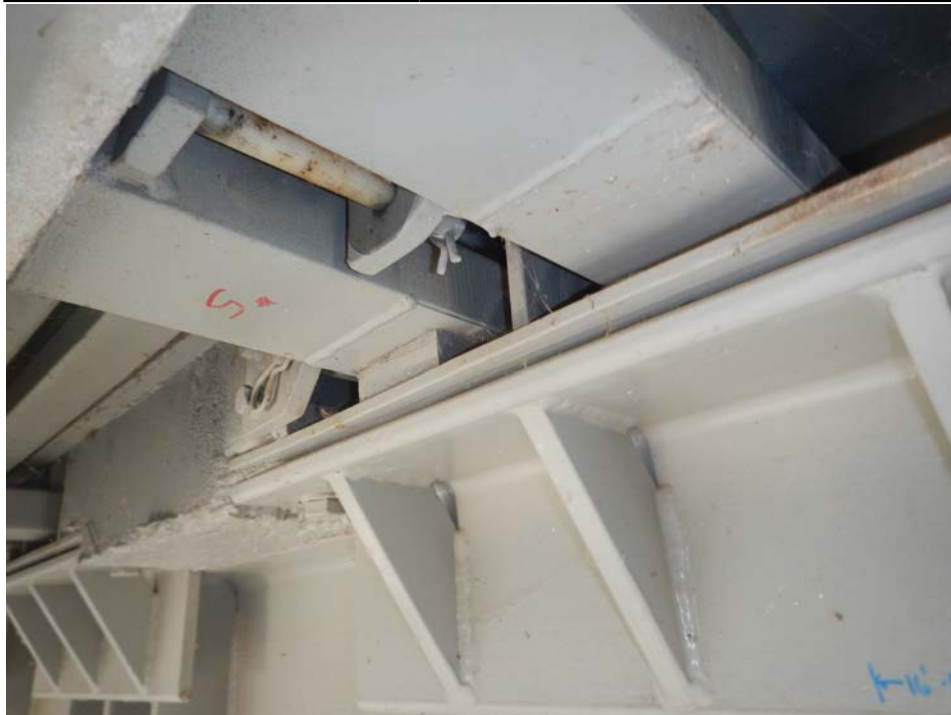
Photograph 6 - Looking east at the underside of the pier 3 modular joint at support box 5. Note: bearing block for support bar 1 is missing at the east support box. Stainless steel sliding surface is painted (typical).
