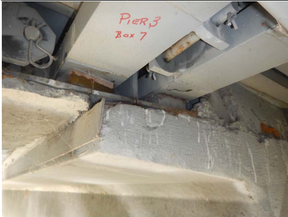
Photograph 7 - Looking west at the underside of the pier 3 modular joint at support box 7. Note: bottom plate of bearing support box is fractured adjacent to vertical plate.
