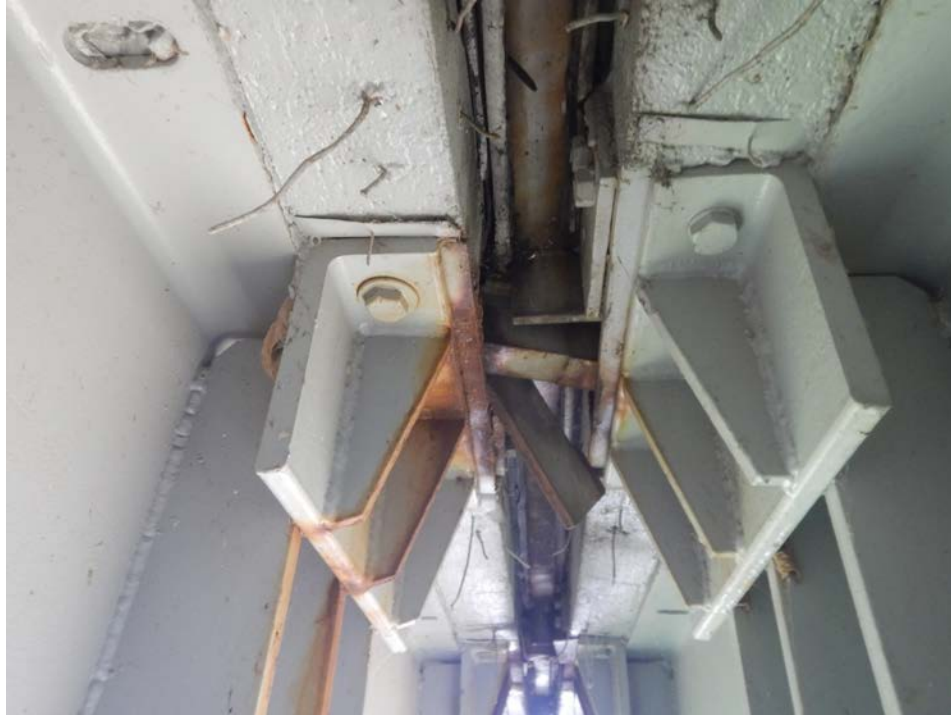
Photograph 13 - Looking south at the underside of the pier 10 modular joint at support box 4. Note: support beam is no longer attached to the transverse support beam and has slid east. South equidistant bar has broken and is wedged in place.
