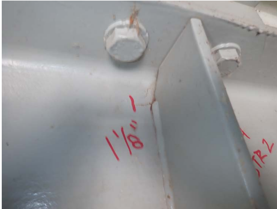
Photograph 17 - Looking northwest at span 4, floor beam 4, stringer 2. Note: no change to 1 1/8-inch-long horizontal crack.
