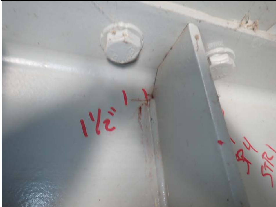
Photograph 14 - Looking northwest at span 4, floor beam 4, stringer 1. Note: no change to 1 1/2-inch-long horizontal crack.
