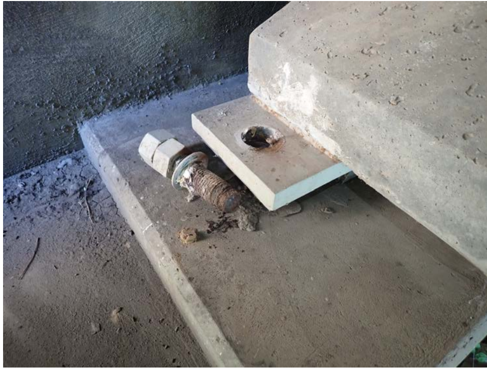
Photograph 39 - Looking northwest at beam 2 at the west abutment. Note: southern bolt is separated from abutment.
