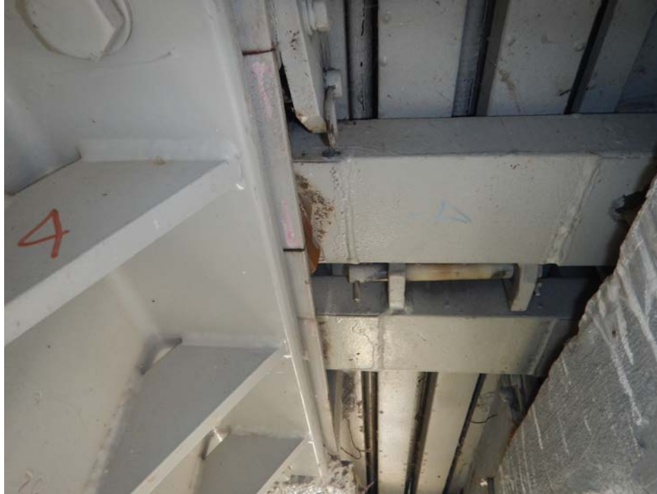
Photograph 5 - Looking south at the underside of the pier 3 modular joint at support box 4. Note: the bottom plate of support box has fractured and support bar 2 is unsupported.
