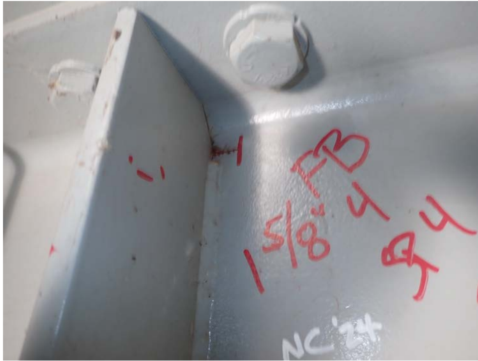
Photograph 15 - Looking southwest at span 4, floor beam 4, stringer 1. Note: no change to 1 5/8-inch-long horizontal crack.
