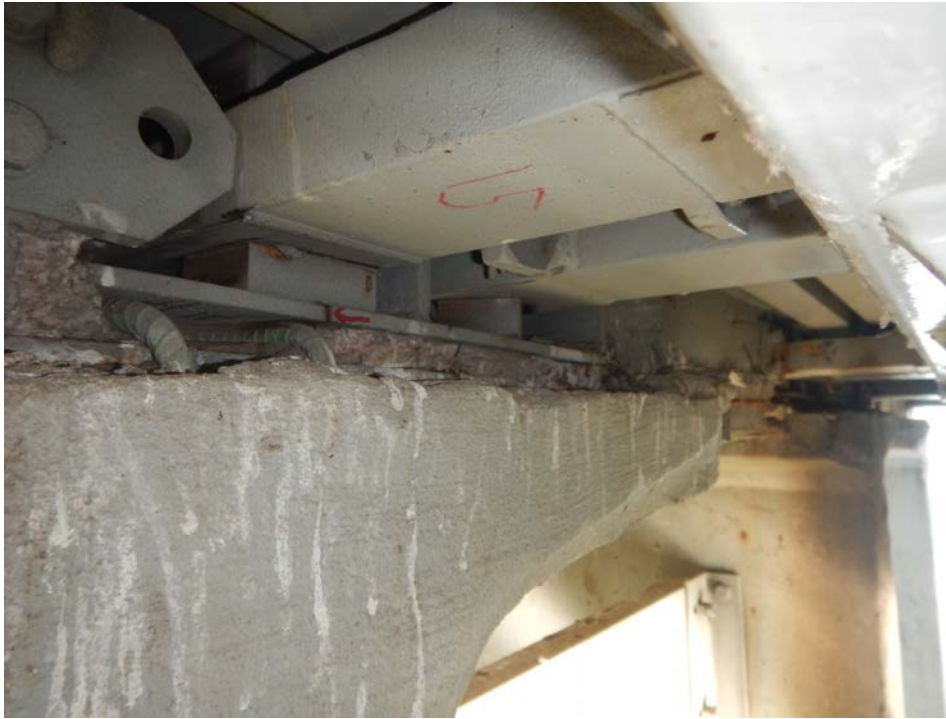
Photograph 9 - Looking west at the underside of the pier 3 modular joint at support box 15. Note: bottom plate of the west support box is fractured beneath the bearing block for support bar 1. Composite reinforcing extending up from beam 10 is exposed with no concrete under support box.
