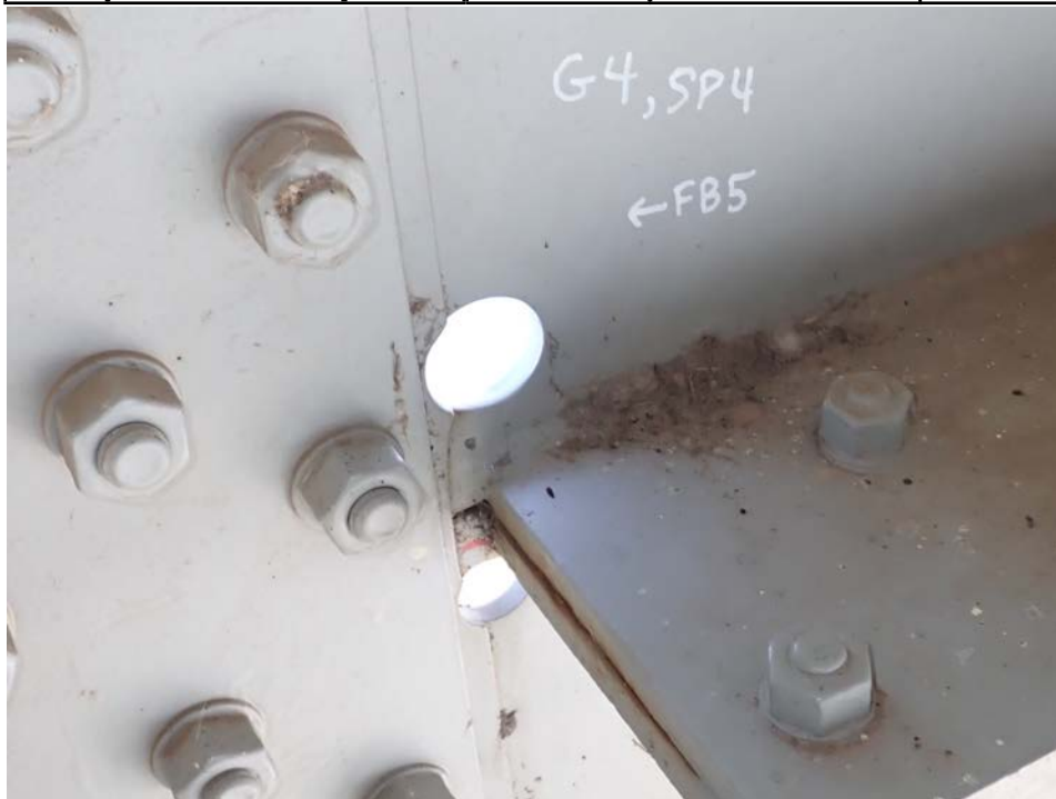
Photograph 24 - Looking northeast at span 4, girder 4, near floor beam 5. Note: no change to 7/16-inch-long crack. No crack apparent in upper web, preventative arrestor hole drilled.
