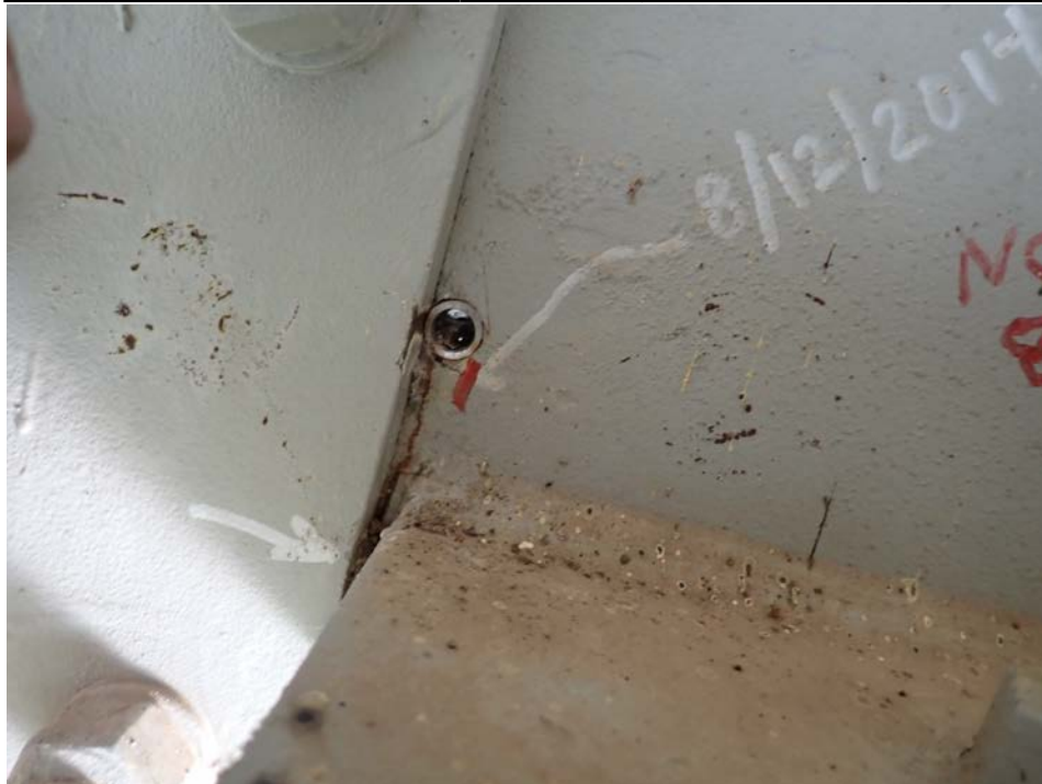
Photograph 26 - Looking north at span 5, girder 2, near floor beam 11. Note: no change to 2-inch-long crack.
