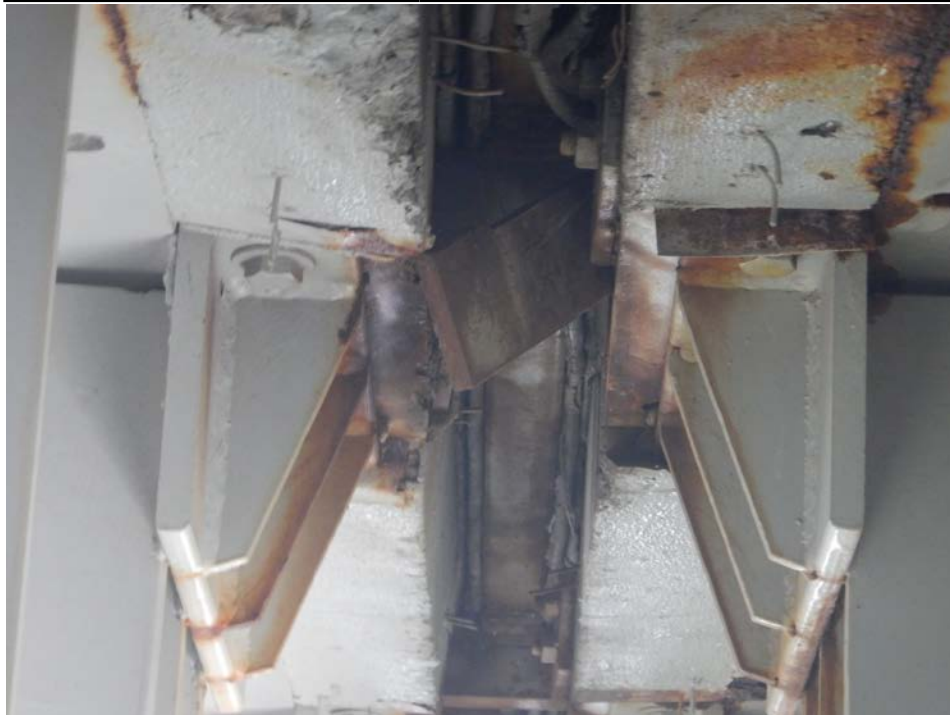
Photograph 12 - Looking north at the underside of the pier 6 modular joint at support box 10. Note: support bar has broken away from the transverse separation beam.
