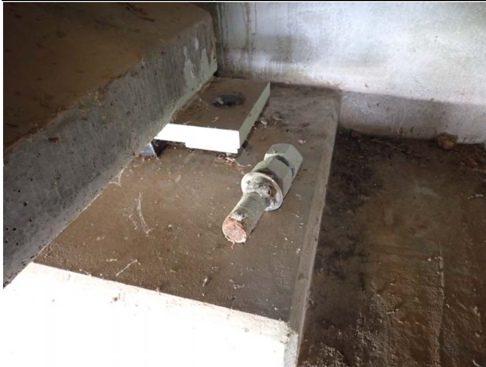
Photograph 40 - Looking west at beam 4 at the west abutment. Note: both bolts separated from abutment.
