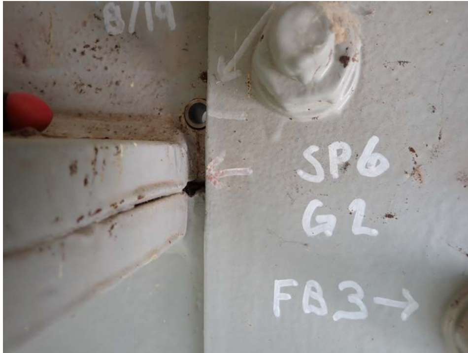
Photograph 31 - Looking north at span 6, girder 2, near floor beam 3. Note: no change to 1-inch-long crack.
