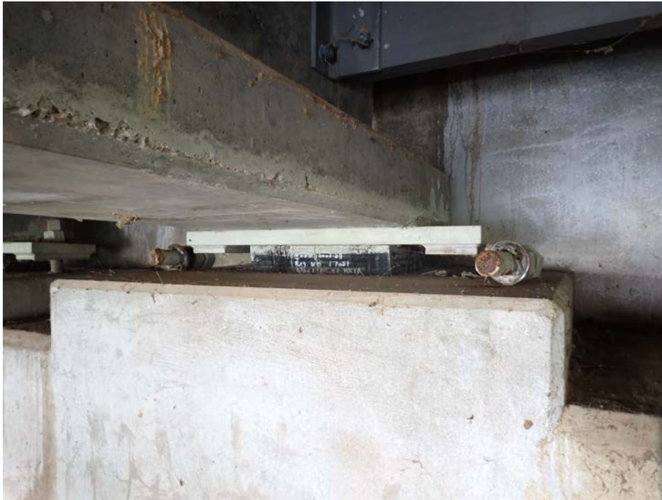
Photograph 41 - Looking west at beam 9 at the west abutment Note: both bolts disconnected from abutment.
