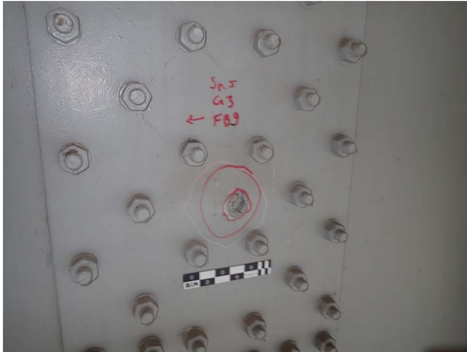
Photograph 35 - Looking south at span 5, girder 3 field splice near floor beam 9. Note: missing bolt with localized deformation.
