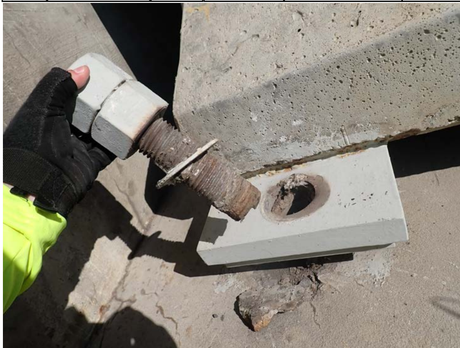
Photograph 38 - Looking north at beam 1 at the west abutment. Note: southern bolt is separated from abutment.
