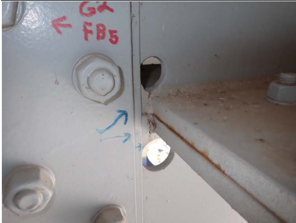
Photograph 23 - Looking northeast at span 4, girder 2, near floor beam 5 at end of longitudinal bolted web splice. Note: no change to upper web 1-inch-long crack or 1 1/2-inch-long crack.
