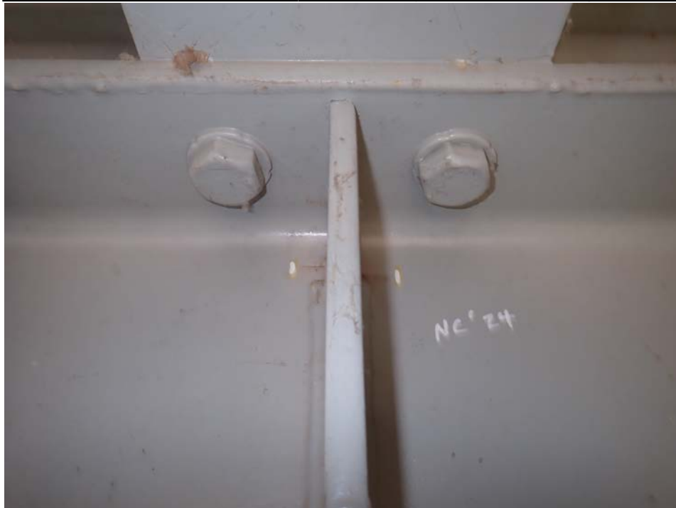
Photograph 16 - Looking east at span 4, floor beam 4, stringer 1. Note: cracks have now daylighted through to west face of web.
