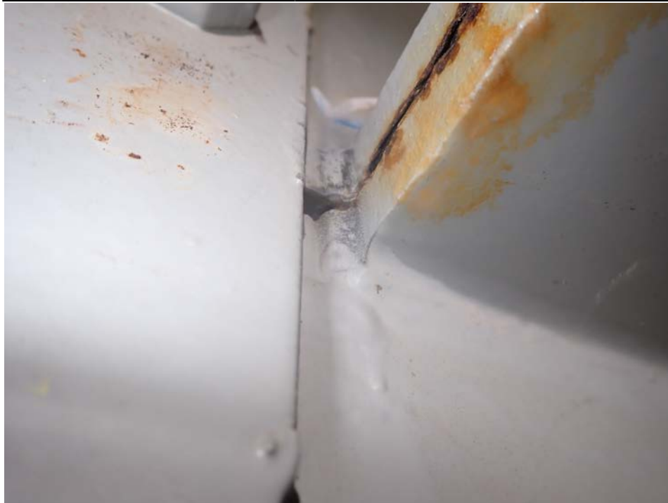
Photograph 32 - Looking south at span 6, girder 3 near floor beam 3. Note: paint cracks previously noted, no cracks found.
