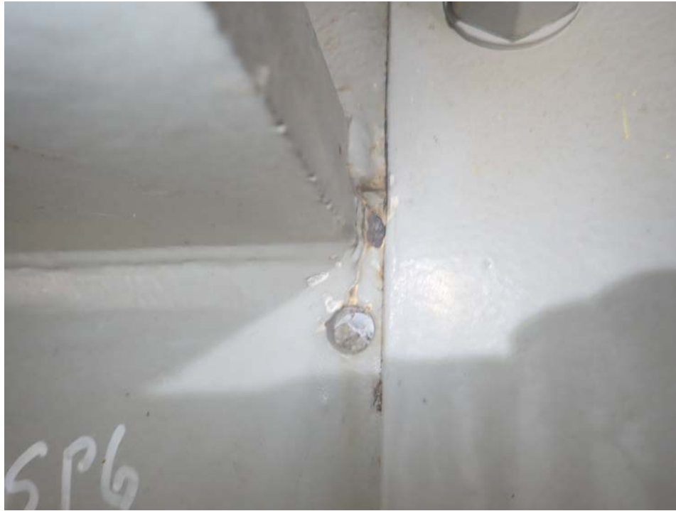
Photograph 33 - Looking north at span 6, girder 4, near floor beam 3. Note: no change to the 1 1/4-inch-long crack.
