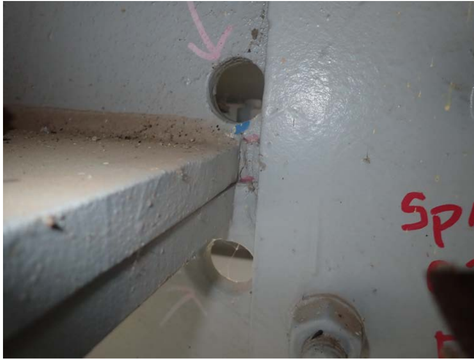
Photograph 27 - Looking south at span 5, girder 3, near floor beam 11. Note: no change to 7/8-inch-long crack.
