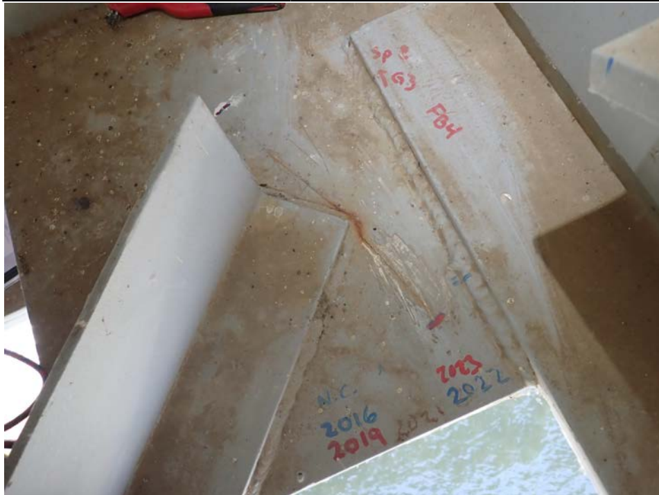
Photograph 20 - Looking southwest at span 8, girder 3 at floor beam 4. Note: no change to 8 1/2-inch-long crack in gusset plate.
