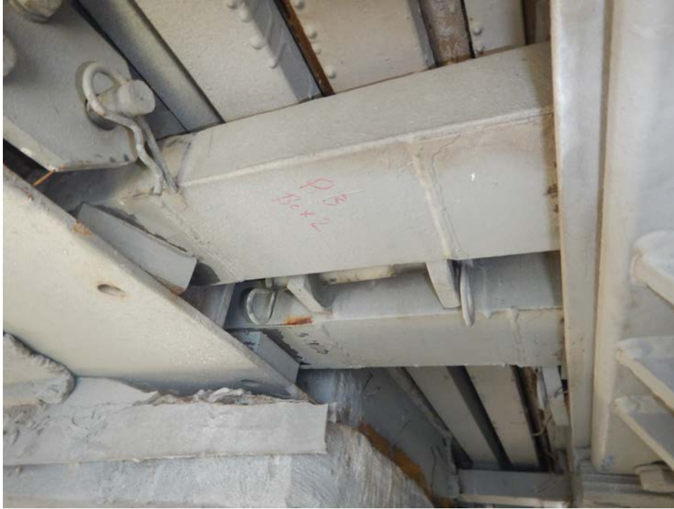
Photograph 3 - Looking northwest at the underside of the pier 3 modular joint at support box 2. Note: bottom plate of the support box is unsupported along the end of span 3. Equidistant spring between support bars is missing (typical).
