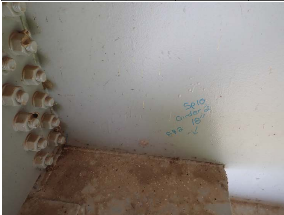
Photograph 21 - Looking north at span 10, girder 2 at floor beam 2. Note: no change to 18-inch-long crack in gusset plate weld.
