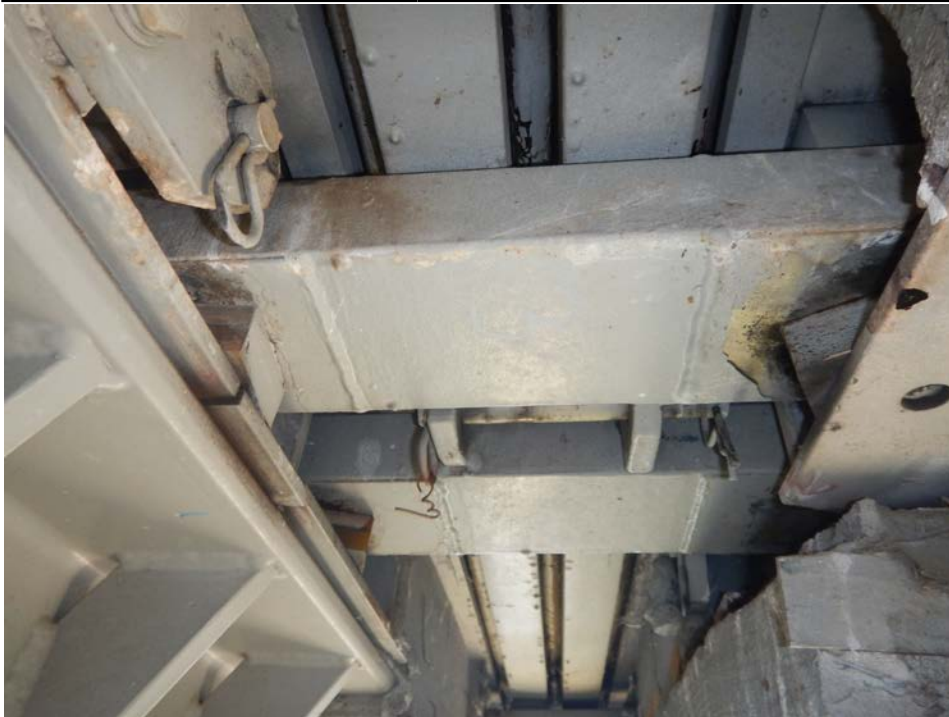
Photograph 4 - Looking south at the underside of the pier 3 modular joint at support box 3. Note: bottom plate of support box has fractured and west end of support bar 1 is unsupported. Bearing block for support bar 2 is dislodged. Stainless steel sliding surface is painted.
