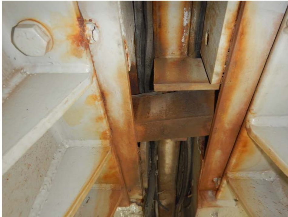
Photograph 11 - Looking south at the underside of the pier 6 modular joint at support box 3. Note: support bar has broken away from the transverse separation beam.
