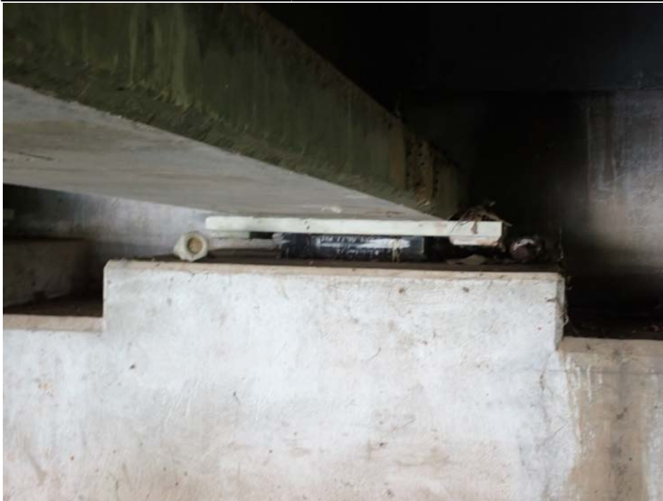
Photograph 42 - Looking west at beam 12 at the west abutment. Note: both nuts separated from abutment.
