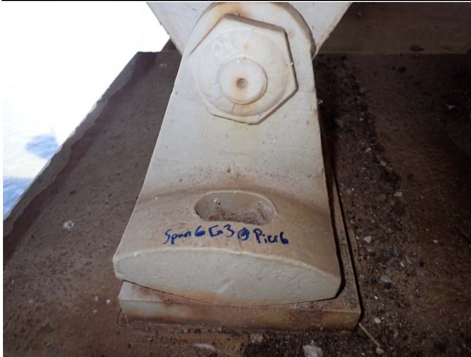
Photograph 37 - Looking north at span 6, girder 3 rocker bearing at pier 6. Note: outboard anchor rod is missing.
