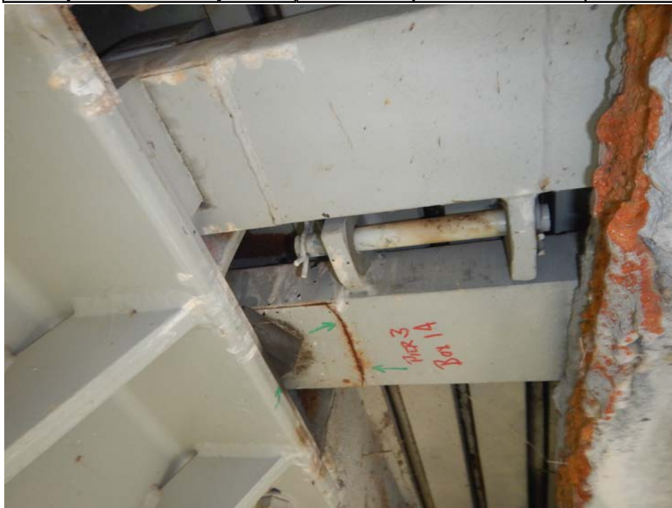
Photograph 8 - Looking south at the underside of the pier 3 modular joint at support box 14. Note: stainless steel plate welded to support bar 1 at the east bearing box has fractured near the west weld.
