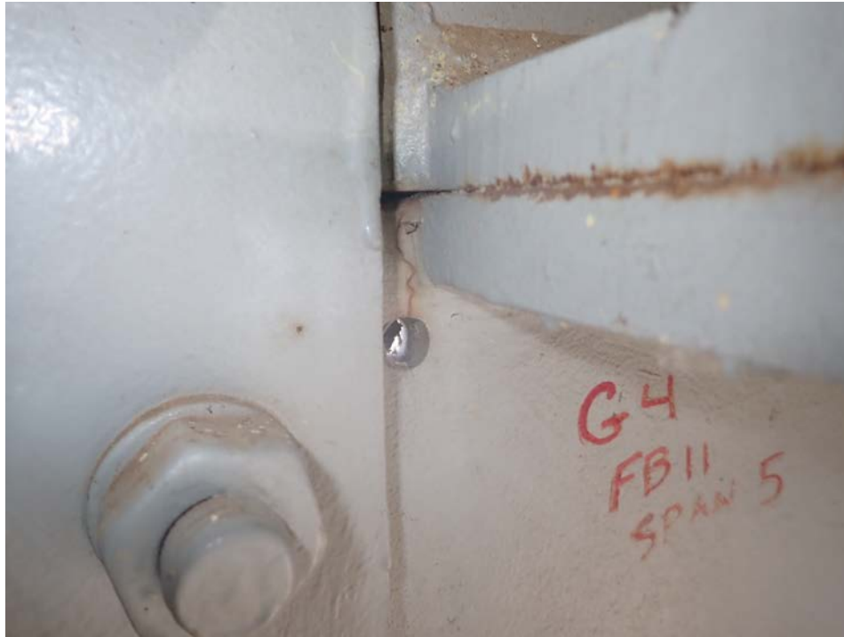
Photograph 29 - Looking northeast at span 5, girder 4, near floor beam 11. Note: no change to 1-inch-long crack.
