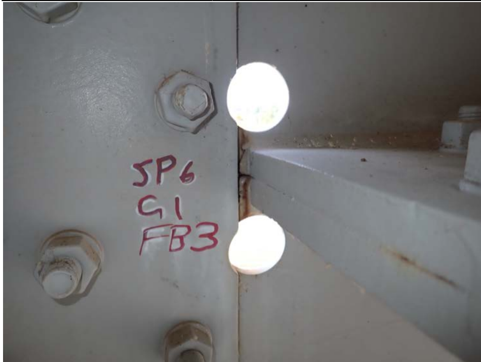
Photograph 30 - Looking south at span 6, girder 1, near floor beam 3. Note: no change to both cracks arrested by a cored hole.
