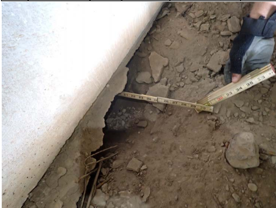
Photograph 44 - Looking west at the west abutment beneath beam 5. Note: undermining up to 20 inches.
