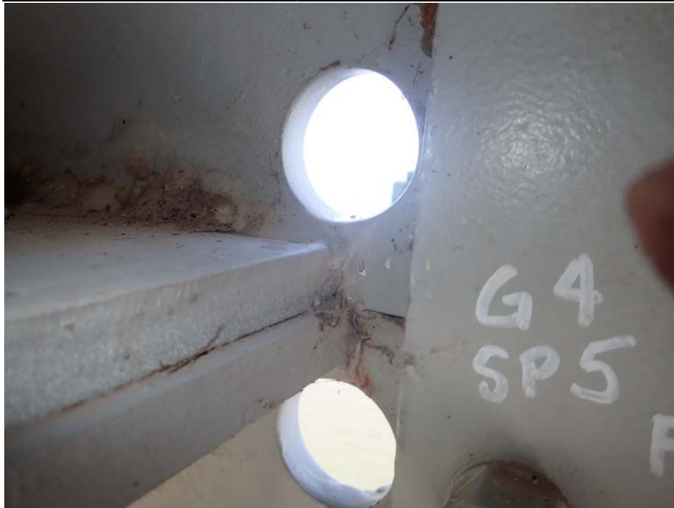
Photograph 28 - Looking north at span 5, girder 4, near floor beam 3. Note: no change to 1 1/8-inch-long crack or 1-inch-long crack.
