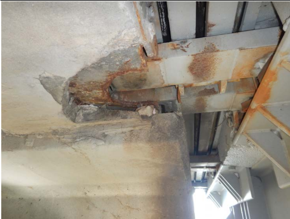
Photograph 10 - Looking north at the underside of the pier 3 modular joint at support box 16. Note: bottom plate of the west support box has fractured away and the west end of support bar 1 is unsupported.
