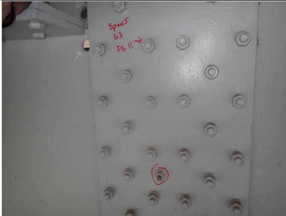
Photograph 34 - Looking south at span 6, girder 3 field splice near floor beam 11. Note: missing bolt.
