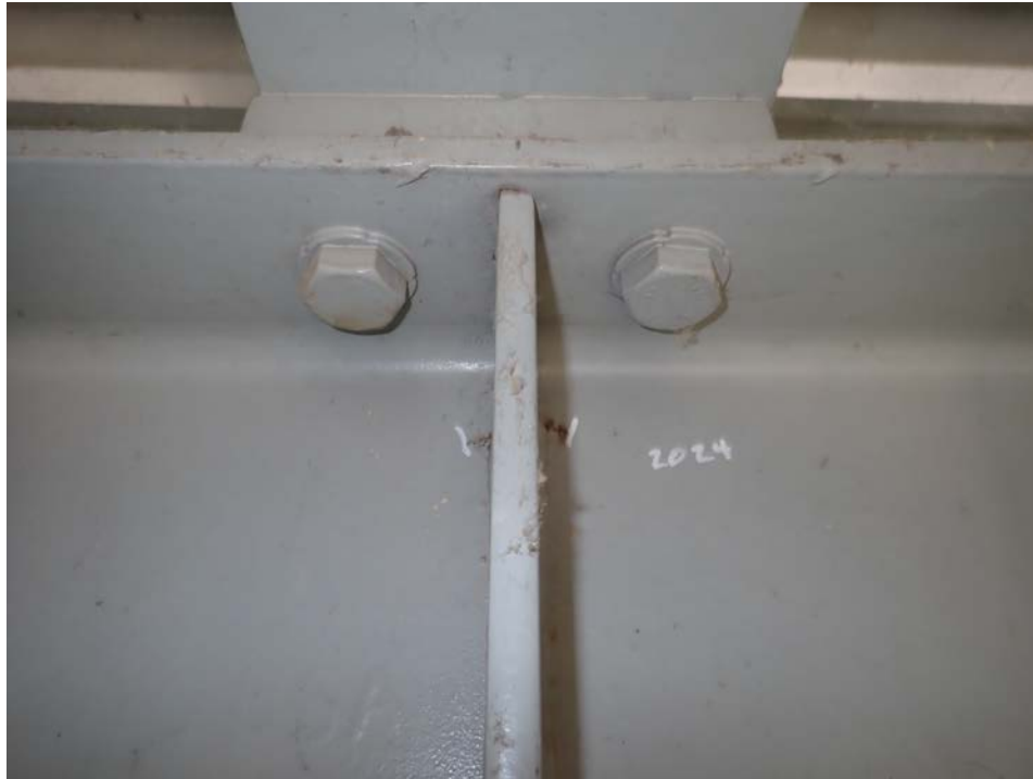
Photograph 19 - Looking east at span 4, floor beam 4, stringer 2. Note: cracks have now daylighted through to west face of web.
