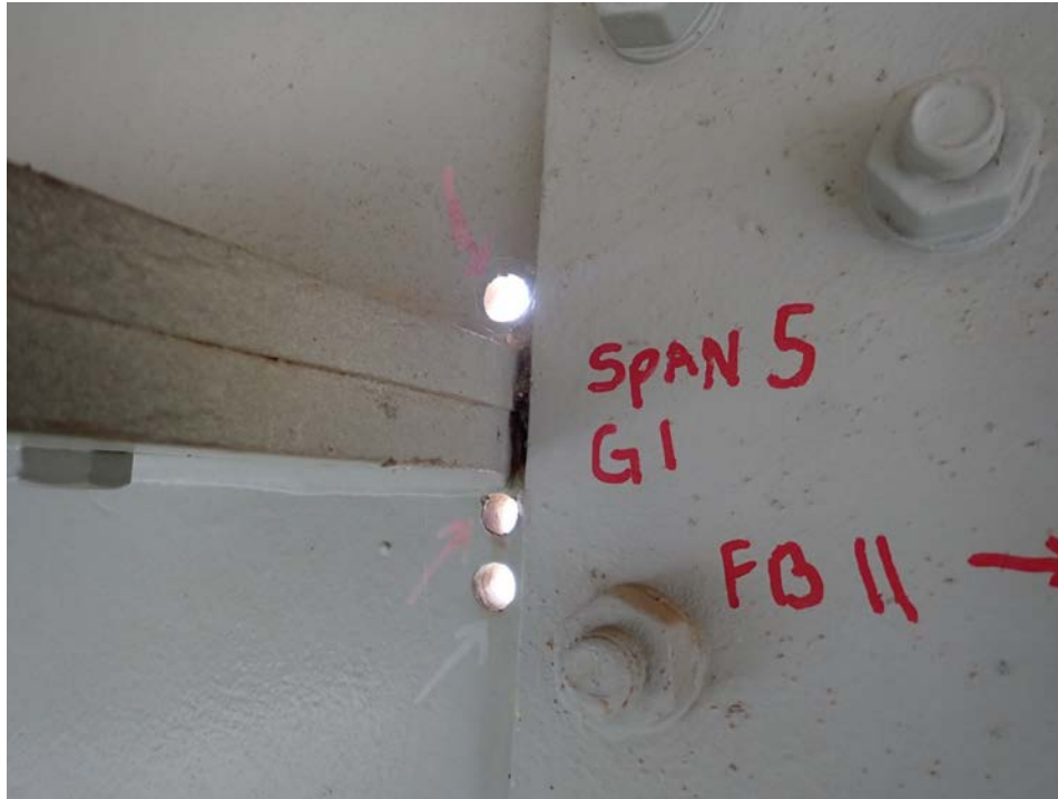
Photograph 25 - Looking south at span 5, girder 1, near floor beam 11. Note: no change to 3/4-inch-long crack or 1 1/4-inch-long crack.
