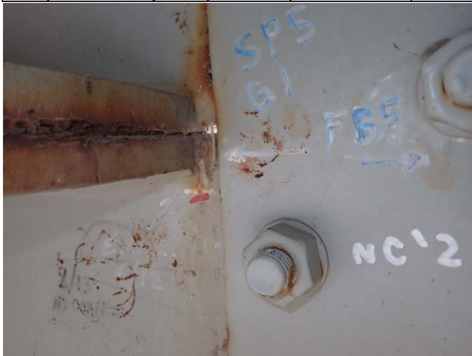
Photograph 4 - Looking southeast at span 5, girder 1 at the field splice near floor beam 5. Note: 5/8 inch-long crack in the inboard face at the horizontal web splice termination, no change.
