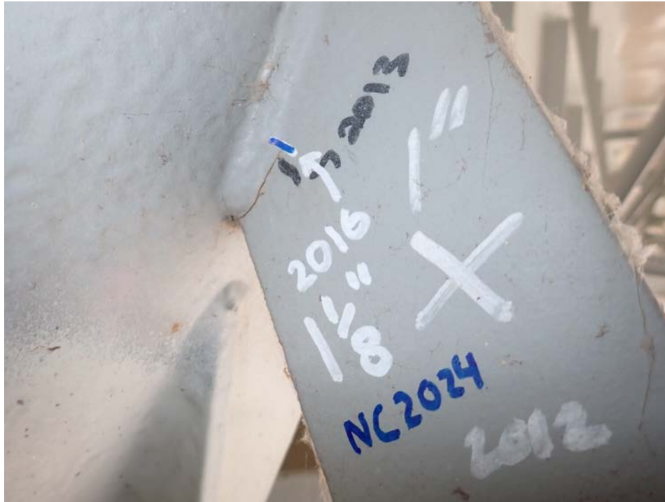
Photograph 21 - Looking east at the span 7, floor beam 0 lower strut connection to girder 2 at pier 6. Note: No change to 1 1/8-inch-long crack in repair plate weld on the west face and no change to the 1/2-inch-long crack on the east face.
