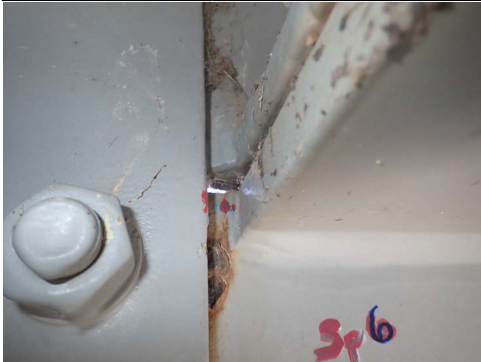
Photograph 10 - Looking northwest at span 6, girder 2 at the field splice near floor beam 11. Note: No change to 3/16-inch-long crack in the inboard face at the horizontal web splice termination.
