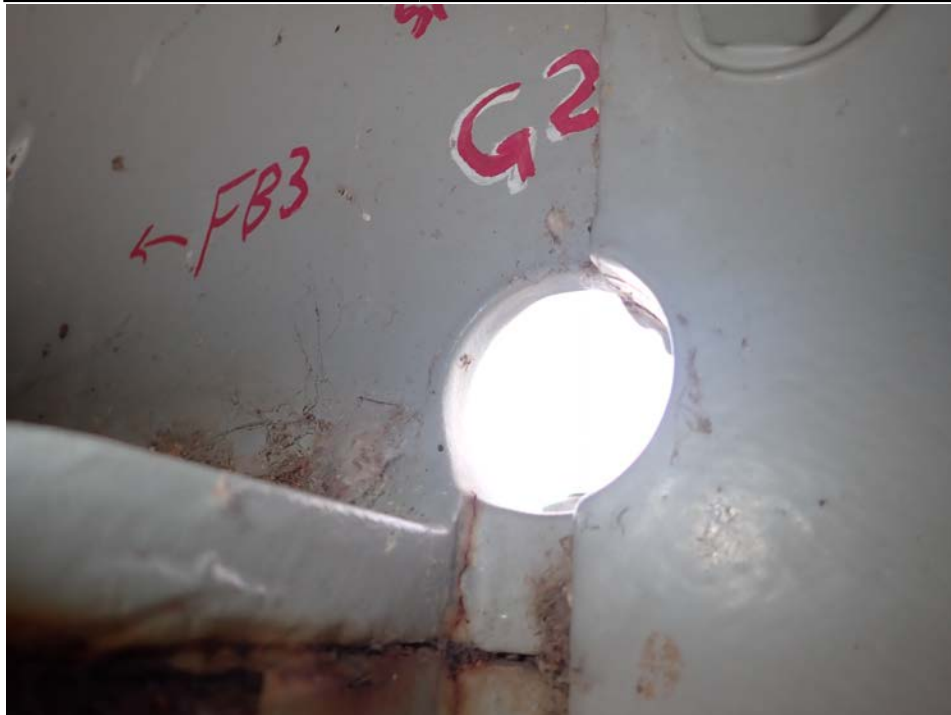
Photograph 12 - Looking north at span 7, girder 2 at the field splice near floor beam 4. Note: 2 arrested cracks, no propagation across the hole.
