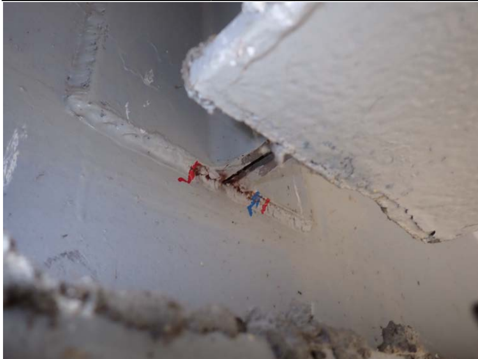
Photograph 16 - Looking west at span 7, stringer 1 connection to floor beam 0. Note: No change to the 3 1/2-inch-long crack along weld on the bottom of the stringer connection angles.
