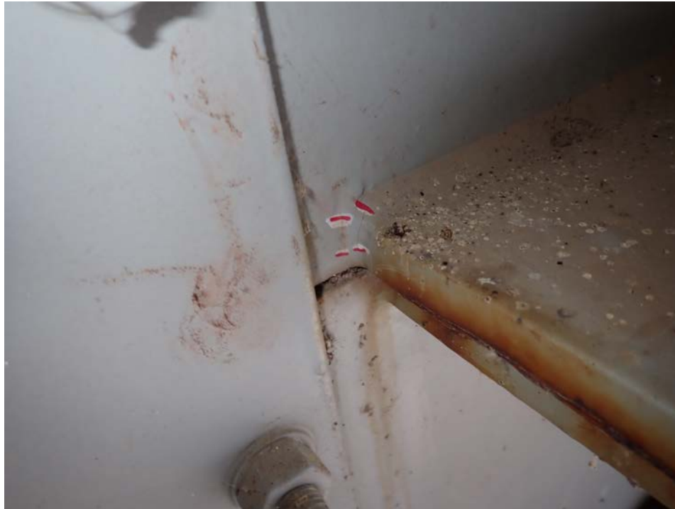
Photograph 5 - Looking northeast at span 5, girder 2 at the field splice near floor beam 5. Note: Two 3/8 inch-long paint cracks in the inboard face at the horizontal web splice termination, no change.
