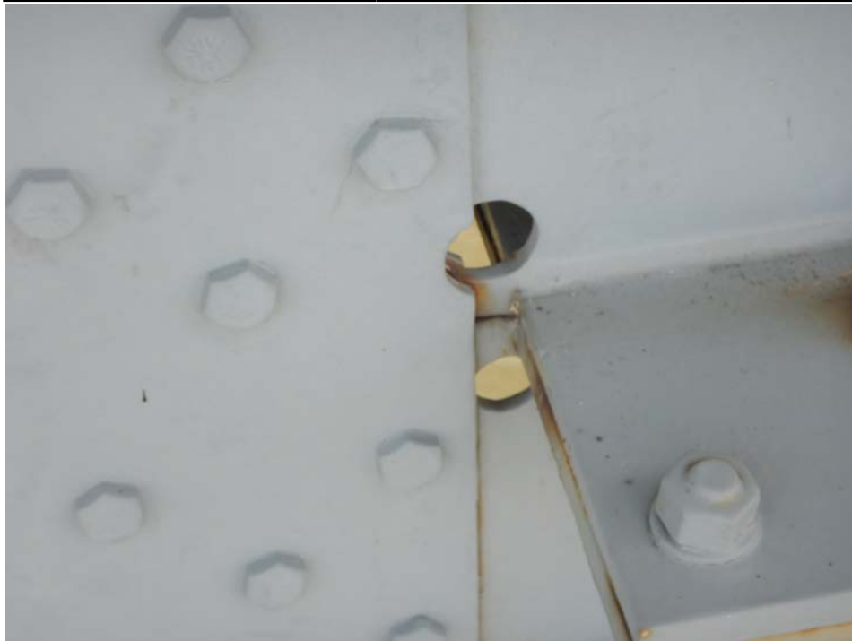
Photograph 14 - Looking south at span 7, girder 2 outboard near floor beam 4 at field splice. Note: Crack with arrestor holes.
