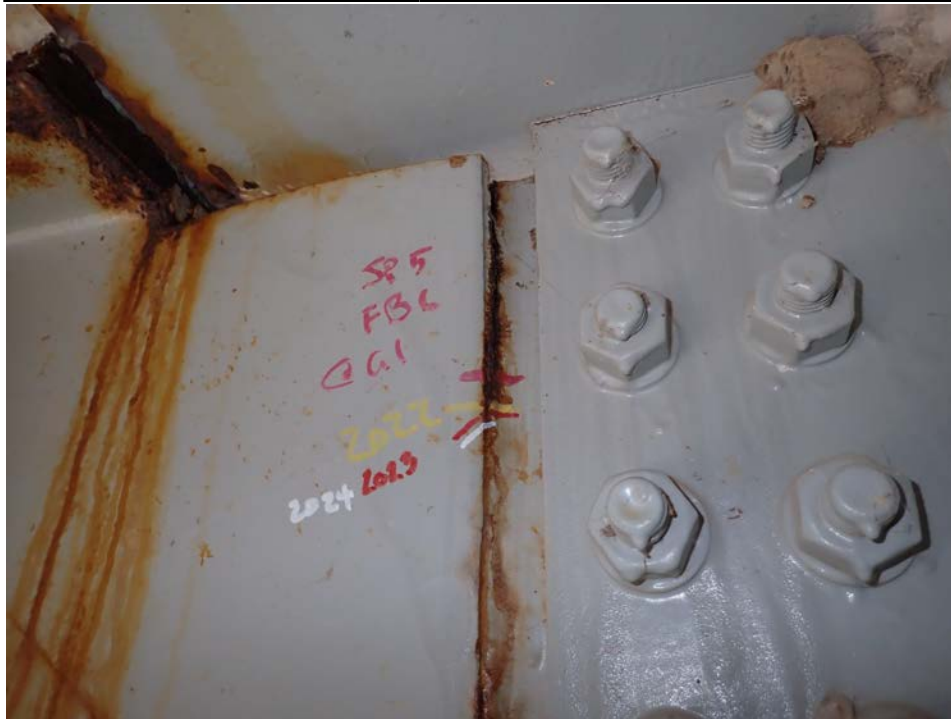
Photograph 19 - Looking east at span 5, floor beam 6 upper connection to girder 1. Note: 5 1/2-inch-long crack in connection plate weld, 3/8-in growth.
