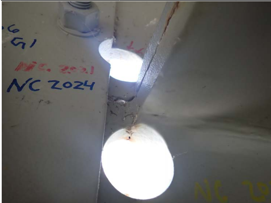
Photograph 6 - Looking south at span 6 girder 1, end of horizontal filed splice near floor beam 3. Note: 3/4-inch-long crack in the inboard face at the horizontal web splice termination has not propagated past the arrestor holes. Also note, 1/2-inch-long paint cracks along the top of the upper arrestor hole.
