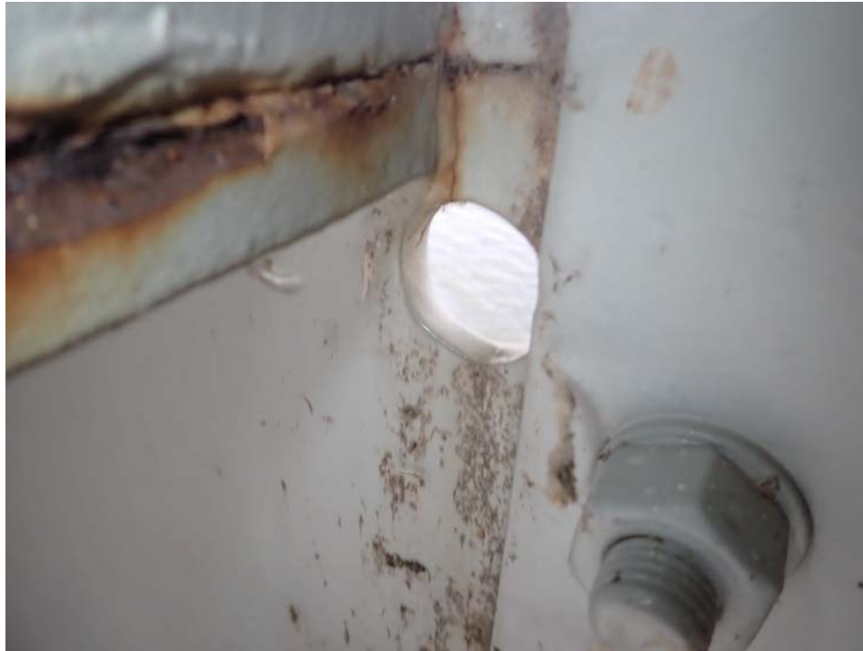
Photograph 13 - Looking north at span 7, girder 2 at the field splice near floor beam 4. Note: 2 arrested cracks, no propagation across the hole.
