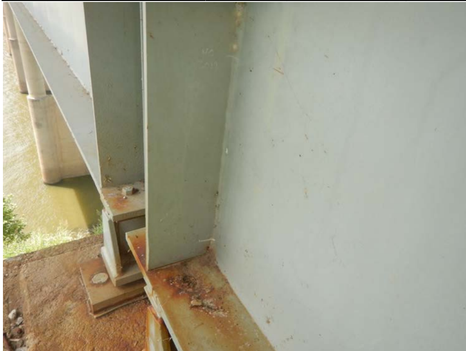
Photograph 18 - Looking northwest at span 15, girder 1 outboard at pier 14. Note: Crack in weld for vertical stiffener.
