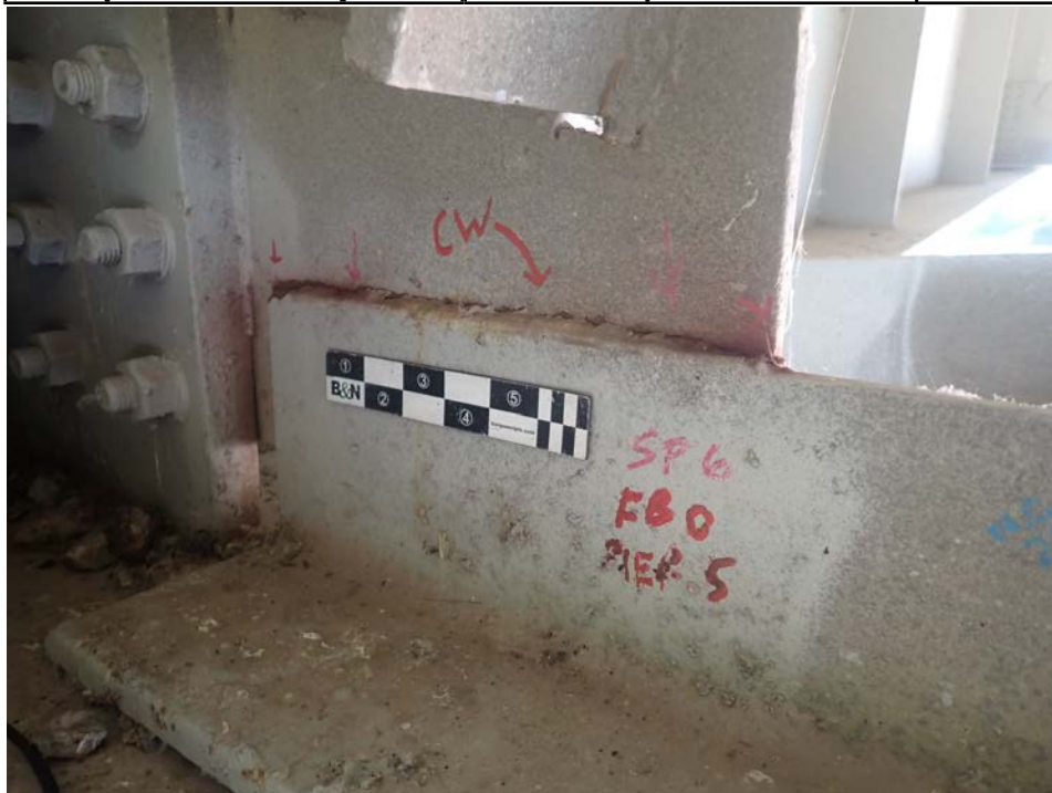
Photograph 20 - Looking northeast at span 6, floor beam 0 lower strut connection to girder 2 at pier 5. Note: Full-length horizontal crack in the weld.
