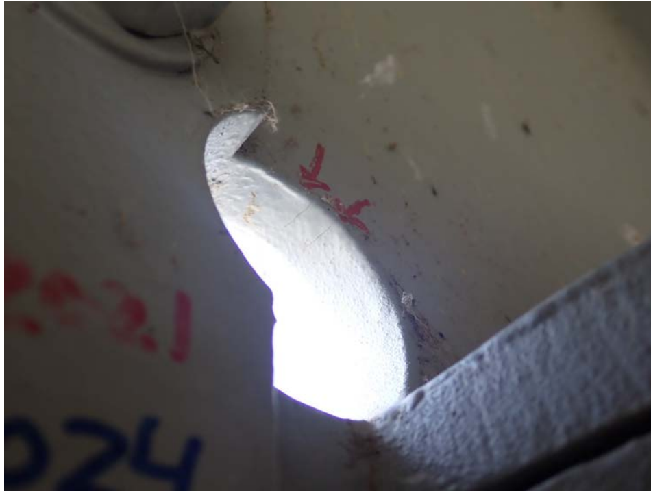
Photograph 7 - Looking southwest at span 6 girder 1, end of horizontal filed splice near floor beam 3. Note: 3/4-inch-long crack in the inboard face at the horizontal web splice termination has not propagated past the arrester holes. 1/2-inch-long paint cracks along the top of the upper arrester
