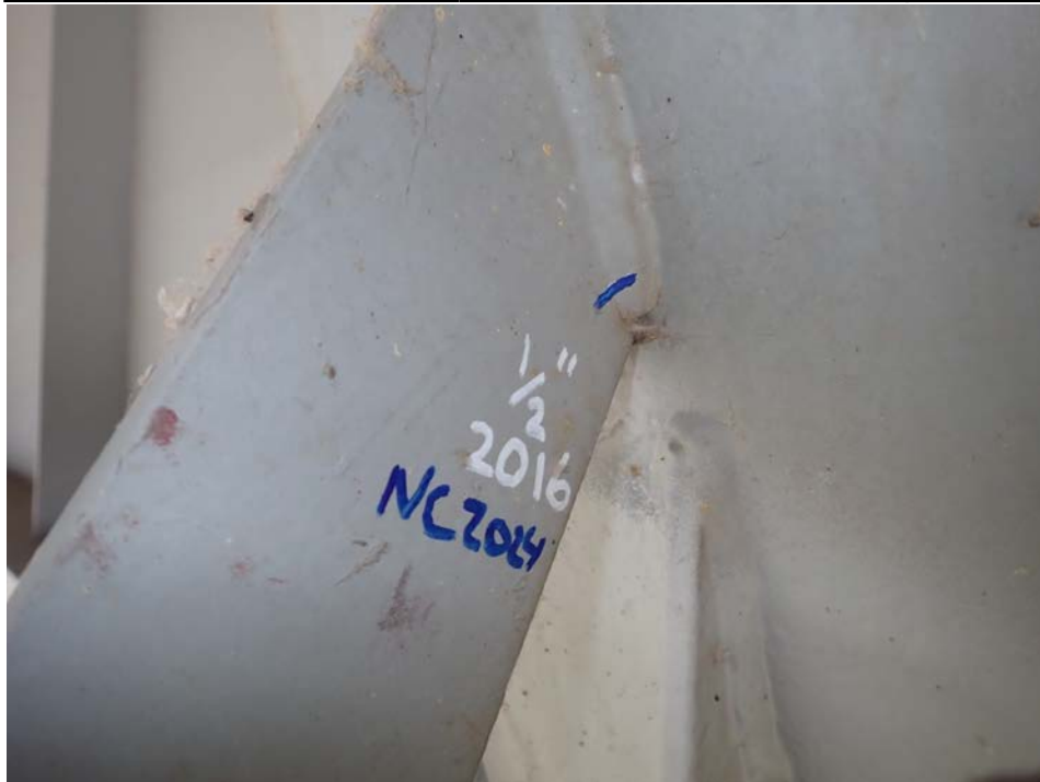
Photograph 22 - Looking west at the span 7, floor beam 0 lower strut connection to girder 2 at pier 6. Note: No change to 1 1/8-inch-long crack in repair plate weld on the west face and no change to the 1/2-inch-long crack on the east face.
