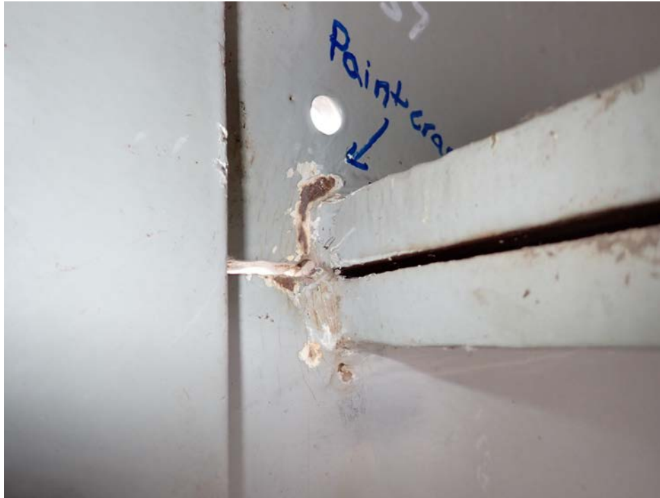
Photograph 11 - Looking south at span 7, girder 1 at the field splice near floor beam 4. Note: 1 inch-long paint crack in the upper web with an arrestor hole, and a 1 1/8-inch-long paint crack in the lower web without an arrestor hole in the inboard face at the horizontal web splice termination.
