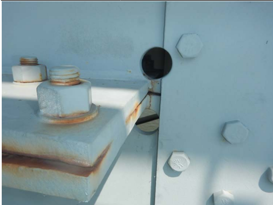
Photograph 8 - Looking north at span 6, girder 1 outboard near floor beam 3 at field splice. Note: crack with arrester holes.
