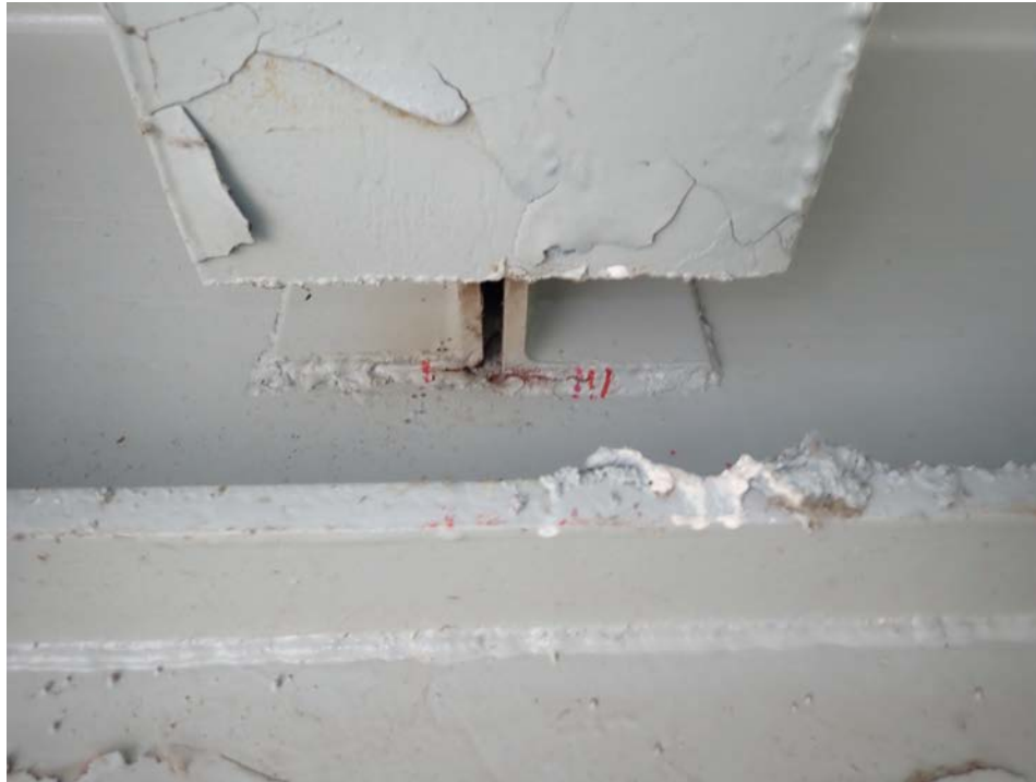
Photograph 15 - Looking west at span 5, stringer 3 connection to floor beam 3 (east face), span 5. Note: 3 1/2-inch long crack along weld on the underside of the stringer connection angles, no change.
