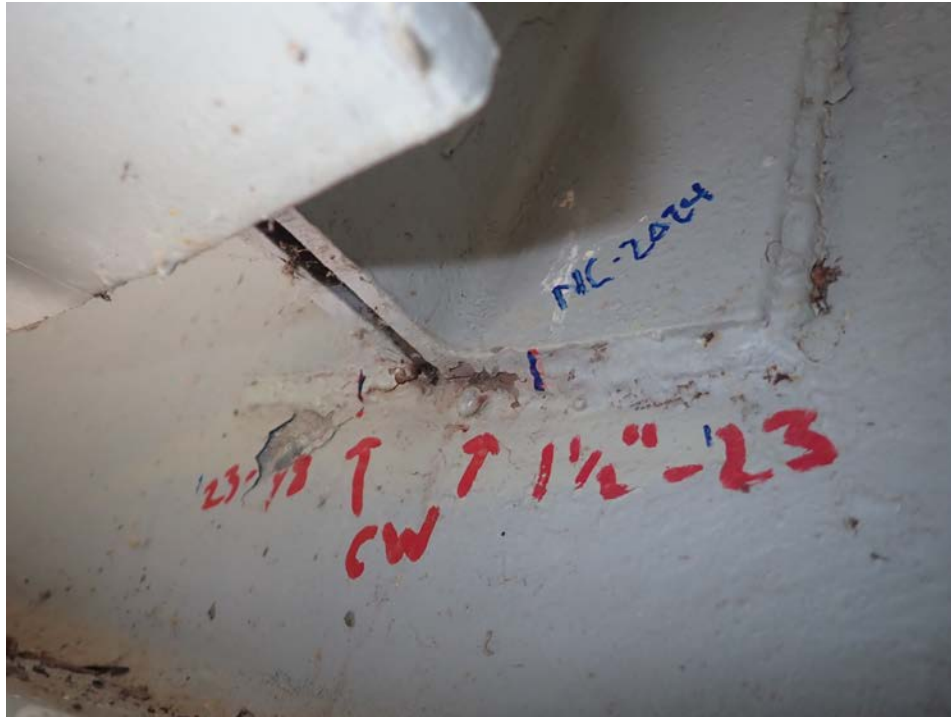
Photograph 17 - Looking west at span 7, stringer 3 connection to floor beam 0. Note: No change to the 1/2-inch and 7/8-inch-long cracks in the weld on the bottom of the stringer connection angles.
