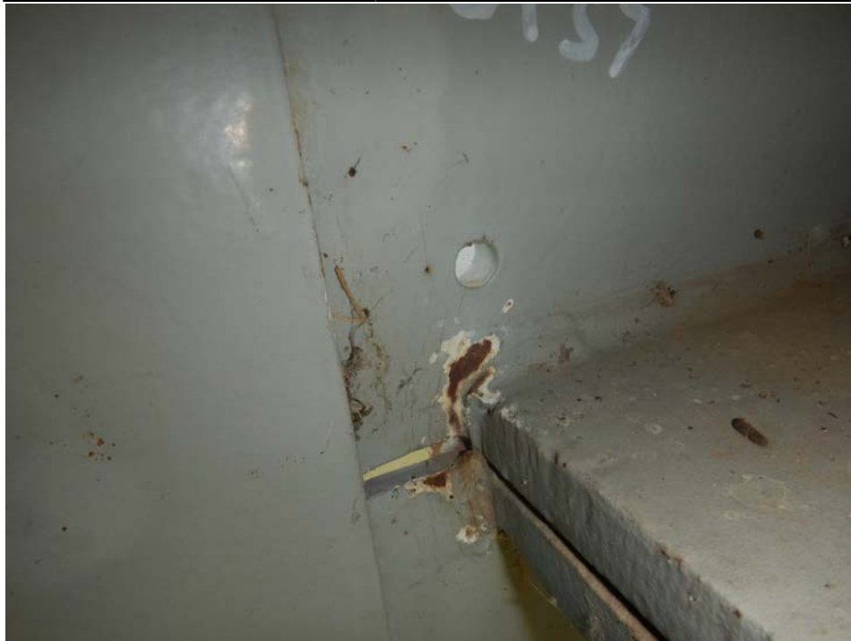
Photograph 24 - Looking southwest at girder 1, span 7 at the field splice near floor beam 4. Note: 1-inch-long paint crack in the upper web with an arrestor hole, and a 1 1/8-inch-long paint crack in the lower web without an arrestor hole in the inboard face at the horizontal web splice termination.
