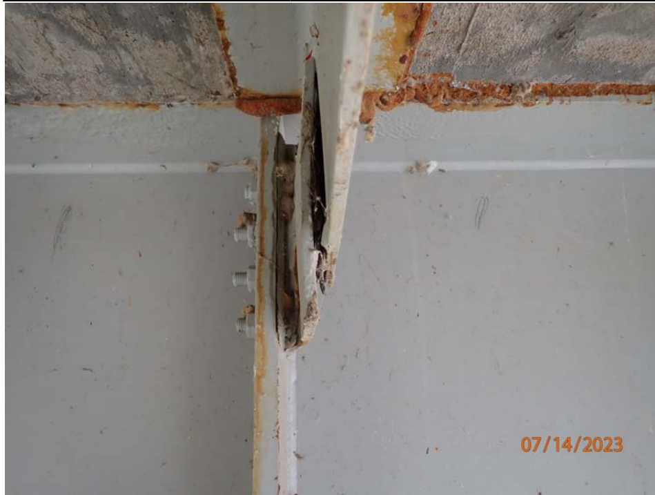
Photograph 33 - Looking south at cross frame connection to girder 3 over pier 12. Note: crack in gusset plate to cross frame connection due to pack rust.
