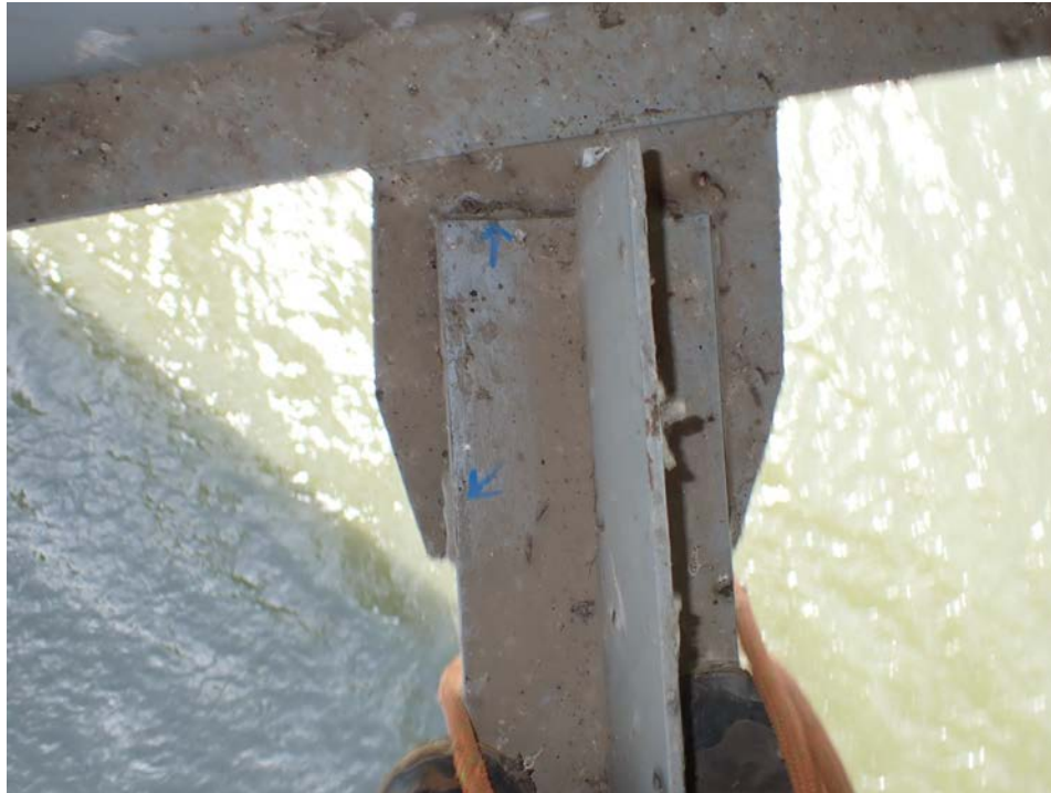
Photograph 55 - Looking southeast at span 6, lower lateral bracing crossbuck connection between floor beams 10 and 11. Note: 2 cracked welds on northeast member due to pack rust.
