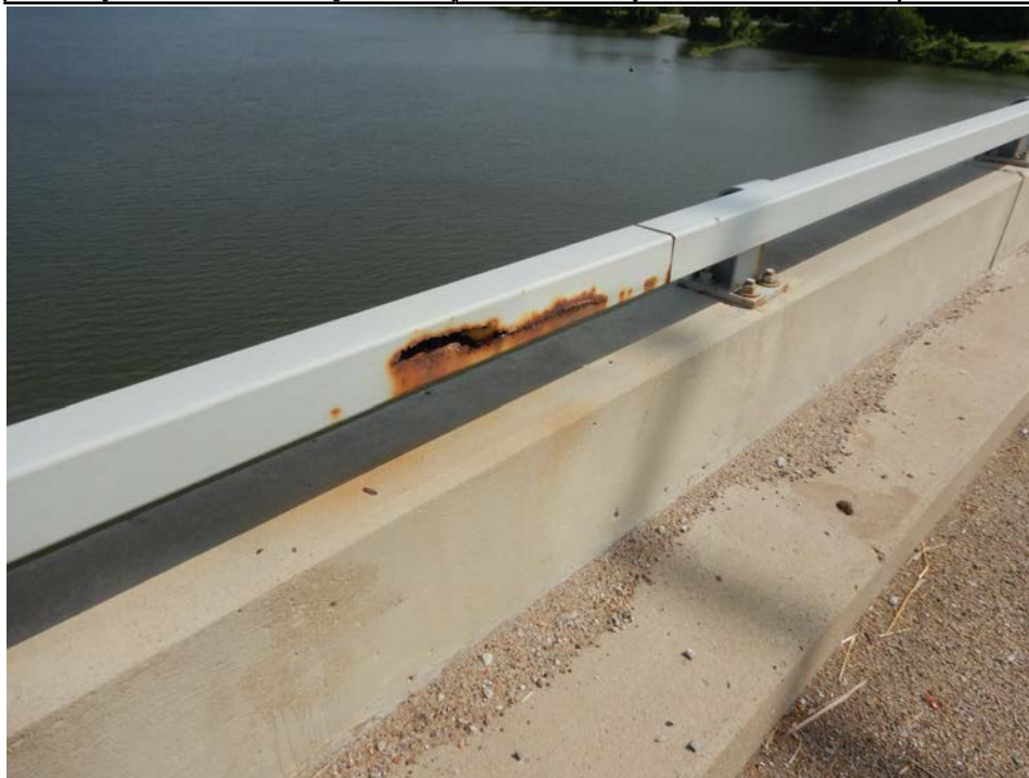
Photograph 4 - Looking northeast at the north bridge railing in span 6 near pier 6. Note: corrosion hole through rail.
