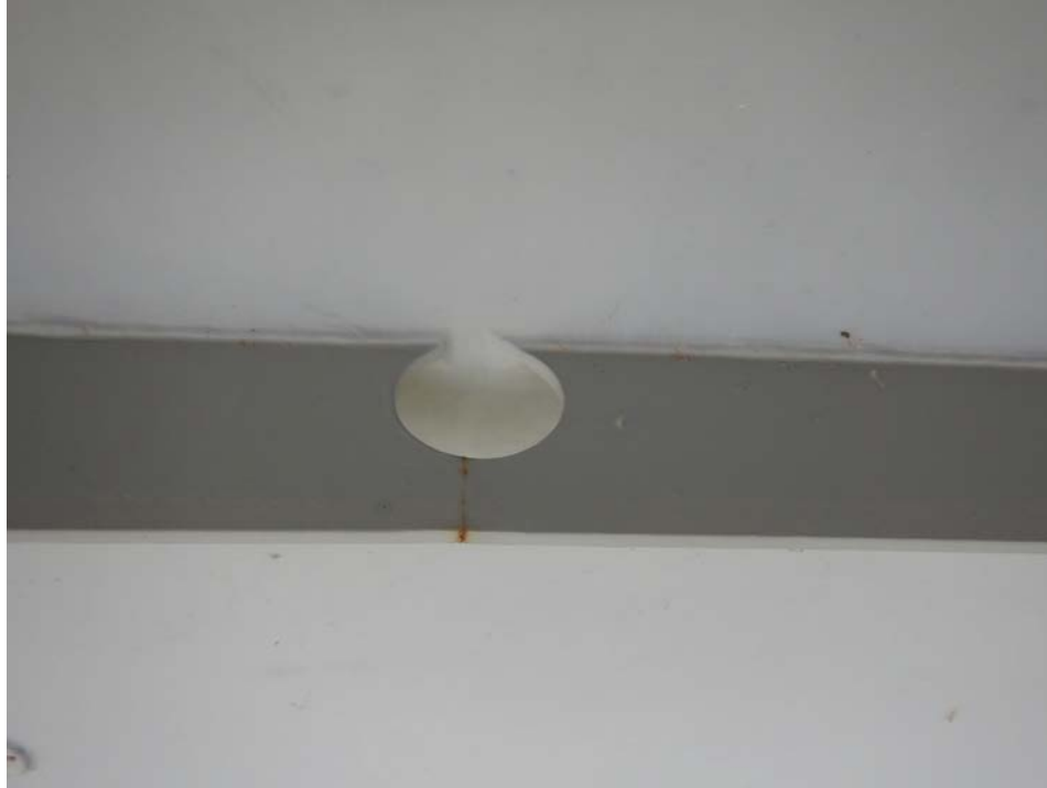
Photograph 29 - Looking north at girder 1, span 6 at the upper longitudinal stiffener splice near floor beam 7. Note: crack in splice on free edge side of cored hole.
