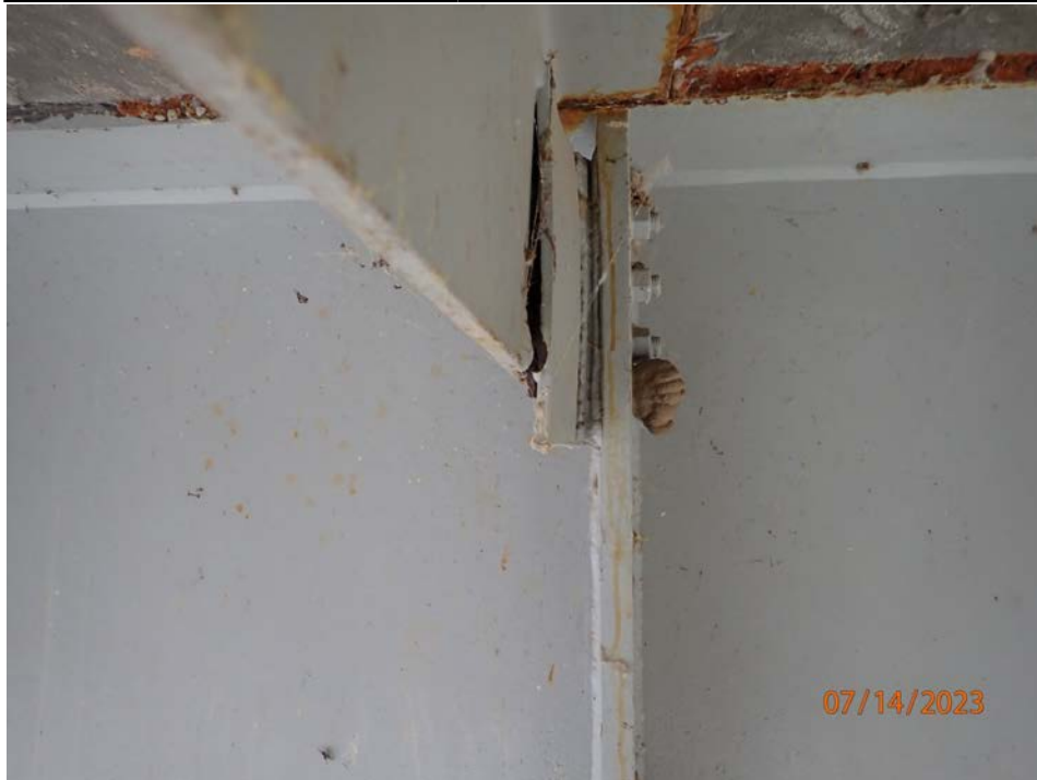
Photograph 32 - Looking north at cross frame connection to girder 2 over pier 12. Note: full-length crack in gusset plate to cross frame connection due to pack rust.
