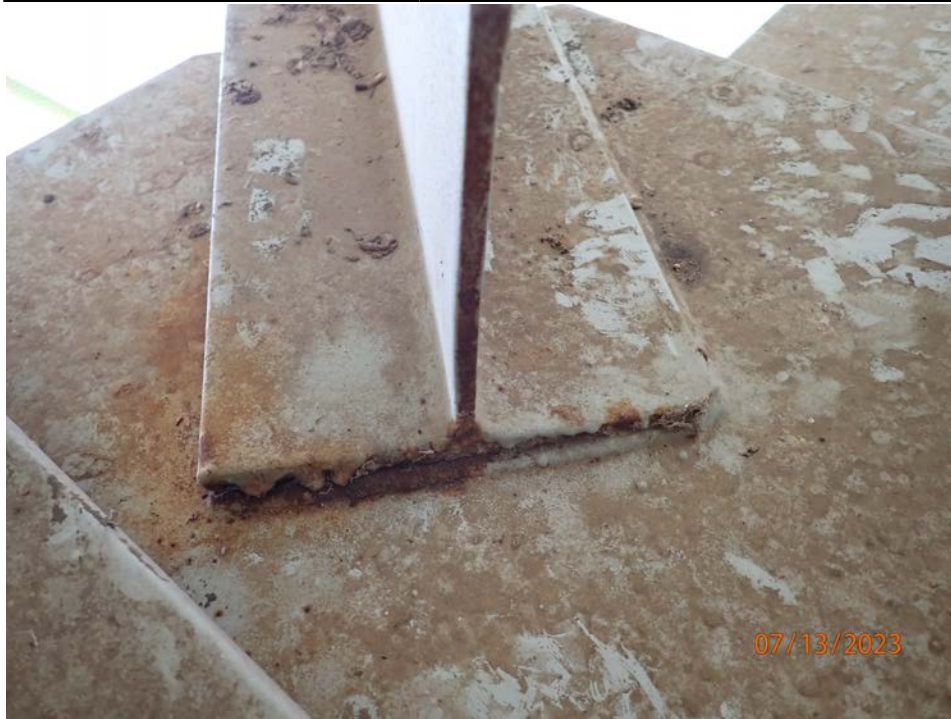
Photograph 53 - Looking southwest at the lower lateral bracing connection to floor beam 1 and girder 2, span 5. Note: bracing is welded along the west edge and end allowing pack rust to form and crack weld at end of bracing.
