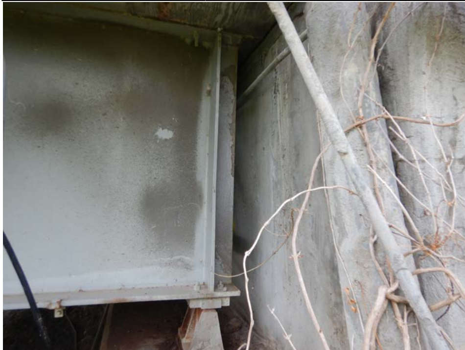
Photograph 58 - Looking south at girder 4, span 1 at the west abutment. Note: backwall is leaning towards the channel with 4 7/8 inches clear to the girder end near the top flange and 7 inches clear near the bottom flange.
