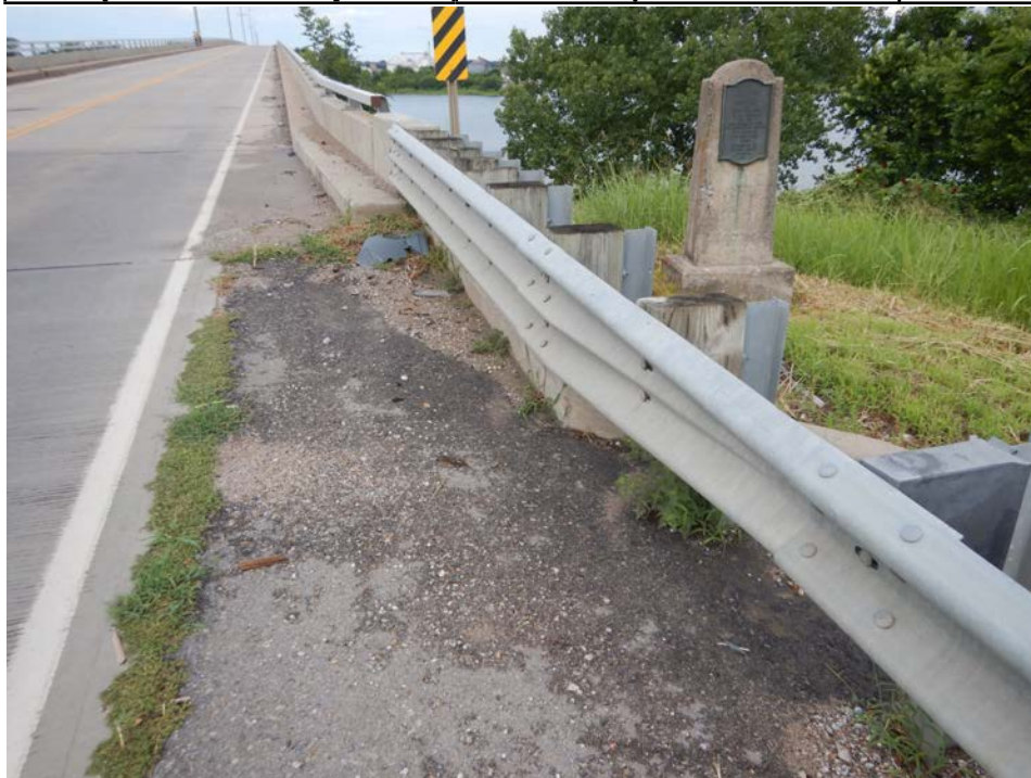
Photograph 8 - Looking west at the northeast approach railing transition. Note: transition meets current standards; however, safety curb extends 14 inches from face of railing and is unprotected.
