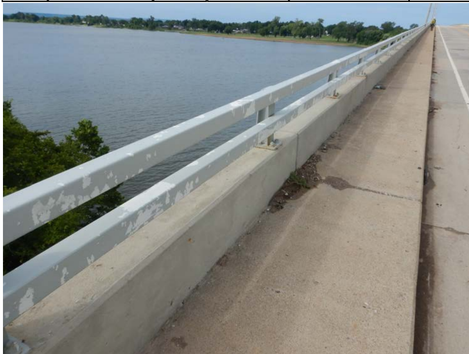
Photograph 6 - Looking southwest at the south bridge railing in span 14. Note: top coat of paint is peeling due to adhesion failure.
