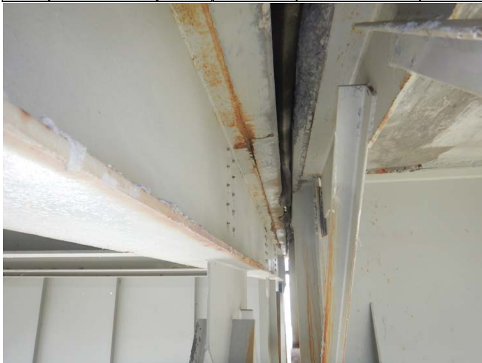
Photograph 18 - Looking north along the underside of the finger joint over pier 7. Note: trough torn and falling through along the underside.
