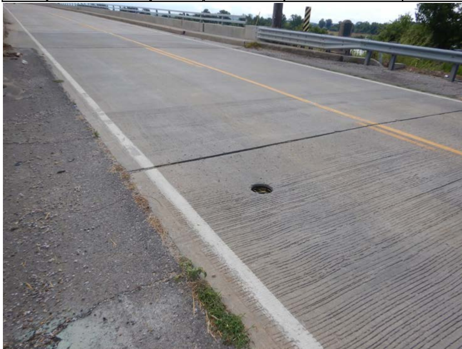
Photograph 74 - Looking southeast at the west approach roadway. Note: 7 1/2-inch diameter filled core hole exists in the westbound lane approximately 40 feet from the west abutment.
