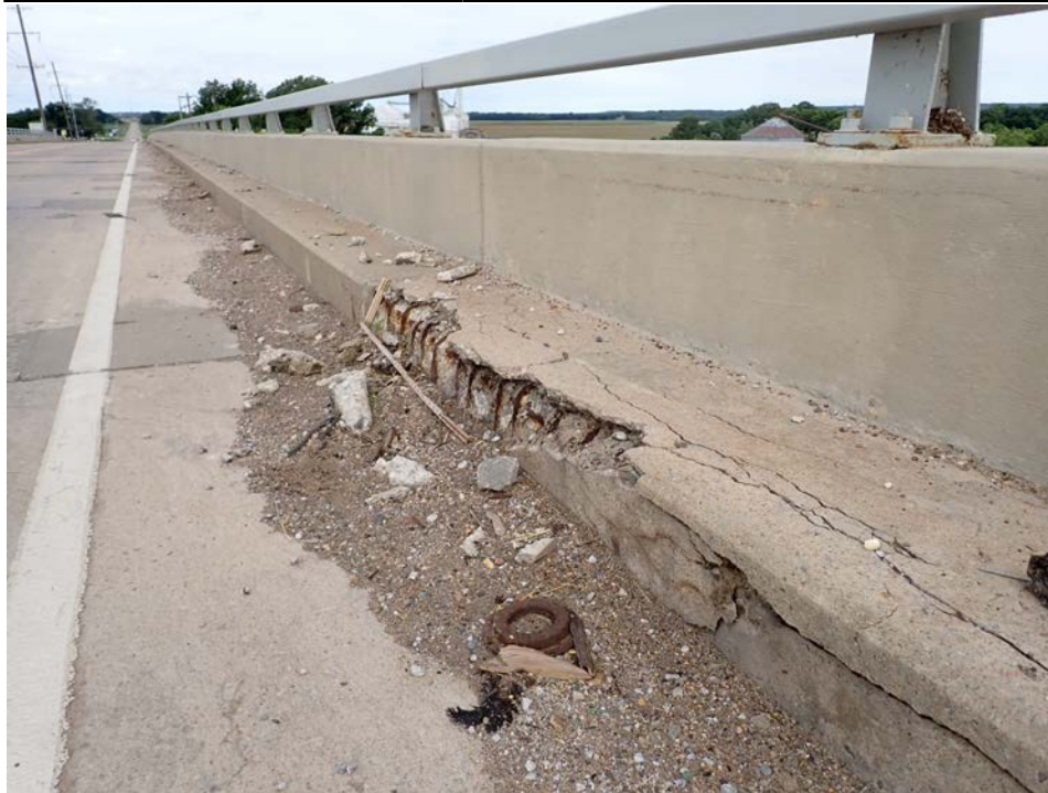
Photograph 7 - Looking northwest at the north concrete curb at mid span of span 3. Note: 7-foot-long by full curb height spall with exposed and corroded reinforcing steel.
