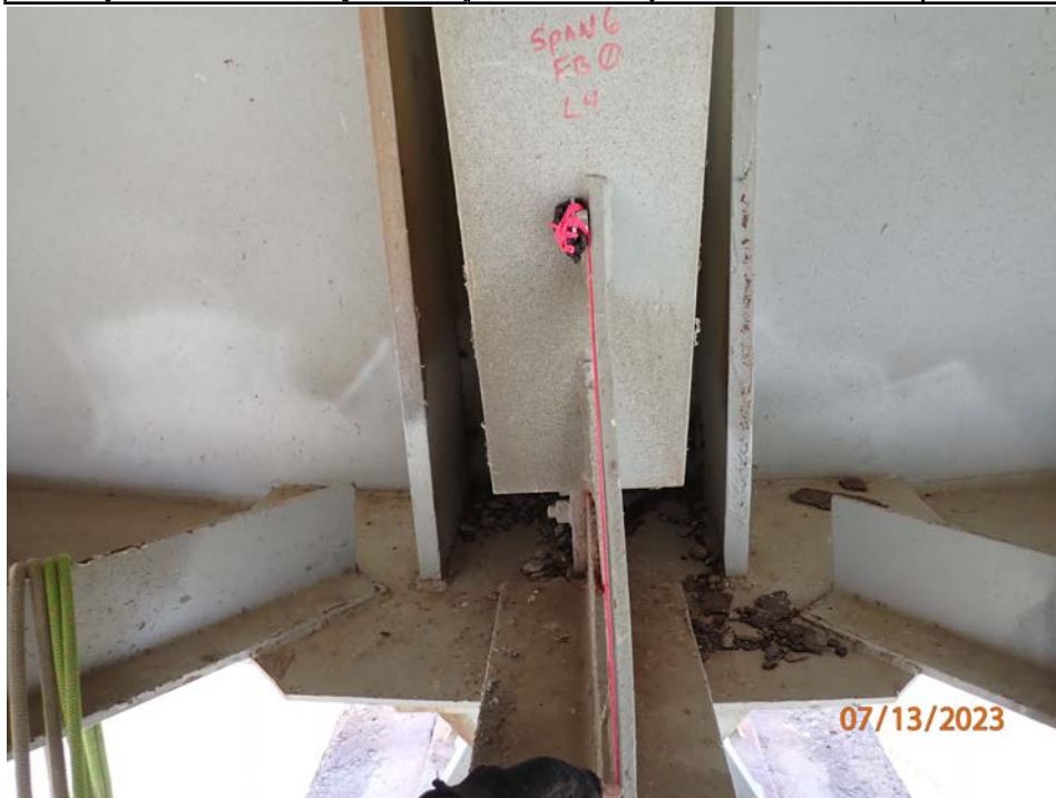
Photograph 42 - Looking north at floor beam 0 lower connection to girder 2 over pier 5. Note: gusset plate has been reinforced with a diagonal bar, which is now bowing out of plane 1/16 inch.
