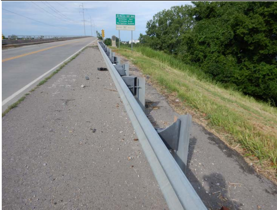
Photograph 5 - Looking west along the northeast approach railing. Note: the blockouts have been damaged for 60 feet near the transition.
