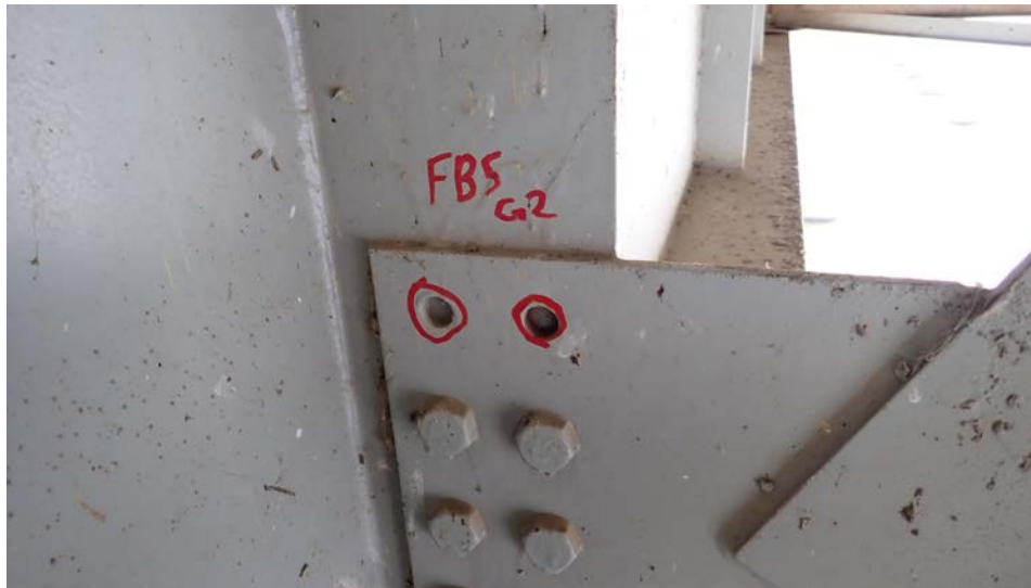
Photograph 45 - Looking east at floor beam 5, span 6 connection to girder 2. Note: 2 blind holes at the top of the connection.
