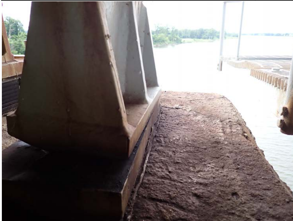
Photograph 70 - Looking south at the girder 1, span 10 expansion bearing at pier 10. Note: misalignment between the rocker and masonry plate with the rocker overhanging the masonry plate 1/4 inch.
