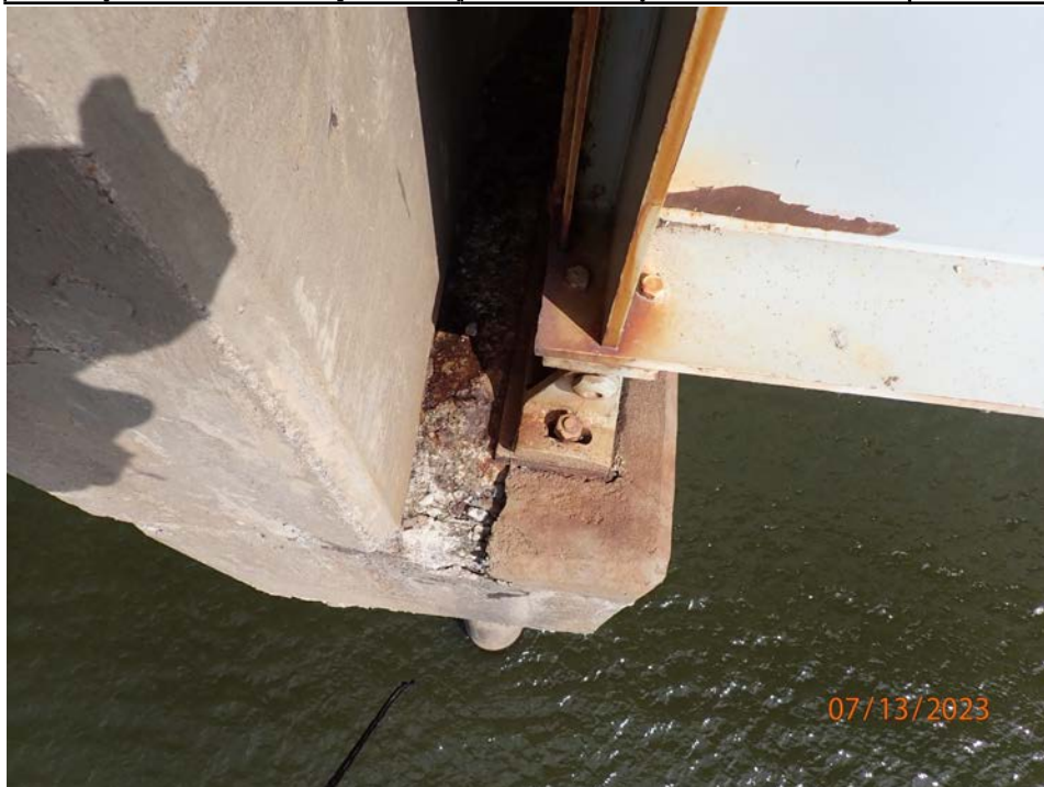
Photograph 62 - Looking north at pier 4 pier cap south end span 5. Note: scaling concrete around the girder 1 bearing.
