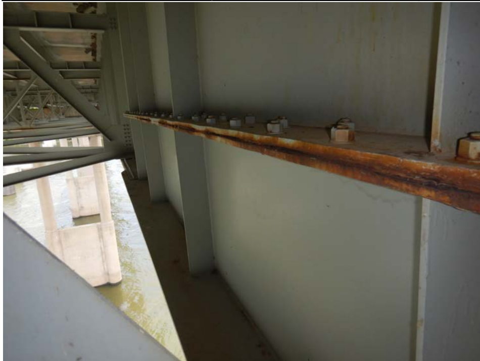
Photograph 30 - Looking south along the girder 1, span 7 horizontal splice. Note: 1/4-inch-thick pack rust exists between the splice plates.
