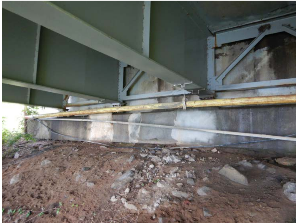
Photograph 57 - Looking northeast at the east abutment. Note: deck drainage leaking on bearing seat. Minor spall along bottom edge of breastwall between girders 2 and 3. 18 inches of penetration noted between girders 2 and 3 with no significant undermining noted vertically.
