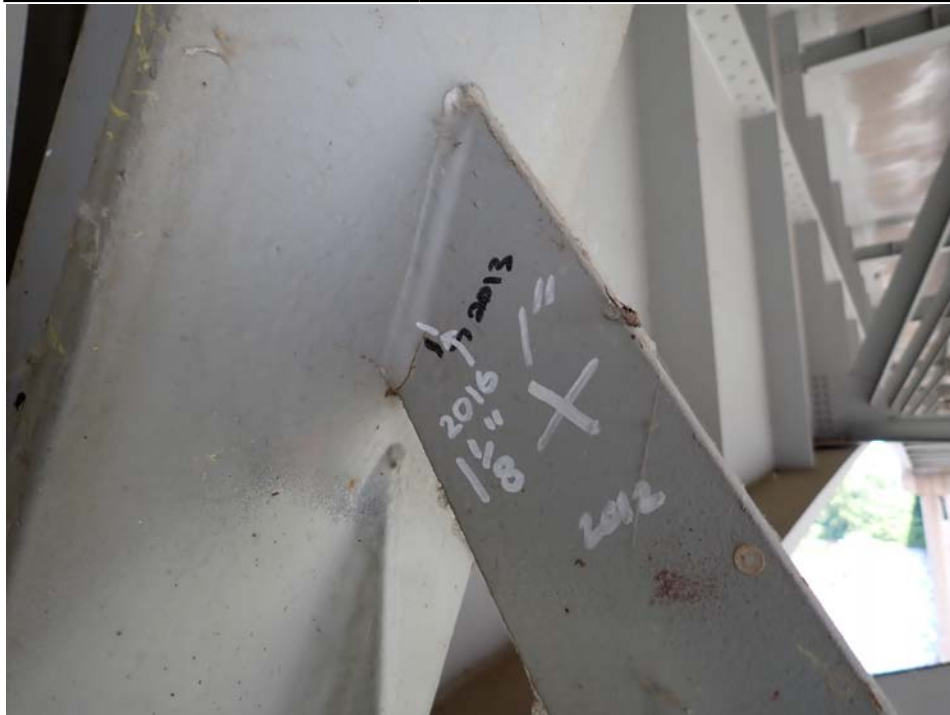
Photograph 48 - Looking northeast at the floor beam 0 lower strut connection to girder 2, span 7. Note: 1 1/8-inch-long crack in repair plate weld on the west face, 1/2-inch-long crack on the east face.
