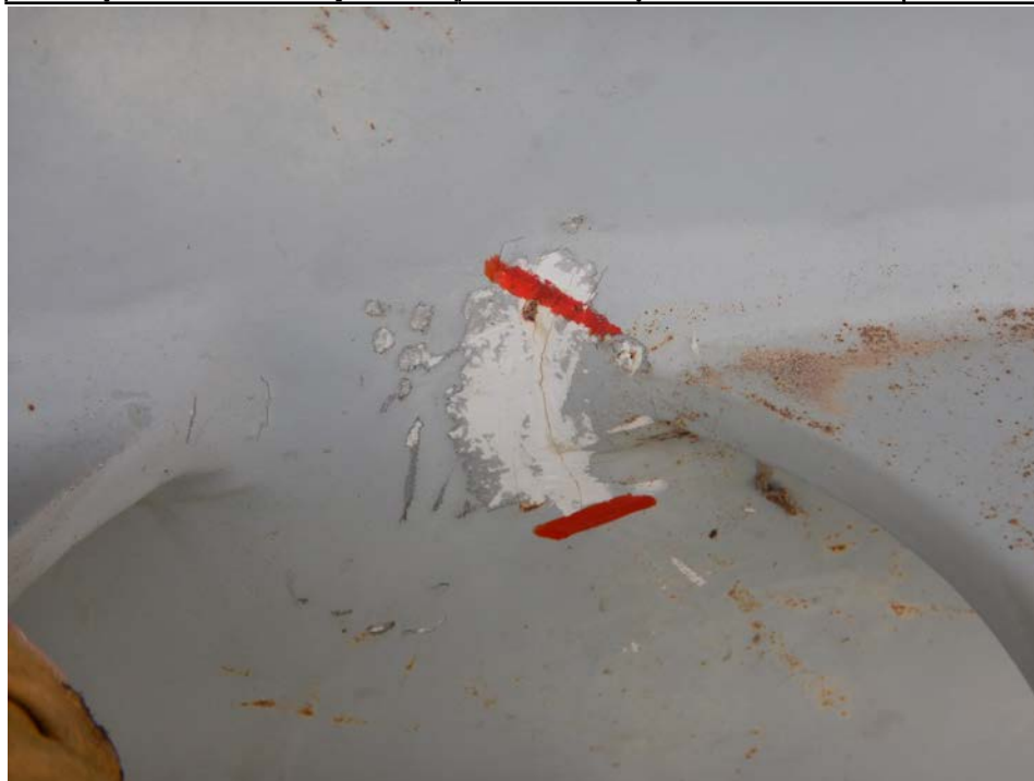
Photograph 28 - Looking north at girder 1, span 5 at the lower longitudinal stiffener splice between floor beams 4 and 5. Note: 1 1/4-inch long vertical paint crack in the girder web.
