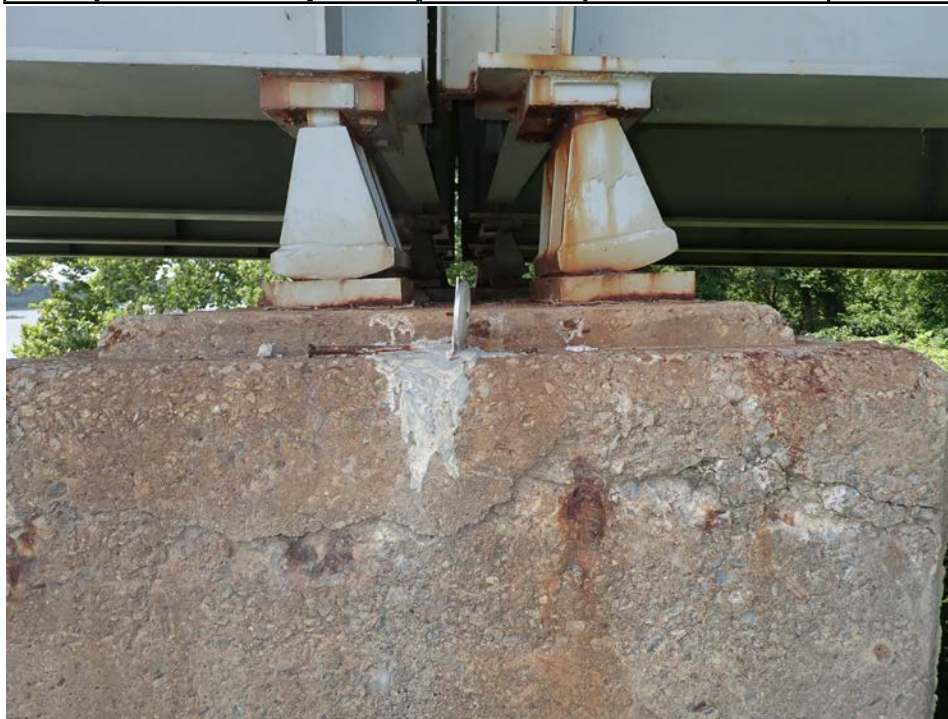
Photograph 65 - Looking north at the end of the pier 14 cap. Note: spalling and delaminations throughout the top of the cap.
