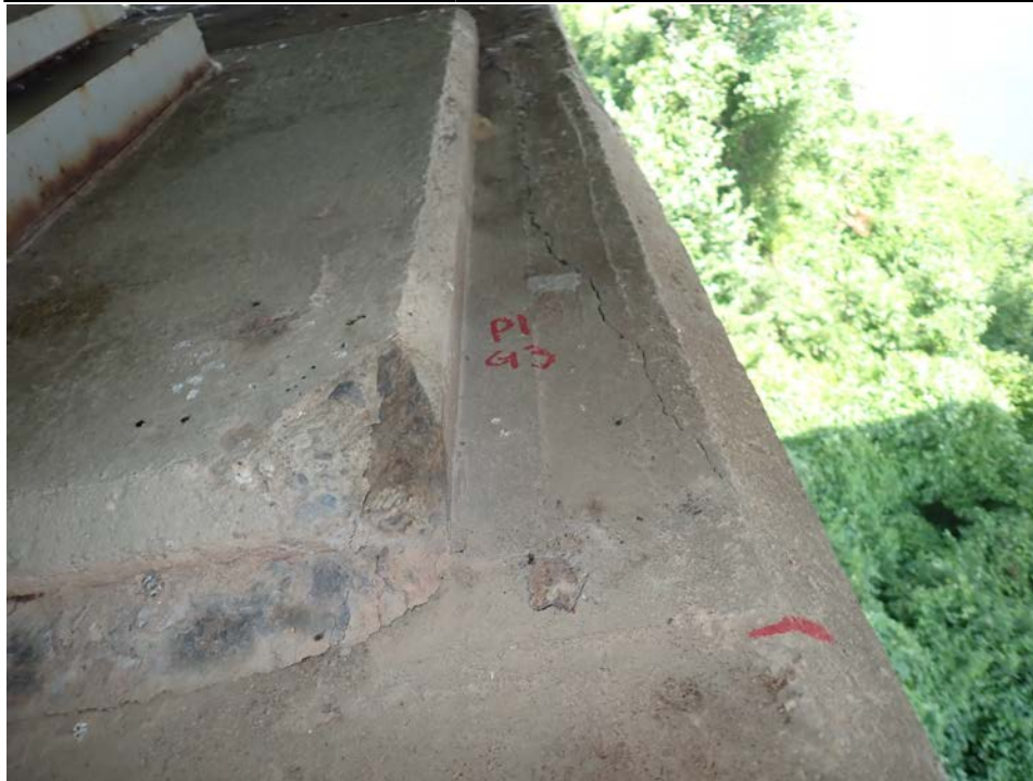
Photograph 61 - Looking north at pier 1 cap east edge near girder 3. Note: 5-foot-long corner spall/delamination.
