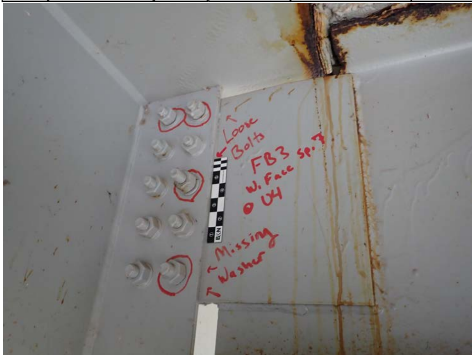
Photograph 46 - Looking east at floor beam 3, span 7 connection to girder 2. Note: 3 loose bolts and 1 missing washer.
