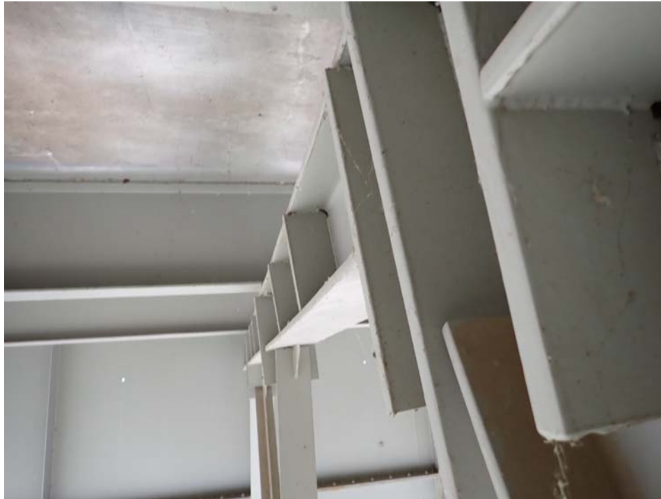
Photograph 49 - Looking south along the top chord of floor beam 1 in span 7 between the stringers. Note: top chord is rotated to the east, kink in upper gusset plate under stringer 3.
