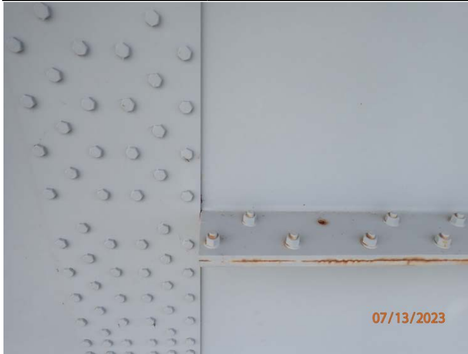
Photograph 27 - Looking north at the span 6, girder 2 field splice near floor beam 12. Note: 1 missing bolt in the horizontal splice.
