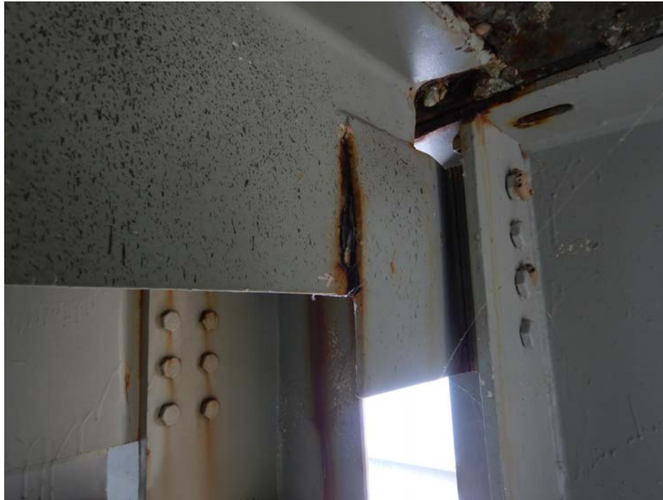
Photograph 31 - Looking southeast at the end diaphragm connection to girder 1, span 4 at pier 4. Note: pack rust has broken the bottom and vertical welds.
