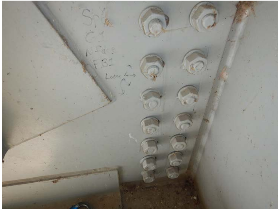
Photograph 43 - Looking east at floor beam 1, span 6 connection to girder 1. Note: loose bolts exist in the bottom strut connection to the girder. Several misdrilled holes exist in the connection.
