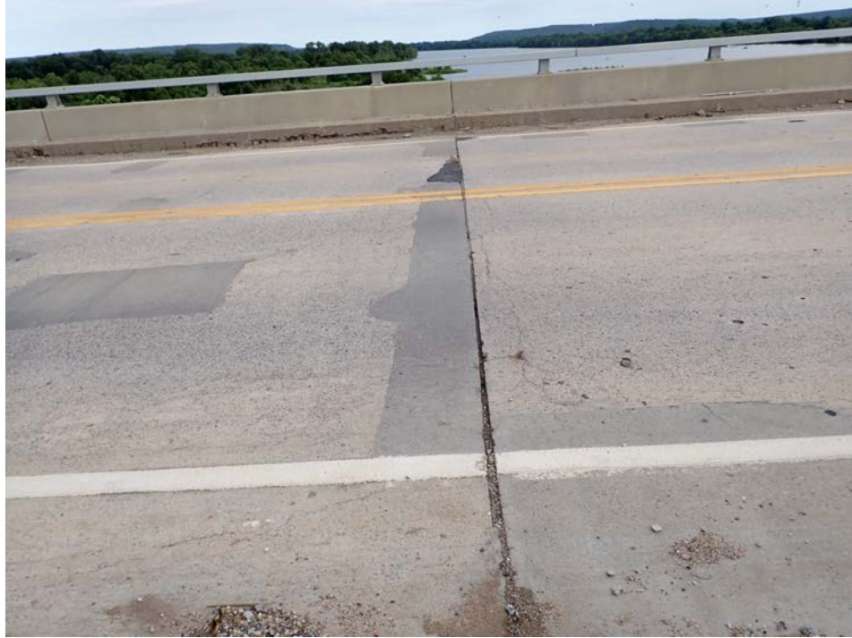
Photograph 19 - Looking north along the construction joint over floor beam 2 in span 3. Note: typical condition, isolated spalls/delaminations with concrete and AC patches.
