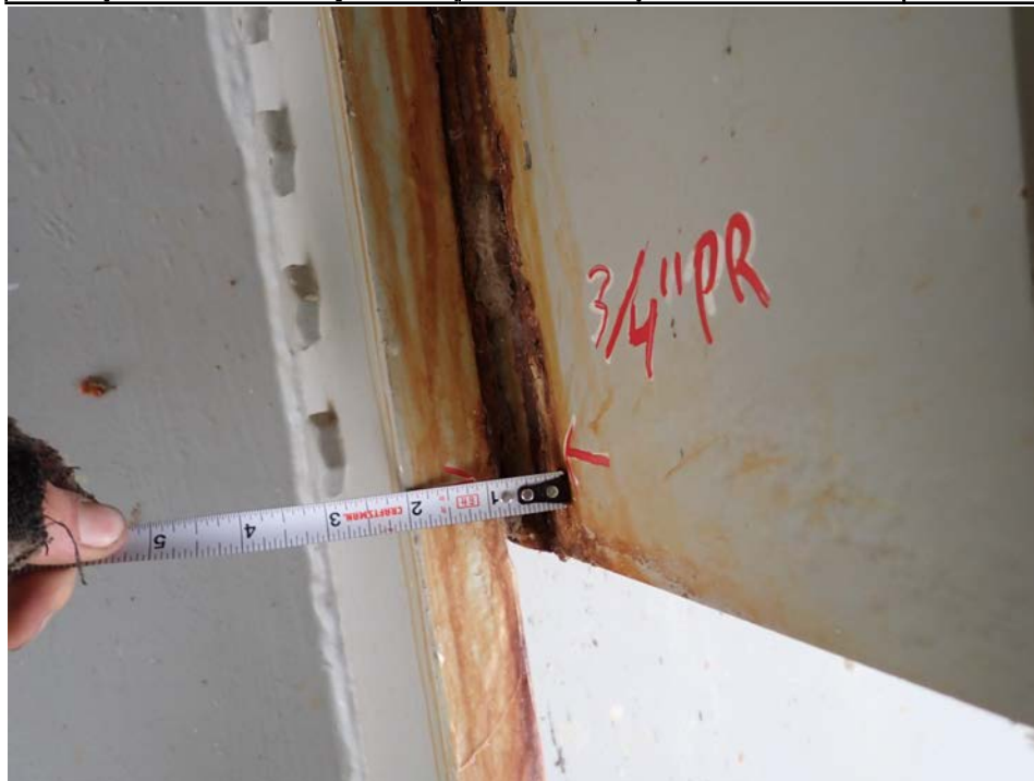
Photograph 34 - Looking southwest at the diaphragm connection to girder 1 over pier 9. Note: typical pack rust between bearing stiffener and diaphragm interface up to 3/4 inch thick.
