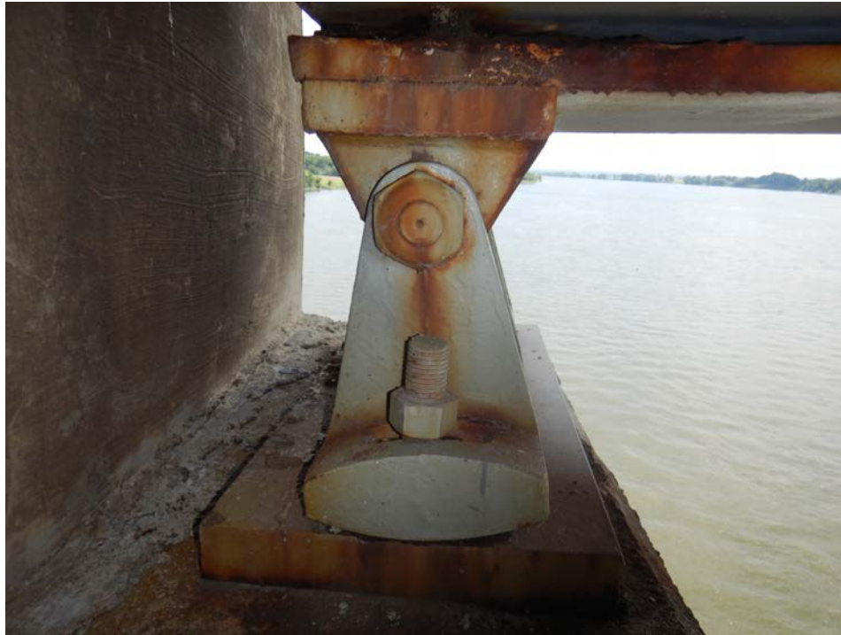
Photograph 71 - Looking south at the girder 1, span 7 expansion bearing at pier 7. Note: bearing in expansion 3 degrees at 96F.
