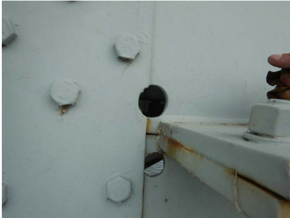
Photograph 25 - Looking south at girder 2, span 7 at the field splice near floor beam 4. Note: no cracks in outboard face of girder web
