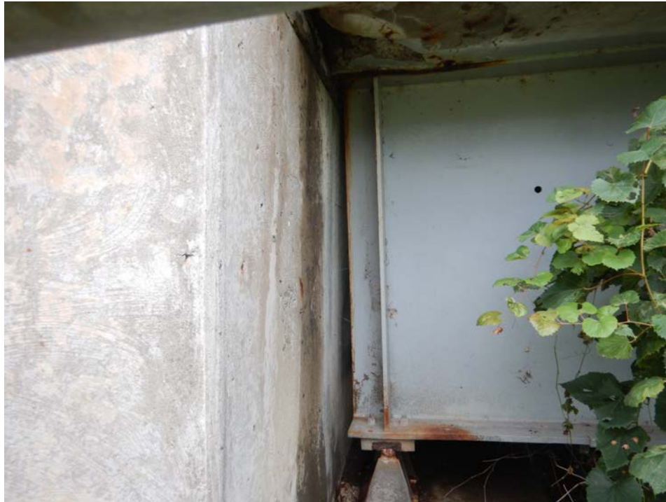
Photograph 59 - Looking south at girder 4, span 15 at the east abutment. Note: backwall is leaning towards the channel with 1 1/8 inches clear to the girder end near the top flange and 3 1/4 inches clear near the bottom flange.
