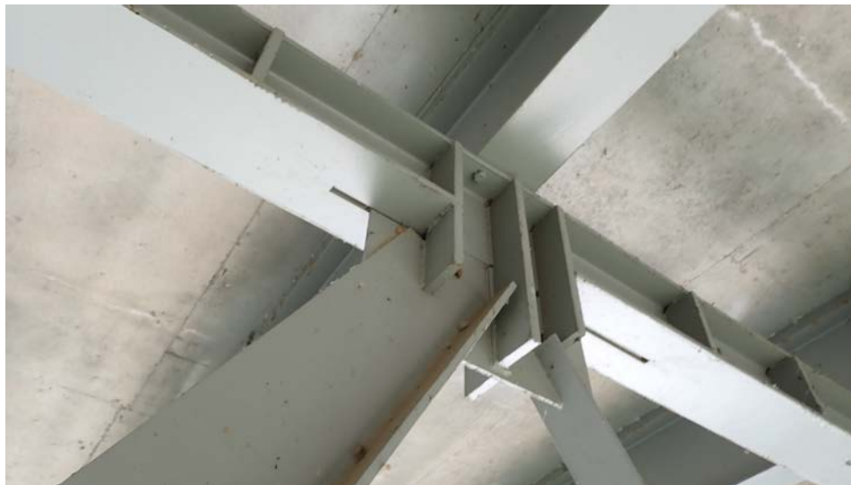
Photograph 36 - Looking southeast at the stringer 3 connection to floor beam 4, span 6. Note: loose bolt stringer connection bolt.
