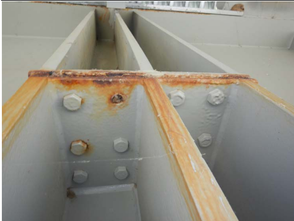
Photograph 26 - Looking up along the outboard face of the bearing stiffener for girder 1 at pier 6. Note: 1 missing bolt in horizontal splice. Corrosion and pitting exist at the splice interface.
