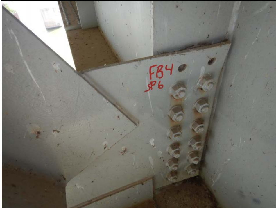
Photograph 44 - Looking east at floor beam 4 span 6, connection to girder 1. Note: 2 blind holes exist in top of the connection plate of the bottom strut. Pack rust is forming between the vertical stiffener and the connection plate.
