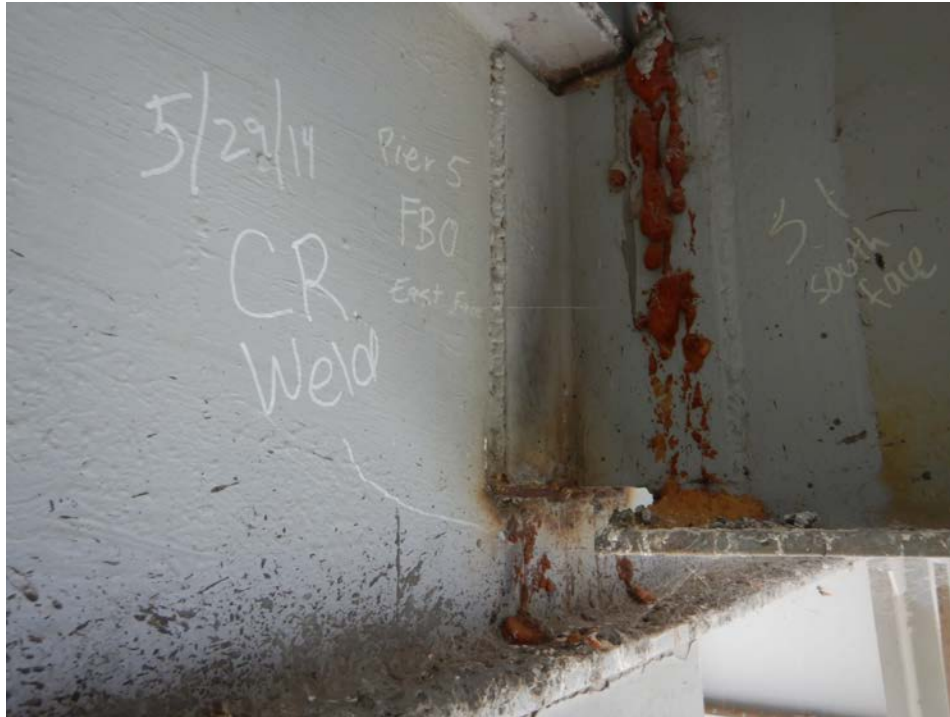
Photograph 47 - Looking northwest at stringer 1 connection to the east face of floor beam 0, span 6. Note: stringer connection angle has been rewelded along the bottom edge.
