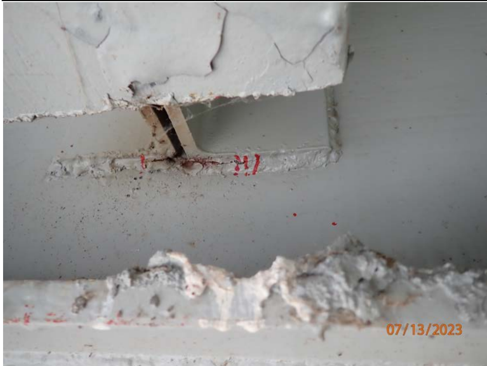
Photograph 38 - Looking west at the stringer 3 connection to floor beam 3, span 5. Note: 3 1/2-inch-long crack along weld on the underside of the stringer connection angles.
