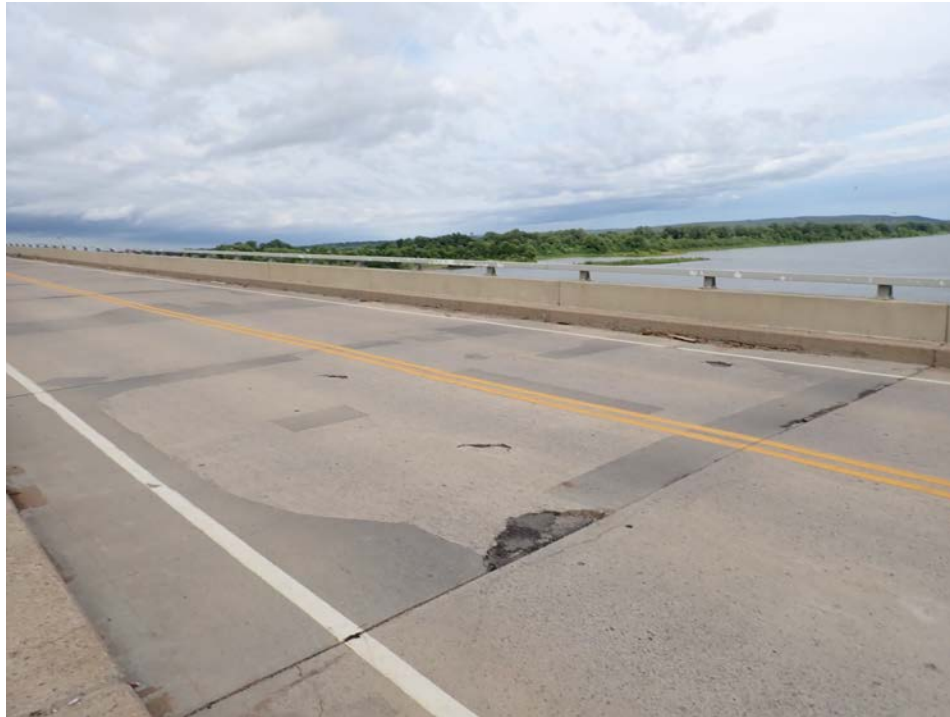
Photograph 13 - Looking northwest at the deck near mid span of span 14. Note: concrete patches throughout with isolated asphalt patches and spalling.
