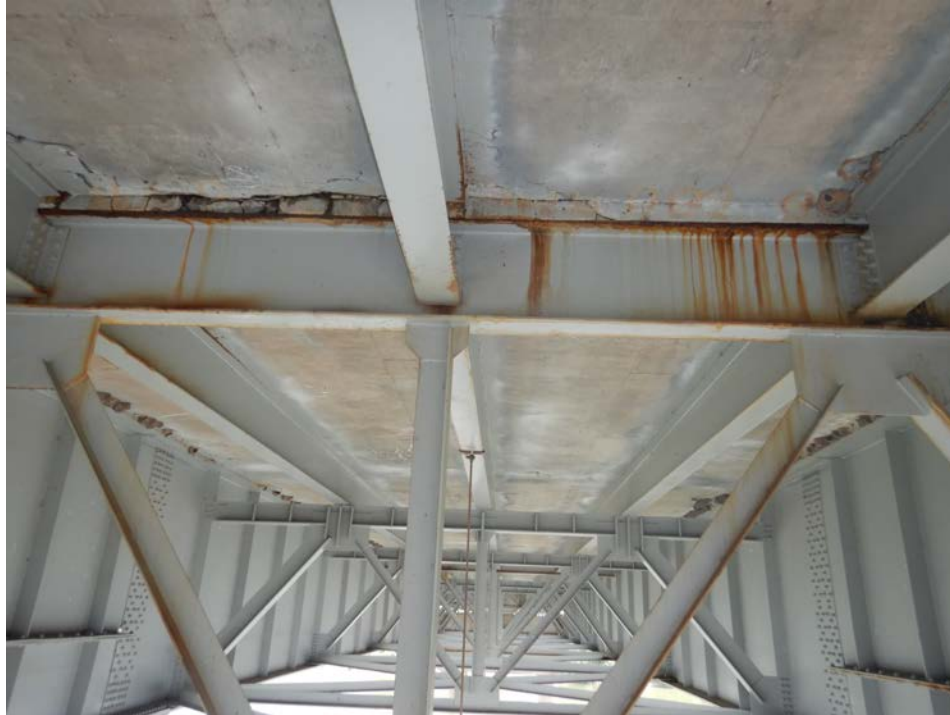
Photograph 15 - Looking east at floor beam 3, span 7. Note: pack rust and section loss exists along the top flange of the floor beam. Spalls are typical in the deck soffit adjacent to the floor beam.
