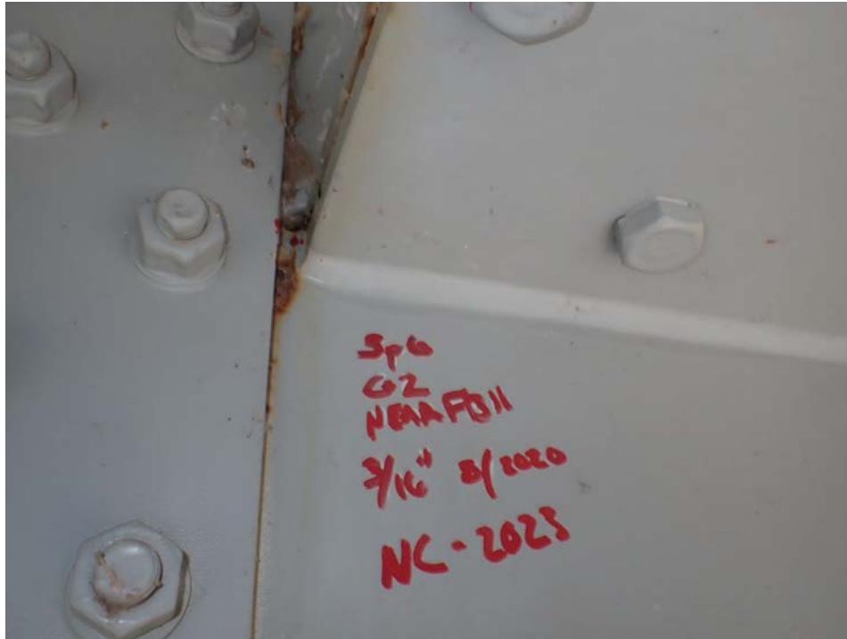
Photograph 23 - Looking north at girder 2, span 6 at the field splice near floor beam 11. Note: 3/16-inch-long crack in the inboard face at the horizontal web splice termination.
