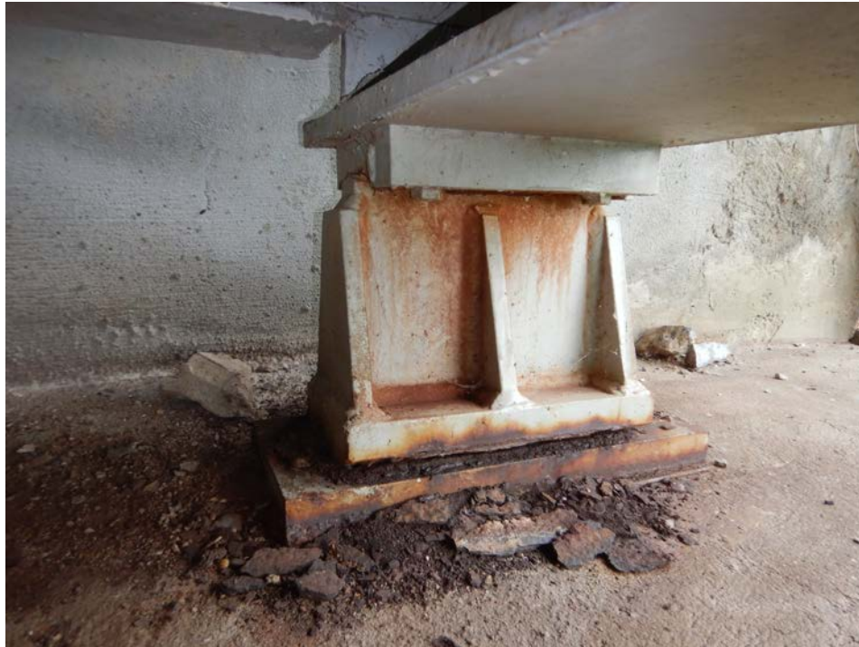
Photograph 69 - Looking west at the girder 4, span 1 expansion bearing at the west abutment. Note: south keeper plate attached to the sole plate is missing and the bearing has moved south 1/2 inch with no significant lateral movement since the last painting.
