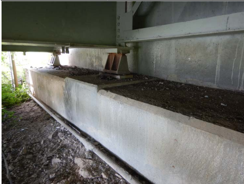
Photograph 60 - Looking southwest at the west abutment. Note: light accumulation of spalled concrete and debris on bearing seat.
