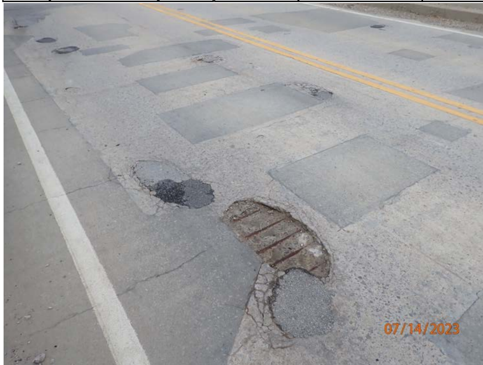
Photograph 10 - Looking northwest at span 7 deck top eastbound lane. Note: 2-foot-long by 1-foot-wide by up to 3-inch deep pothole with 5 exposed and corroded transverse reinforcement.
