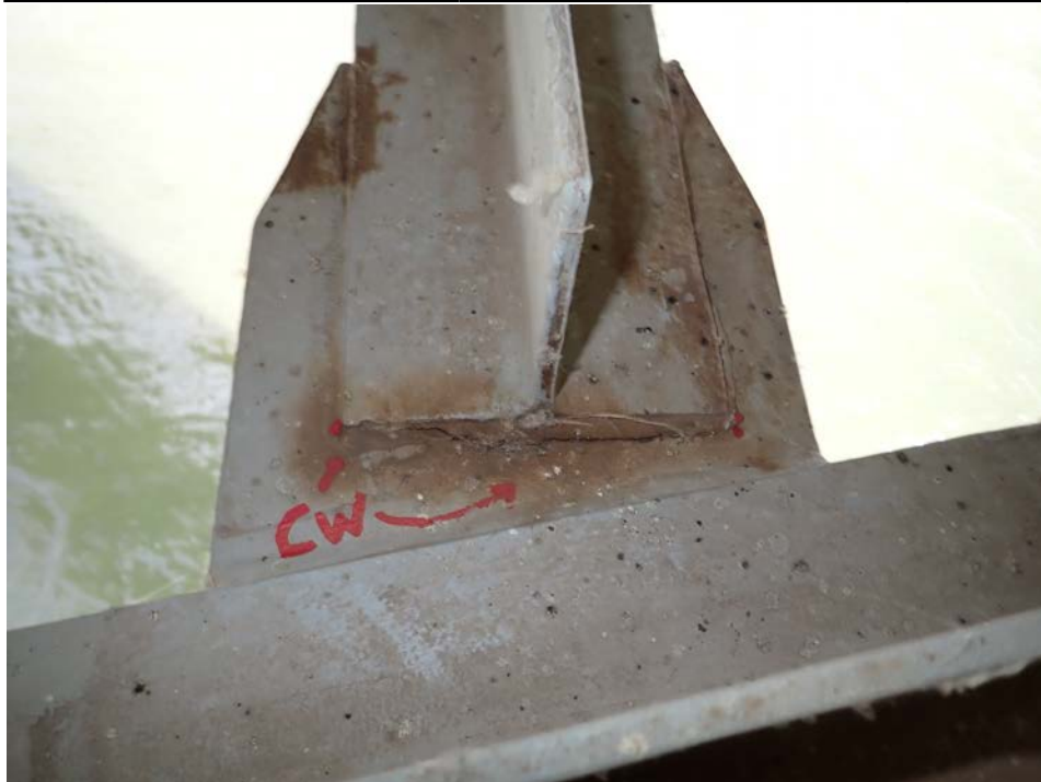
Photograph 56 - Looking southeast at span 7, lower lateral bracing crossbuck connection between floor beams 3 and 4. Note: cracked weld on southeast member due to pack rust.
