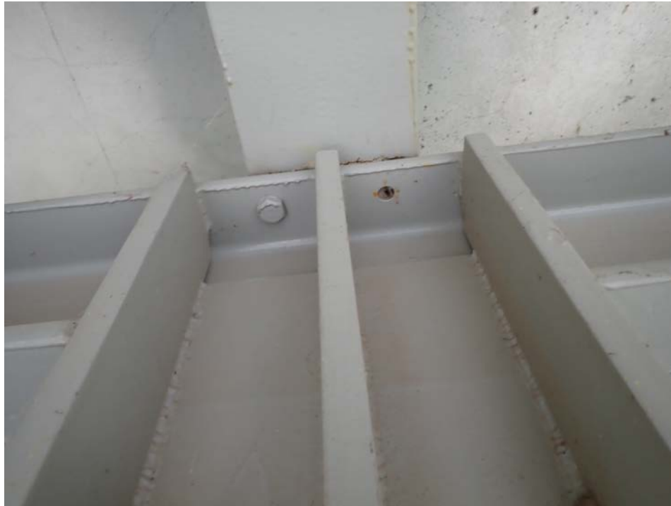
Photograph 37 - Looking east at the stringer 3 connection to floor beam 4, span 7. Note: one missing stringer connection bolt.
