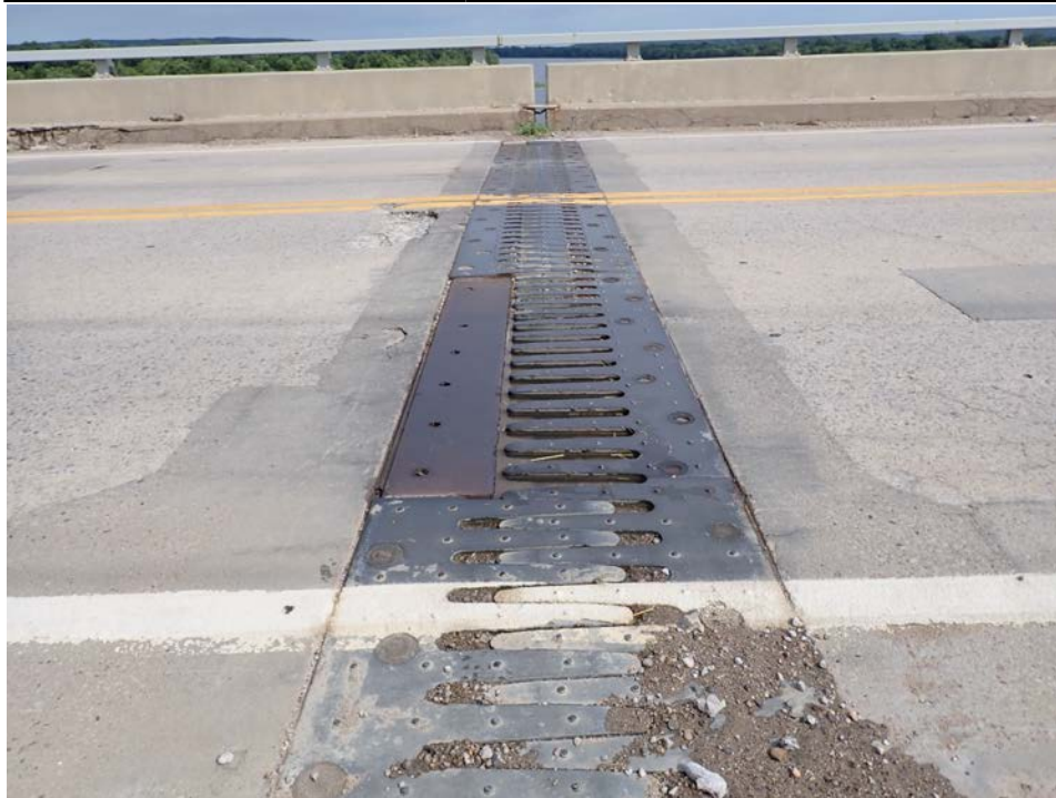
Photograph 17 - Looking north along the finger joint over pier 4. Note: 5 feet of missing fingers on span 4 side in east travel lane, 4 feet missing in span 4 side near the north shoulder. Heavy debris compaction for the full length inhibits expansion of joint.
