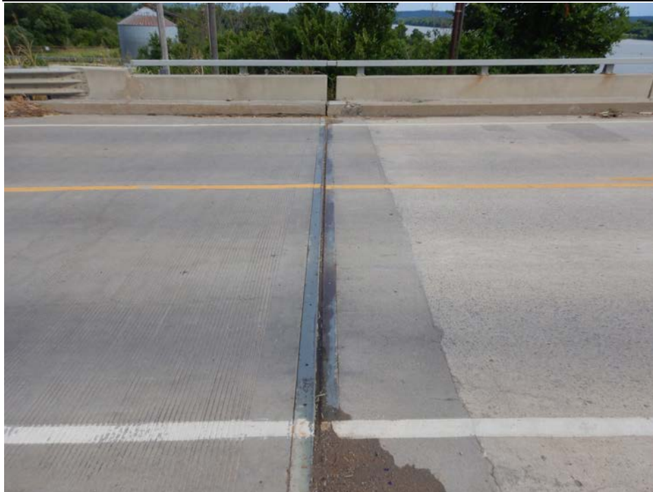
Photograph 16 - Looking north along the sealed expansion joint at the west abutment. Note: moderate debris impactation throughout.
