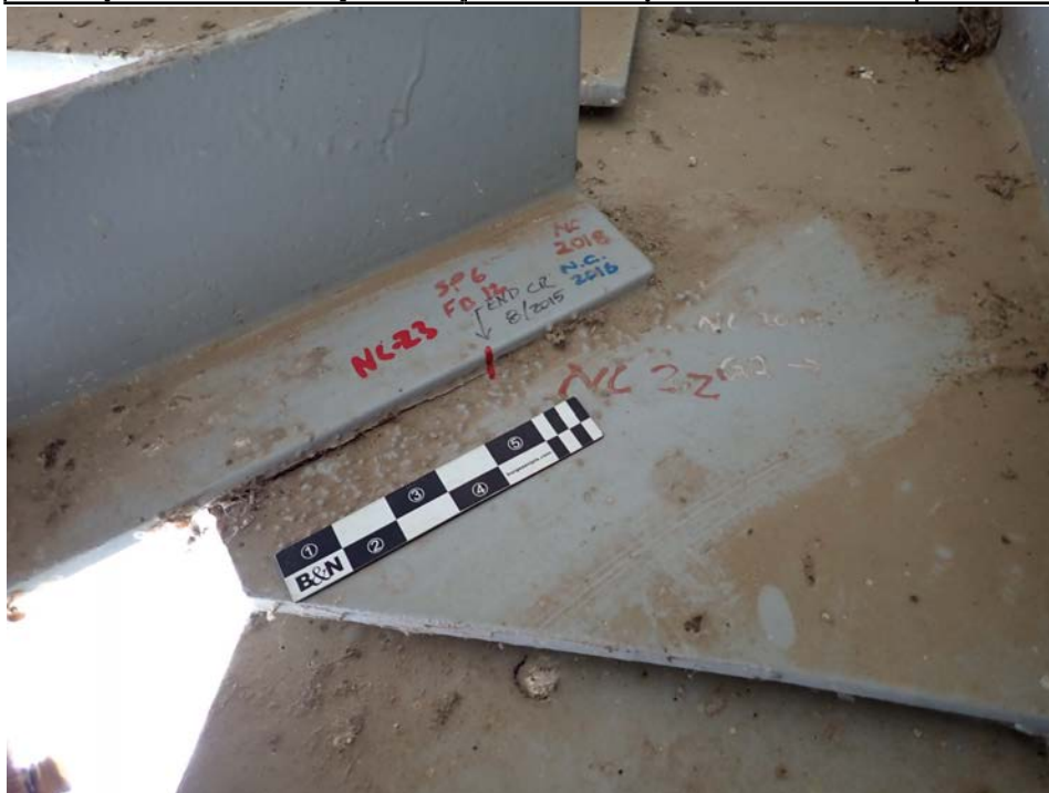
Photograph 52 - Looking west at the lower lateral bracing connection to floor beam 12 and girder 2, span 6. Note: 5 3/4-inch-long crack in weld between lower lateral bracing and gusset plate.
