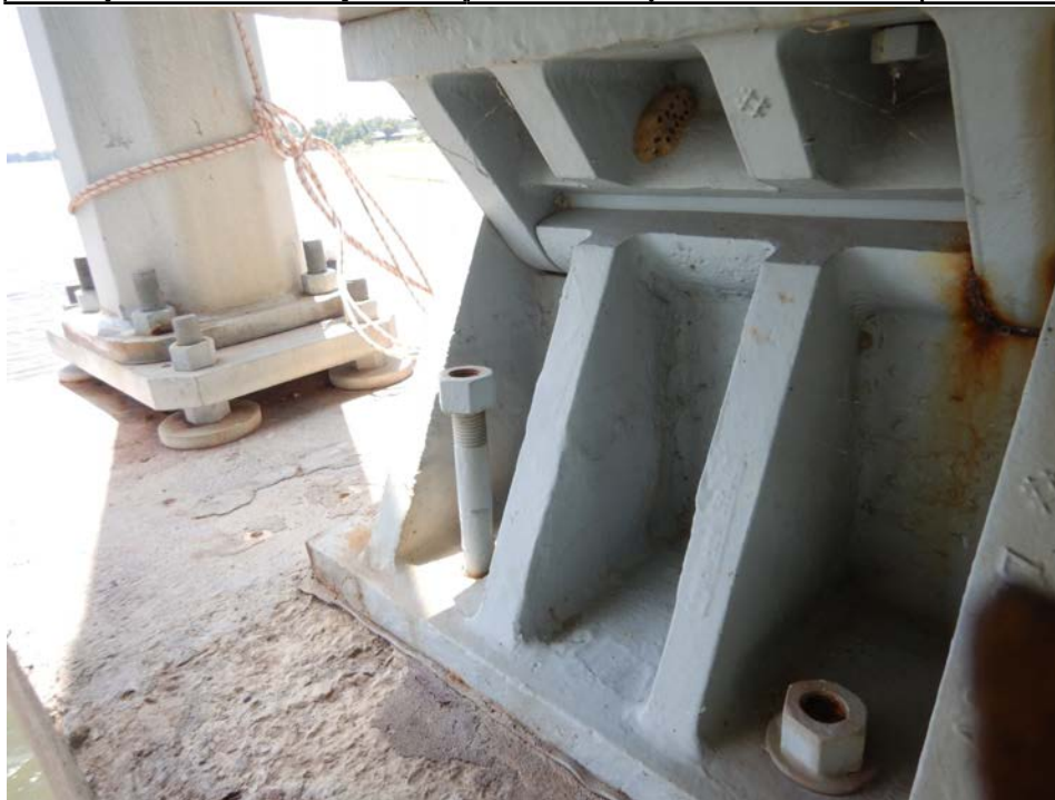
Photograph 67 - Looking southwest at the girder 1, pier 5 fixed bearing. Note: anchor bolt lifted and nuts not fully seated.
