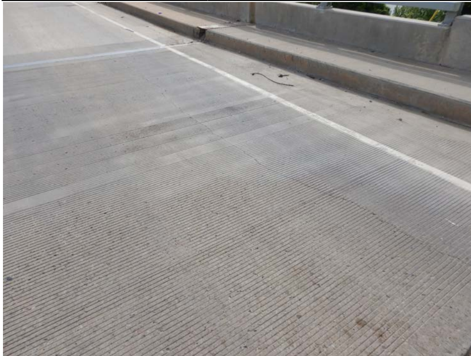
Photograph 73 - Looking southeast at the west approach slab in the eastbound lane. Note: longitudinal crack running the full length of the slab with intersecting transverse cracks.
