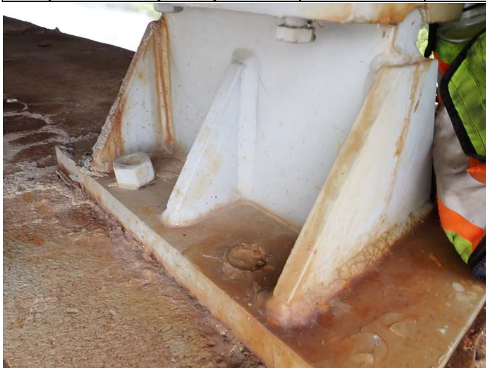
Photograph 68 - Looking northeast at girder 2 fixed bearing at pier 8. Note: missing anchor bolt.
