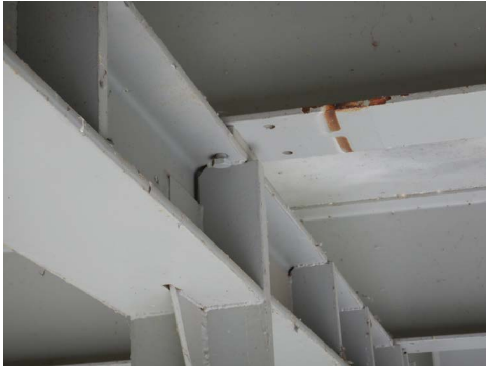
Photograph 35 - Looking north at the stringer 2 connection to floor beam 4, span 5. Note: bolt on east face is loose and bolt holes punched in wrong location.
