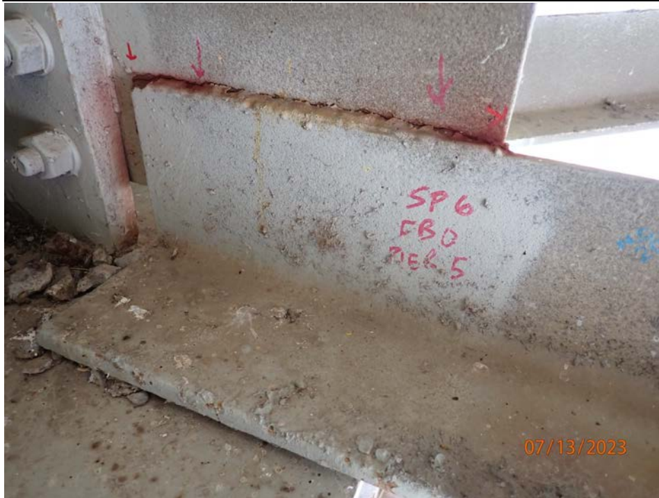
Photograph 41 - Looking east at floor beam 0 lower connection to girder 2 over pier 5. Note: full width crack along the floor beam to gusset plate weld on both faces.
