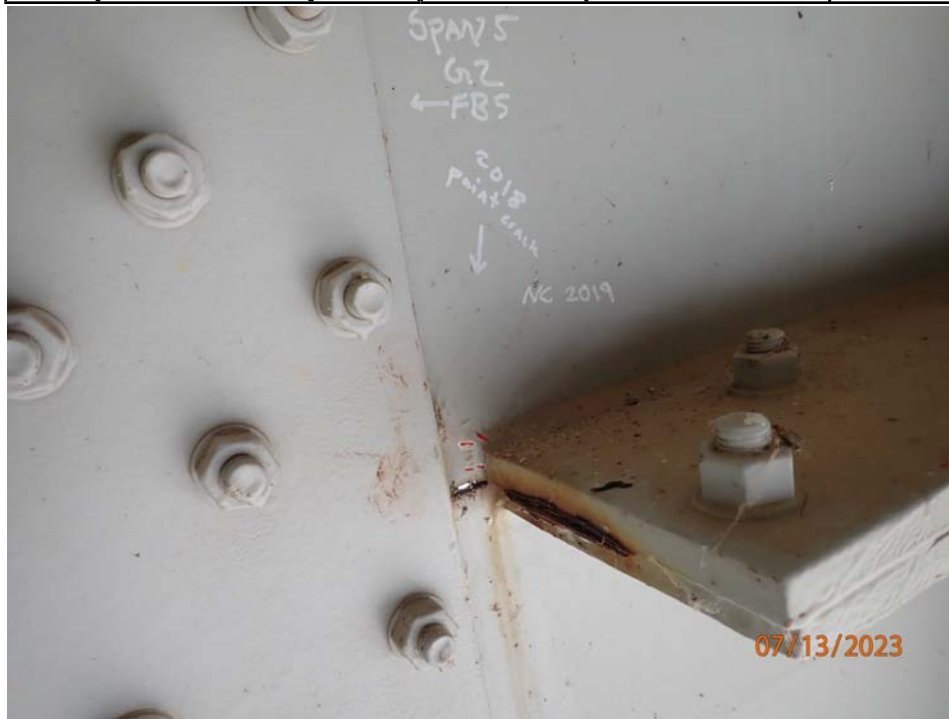
Photograph 21 - Looking northeast at girder 2, span 5 at the field splice near floor beam 5. Note: 3/8-inch-long paint crack in the inboard face at the horizontal web splice termination.
