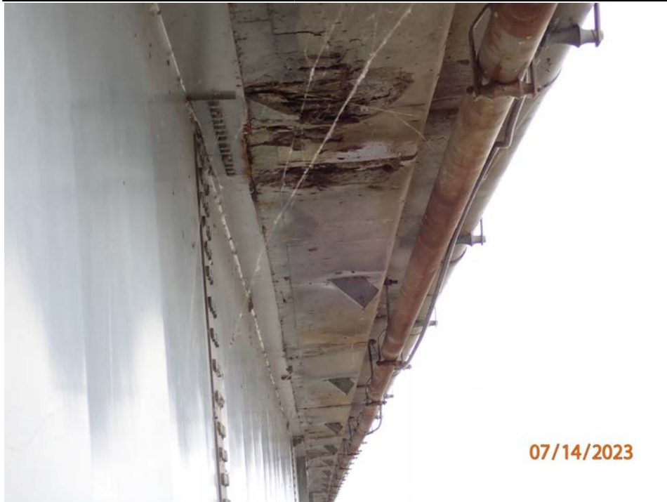
Photograph 14 - Looking west at span 12 north soffit overhang near pier 12. Note: typical spalling with exposed and corroded reinforcement.
