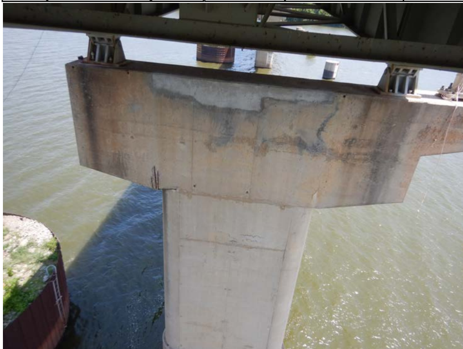
Photograph 64 - Looking east at pier 5. Note: patched area and spall with exposed reinforcing steel in cap due to deck drainage passing through previous deck control joint.
