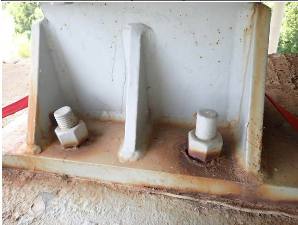
Photograph 66 - Looking west at girder 1, pier 3 bearing. Note: fixed bearing anchor bolts are bent.
