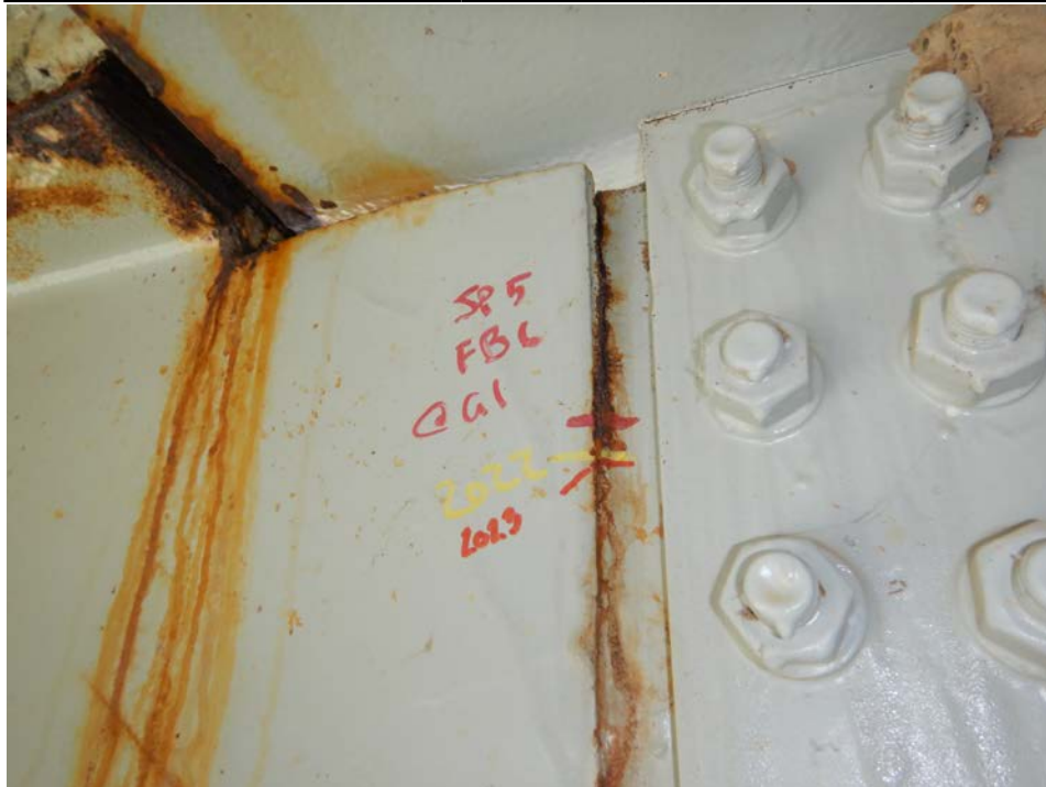
Photograph 40 - Looking east at floor beam 6 connection to girder 1, span 5. Note: 5 1/8-inch vertical crack in connection weld.
