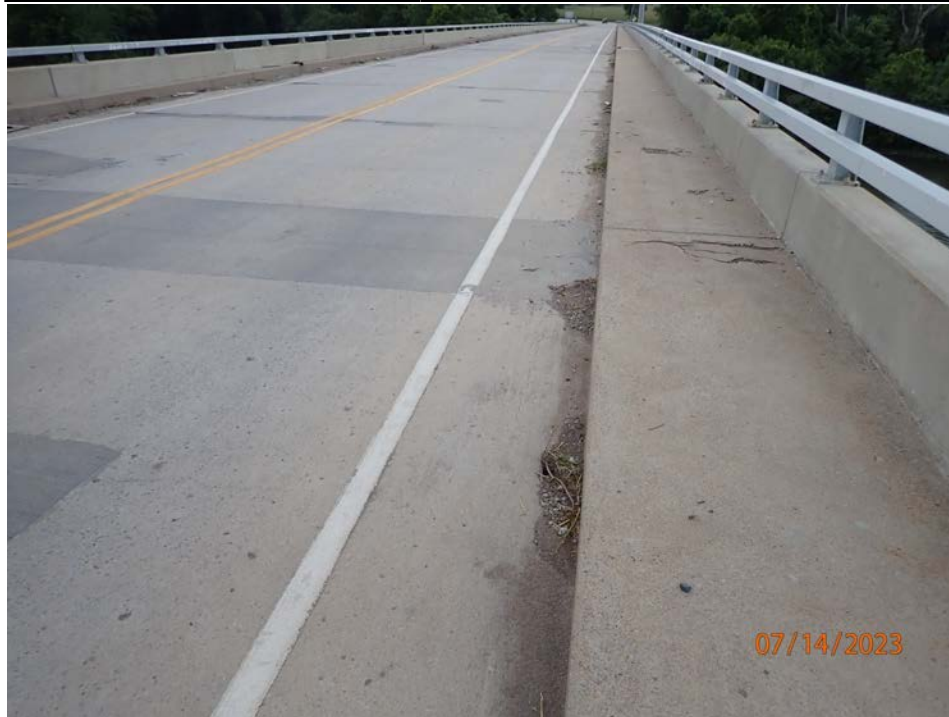
Photograph 9 - Looking east along the south curb in span 10. Note: isolated scuppers clogged with debris. Moderate debris exists along edge of deck full length.
