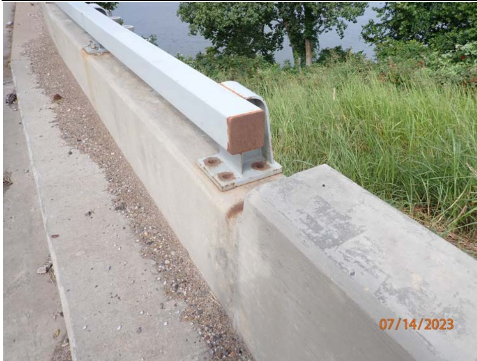
Photograph 3 - Looking northwest at the north rail east end post. Note: rail post is missing all four anchor bolts.
