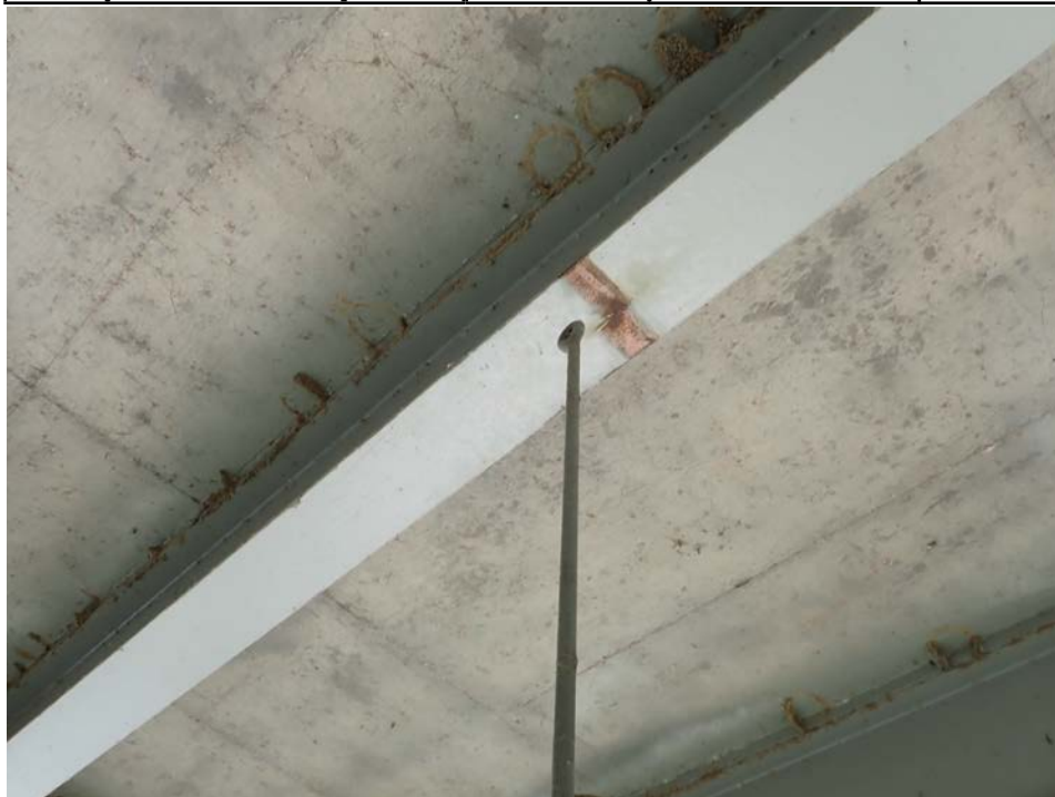
Photograph 54 - Looking southeast at the lower lateral bracing hanger rod in span 6, between floor beams 5 and 6. Note: missing clamp to stringer bottom flange.
