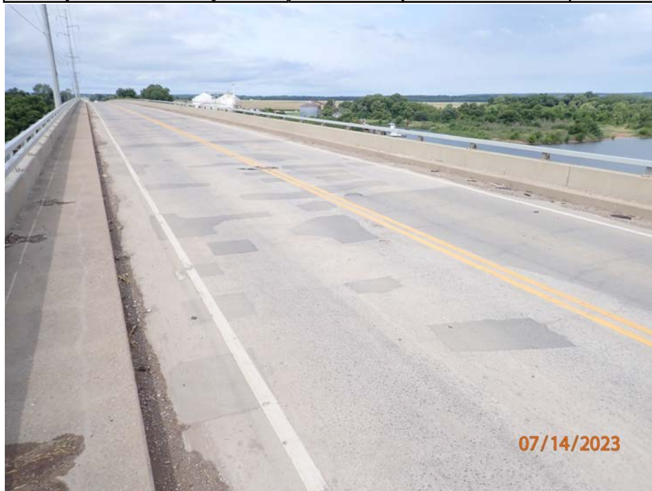
Photograph 12 - Looking northwest at span 7 deck top. Note: typical patching in good condition throughout the bridge.
