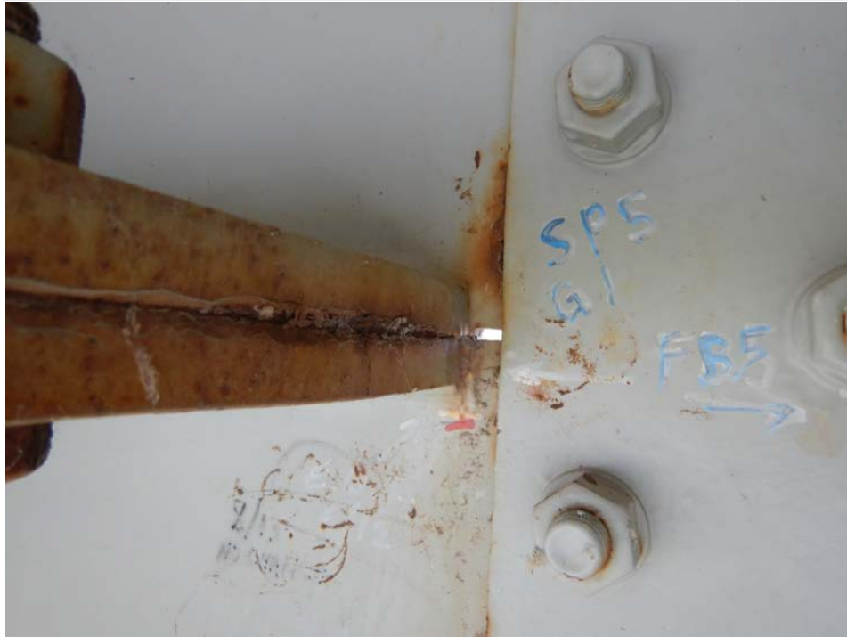
Photograph 20 - Looking southeast at girder 1, span 5 at the field splice near floor beam 5. Note: 5/8-inch-long crack in the inboard face at the horizontal web splice termination.
