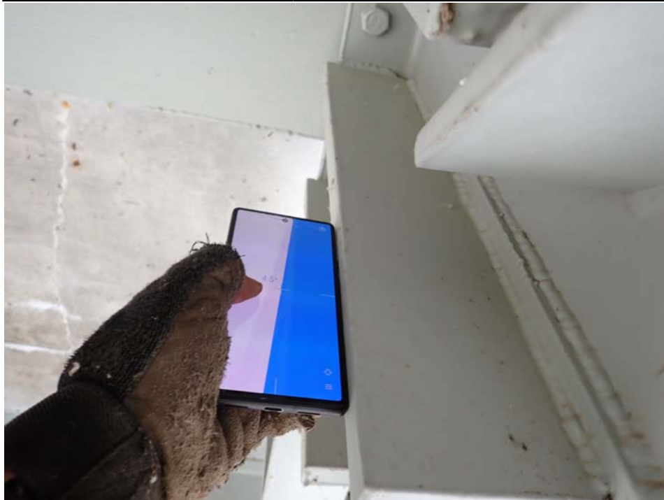
Photograph 50 - Looking northwest at floor beam 5, span 7 under stringer 3. Note: top chord/strut is rotated 4.5 degrees east.
