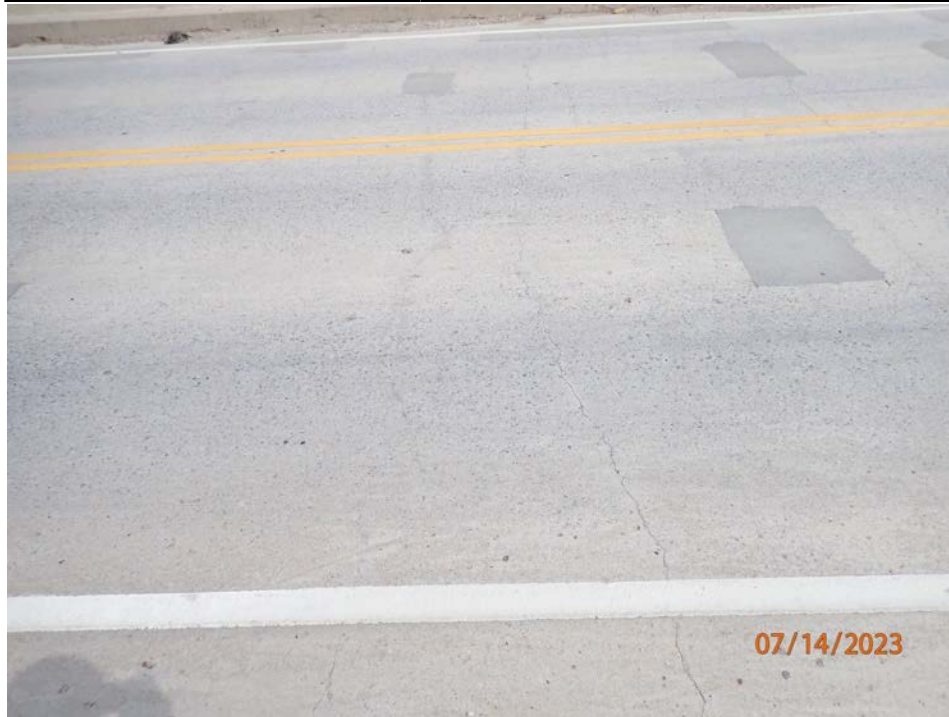
Photograph 11 - Looking north at span 5 top of deck. Note: transverse cracking spaced 1 to 3 feet apart.
