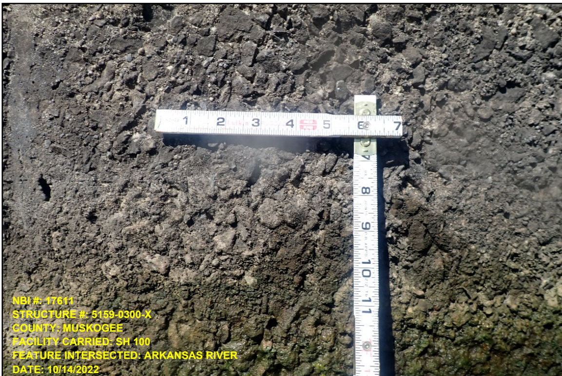
Photo 12 – Typical Concrete Condition Above the Waterline (Abrasion)
