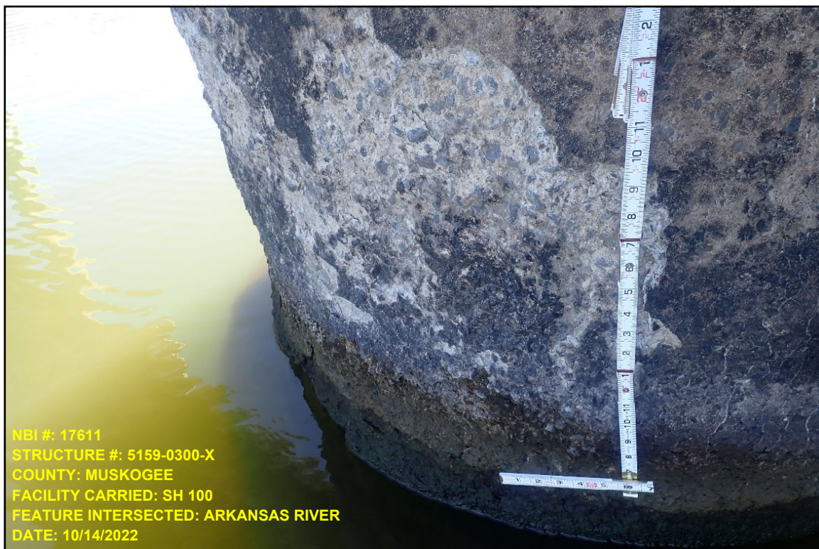
Photo 20 – Pier 7, Column 2, Spall 48-in W x 2 1/2-in D
