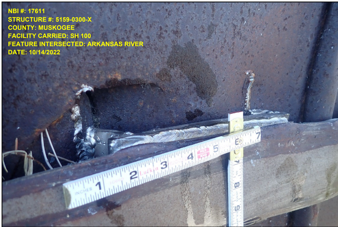
Photo 19 – Pier 6 Dolphin, Impact Damage
