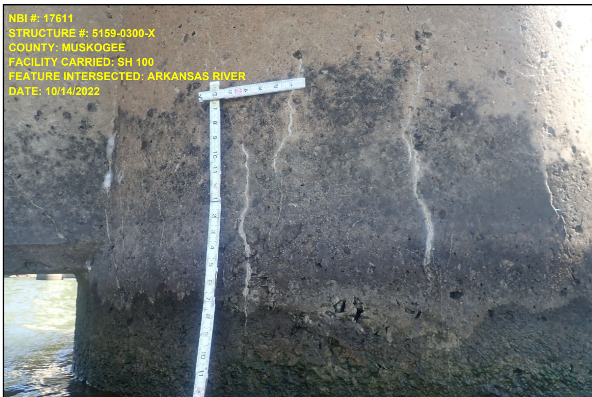
Photo 22 – Pier 11, Both Columns, Typical Cracks up to 1/16-in Wide with Efflorescence
