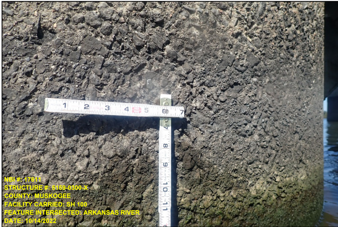
Photo 11 – Typical Concrete Condition Above the Waterline (Abrasion)
