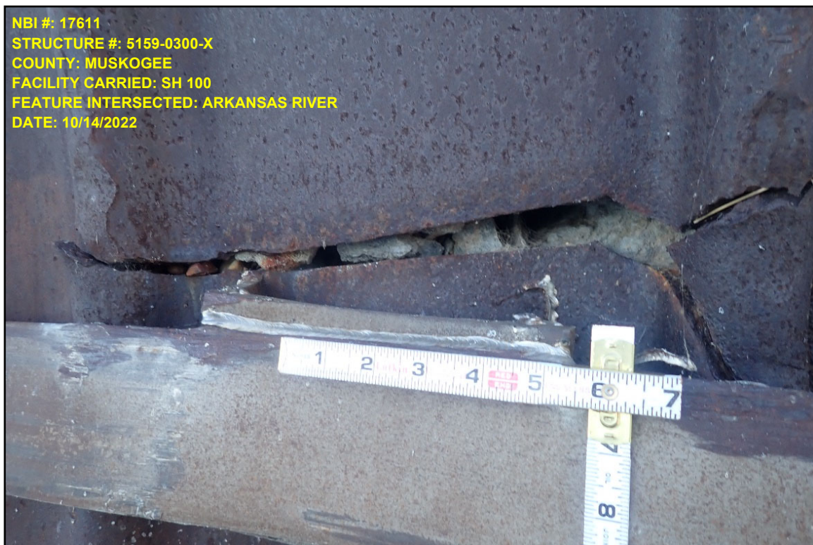
Photo 18 – Pier 6 Dolphin, Impact Damage
