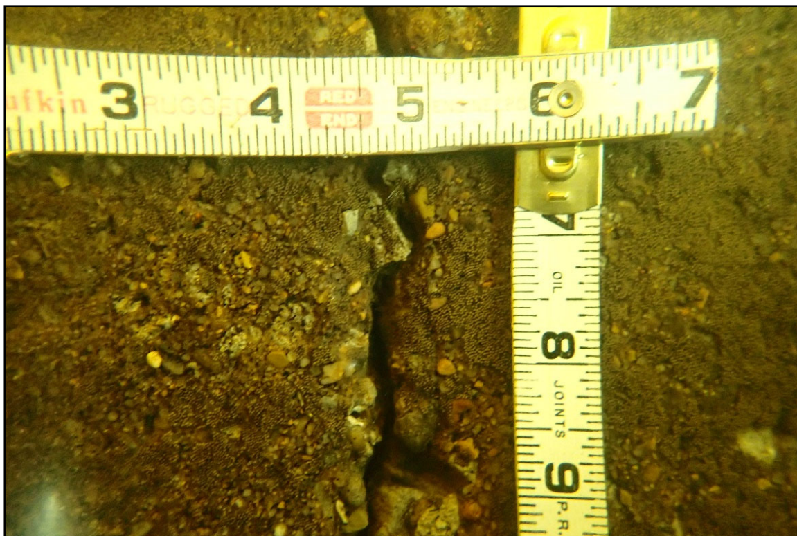
Photo 23 – Pier 12, Column 1, Vertical Crack up to 3/16-in Wide Below the Waterline
