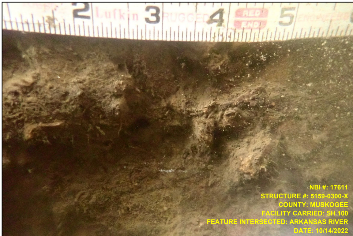
Photo 16 – Pier 6, Footing/Column Interface, Voiding 3-in H x 1/2-D
