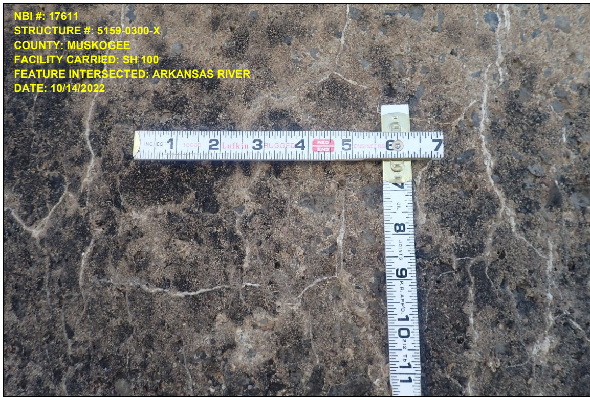
Photo 21 – Pier 7, Column 2, Map Cracking with Efflorescence
