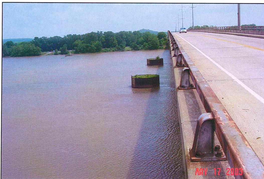
Figure A7: Upstream side of the SH-100 Bridge and existing dolphins, facing east bank.
