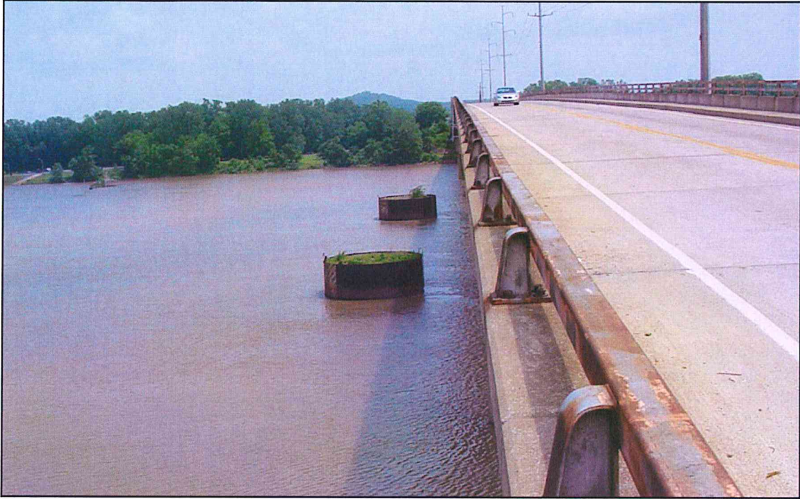
Figure 2.4-1: Sheet Pile Dolphins at Piers 5 and 6
