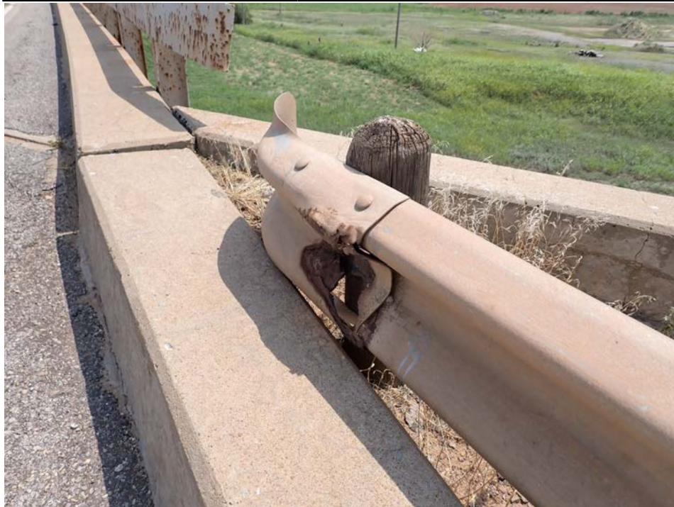
Photograph 8 - Looking north at the south east approach rail. Note: end is corroded and incorrectly lapped.
