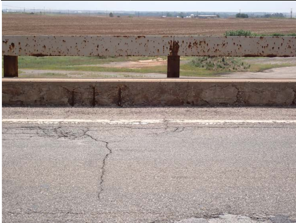
Photograph 12 - Looking east at the east curb in span 5. Note: spalls with exposed reinforcing steel due to shallow cover.
