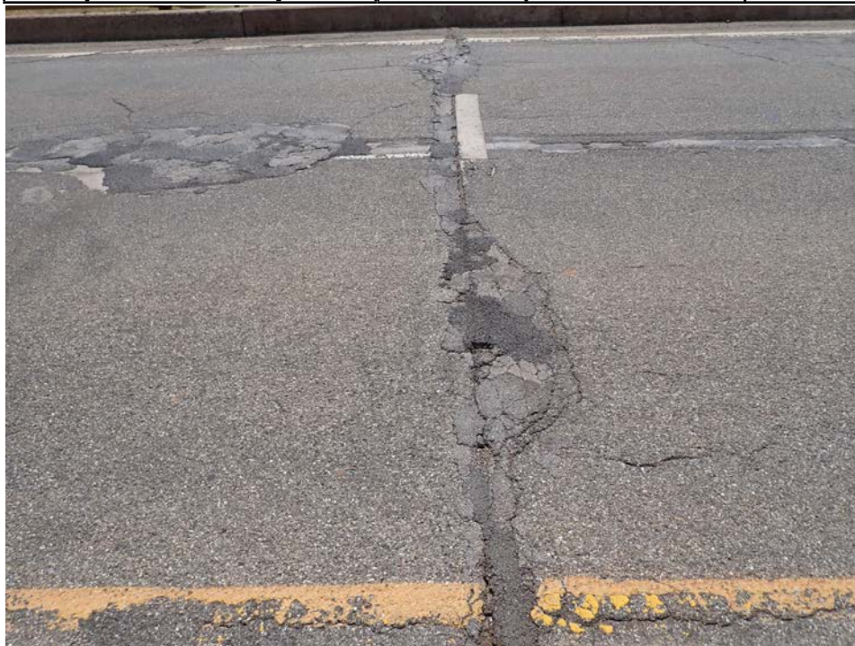
Photograph 10 - Looking east along the fixed joint at pier 5. Note: asphalt and concrete patches in the driving surface and along the joint.
