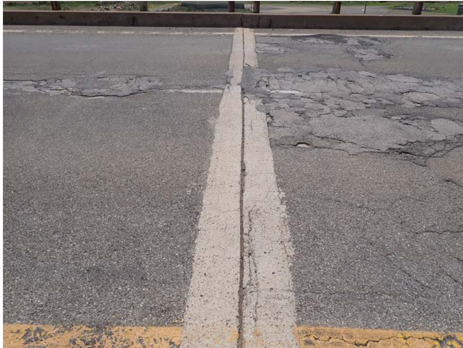
Photograph 20 - Looking east at the fixed joint over pier 1. Note: joint header has been replaced with concrete with multiple asphalt patches at the roadway centerline. Poured seal exhibits adhesive failure in isolated areas throughout with evidence of leakage on the pier cap below.
