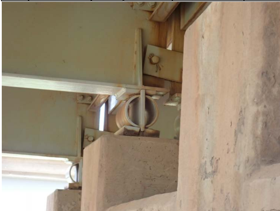
Photograph 52 - Looking northwest at the beam 2, span 5 canister bearing at pier 5. Note: beam is lifted from the canister bearing 1/16 inch.
