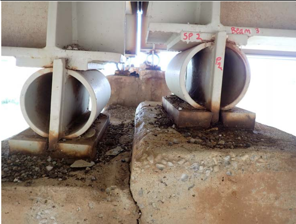
Photograph 48 - Looking east at the beam 3 canister bearings at pier 2. Note: light scaling of the concrete. Lead plugs over the anchor studs are extruded and inhibit movement of the canister.
