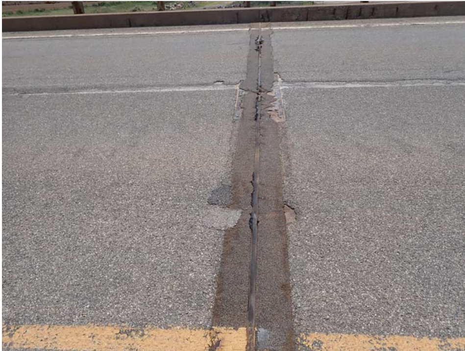
Photograph 16 - Looking east along the expansion joint over pier 2. Note: spalling at the centerline of the east travel lane, the joint seal has failed in this area. Spalling of the elastomeric covering the original finger joint plates.
