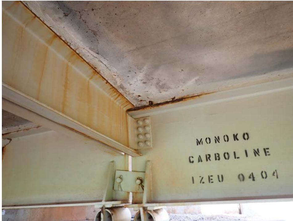
Photograph 37 - Looking southwest at beam 1 over pier 1. Note: pack rust between the beam and diaphragm top flange and the deck. Paint stencil notes IZEU paint applied April, 2004.
