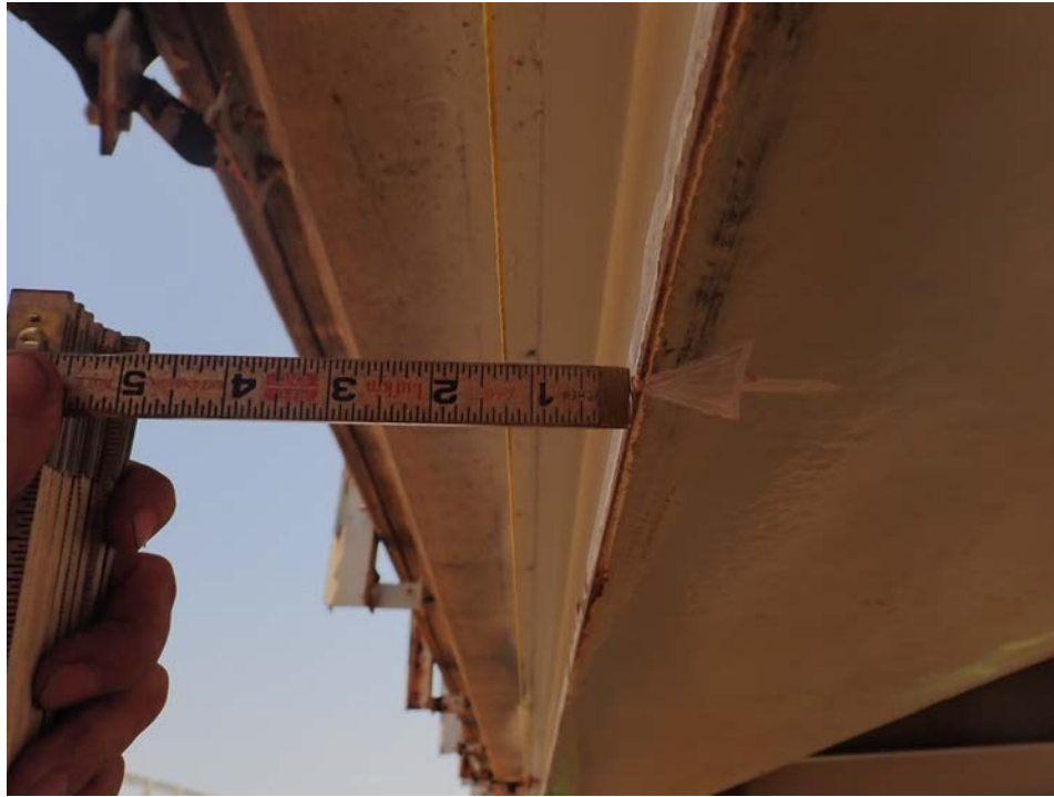
Photograph 29 - Looking north along the beam 1, span 2, near the 1/4 span. Note: 1 1/4-inch global sweep to the east.
