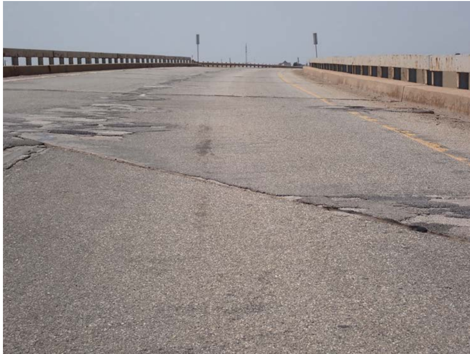
Photograph 11 - Looking south at the driving surface from the north approach. Note: patches in the asphalt overlay along the roadway centerline and joints. Minor rutting in the wheel lines and weathering of the asphalt overlay.
