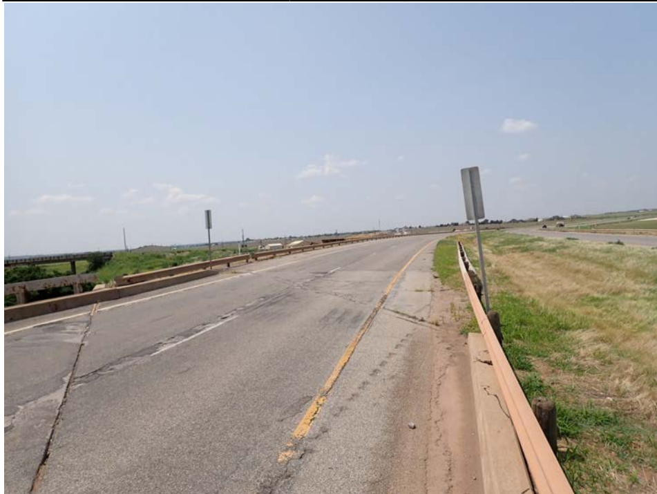
Photograph 54 - Looking south at the south approach. Note: cracks in the asphalt at the end of the approach slab.
