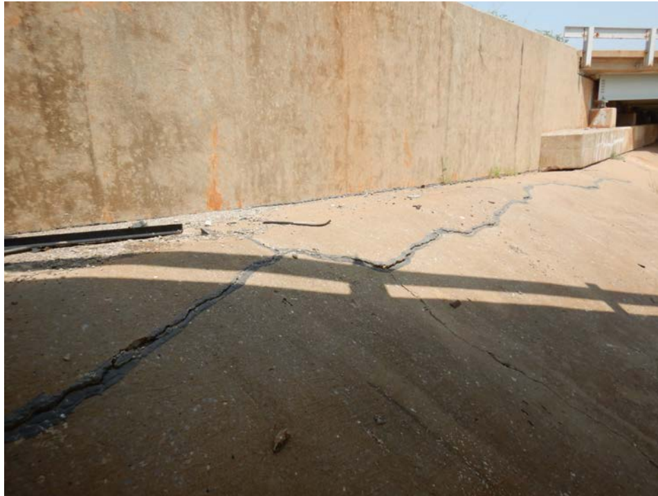
Photograph 43 - Looking west at the south embankment slope wall in the median. Note: previously sealed crack has reopened.
