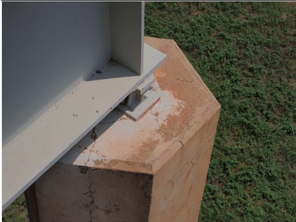
Photograph 50 - Looking northeast at column 2 at pier 3. Note: vertical cracks in column radiating from the bearing. Extruding lead bearing pad under the fixed bearing.
