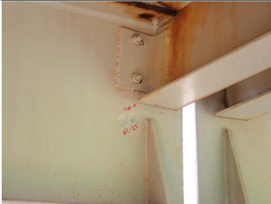
Photograph 30 - Looking northwest at beam 1, span 2, over pier 2. Note: 2 1/2-inch-long horizontal crack in weld.
