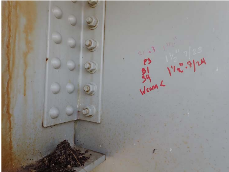
Photograph 23 - Looking southeast at the beam 1, span 4 connection angle to the pier beam at pier 3. Note: 1 1/2-inch-long vertical crack at the bottom of the connection angle. Bird droppings on beam bottom flange.
