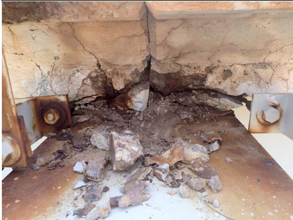
Photograph 38 - Looking east at the west deck edge over pier beam 3. Note: pack rust and active corrosion in the pier beam top flange with spalling of the deck.
