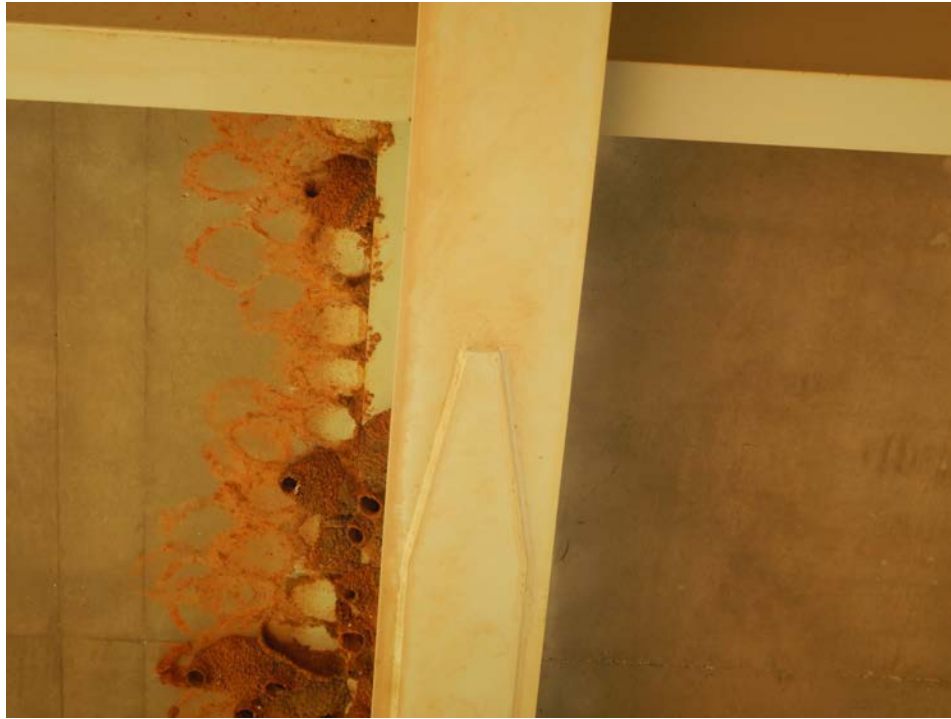
Photograph 35 - Looking up at beam 4, span 4 at the 1/4-span location. Note: welded cover plate tapered end termination.
