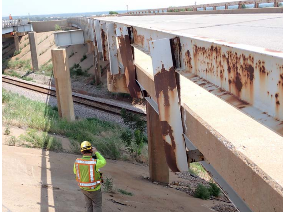
Photograph 3 - Looking north along the west bridge railing from the south abutment. Note: railing consists of a steel channel supported by steel posts. Two posts nearest the south abutment have impact damaged. Railing coating has failed.
