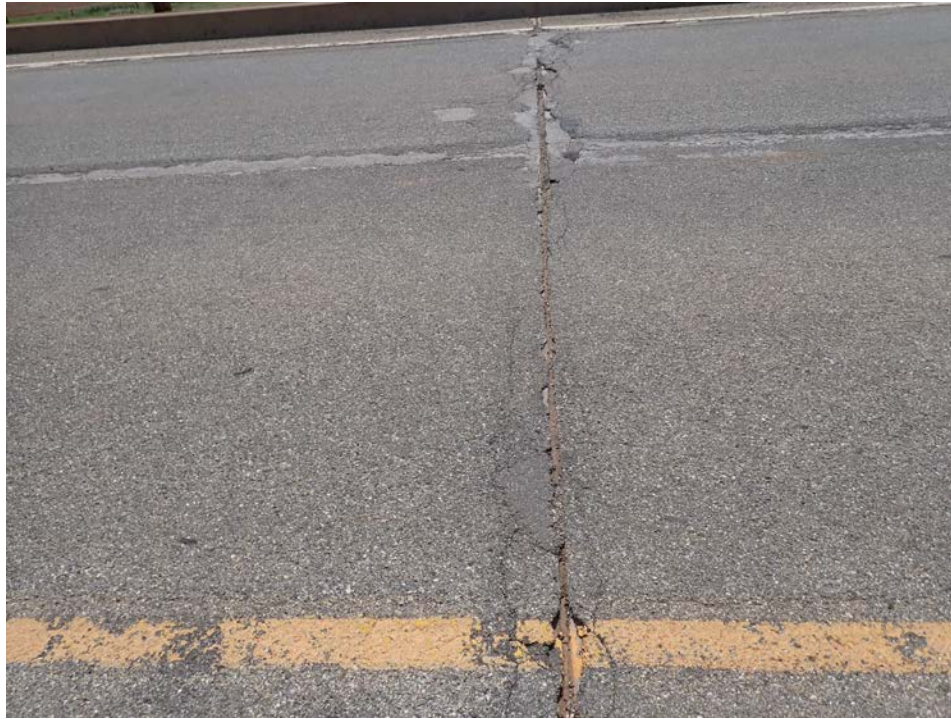
Photograph 21 - Looking east along the fixed joint over the pier beam at pier 3. Note: parallel cracks and asphalt patches exist in the asphalt wearing surface along the joint and are most prominent in the east lane. The joint seal exhibits some tears and is partially paved over.
