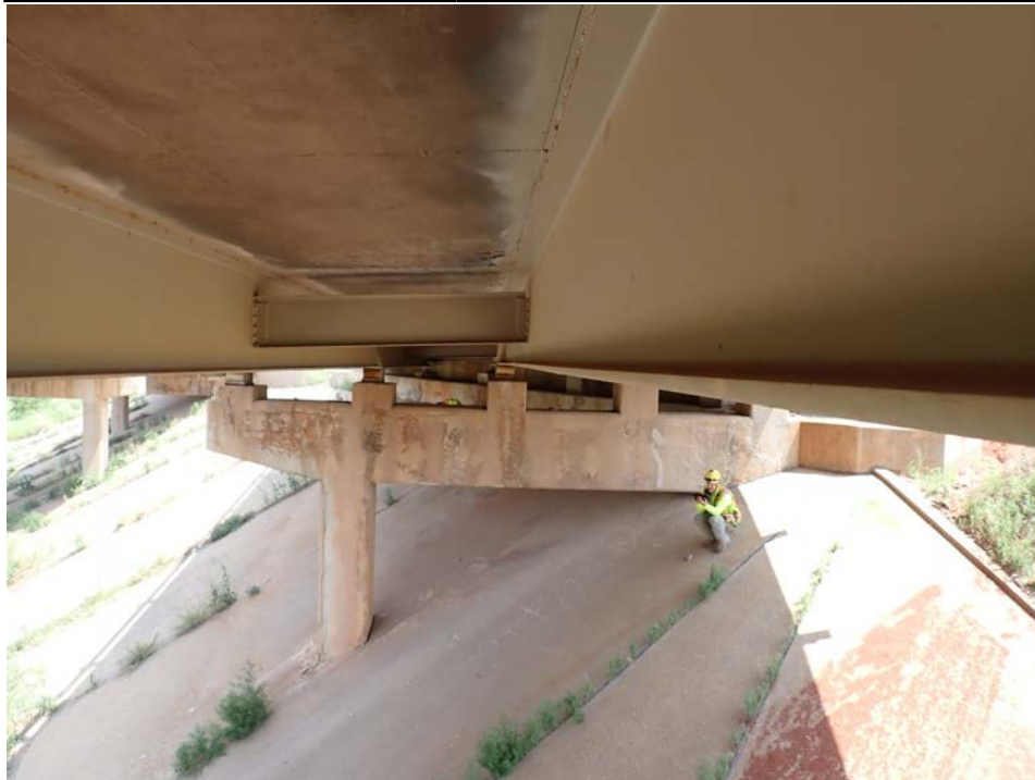
Photograph 42 - Looking north at the north embankment slope wall. Note: vegetation growing through the joints and cracks.
