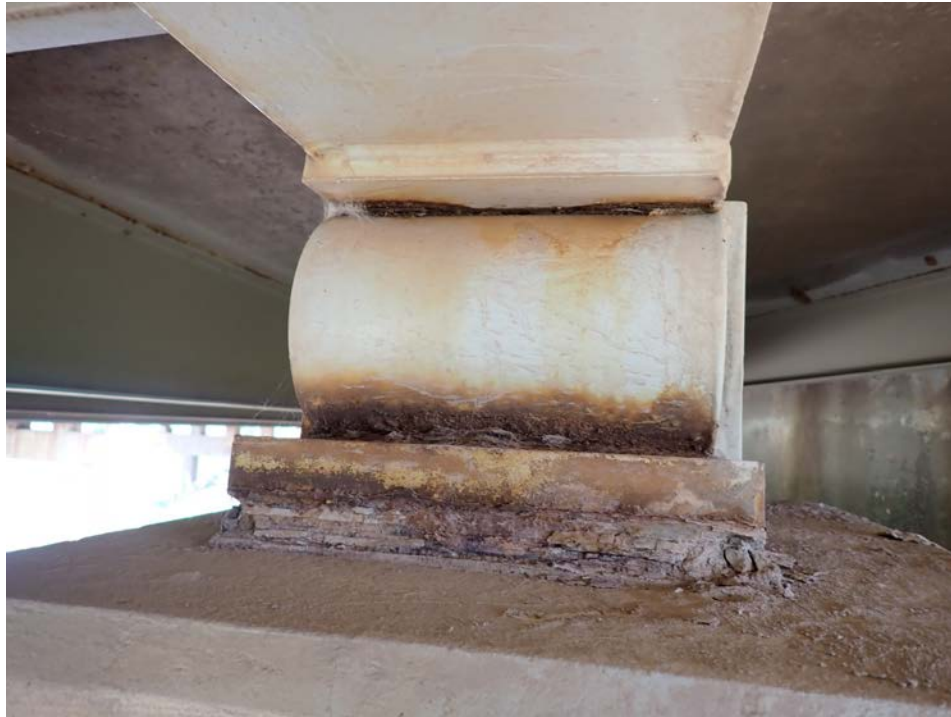
Photograph 53 - Looking north at the beam 4, span 5 canister bearing at pier 5. Note: 1-inch-thick pack between bearing pedestal and the masonry plate. Corrosion exists at the contact point between the canister and masonry and sole plates.
