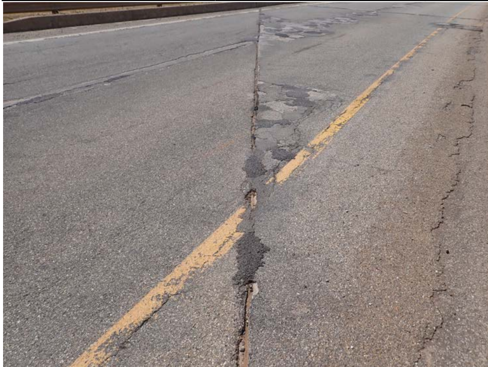
Photograph 22 - Looking southeast along the joint over the north abutment. Note: multiple asphalt patches exist along the joint. Isolated areas of the seal exhibit signs of debonding from the header.
