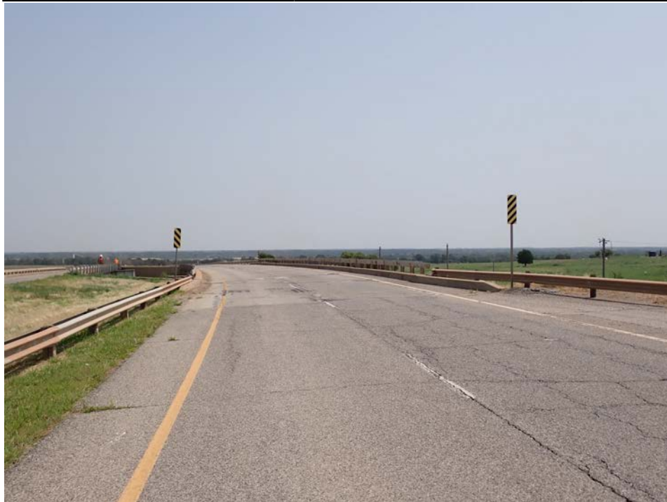
Photograph 2 - Looking north at the bridge end view. Note: approach railing is low especially at the transition. Approach railing is neither attached to nor stiffened at the bridge rail.
