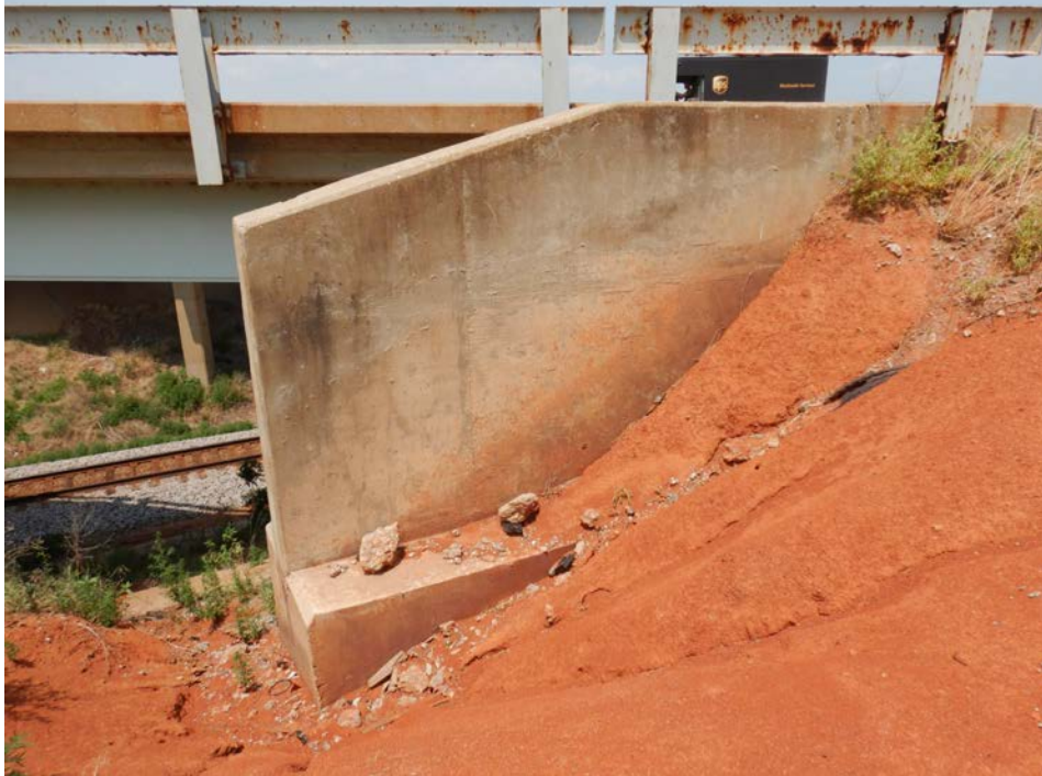
Photograph 39 - Looking south at end of the northeast wingwall. Note: erosion has exposed the top of the pile cap for 31 inches vertically. The abutment is supported by concrete piles.
