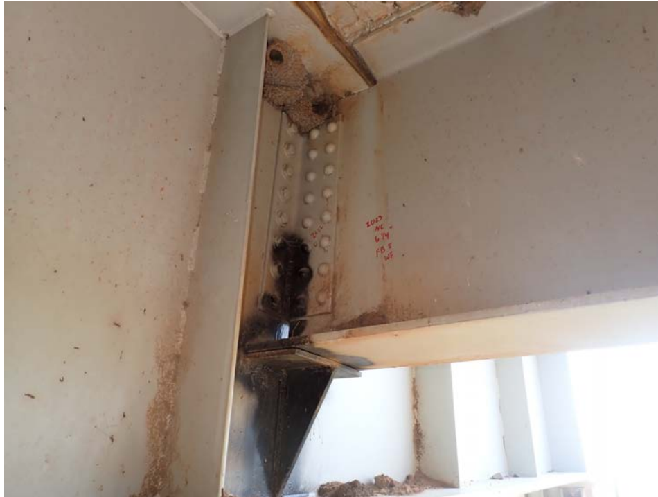
Photograph 27 - Looking northeast at the beam 5 connection angle to the pier beam at pier 3. Note: crack welded in connection angle and beam seat welded to the pier beam web. Bird nests along top flange and soil on bottom flange of pier beam.
