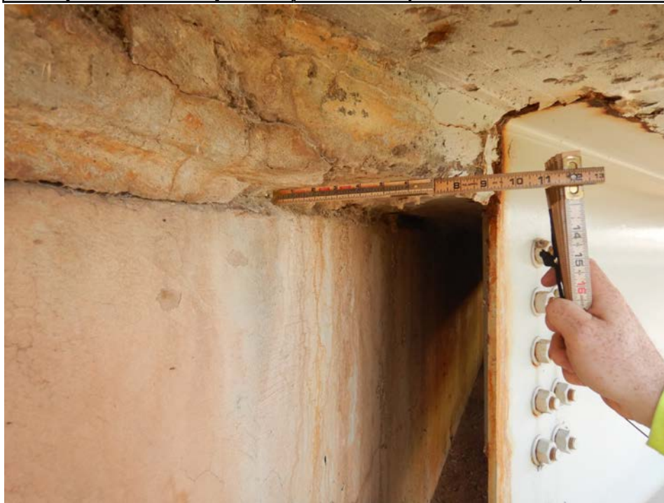
Photograph 13 - Looking east at the north abutment backwall near beam 1. Note: 1 3/8-inch longitudinal offset between end of deck and abutment backwall.
