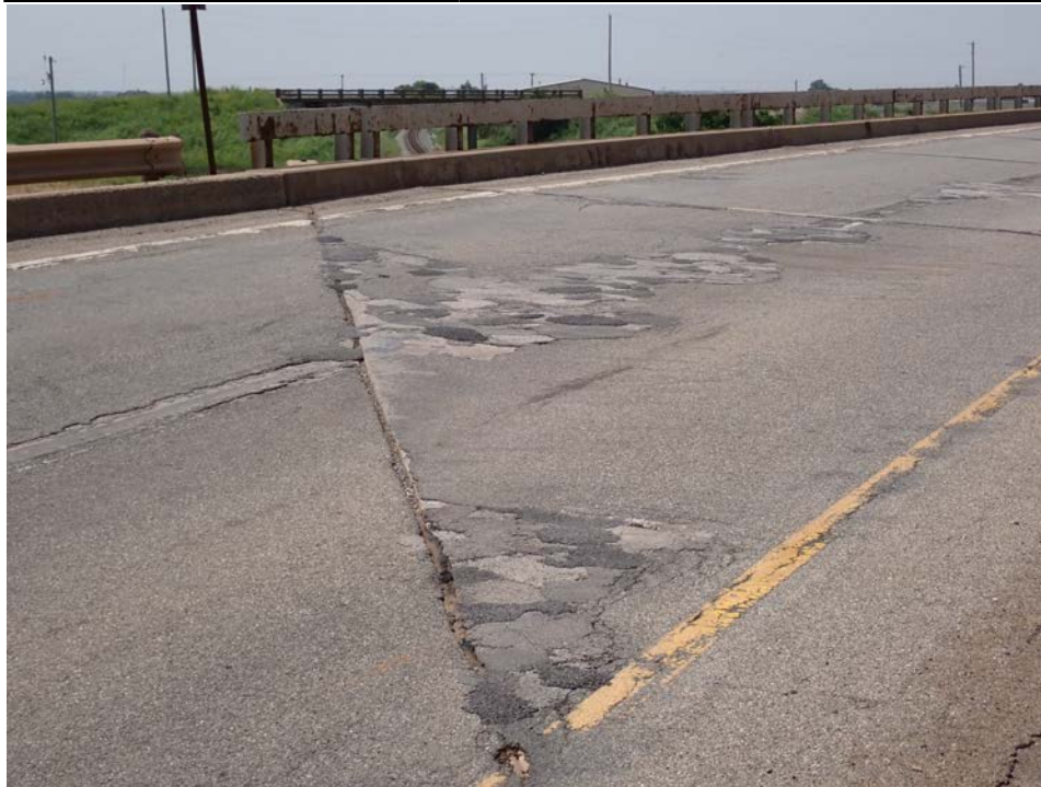
Photograph 9 - Looking southeast at the driving in span 6. Note: asphalt patches in the driving surface.
