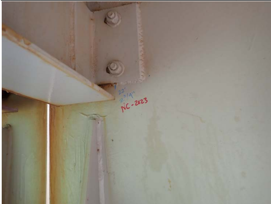
Photograph 32 - Looking west at beam 1, span 5 over pier 4. Note: 2 3/4-inch-long horizontal crack in weld.
