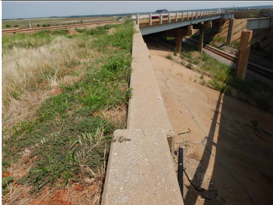
Photograph 44 - Looking northwest along the south embankment retaining wall in the median. Note: wall has rotated 3 1/2 inches north relative to the wingwall.
