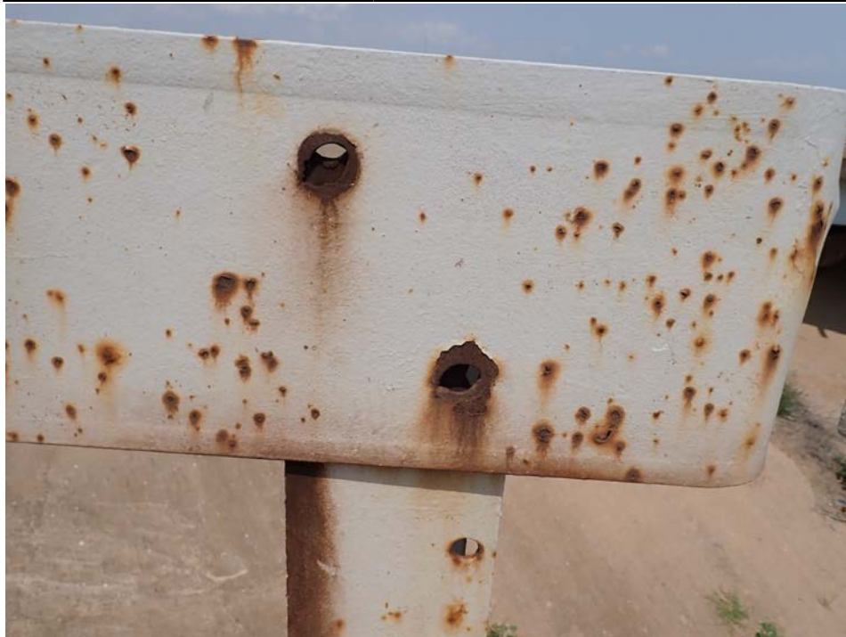
Photograph 4 - Looking west at the west bridge railing above pier 2. Note: missing bolts between the rail and post.
