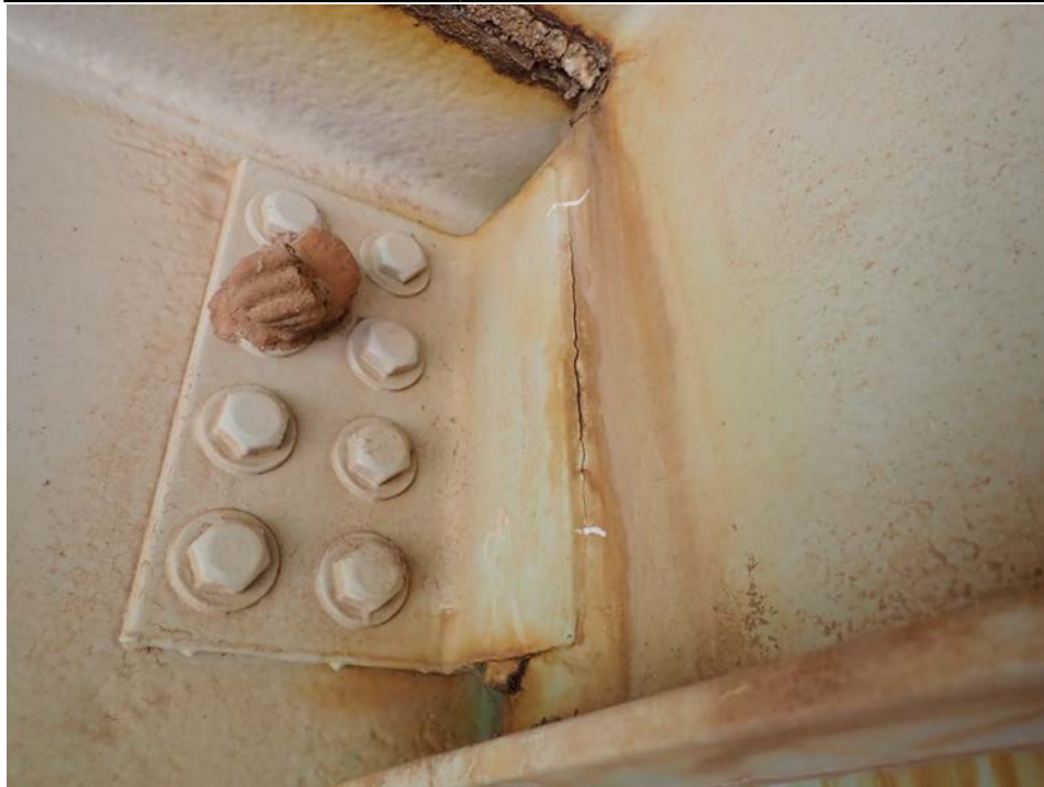
Photograph 34 - Looking southeast at beam 5, span 6 at pier 5. Note: 9-inch-long vertical crack and 4-inch-long horizontal crack in the weld.
