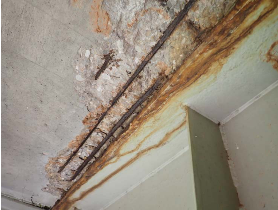
Photograph 15 - Looking southeast at the pier beam at pier 3 between beams 2 and 3. Note: spalling adjacent to the pier beam flange with exposed and corroded reinforcing steel. Corrosion reactivating where painted over pitting exists in the underside of the pier beam top flange.
