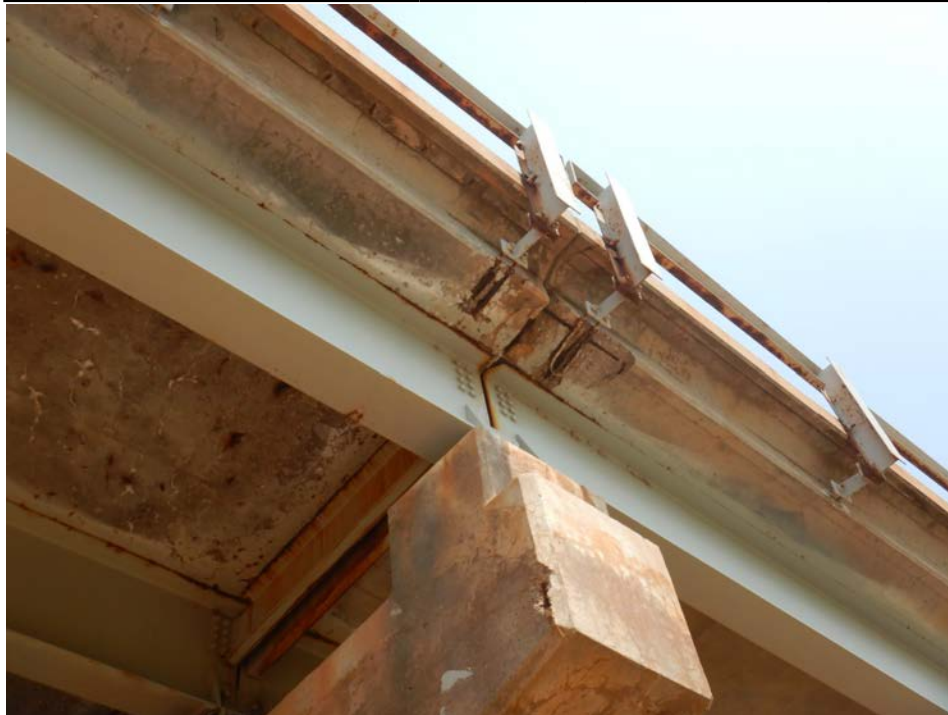
Photograph 6 - Looking up at the underside of the east overhang at pier 1. Note: soffit is spalled and anchorage for the railing posts is exposed and separating from the deck.
