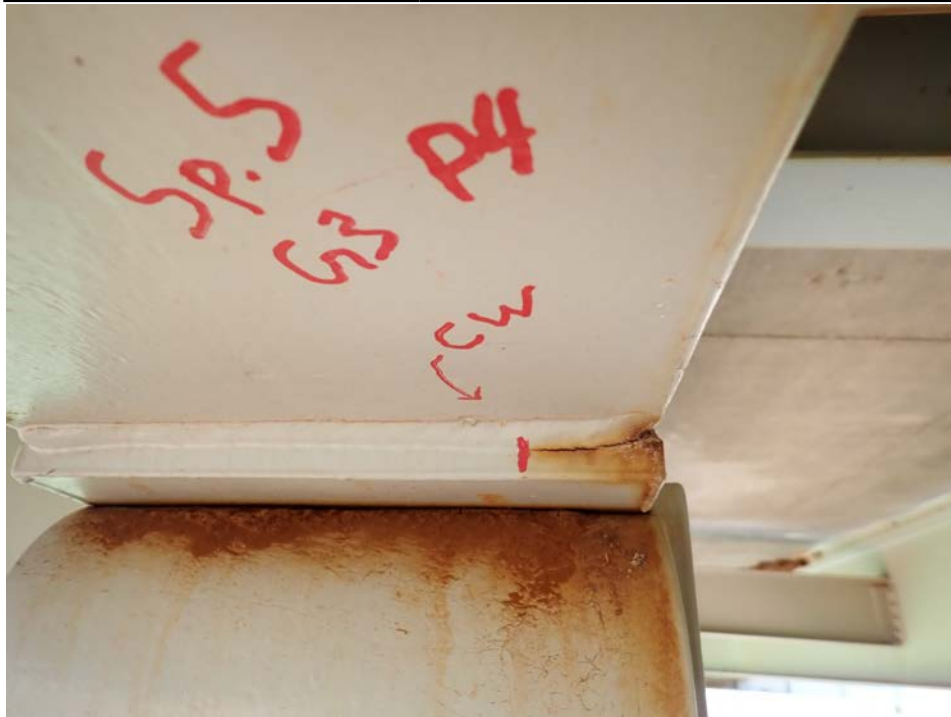
Photograph 36 - Looking south at the beam 3, span 5 canister bearing at pier 4. Note: 1 5/8-inch-long horizontal crack in the weld between the beam bottom flange and sole plate.
