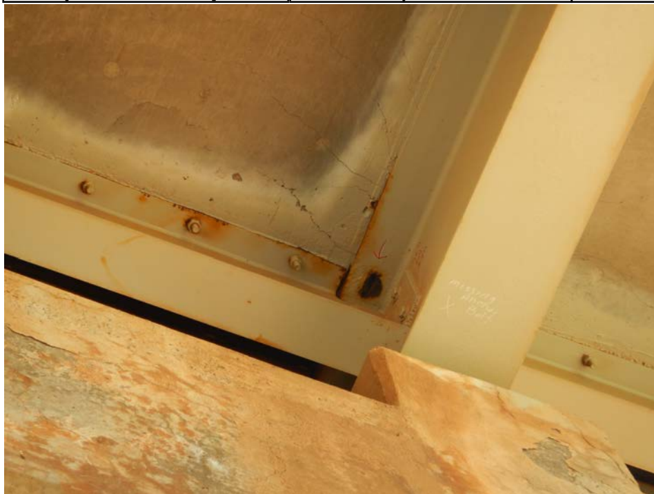
Photograph 18 - Looking up at the underside of span 4, beam 4 at the west face of pier 4. Note: missing expansion joint anchor bolt.
