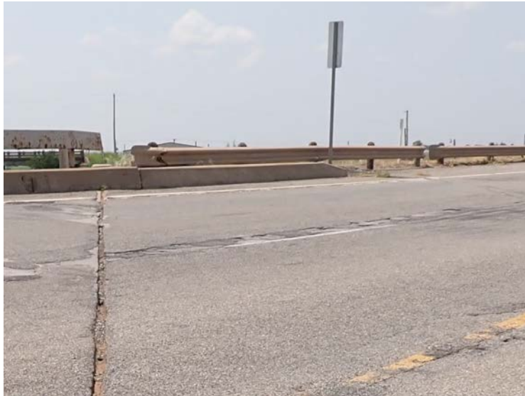
Photograph 5 - Looking southeast at the southeast approach railing. Note: break in railing has flared end treatment.
