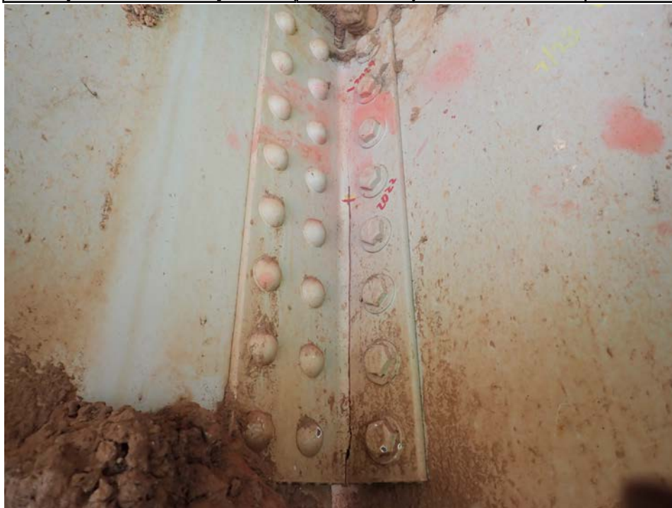
Photograph 26 - Looking northwest at the beam 4 connection angle to the pier beam at pier 3. Note: 14 1/4-inch-long crack in connection angle (1-inch growth) with additional 7-inch-long paint crack. Soil from bird nests on beam bottom flange.
