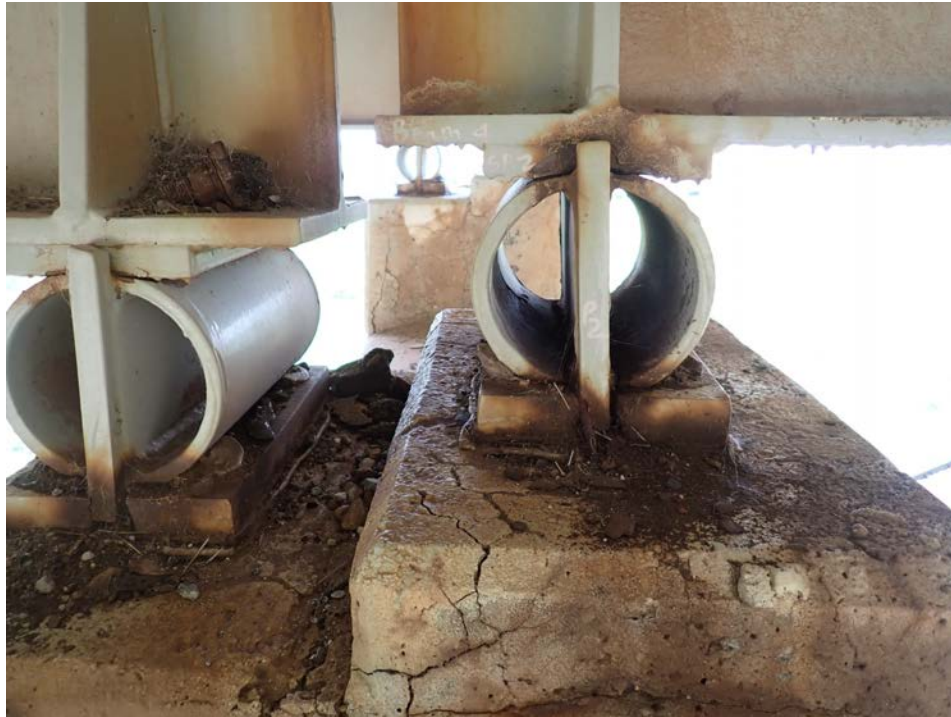
Photograph 49 - Looking east at the beam 4, span 2 canister bearing at pier 2. Note: bearing pedestal exhibits cracking and delaminations. Lead plugs over the anchor studs are extruded and inhibit movement of the canister.
