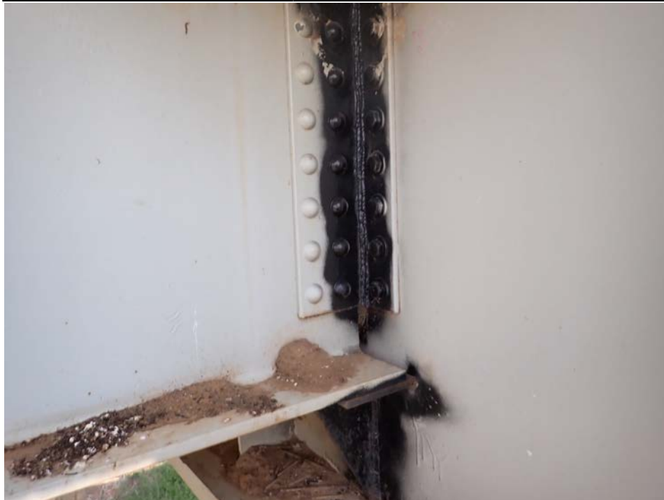
Photograph 28 - Looking northwest at the beam 5 connection angle to the pier beam at pier 3. Note: crack welded in connection angle and beam seat welded to the pier beam web. Soil and bird droppings on the beam and pier beam bottom flange.
