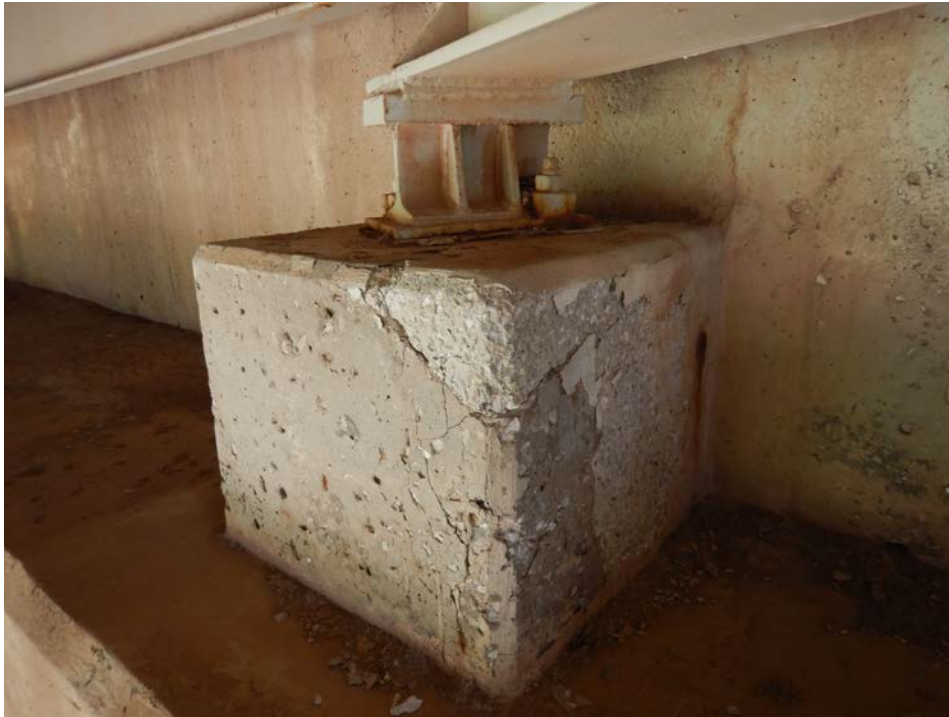
Photograph 45 - Looking north at the beam 4, span 6 bearing pedestal at the north abutment. Note: cracks and scaling concrete in the bearing pedestal. Popouts exposing aggregate and rust stains exist in the face of the pedestal. Lead bearing pad is extruding.
