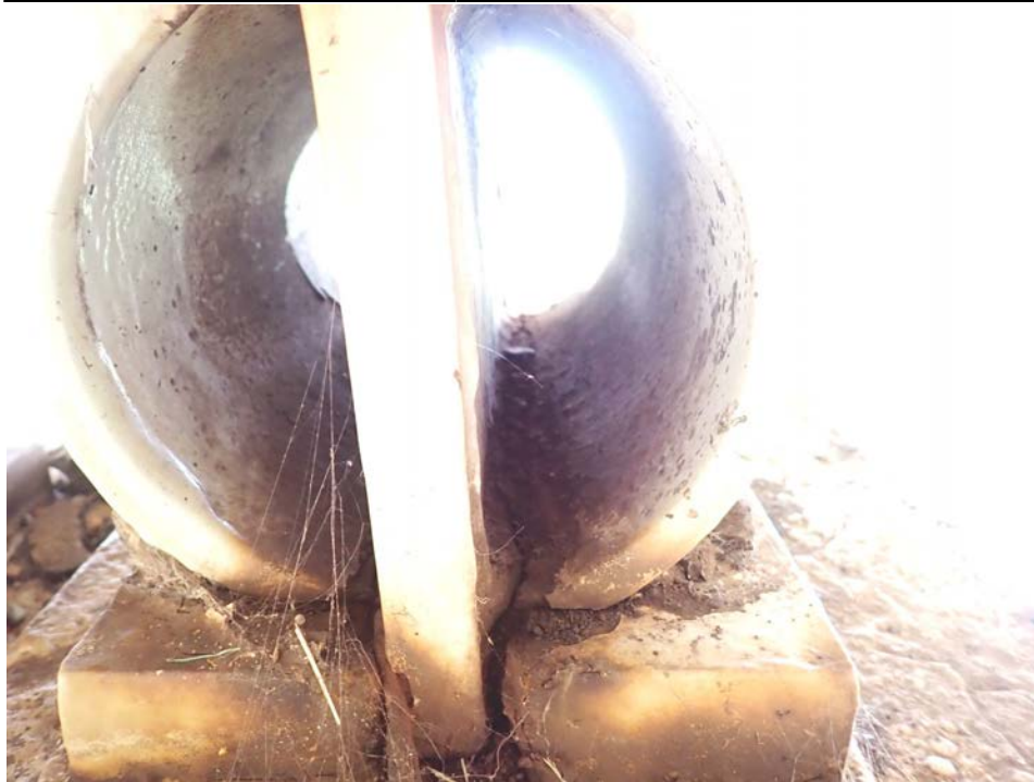
Photograph 51 - Looking east at the beam 4, span 2 canister bearing at pier 2. Note: corrosion hole in bottom of bearing with crack between canister and stiffener.
