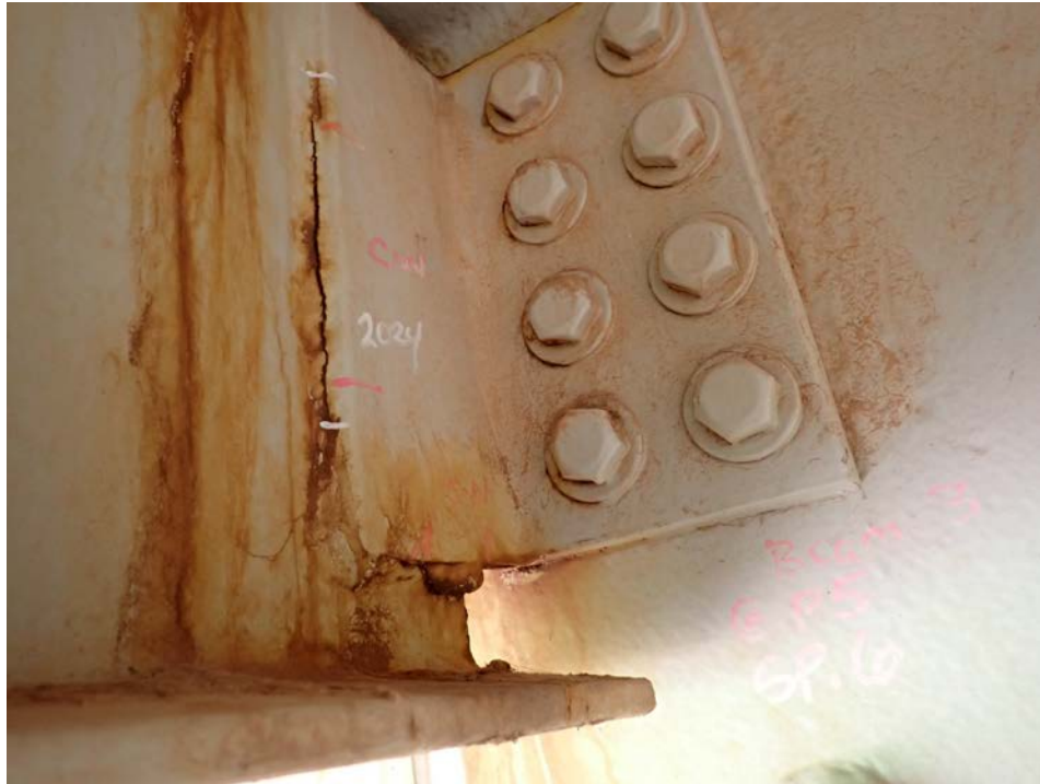
Photograph 33 - Looking northeast at beam 3, span 5 at pier 5. Note: 8-inch-long vertical crack and full length horizontal crack in the weld.
