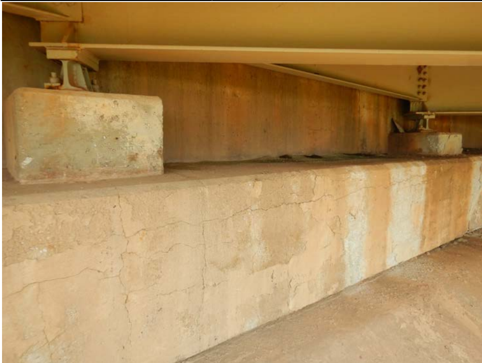
Photograph 40 - Looking southwest at the south abutment breastwall between beams 3 and 4. Note: 1/16-inch-wide vertical and horizontal cracks with delaminations throughout.
