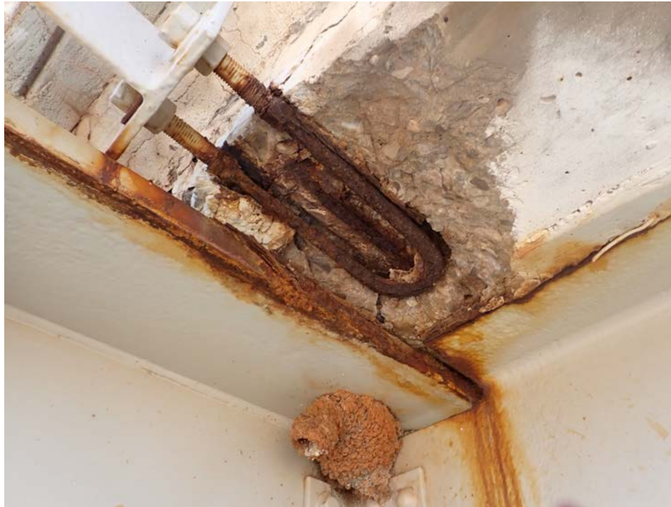
Photograph 7 - Looking northeast at the underside of the west overhang adjacent to the pier beam at pier 3. Note: heavy spalling with exposed anchor U-bolts for steel railing posts with up to 50% section loss. Corrosion of the pier beam top flange.
