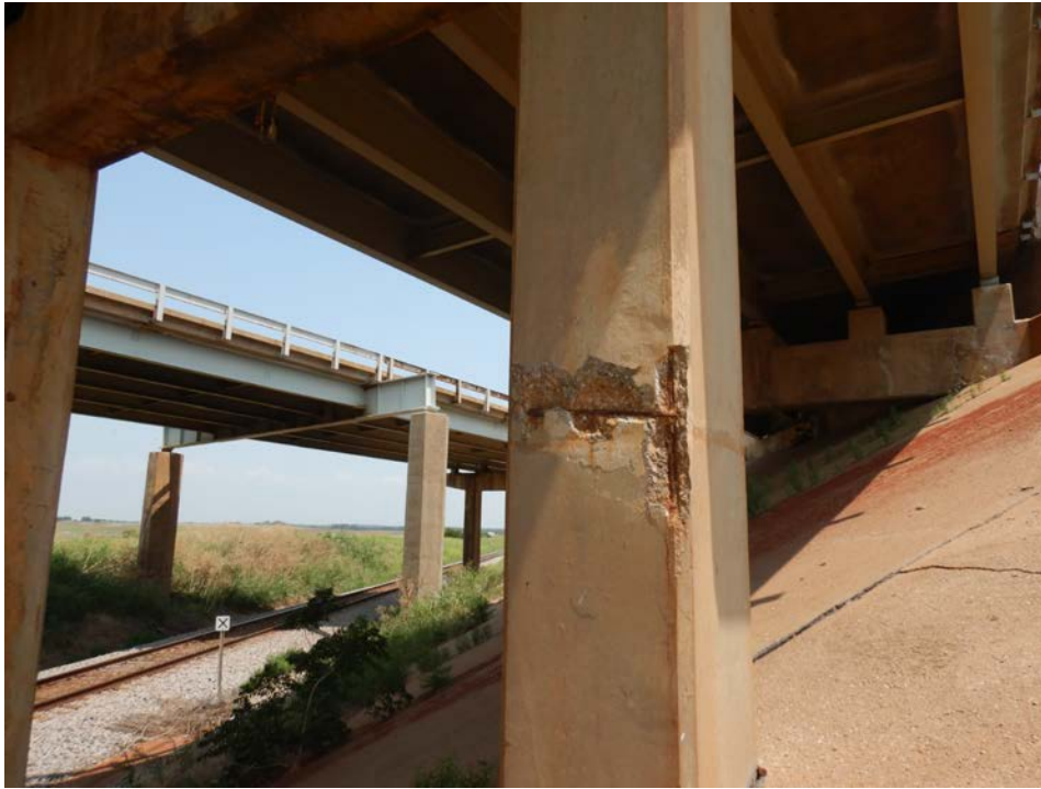
Photograph 47 - Looking north at column 2, pier 4. Note: 2-foot-vertical by full-width spall with exposed corroded reinforcing hoop steel.
