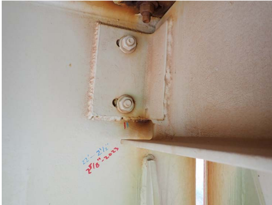
Photograph 31 - Span 4, beam 1 over pier 4. Note: 2 5/8-inch-long horizontal crack in weld.
