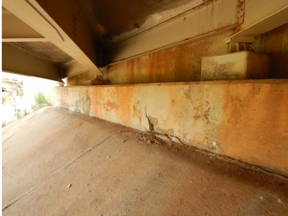
Photograph 41 - Looking northwest at the north abutment breastwall between beams 1 and 3. Note: spall with exposed reinforcing steel. Horizontal crack along the top reinforcing steel in the face of the breastwall.
