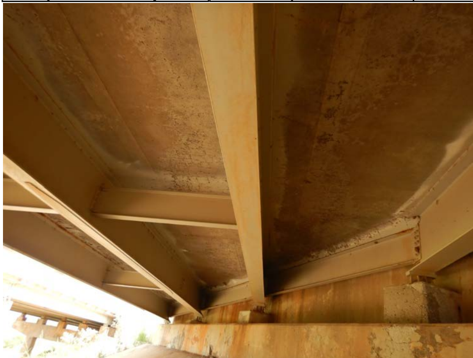
Photograph 14 - Looking north at underside of span 6 between beams 2 thru 4. Note: discolored concrete and pattern cracking in soffit.
