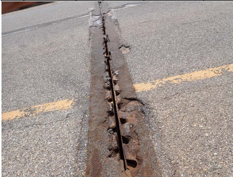
Photograph 17 - Looking east at the joint over pier 4. Note: Looking west at the pourable joint seal above pier 4. Note: seal is missing along the west travel lane and partially along the west half of the east lane.
