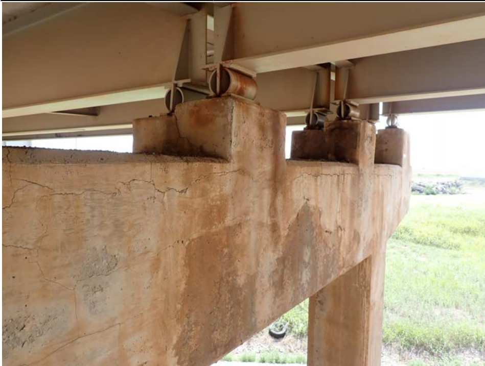
Photograph 46 - Looking northeast at pier 2. Note: pier exhibits cracking and delaminations.
