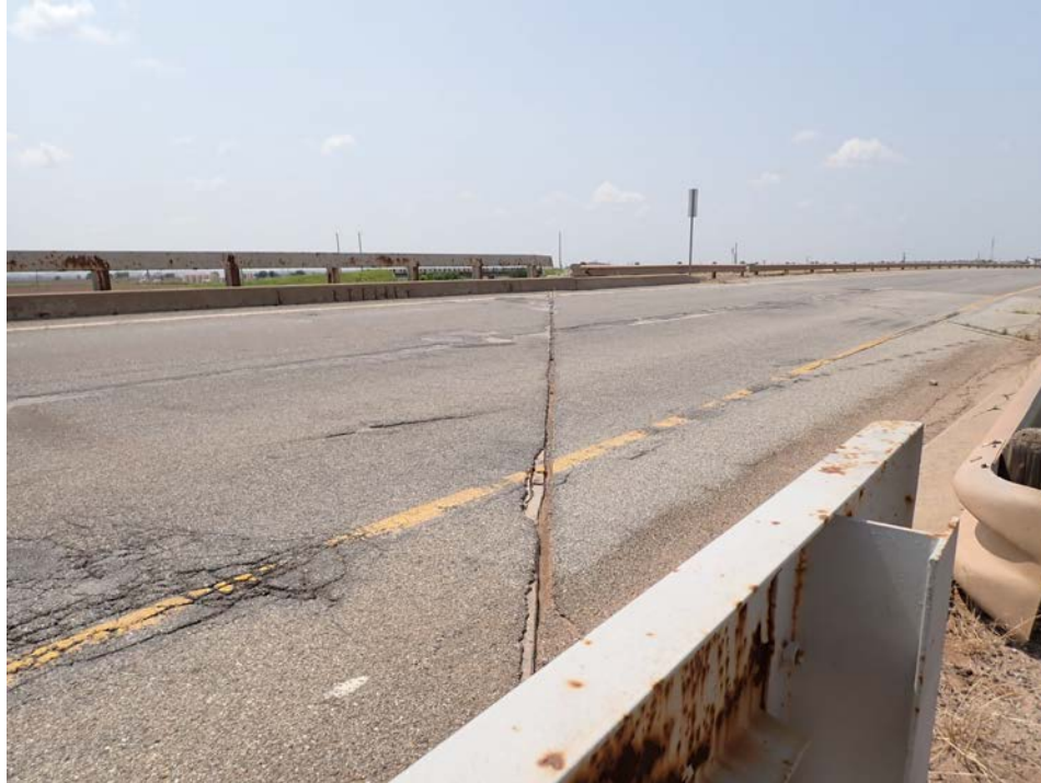
Photograph 19 - Looking southeast along the fixed joint over the south abutment. Note: minor edge spalls and patches exists in the asphalt wearing surface along the joint with evidence of leakage.
