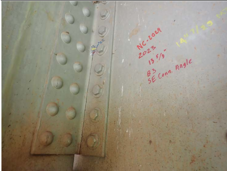
Photograph 25 - Looking northwest at the beam 3 connection angle to the pier beam at pier 3. Note: 14-inch-long crack along the bottom of the connection angle.
