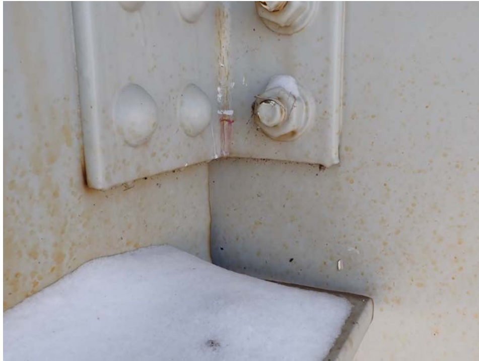
Photograph 3 - Looking southeast at the beam 1, span 4 west connection angle to the north face of the pier beam at pier 3. Note: 1 1/2-inch-long vertical crack (no change).
