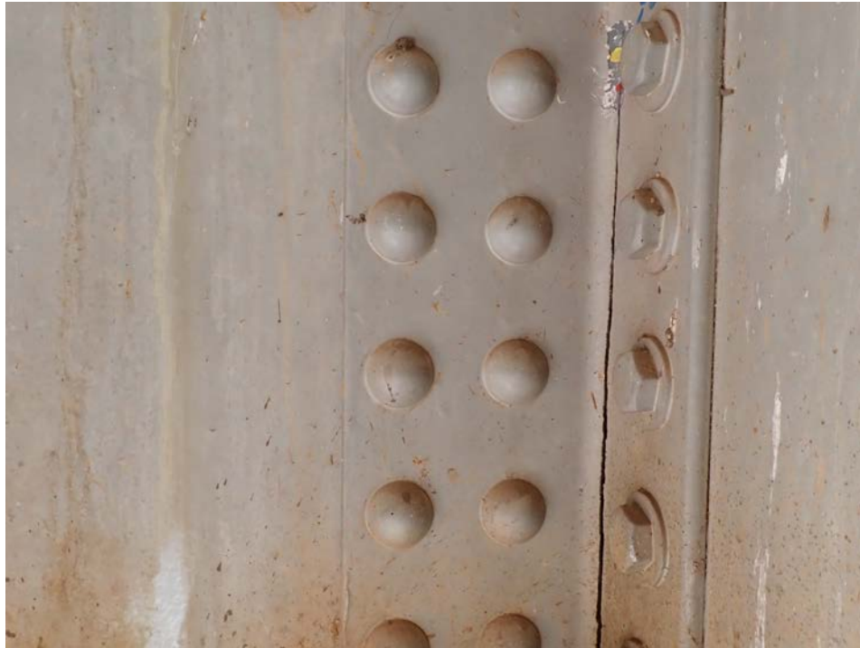
Photograph 5 - Looking northwest at the beam 3, span 3 east connection angle to the south face of the pier beam at pier 3. Note: 14-inch-long overall vertical crack (no change).
