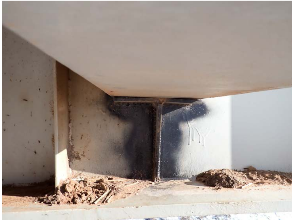
Photograph 7 - Looking north along the beam 5, span 3 bottom flange at the connection to the pier beam at pier 3. Note: seat has been installed beneath the beam.
