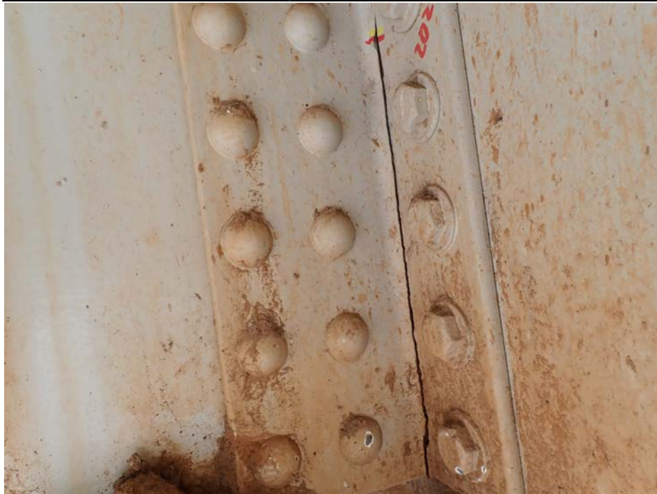
Photograph 6 - Looking northwest at the beam 4, span 3 east connection angle to the south face of the pier beam at pier 3. Note: 13 3/4-inch-long vertical crack (1/2-inch growth)..
