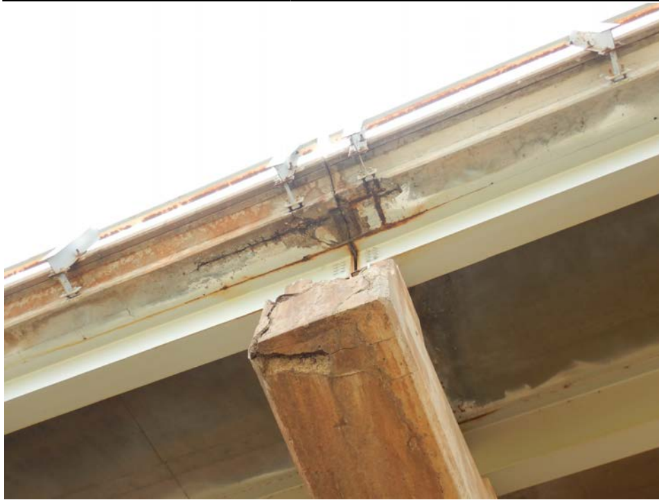
Photograph 41 - Looking up at the west end of the pier 5 cap. Note: spall in the west end of the cap adjacent to the beam 1 bearing.
