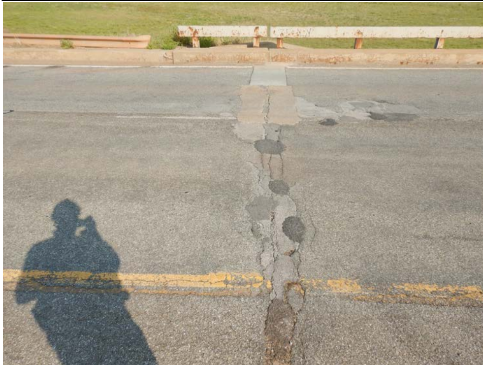
Photograph 13 - Looking north along the expansion joint over pier 1. Note: asphalt and concrete patches exist along the joint.
