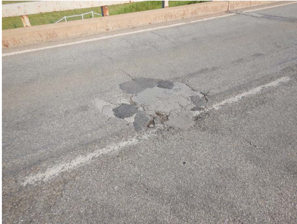
Photograph 9 - Looking northwest at the driving surface in span 3. Note: 3-foot-diameter asphalt patch at the roadway centerline. Cracks exist in the asphalt along the roadway centerline and the west lane.
