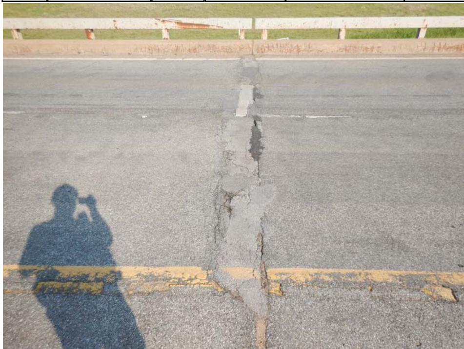
Photograph 18 - Looking west along the poured seal fixed joint over pier 3. Note: asphalt and concrete patches exist along the joint.
