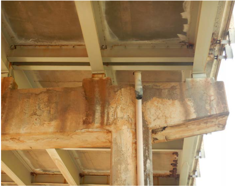
Photograph 43 - Looking south at the west end of the pier 4 cap. Note: cracks with corrosion stains and delaminations exist in the vertical face and underside of the cap.
