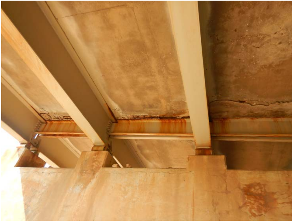
Photograph 11 - Looking south at the underside of span 2 at pier 1 between beams 1 and 4. Note: spalling with exposed reinforcing steel along the end diaphragm. Full-depth patch exists between beams 3 and 4.
