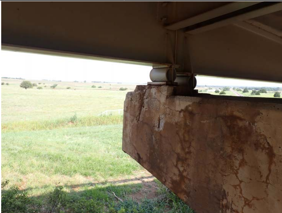
Photograph 44 - Looking northwest at the beam 1 bearing pedestal on pier 2. Note: spall encroaching on the masonry plate with exposed reinforcing steel. Discolored concrete exists in the cap.
