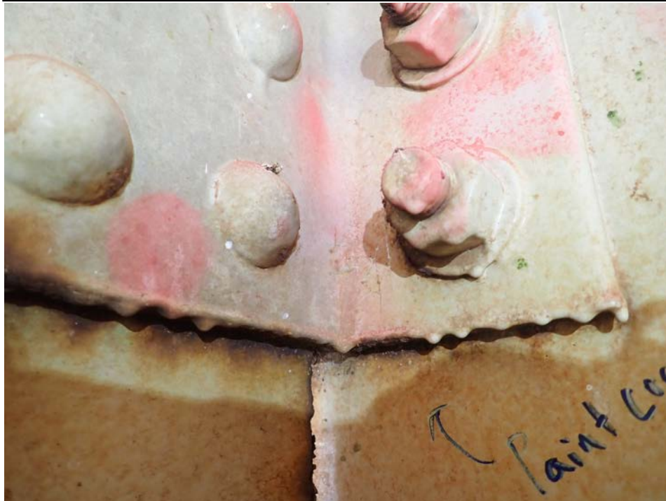
Photograph 24 - Looking southeast at the beam 3, span 4 northwest connection angle to the pier beam at pier 3. Note: fine paint cracks in the bottom typical paint cracks at the bottom of the connection angle.
