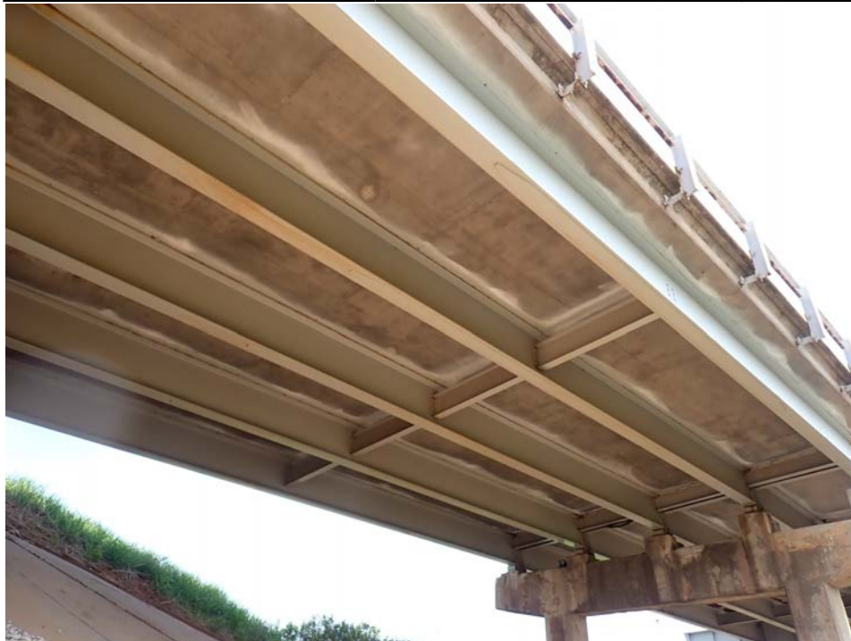
Photograph 28 - Looking northwest at the underside of span 2. Note: partial-length welded cover plates exist on the bottom flange of the beams.
