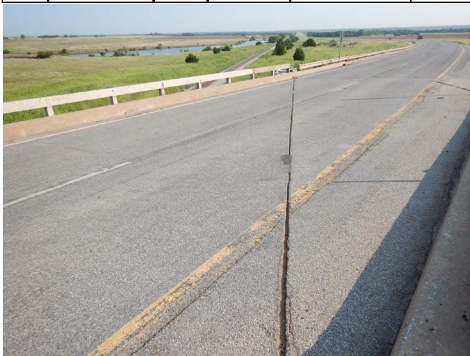
Photograph 20 - Looking northwest along the poured seal fixed joint over the south abutment. Note: few asphalt patches along the joint.
