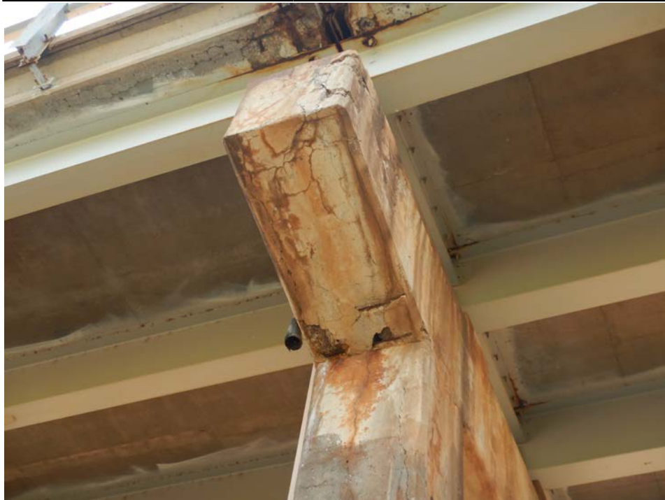
Photograph 38 - Looking up at the west end of the pier 4 cap. Note: cracking and spalling.
