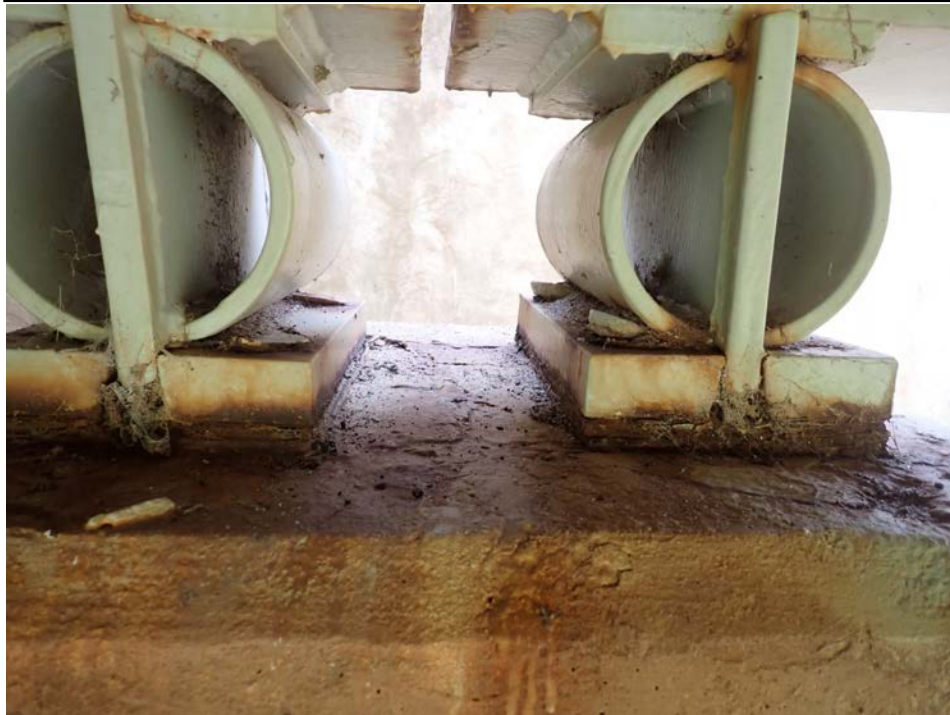
Photograph 48 - Looking east at the beam 5 canister bearing at pier 5. Note: lead plugs are extruded and inhibit expansion of the canisters. Pack rust exists between the masonry plate and the bearing seat.
