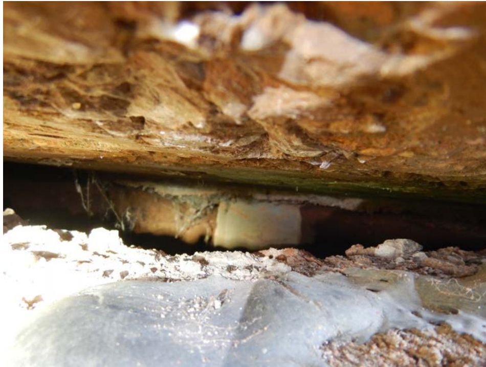
Photograph 33 - Looking south beneath the south abutment breastwall near the west end. Note: settlement of the embankment has exposed one concrete pile.
