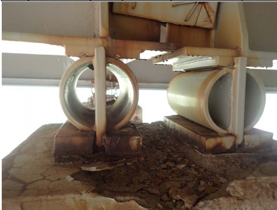
Photograph 46 - Looking west at the beam 4 canister bearings at pier 5. Note: scaling concrete in the bearing seat adjacent to the masonry plates. Beam 4, span 6 bearing is lifted from the canister.
