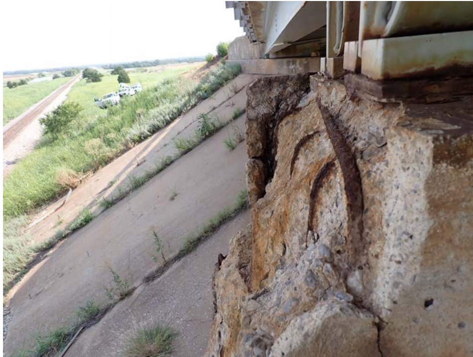
Photograph 47 - Looking north at the west end of pier 5. Note: scaling concrete has undermined the southwest corner of the beam 5, span 5 masonry plate 1 inch.
