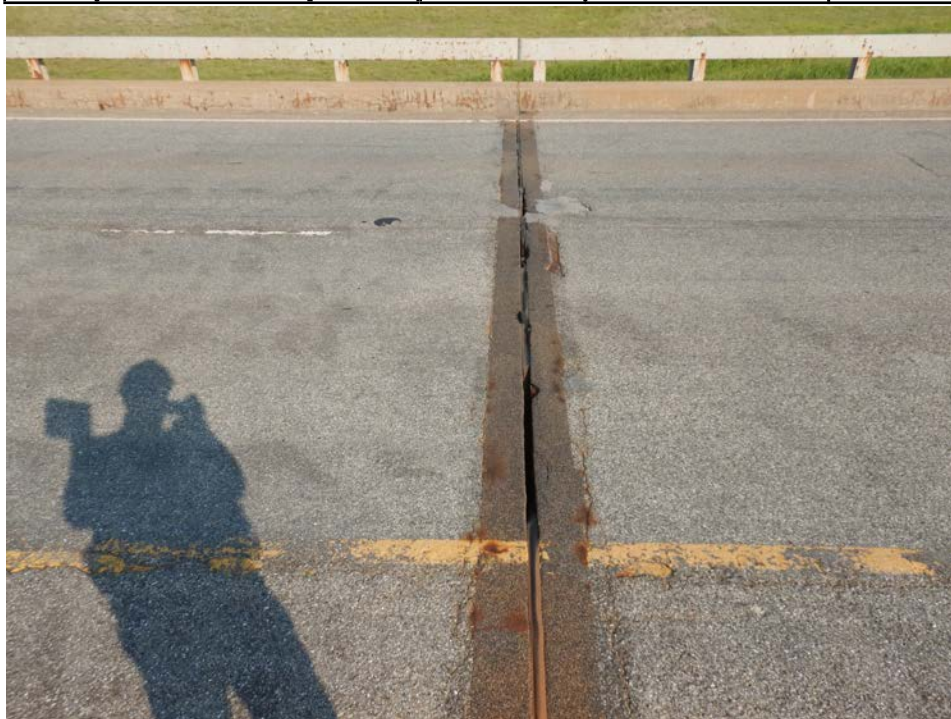
Photograph 16 - Looking west along the poured seal expansion joint over pier 4. Note: seal is missing in both lanes. Joint is closed at the west bridge railing. Rust stains exist along the edges of the elastomeric concrete header.
