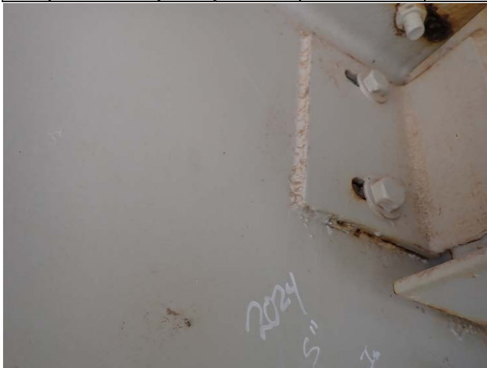
Photograph 26 - Looking northwest beam 2, span 4 at pier 4. Note: 5-inch-long horizontal crack in the bottom weld between the end diaphragm connection angle and the beam web.
