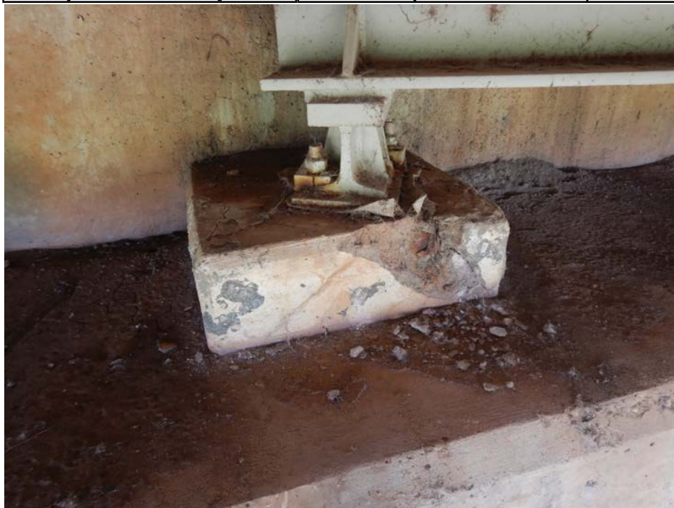
Photograph 32 - Looking east at the beam 2, span 6 bearing pedestal at the north abutment. Note: spall encroaching on the bearing. Lead bearing pad extruded along the south and west edges.
