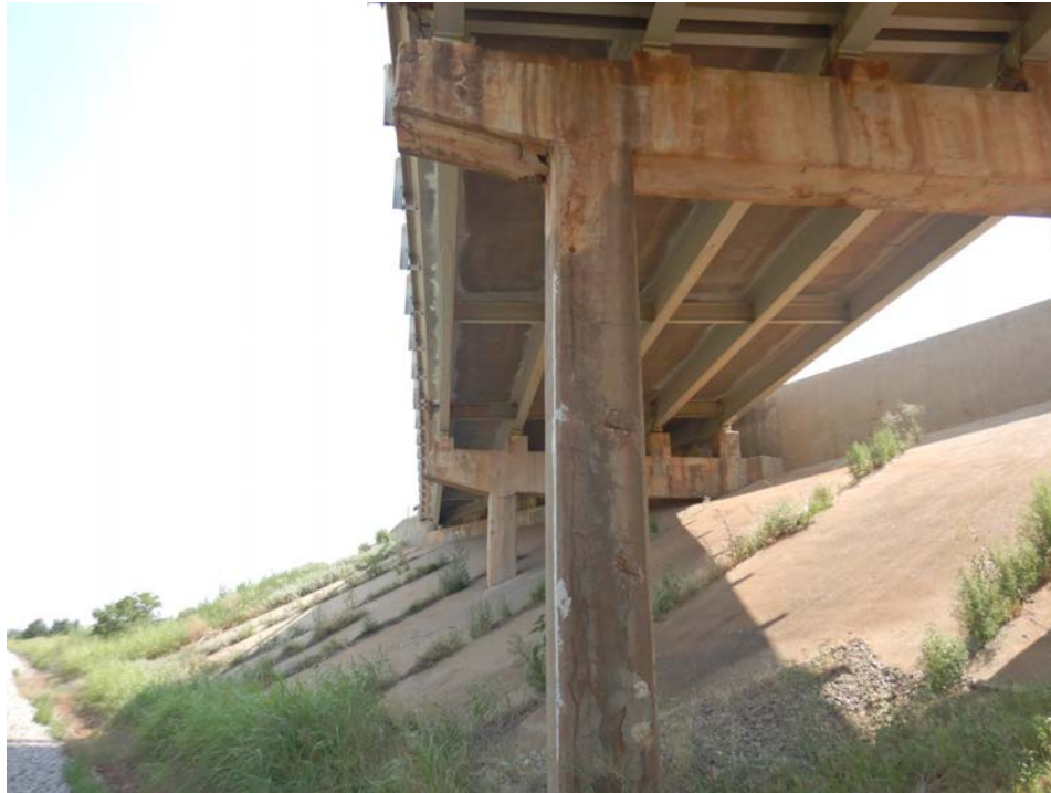
Photograph 37 - Looking north at pier 4, column 1. Note: cracks and spalls with exposed reinforcing steel.
