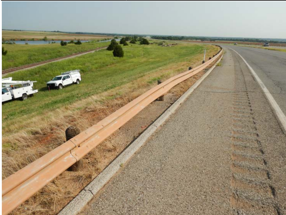
Photograph 4 - Looking north along the northwest approach railing. Note: approach railing is low and blockouts were not used.
