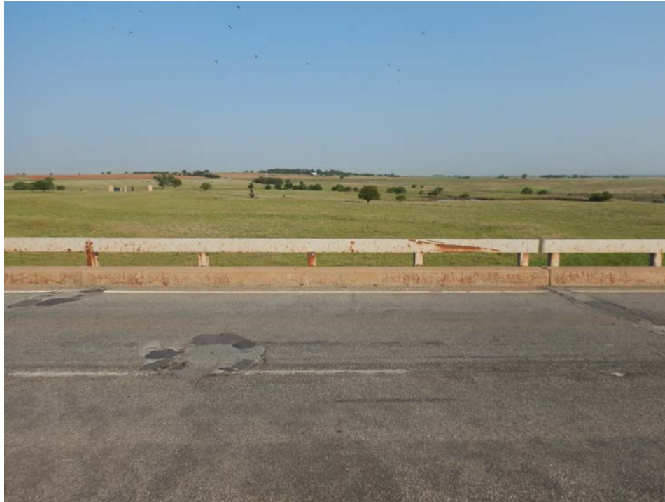
Photograph 3 - Looking west at the west bridge railing in span 4. Note: the railing is obsolete. Cracks with corrosion stains exists in the face of the curb and impact damage exists to the rail.
