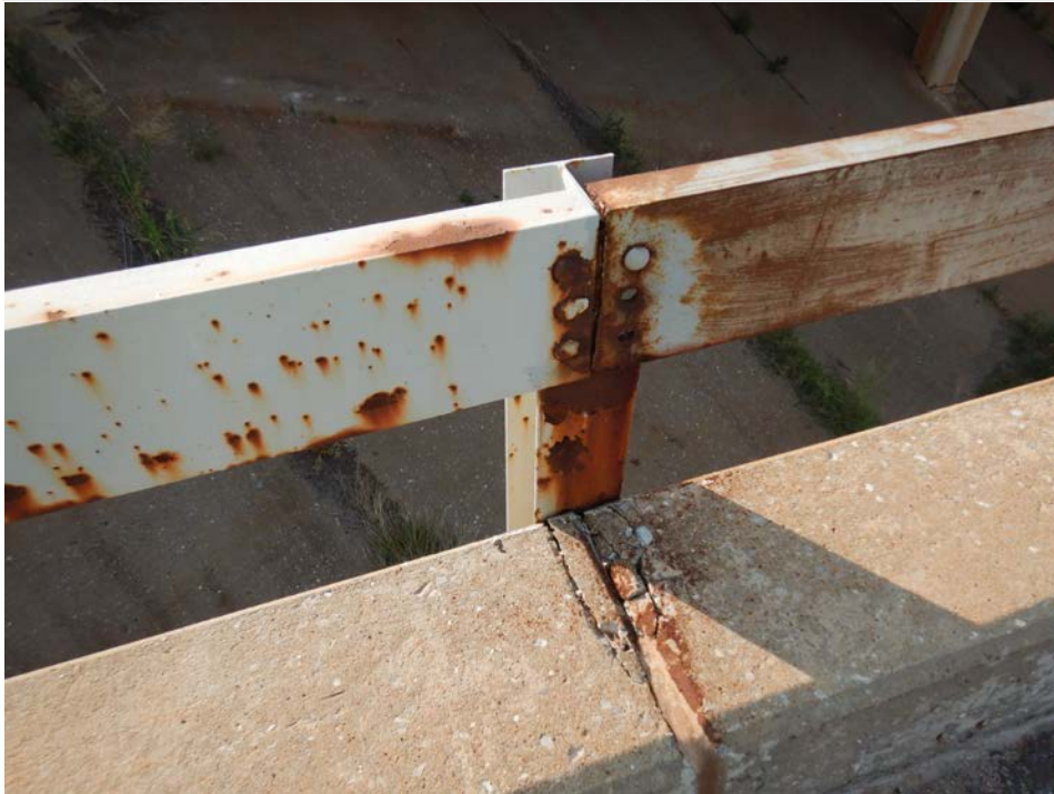
Photograph 6 - Looking east at the east bridge railing at the 5th post in span 3. Note: typical surface corrosion to the rail and post, and missing connection bolts
