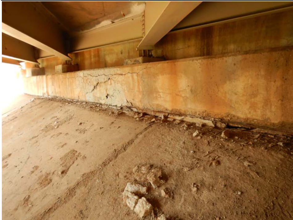
Photograph 30 - Looking south at the south abutment. Note: horizontal cracks in the breastwall with areas of delaminations and spalls forming.
