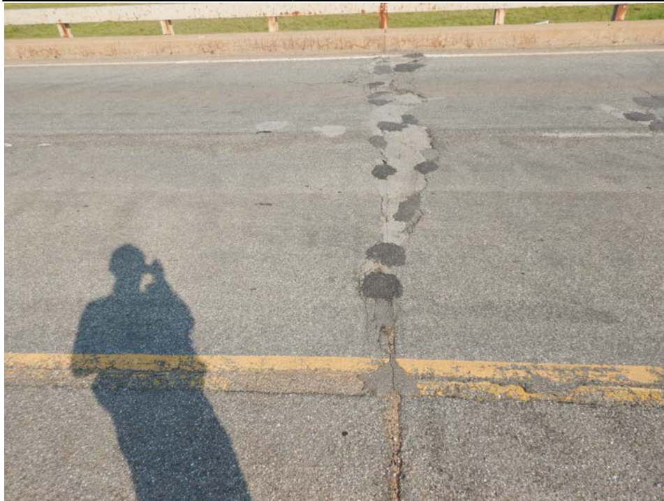
Photograph 10 - Looking west along the north deck control joint in span 3. Note: asphalt patches along the control joint.
