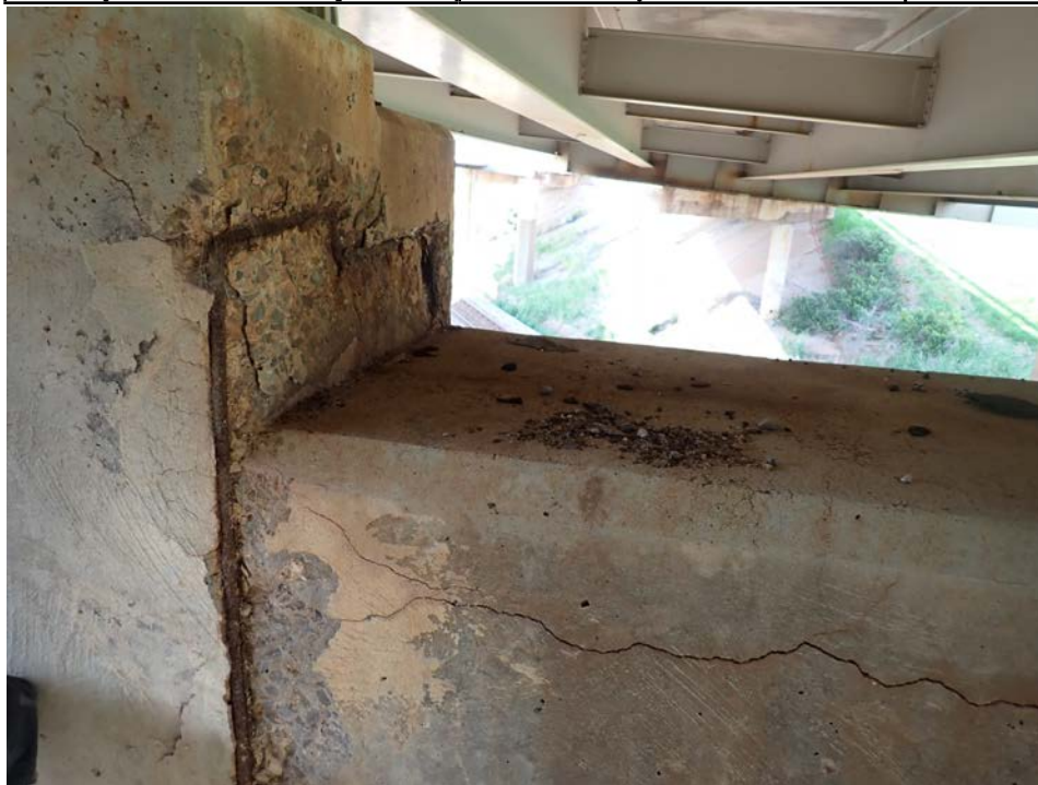
Photograph 45 - Looking south at the west face of the beam 4 bearing pedestal on pier 4. Note: spall with exposed reinforcing steel.
