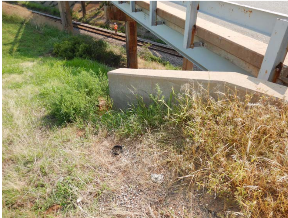
Photograph 29 - Looking northeast at the southwest wingwall. Note: back face of wingwall exposed due to erosion.
