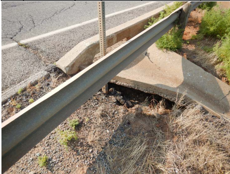
Photograph 51 - Looking south at the northwest corner of the north approach slab. Note: paved drainage flume undermined with approximately 1 foot of penetration.
