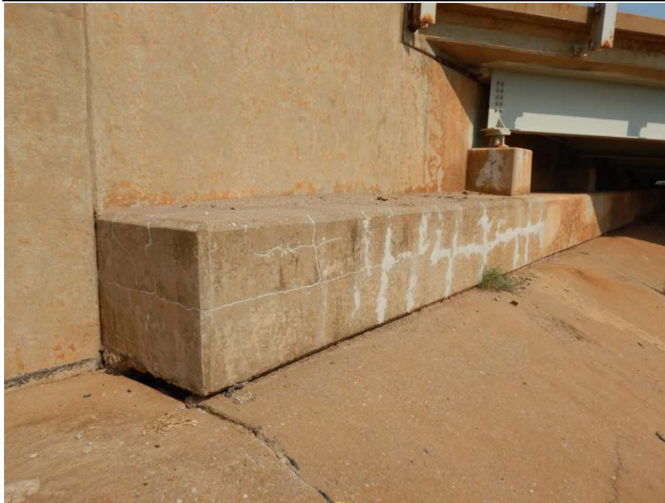
Photograph 31 - Looking southwest at east end of the south abutment. Note: cracks in the breastwall have been seal. Breastwall and slope wall undermined due to settlement of the embankment.
