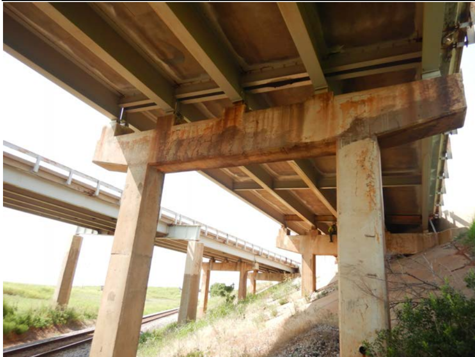
Photograph 36 - Looking south at pier 2. Note: cracking and spalling in column 1 and pier cap.
