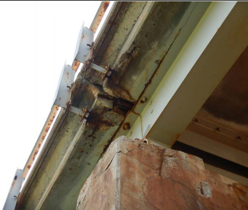
Photograph 8 - Looking northeast at the west overhang at pier 2. Note: spall in soffit exposing the U-bolt anchorage for the bridge railing post.
