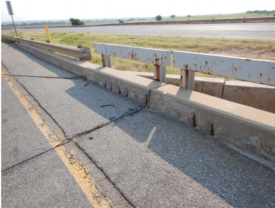
Photograph 5 - Looking northeast at the northeast approach railing and east bridge railing in spans 5 and 6. Note: approach railing transition is insufficient with flared end approach rail termination at the bridge. Curb is spalled with exposed reinforcing steel due to insufficient cover.
