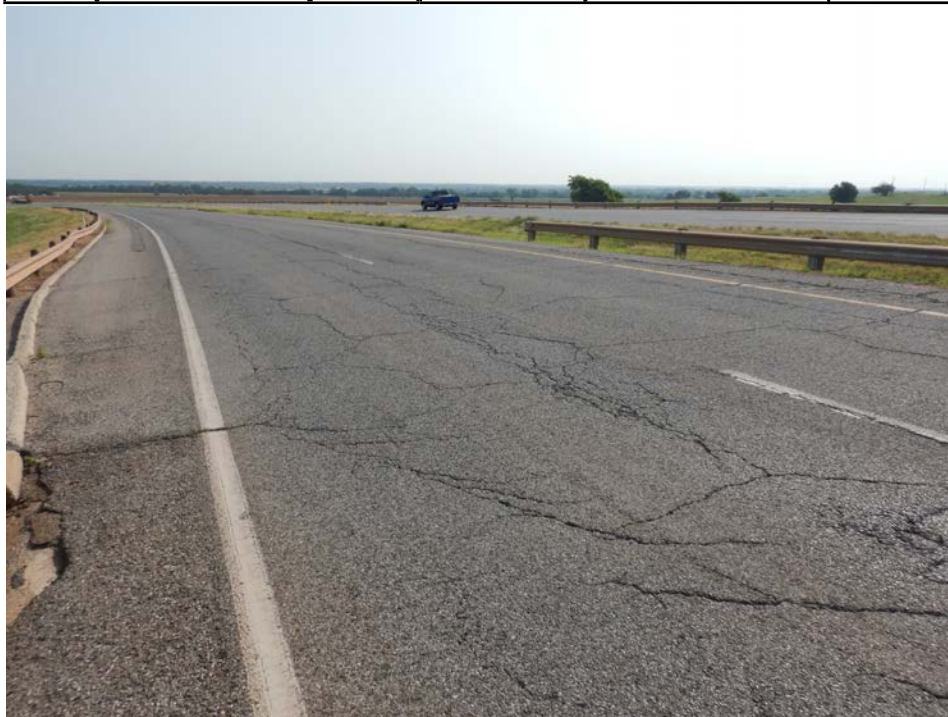
Photograph 50 - Looking northeast at north approach asphalt roadway. Note: longitudinal cracking in the wheel paths.
