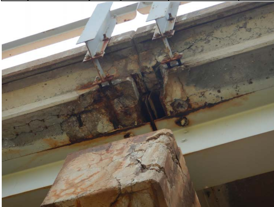
Photograph 14 - Looking east at Underside of deck overhang at Pier 4. Note: spalling and cracking at u bolts for bridge railing.
