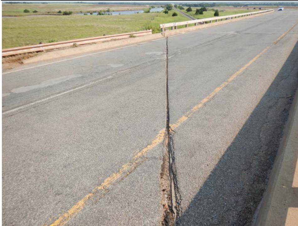
Photograph 17 - Looking northwest along the poured seal fixed joint over the south abutment. Note: minor spalling and patching of the asphalt exists along the joint.
