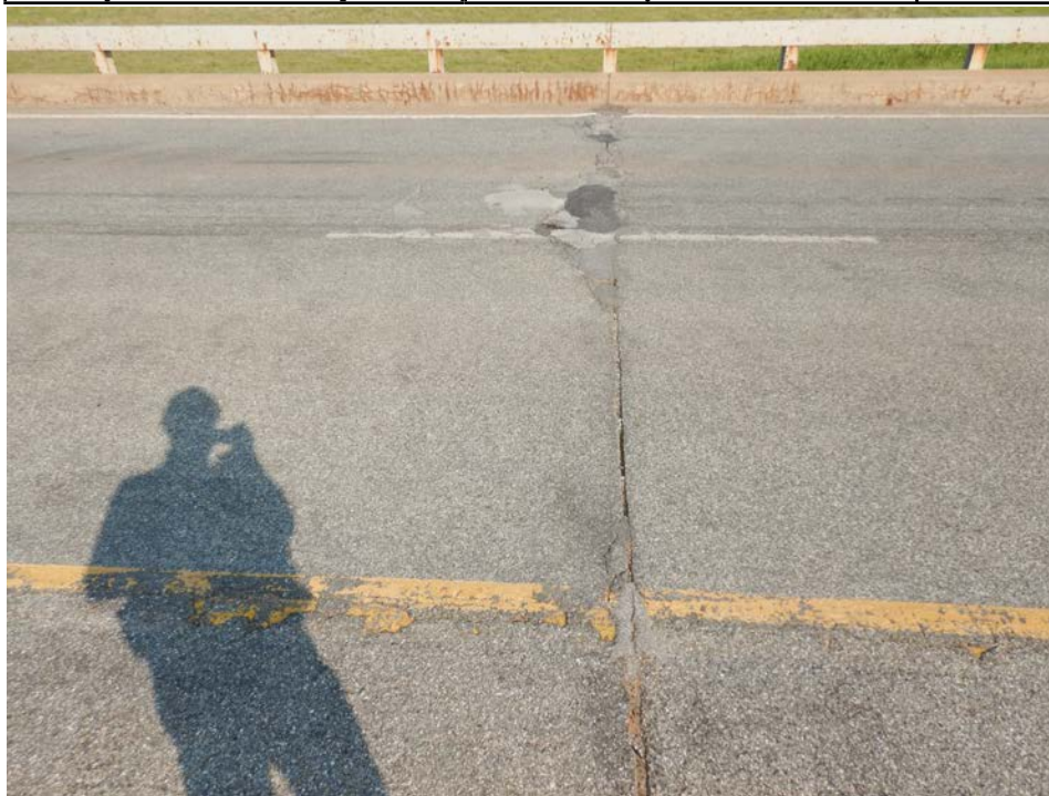
Photograph 21 - Looking west along the north deck control joint in span 4. Note: asphalt patches along the control joint.
