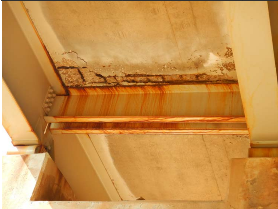
Photograph 12 - Looking south at the underside of span 2 at pier 1 between beams 1 and 2. Note: spall extending above the bottom reinforcing steel.
