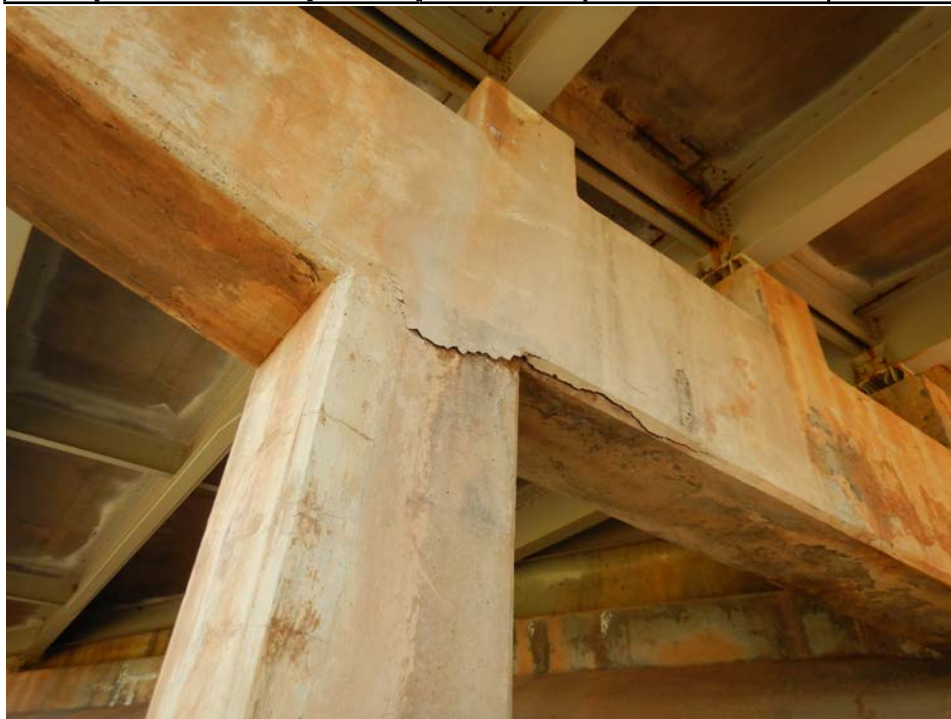
Photograph 42 - Looking northeast at pier 5 . Note: horizontal crack along bottom steel of cap with adjacent 2-foot by 5-foot delamination near column 1.
