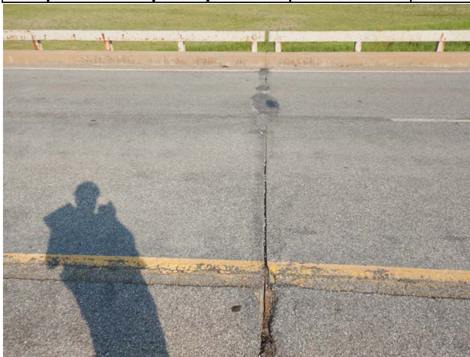
Photograph 19 - Looking west along the poured seal fixed joint over pier 5. Note: asphalt patches exist along the joint in the west lane.
