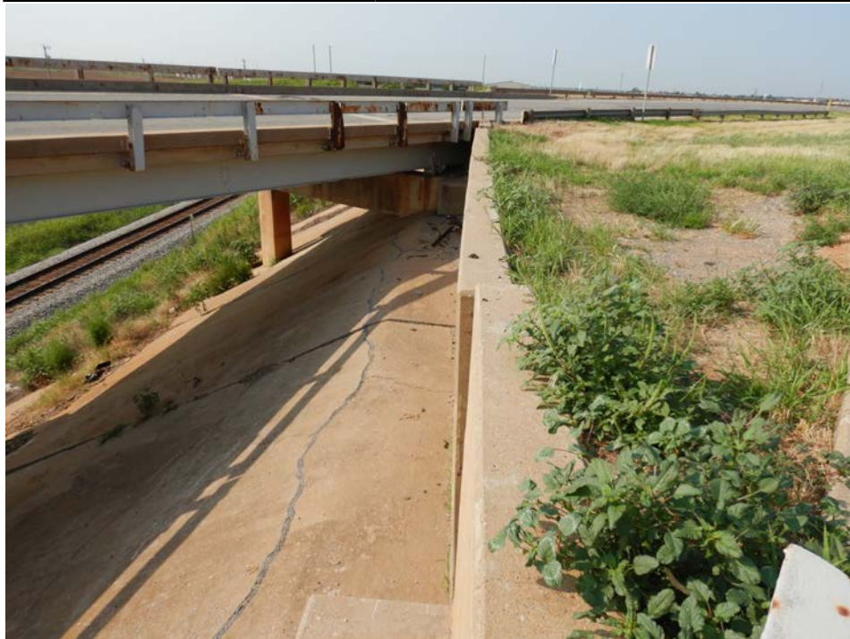
Photograph 34 - Looking southeast along the south retaining wall in the median. Note: wall is leaning 3 1/2 inches away from the embankment relative to the wingwall.
