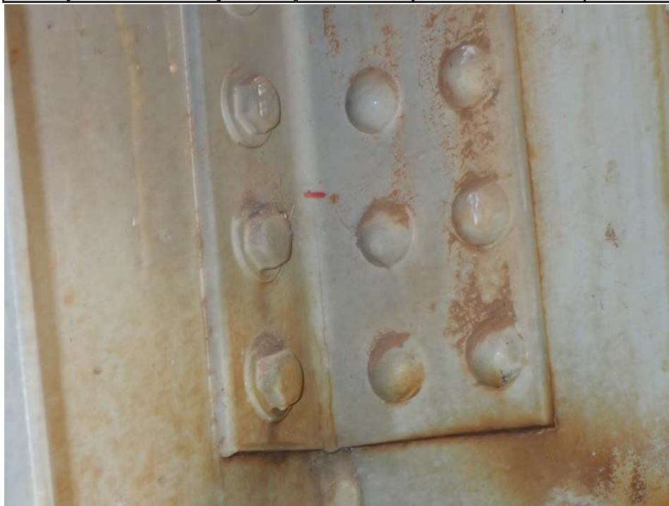
Photograph 22 - Looking northeast at the beam 4, span 3 southwest connection angle to the pier beam at pier 3. Note: 5 3/4-inch-long vertical paint crack at the bottom of the connection angle.
