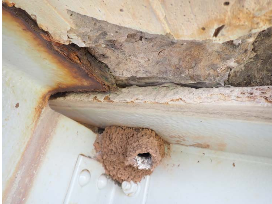
Photograph 27 - Looking southeast at the beam 1, span 4 top flange at the pier beam at pier 3. Note: laminating corrosion and 1/8-inch-deep section loss in the top flange of the beam. 16-inch-deep section loss to the top flange of the pier beam. Deck is lifted off the pier beam top flange.
