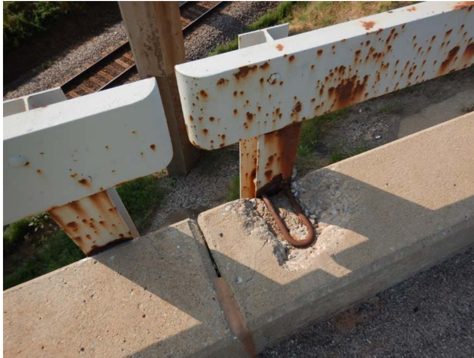
Photograph 7 - Looking east at the east curb in span 1 at pier 1. Note: spall in the top face of the curb exposing the U-bolt anchorage for the bridge railing post.
