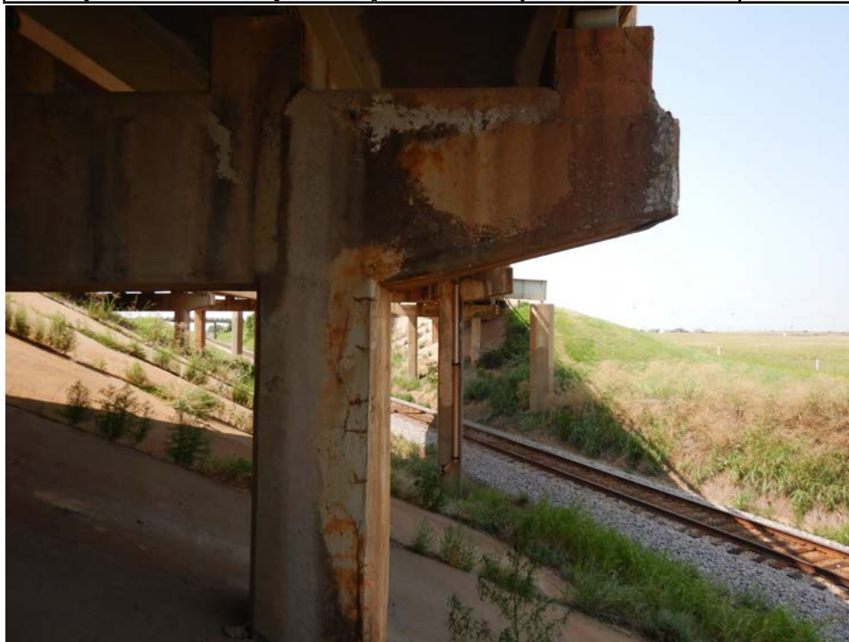
Photograph 40 - Looking south at the west end of the pier 5 cap. Note: vertical cracking up to 1/8 inch wide in column 1 in the west and north faces of the column.
