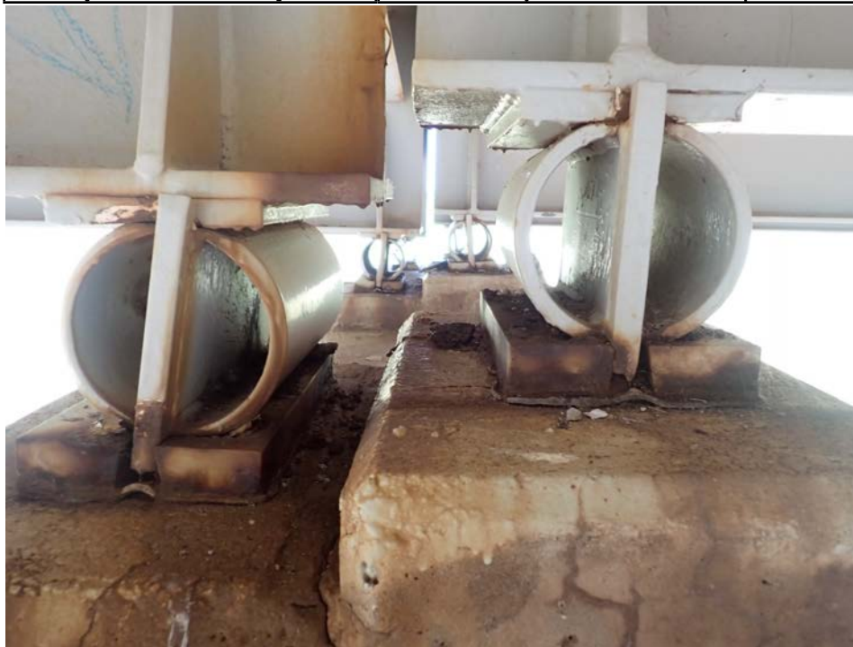
Photograph 49 - Looking west at the beam 3, canister bearings at pier 4. Note: the span 4 bearing is offset from the bearing stiffener and rotated in expansion. The span 5 bearing is aligned with the vertical stiffener and rotated in contraction. Canister thickness is worn at the point of contact with the
