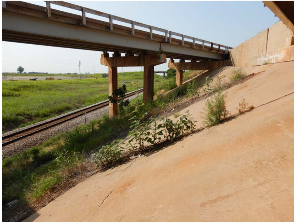
Photograph 35 - Looking southeast at the south slope wall. Note: vegetation growing in joints.
