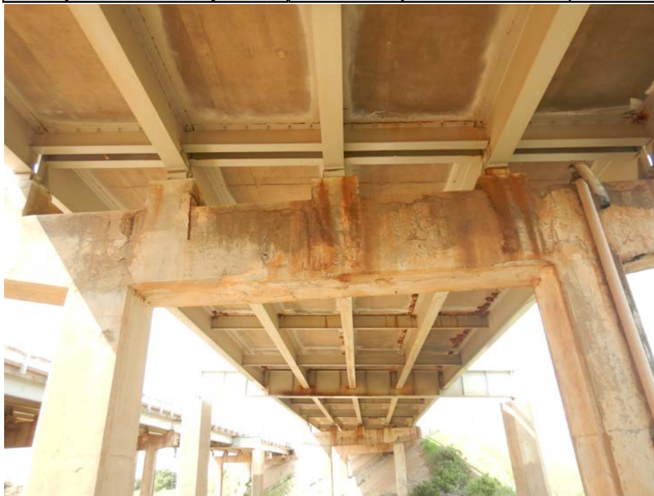
Photograph 39 - Looking south at pier 4. Note: cracking and spalling with exposed reinforcing steel in the beam 2 pedestal.
